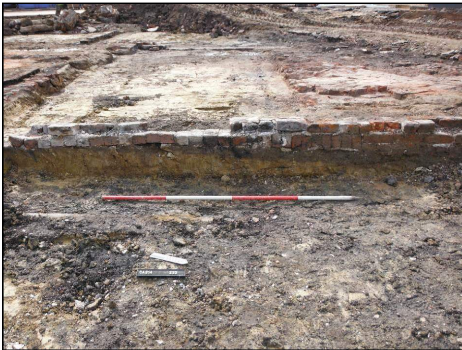
Figure 27- WSW facing shot of wall (233). Note poor construction and use of levelling clay (192) below the brickwork at the northern extent (Scale- 1 x 2m).
