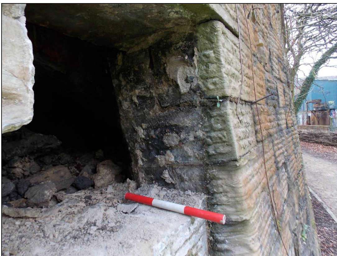
Figure 12: Detail of wall thickness of the lower Catacombs.
