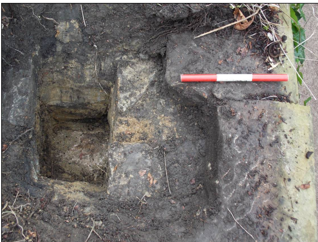
Figure 18: Detail of excavated area showing brick vault extrado .
