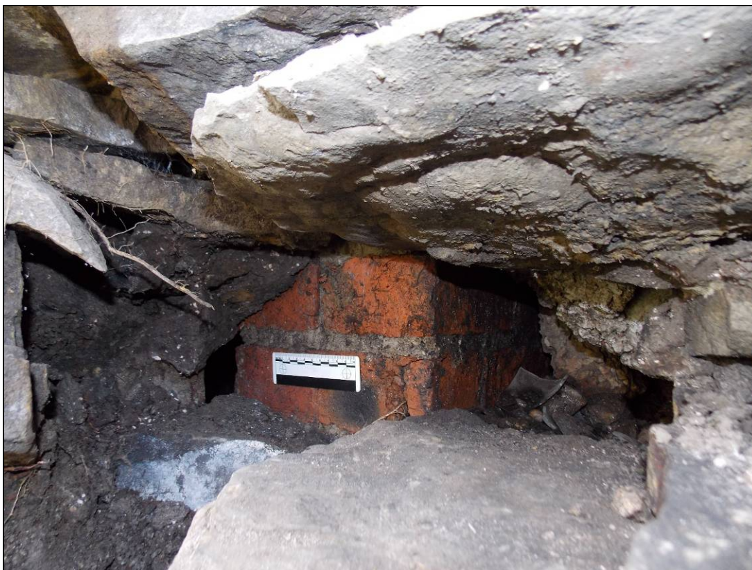
Figure 37: Brick wall abutting the rubble infill of the retaining wall.
