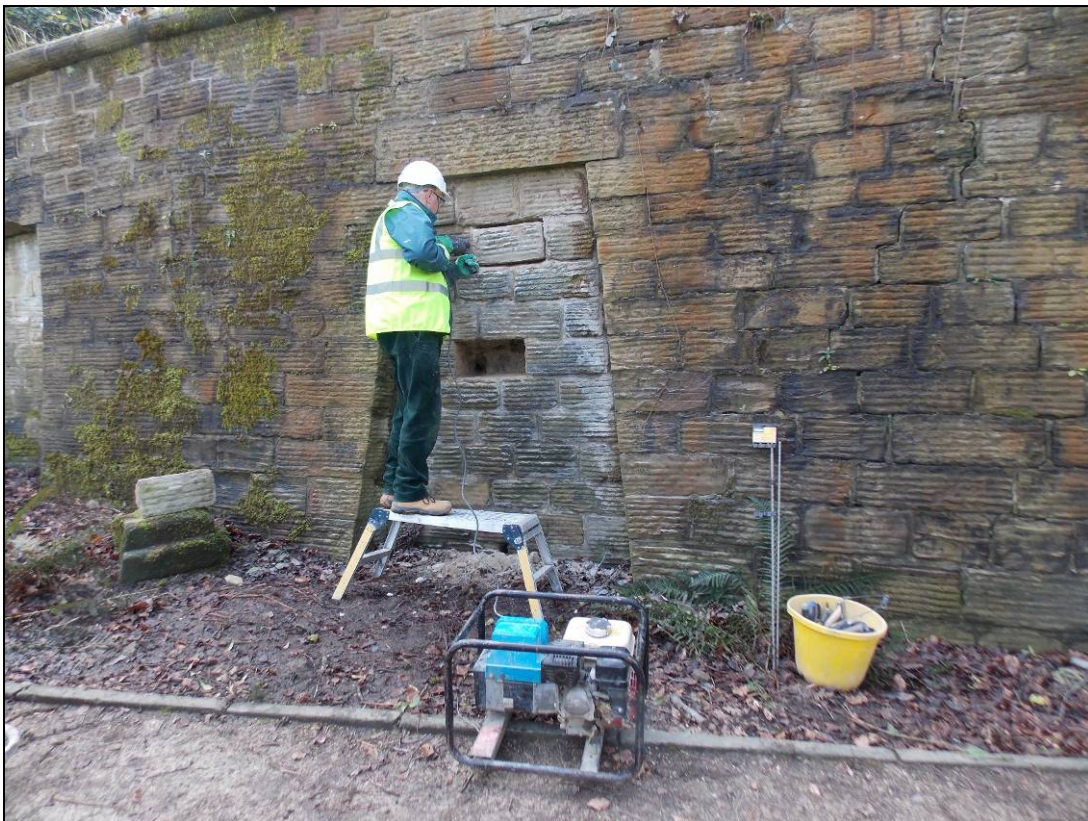
Figure 9: Inspection opening of Catacomb DD.
