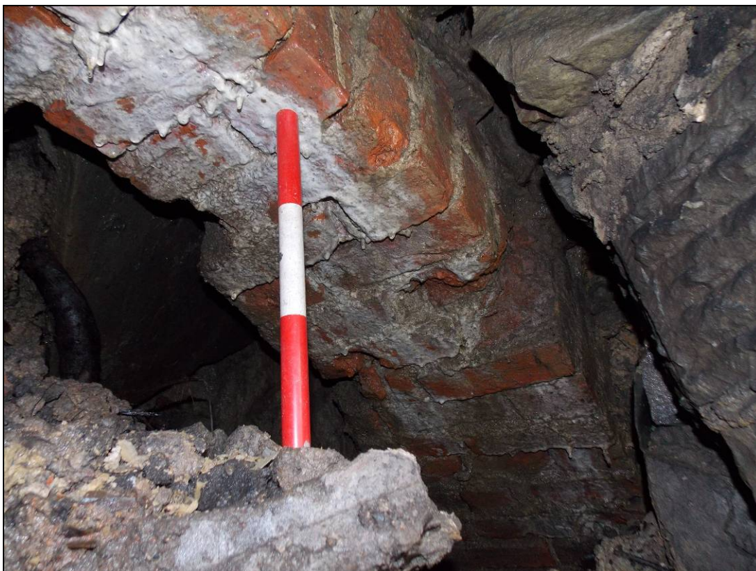
Figure 13: Brick barrel vaulted chamber.
