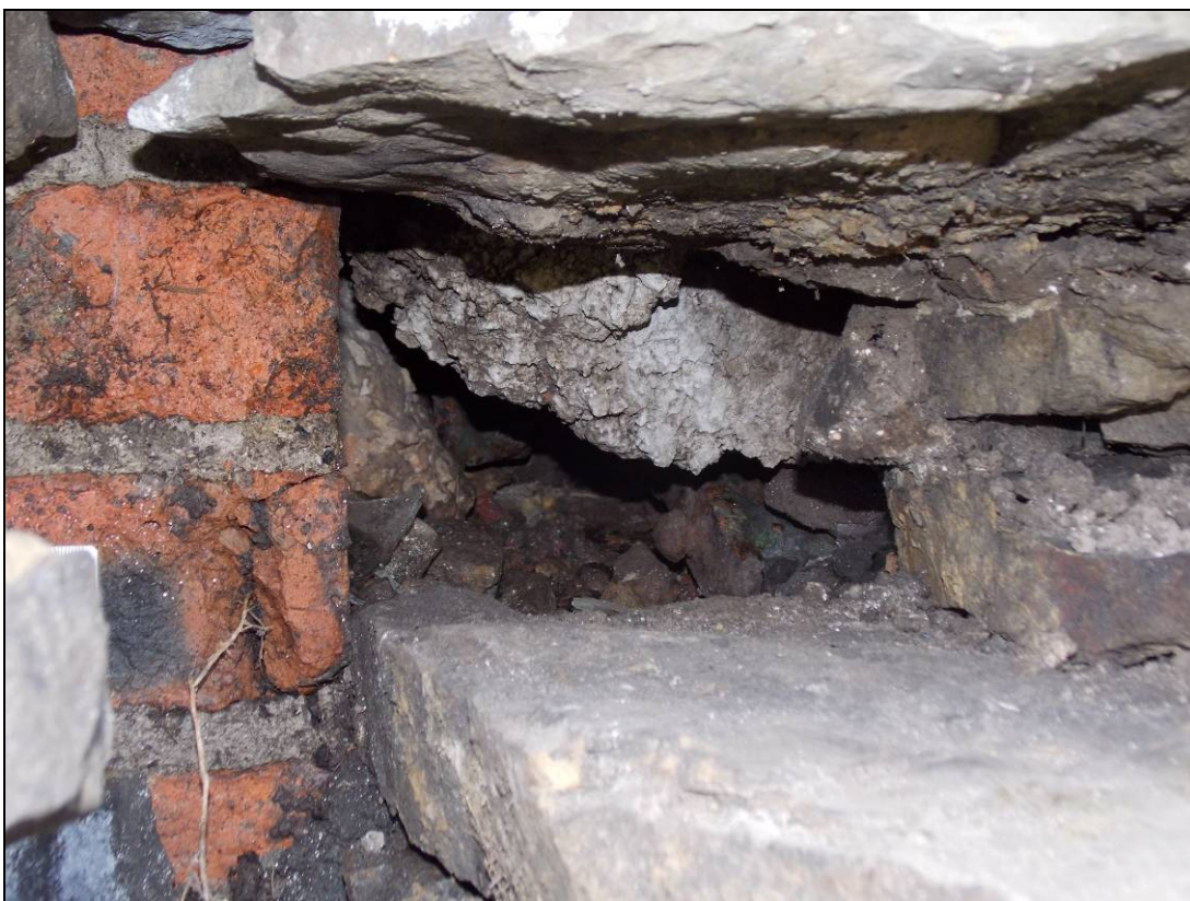
Figure 40: Basal section of adjacent concrete structure with metal and glass aggregate/packing.
