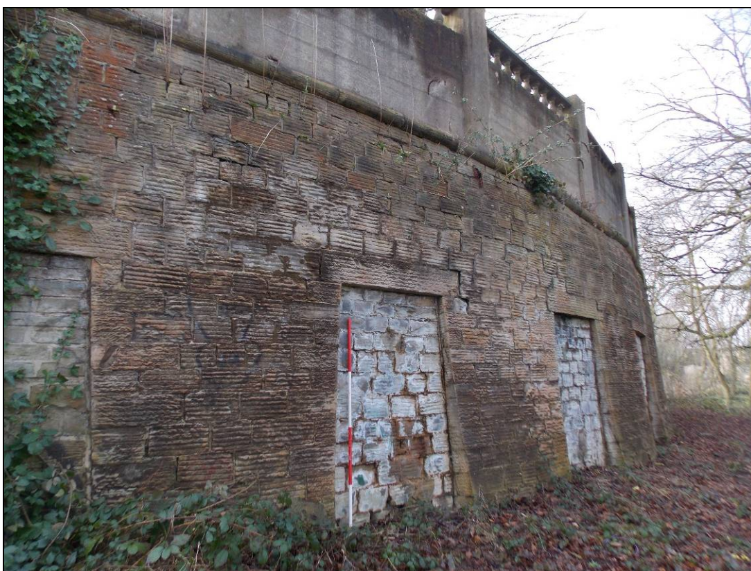
Figure 24: Doorway of Catacomb D within the upper level.
