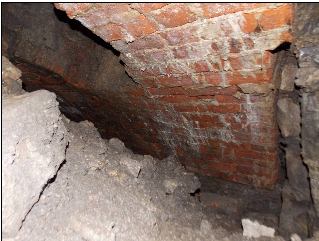
Figure 15: Brick barrel vault springing from a stone cross wall.
