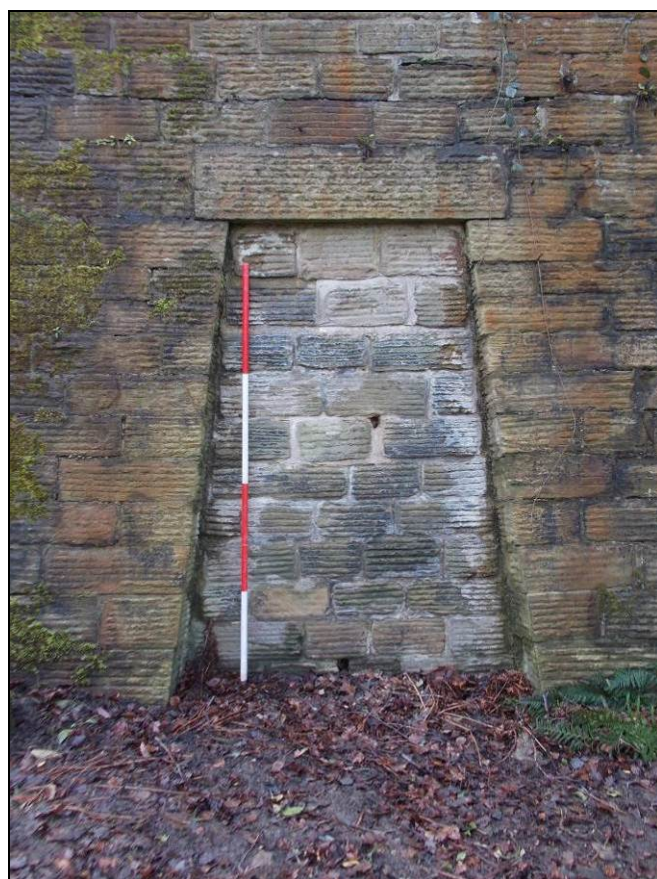
Figure 8: Detail of blocked-up doorway of Catacomb DD.
