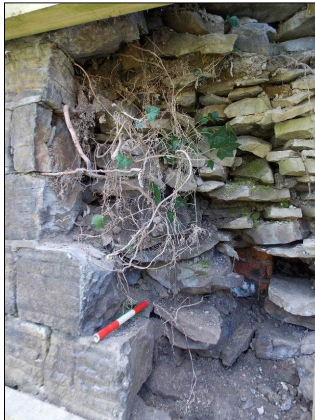
Figure 36: Inspection hole through the exposed rubble infill.
