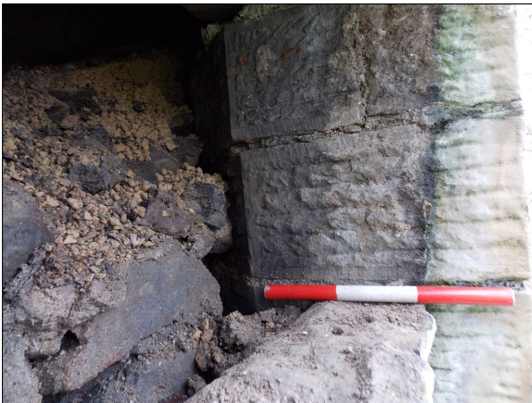
Figure 31: Original doorway jamb with internal splayed edges.
