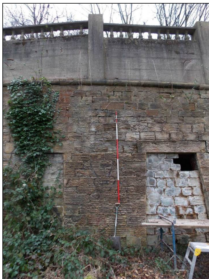
Figure 26: Inspection hole within the blocked-up doorway of Catacomb D.
