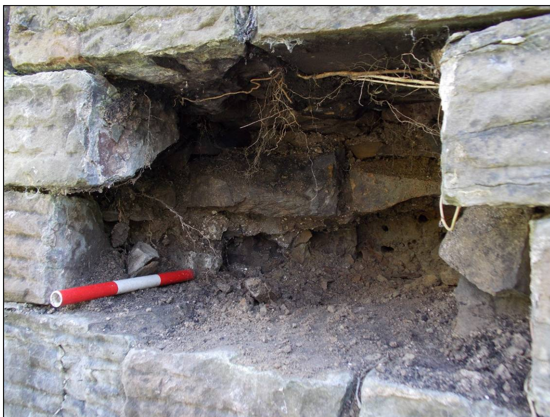
Figure 46: Detail of trial hole.
