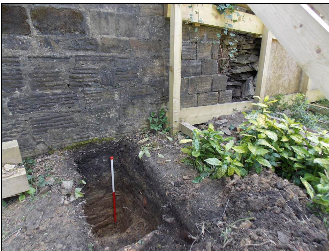
Figure 42: Test pit adjacent to the partially demolished retaining wall of the upper level.
