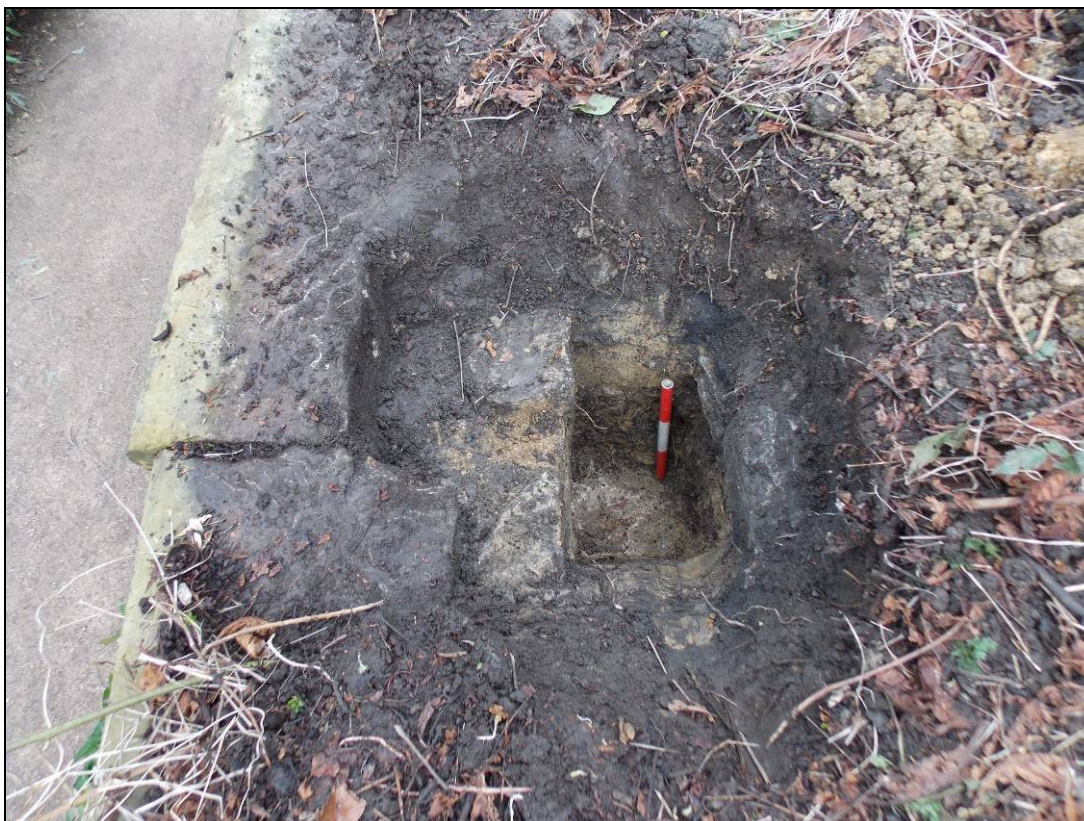
Figure 17: Excavation over the brick vault.
