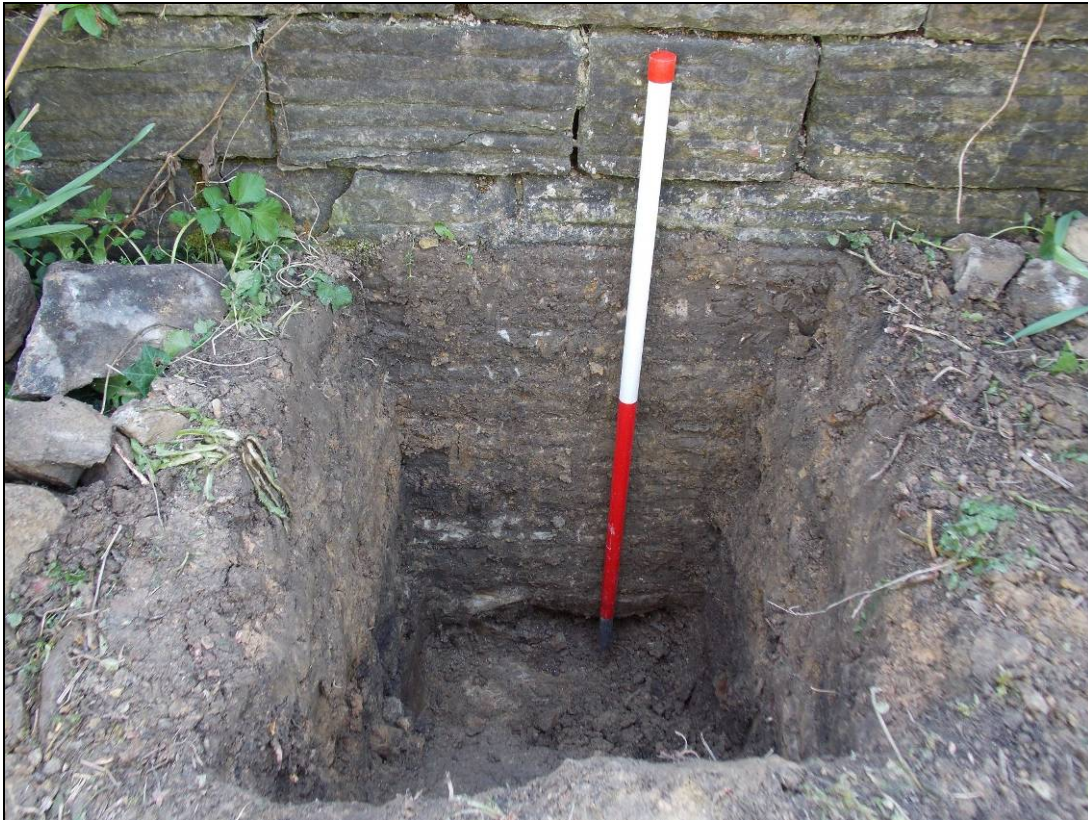
Figure 47: Detail of test pit showing the wall over the natural bedrock.
