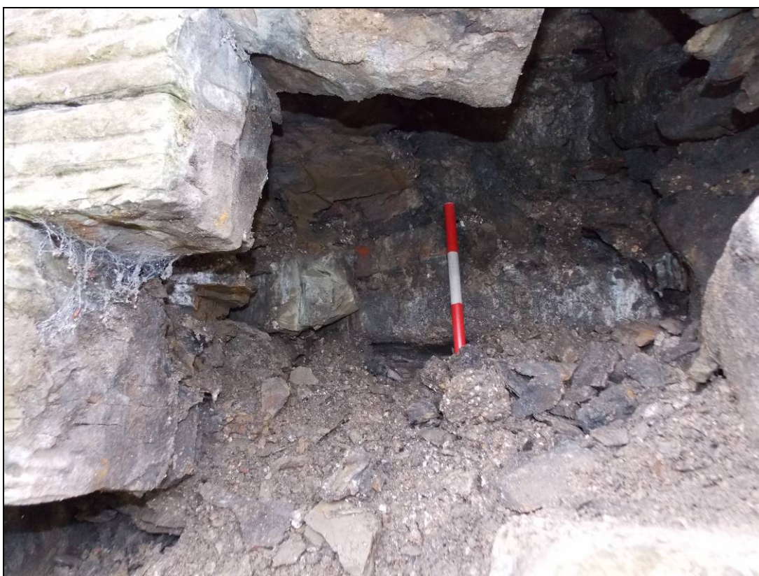
Figure 22: Internal view showing the external masonry, rubble infill and masonry of the Catacomb inside.
