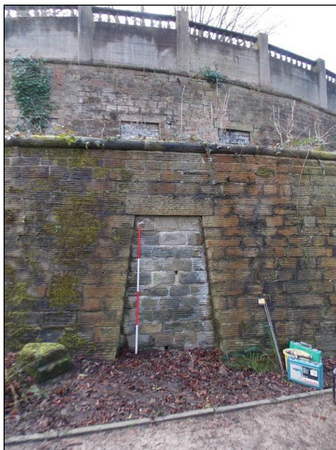
Figure 7: Catacomb DD within the lower level.
