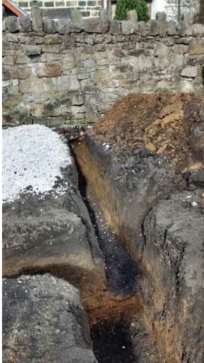
Figure 7. Service trench facing north. Scale = 0.3m.
