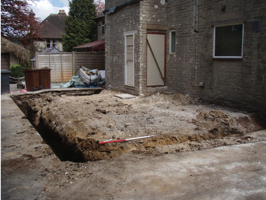
Figure 5. The excavation facing south. Scale 1m.
