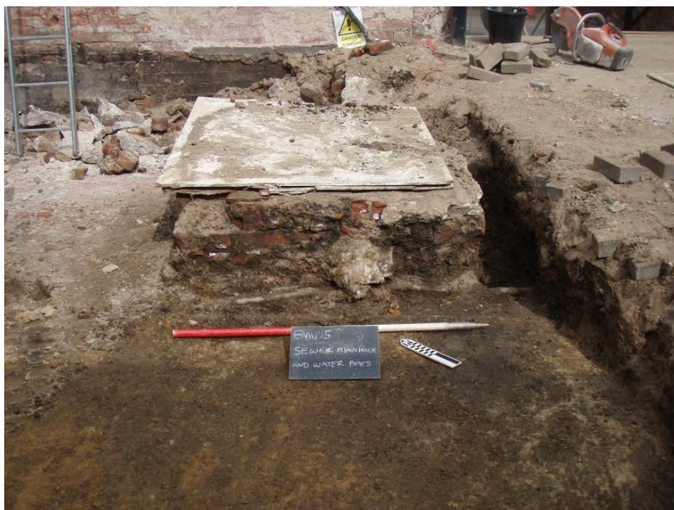
Figure 13. The manhole for sewer maintenance, post-excitation to a depth of 0.5m. The manhole was left in-situ , along with the water pipes visible just to the fore of the manhole.
