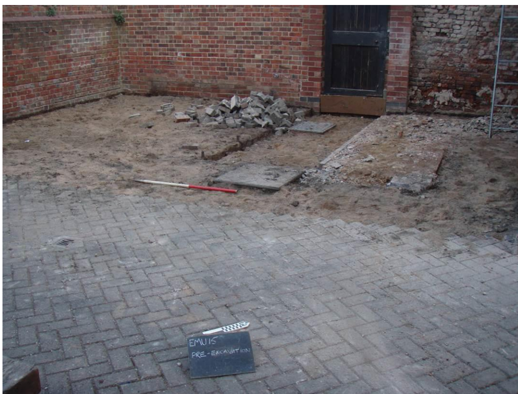
Figure 11. Pre-excitation photograph facing north-west showing manhole locations and brick boundary walls of a modern path leading to the wooden door. Scale 1m.
