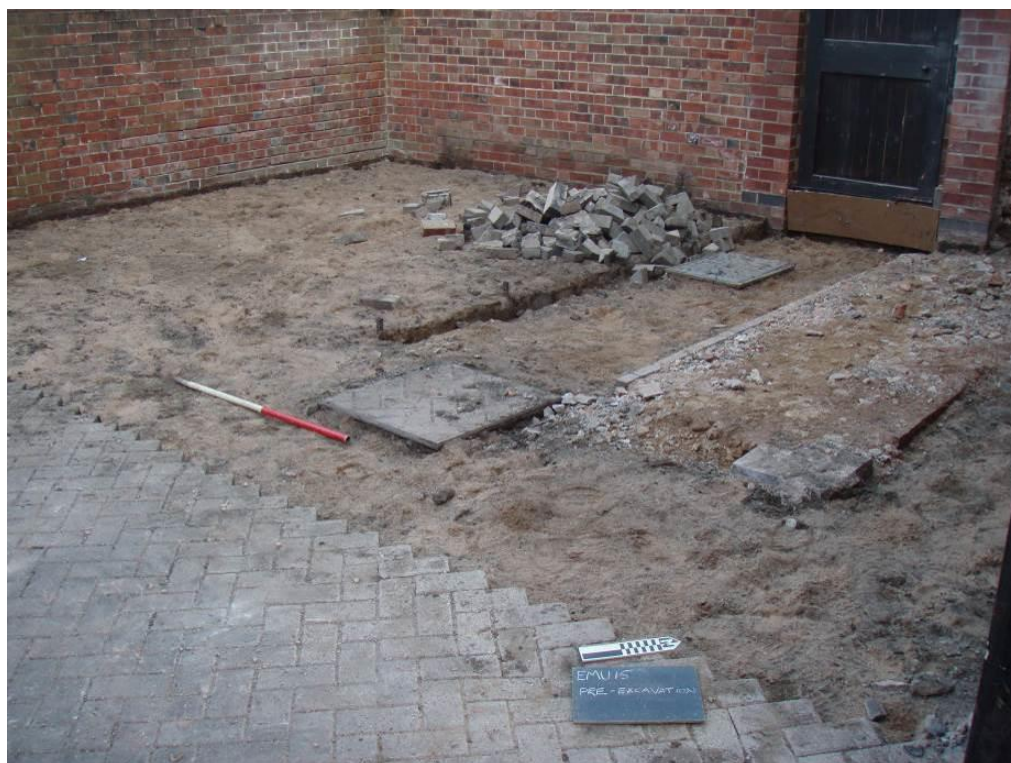
Figure 3. Pre-excitation photograph showing the excavation area facing west. The herringbone paving bricks were removed prior to excavation, exposing the levelling sand deposit (101), and manhole covers. To the right is the base of a brick staircase which was also removed prior to excavation. Scale 1m.
