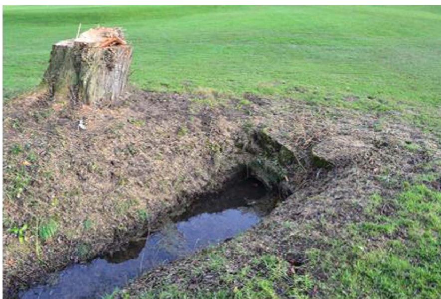
Figure 9: View E at pipe draining into lake from Moor Road
