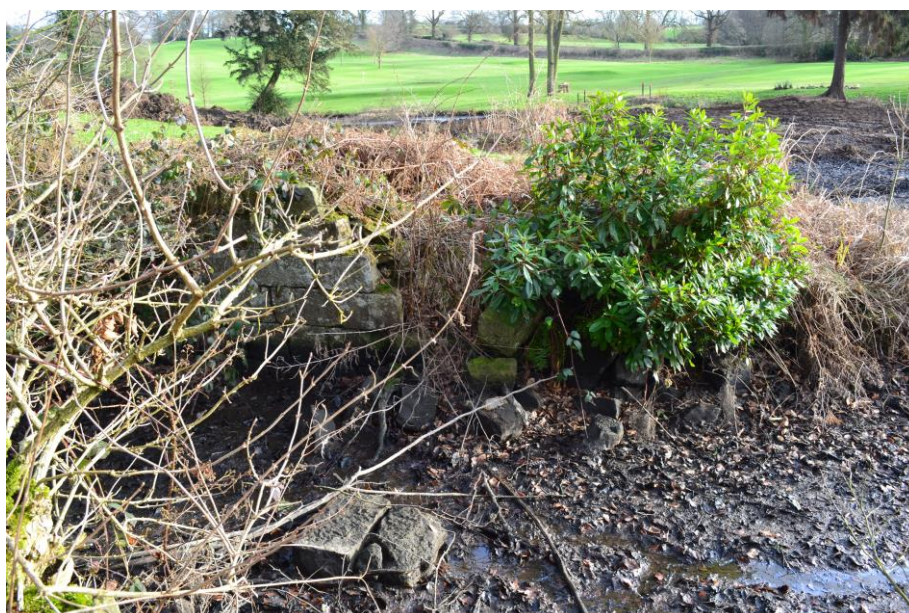
Figure 11: View E of foundations of boathouse
