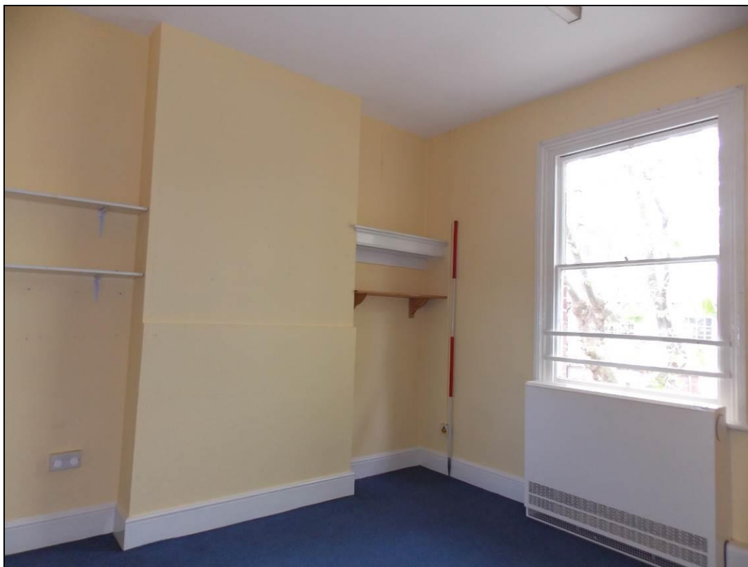
Figure 39: South-eastern Class Room of the first floor with original chimney breast.
