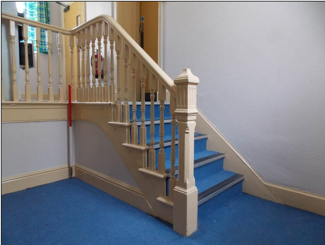
Figure 41: Detail of newell post, open-string and turned balusters.
