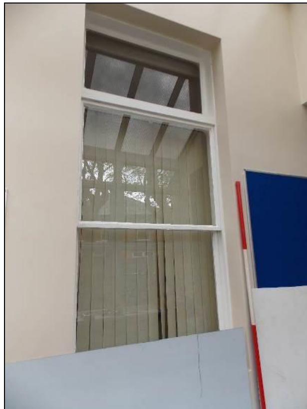
Figure 24: Detail of tall sash window.
