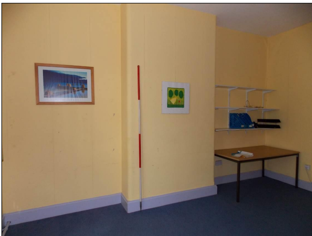
Figure 47: Managers Office with original chimney breast.
