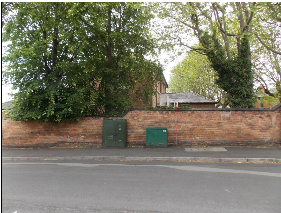
Figure 21: Boundary wall along Handford Street.
