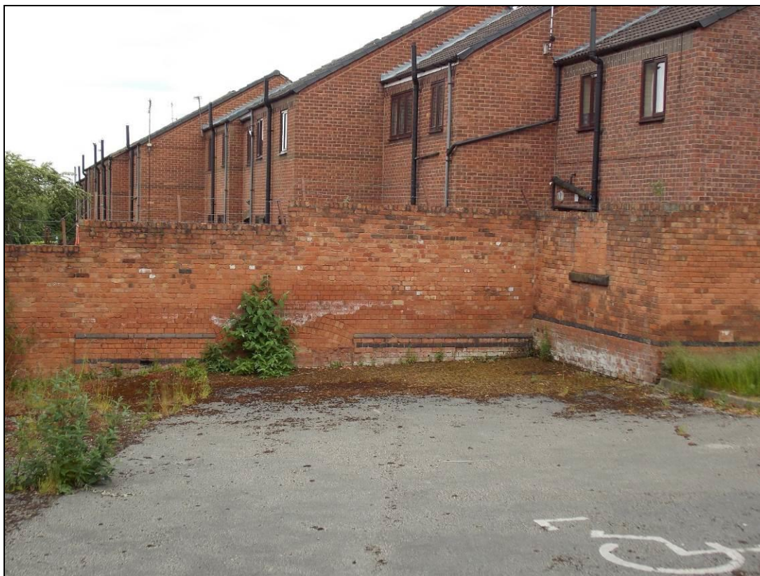
Figure 19: Boundary wall of the car park composed of former structural remains.
