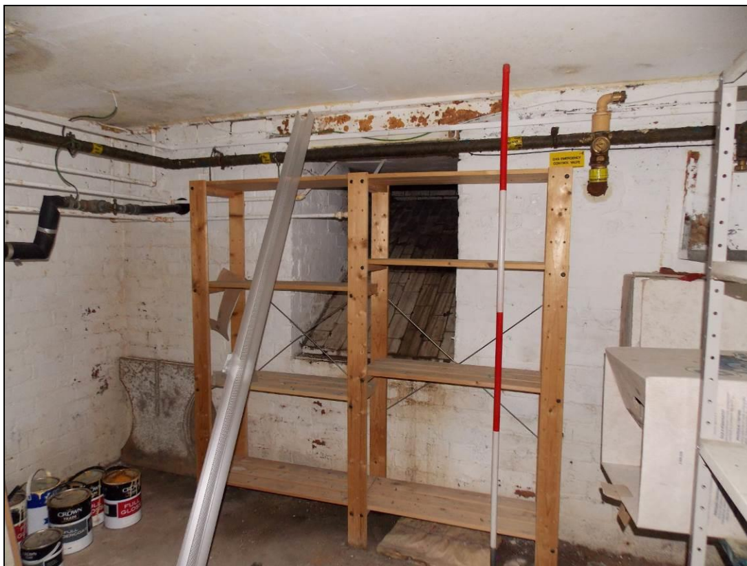
Figure 37: Coal chute within the southern wall of the cellar.
