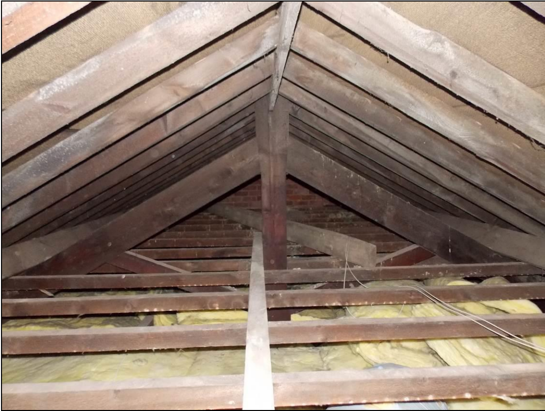
Figure 45: King-post truss over the Staff Room.
