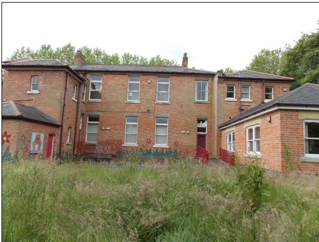
Figure 17: General view of the north elevation with projecting cross-wings.
