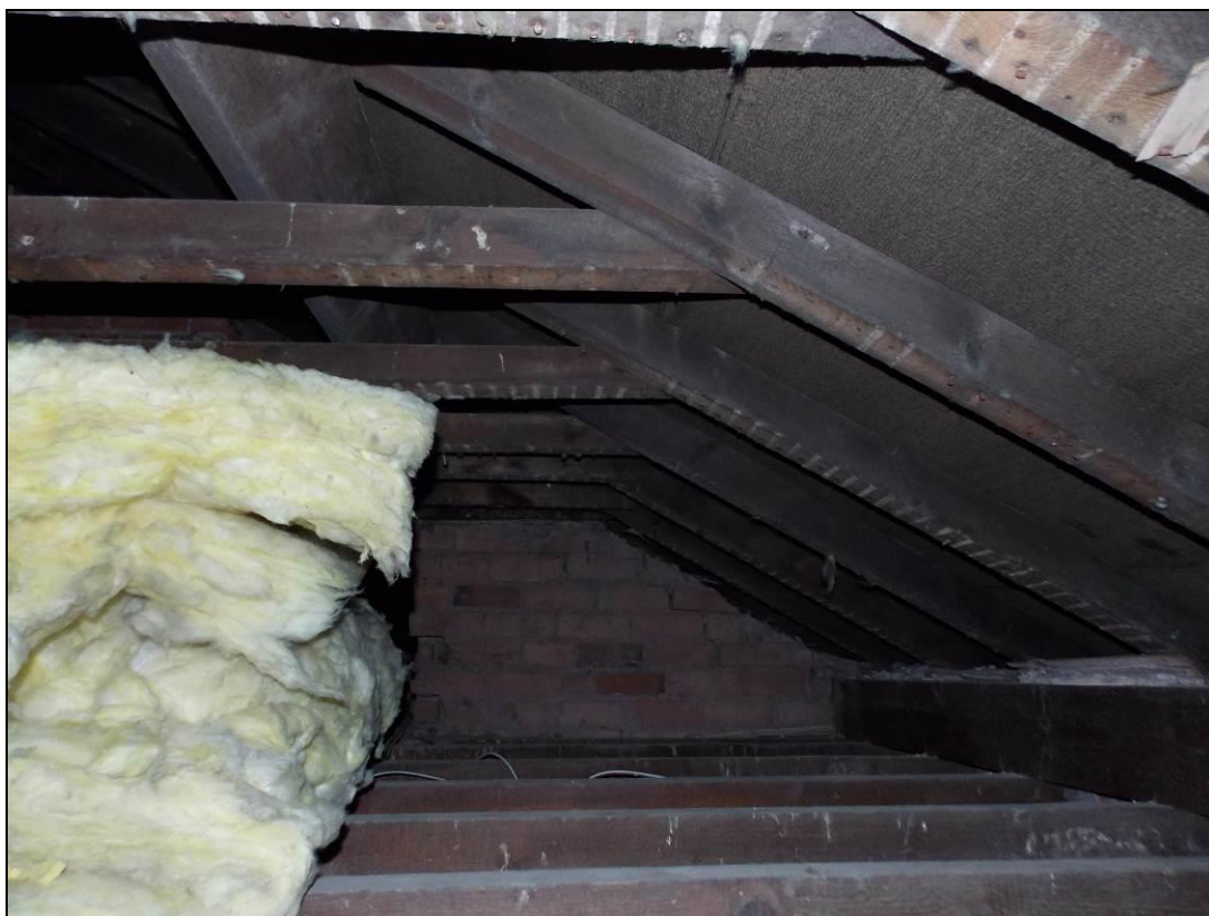
Figure 44: Roof structure over the Staff Room.
