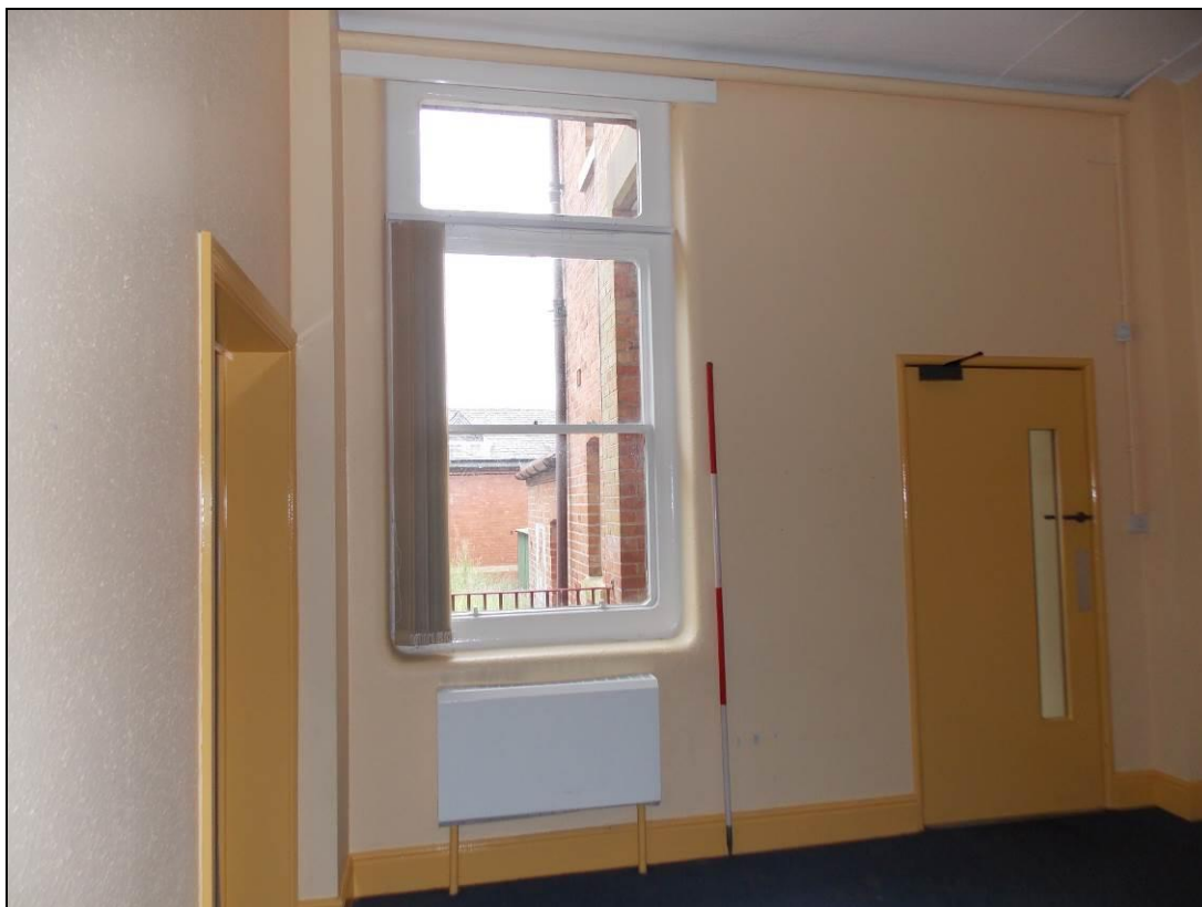
Figure 29: Detail of window within the central Class Room.
