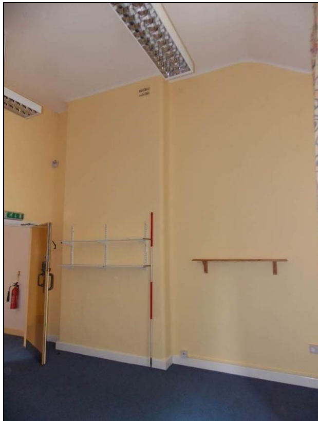
Figure 46: Central Class Room with original chimney breast.
