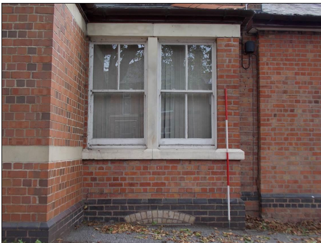
Figure 14: Detail of arched head of a former coal chute.
