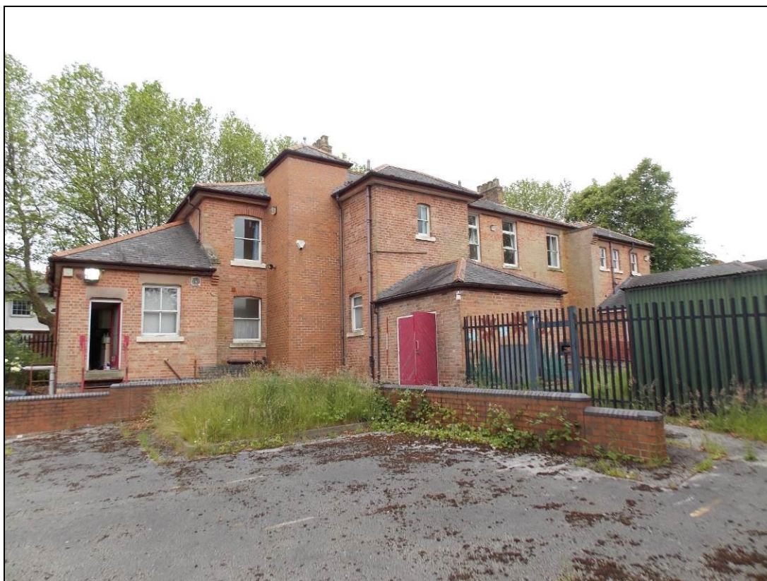
Figure 18: North elevation viewed from the north-western car park.
