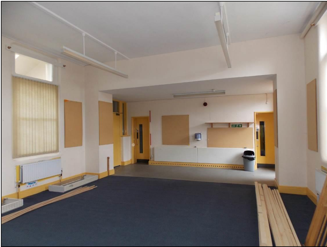
Figure 31: Main Play Room with western wall partially removed.
