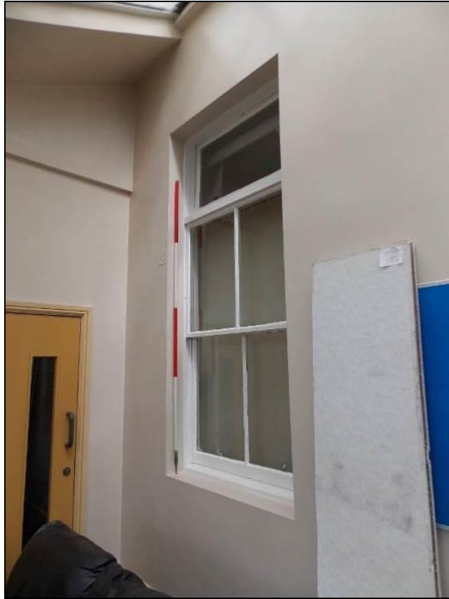
Figure 23: Detail of short sash window.
