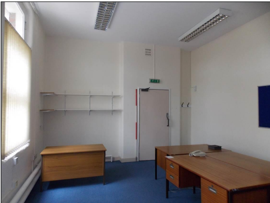
Figure 42: Staff Room with inserted doorway within an original chimney breast.
