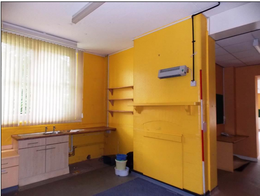
Figure 32: Kitchen with original chimney breast.
