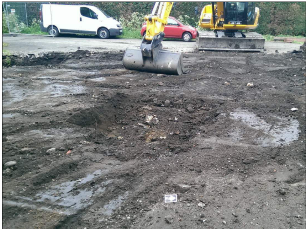
Figure 32: Area 3 Following ground reduction, showing context (001) looking west.
