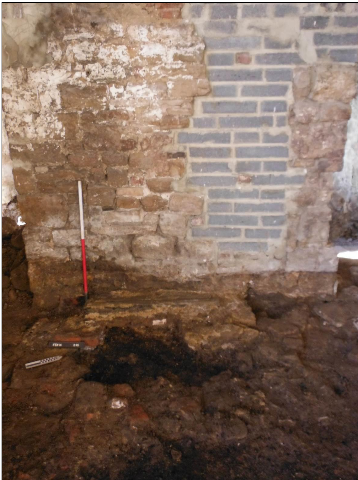
Figure 44- W-facing view of fireplace (616/617) blocked by late 19 th -20 th century remodeling (Scale- 1 x 1m).
