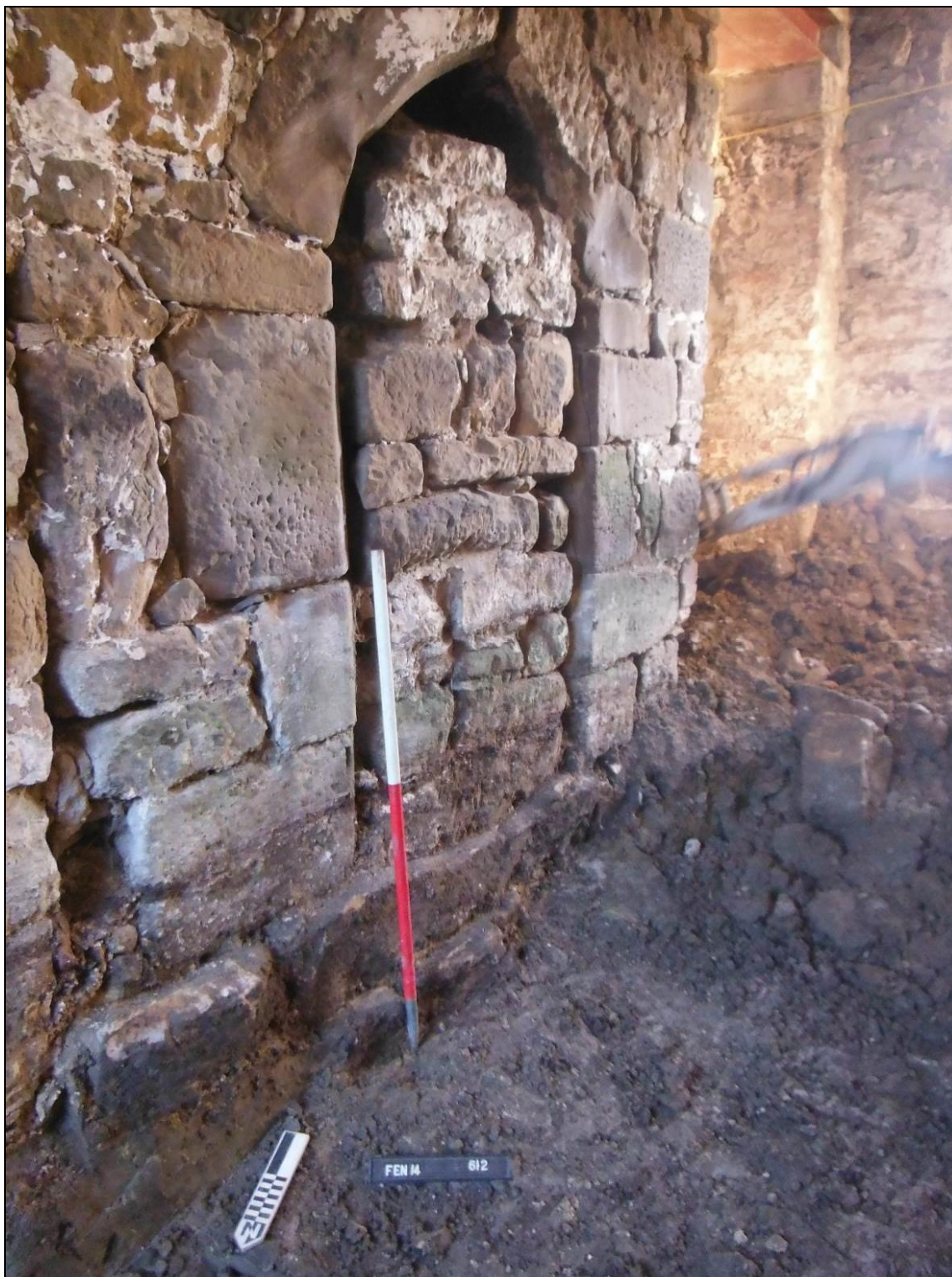
Figure 41- S-facing oblique view of wall (613) and the blocked 16 th -17 th century byre doorway (Scale- 1 x 1m)
