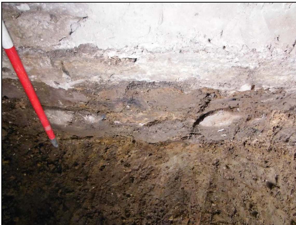
Figure 37- Pre-excitation view of foundation trench F.634 for north wall of the bastle (647) (Scale-1 x 1m)
