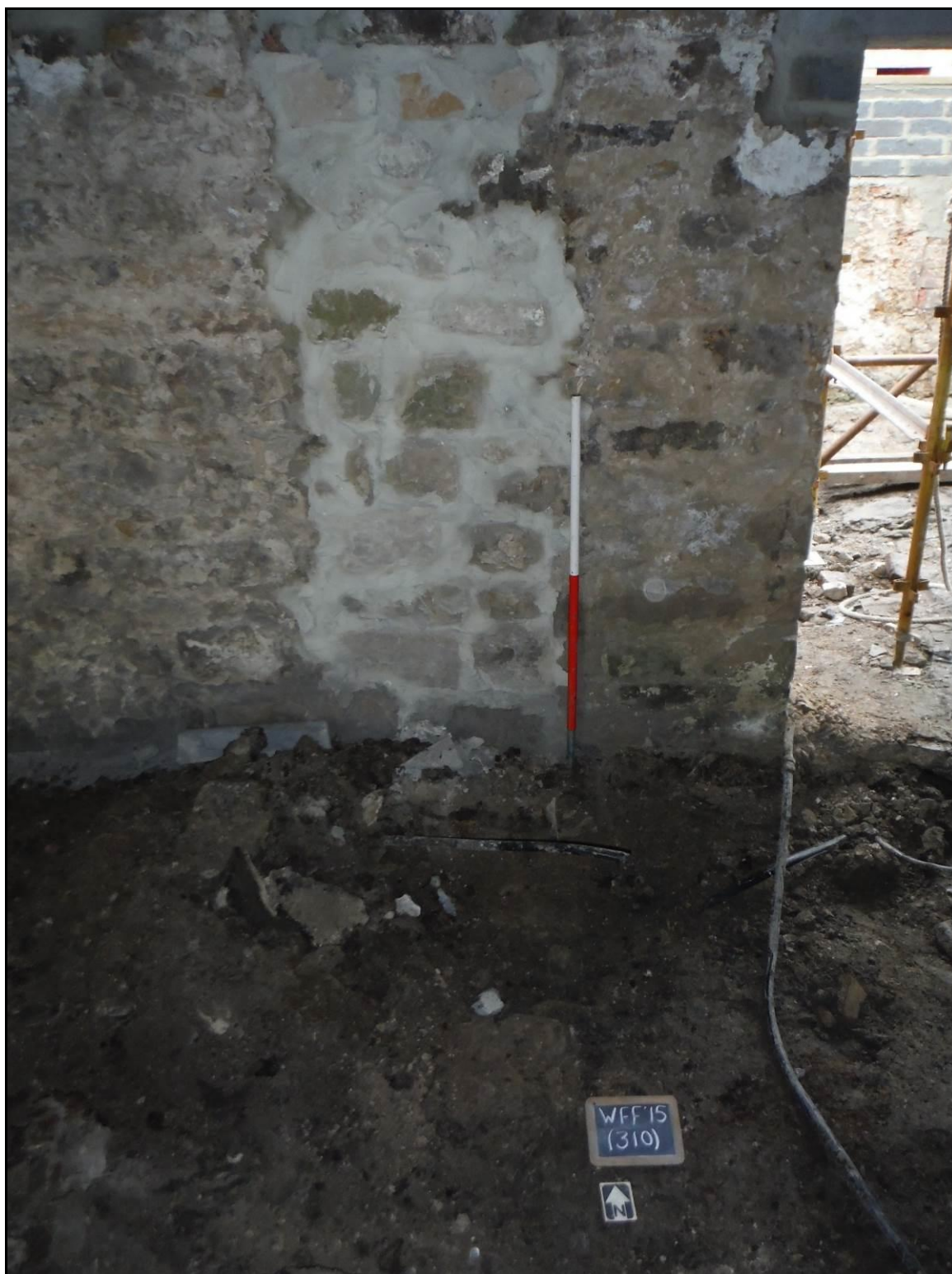
Figure 31- N-facing view of wall foundation (310) in relation to the construction scar in the south facing wall of Building 6 (Scale- 1 x 1m)
