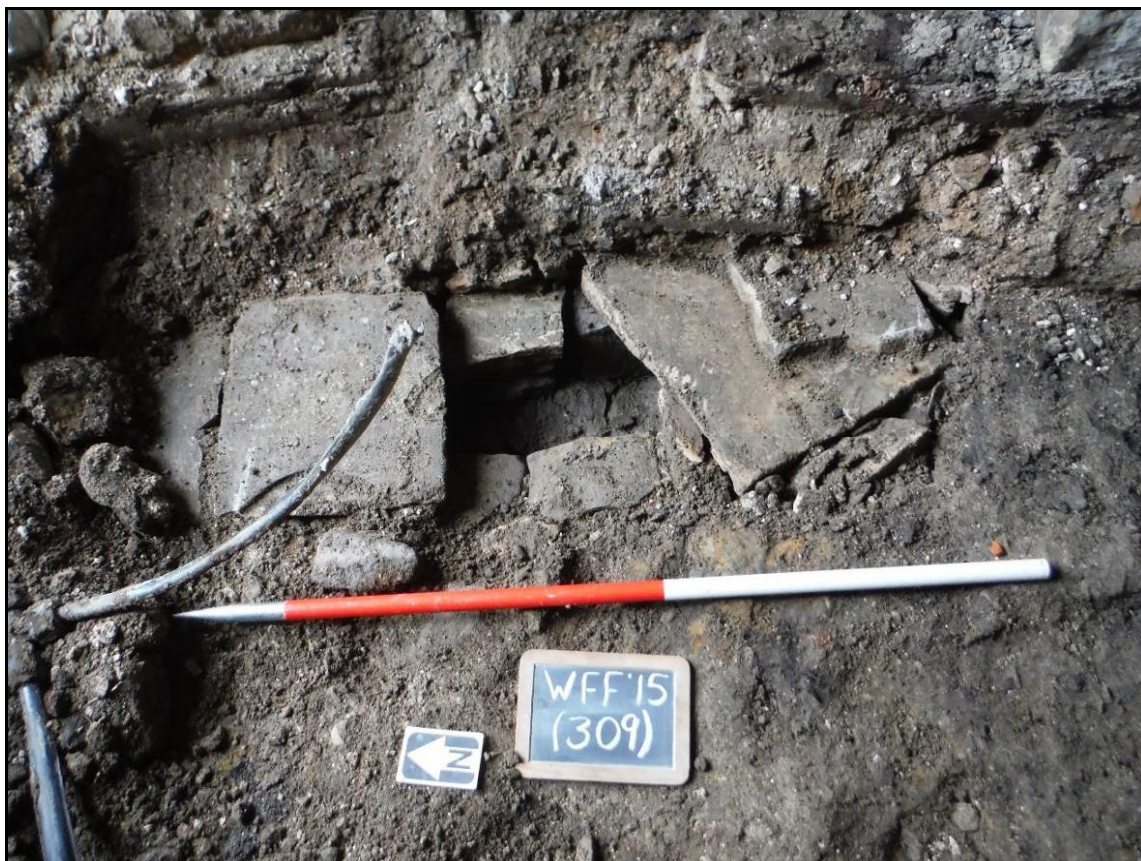
Figure 29- E-facing view of F.313 displaying interior culvert structure (Scale- 1 x 1m)
