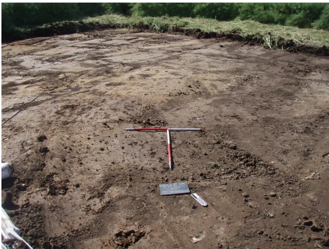
Figure 6. View of stripped area for crane hard standing area.
