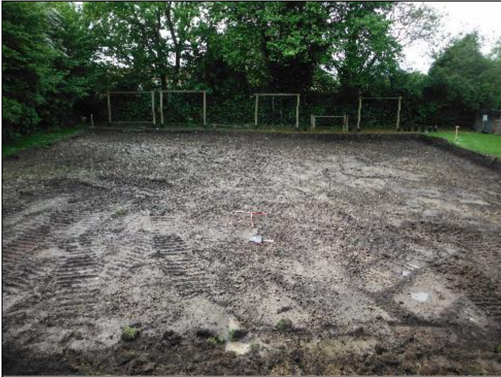
Figure 4. Trench 1. West facing. Scale = 2x1m.
