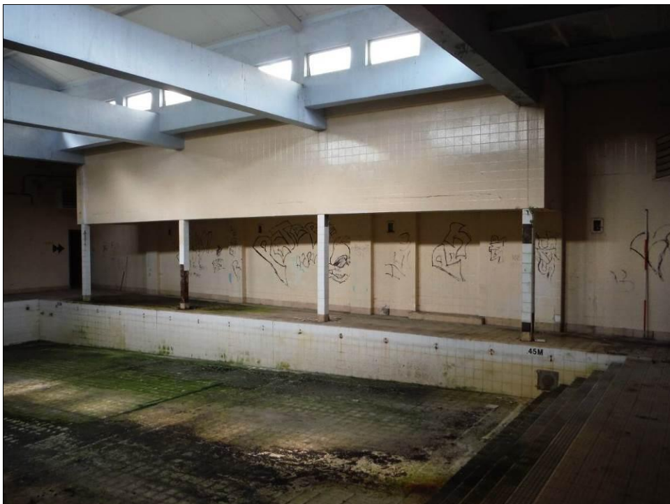
Figure 97: North wall of Room G12, Building B (Scale = 2m).
