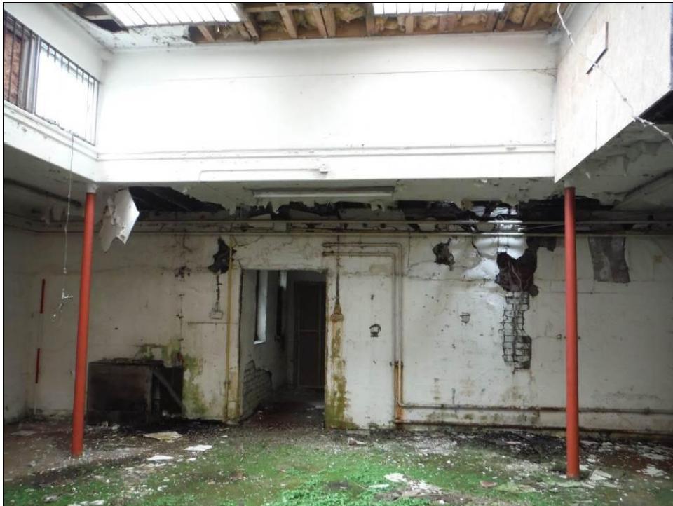
Figure 44: West wall of Room G5, Building A (Scale = 2m).
