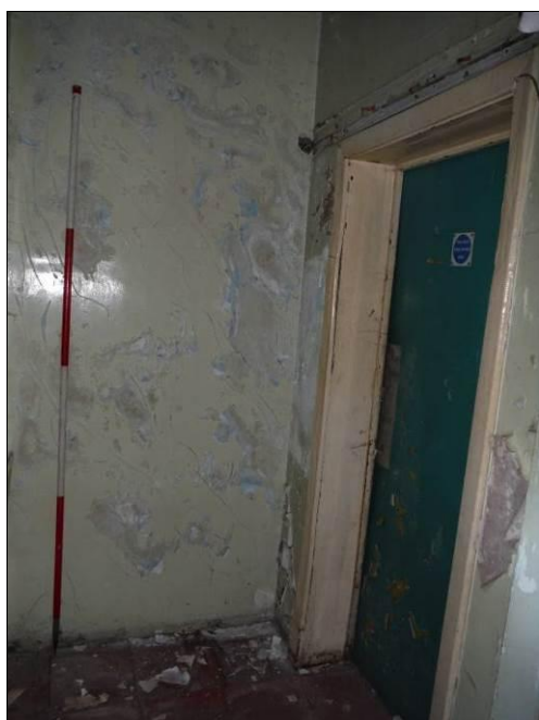
Figure 88: Room G7, Building B (Scale = 2m).
