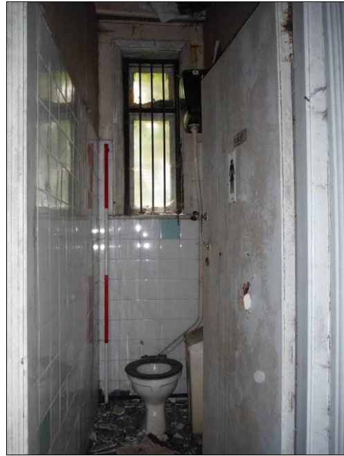
Figure 52: Room G10, Building A (Scale = 2m).
