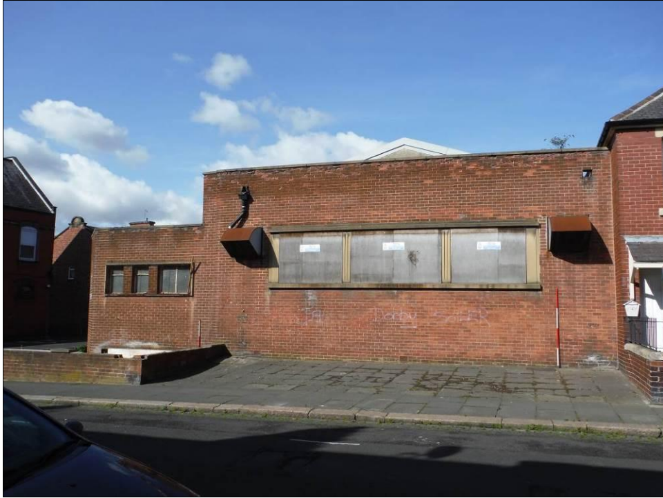
Figure 70: North East elevation of Building B (Scale = 2 x 2m).
