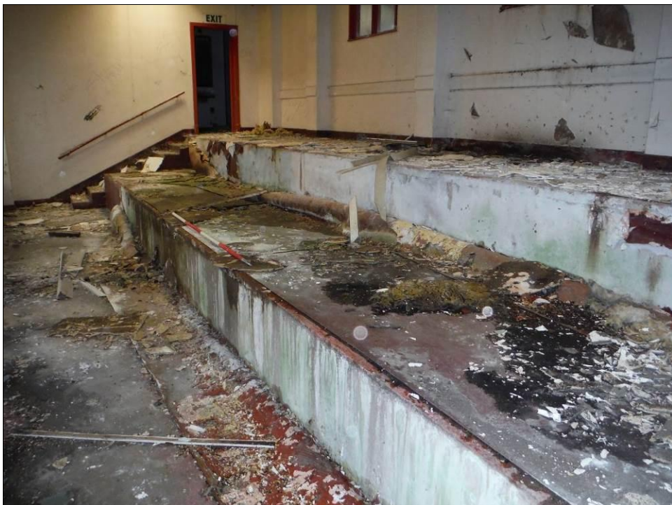
Figure 131: Detail of tiered seating in Room F6, Building B (Scale = 2m).
