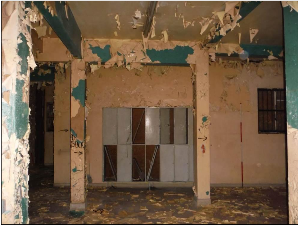
Figure 77: North wall of Room G3, Building B (Scale = 2m).
