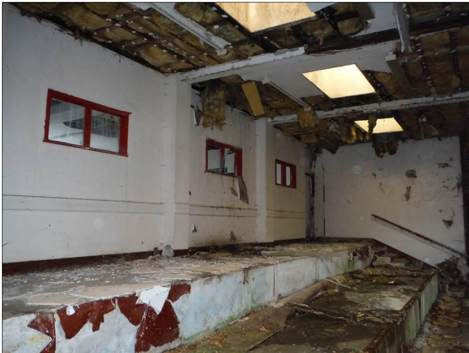
Figure 129: East and south wall of Room F6, Building B (Scale = 2m).
