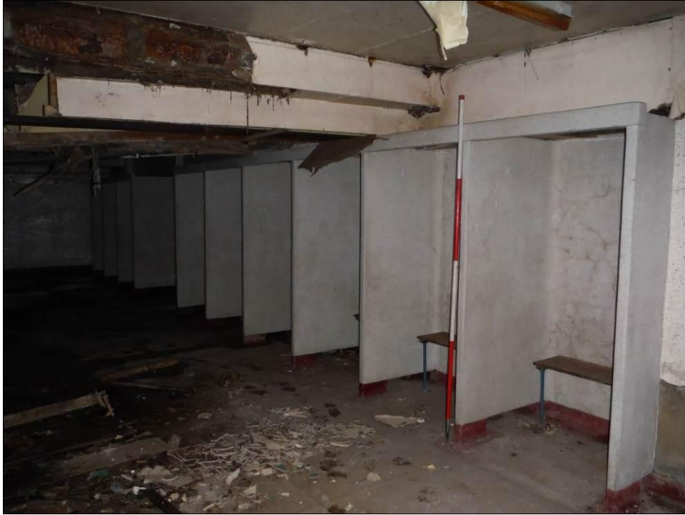
Figure 106: South and west walls of Room B5, Building B (Scale = 2m).
