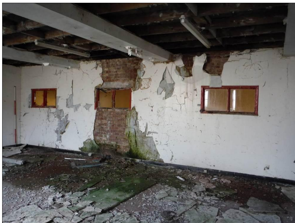
Figure 123: West wall of Room F4, Building B (Scale = 2m).
