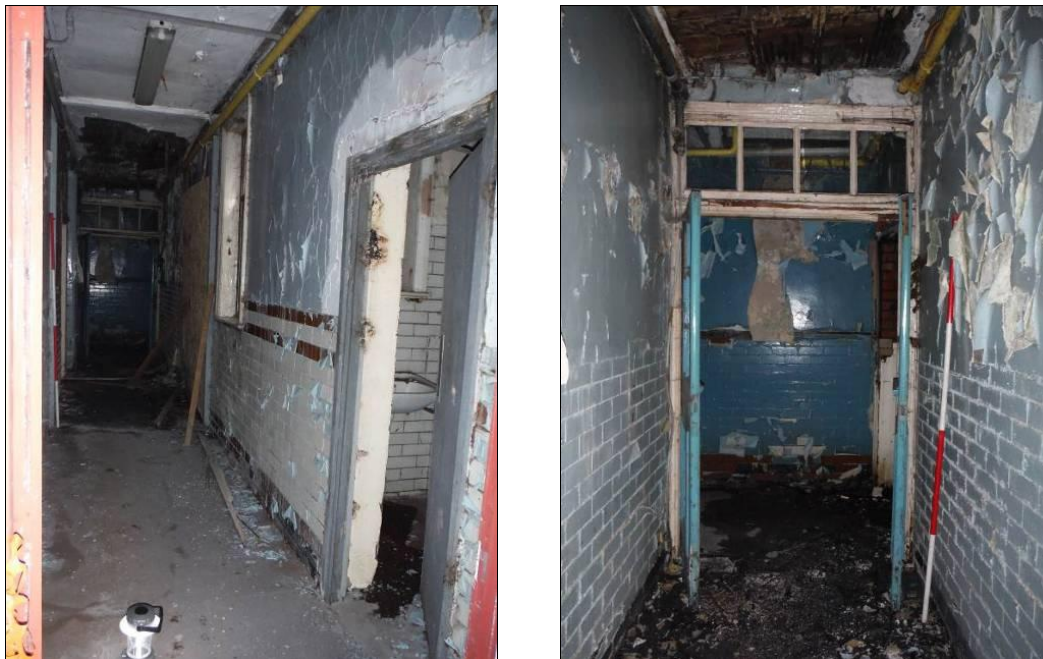
Figure 39: North facing views of Room G3, Building A (Scale = 2m).
