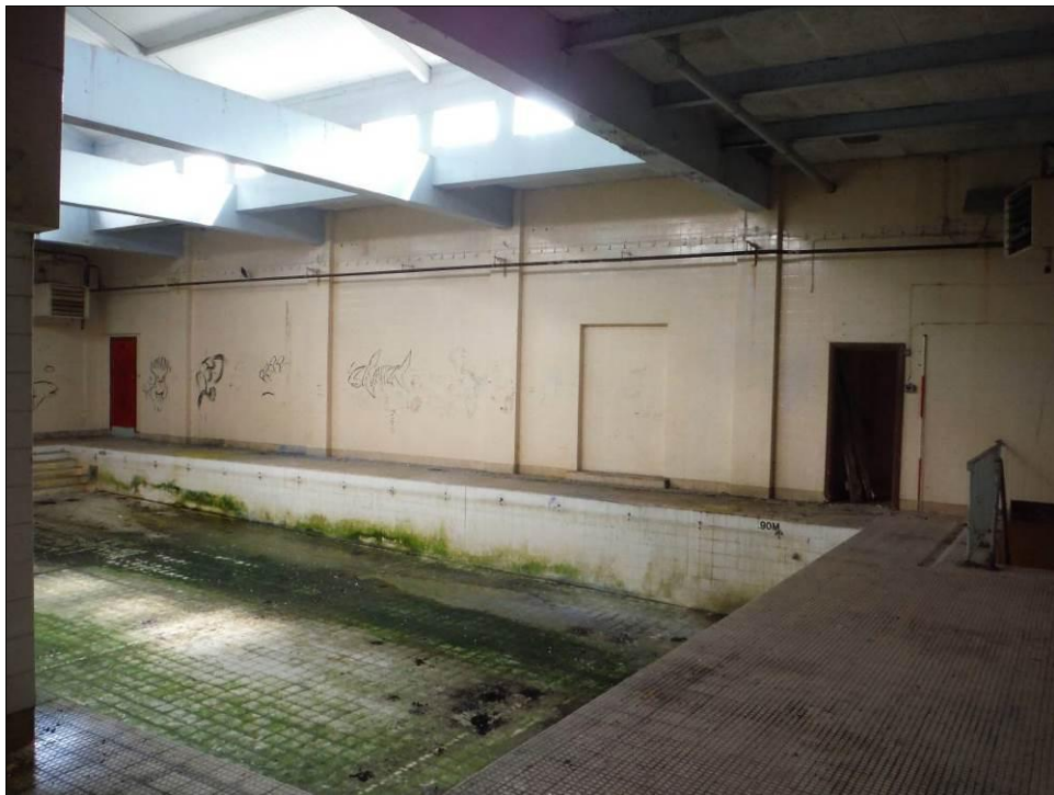
Figure 95: South wall of Room G12, Building B (Scale = 2m).
