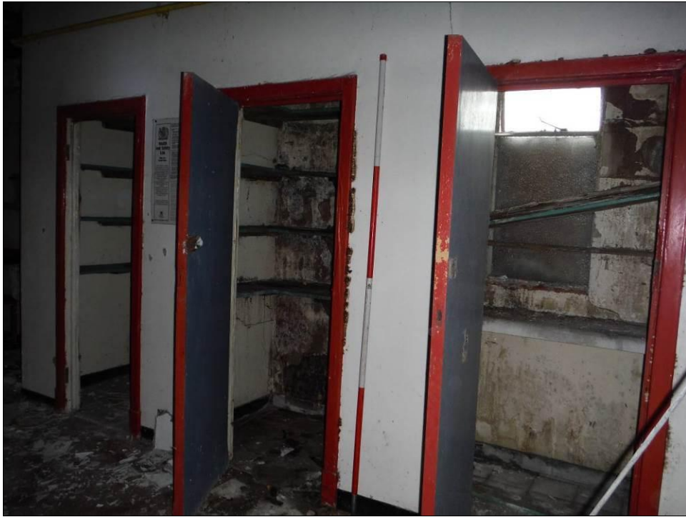
Figure 126: North wall of Room F5, Building B (Scale = 2m).
