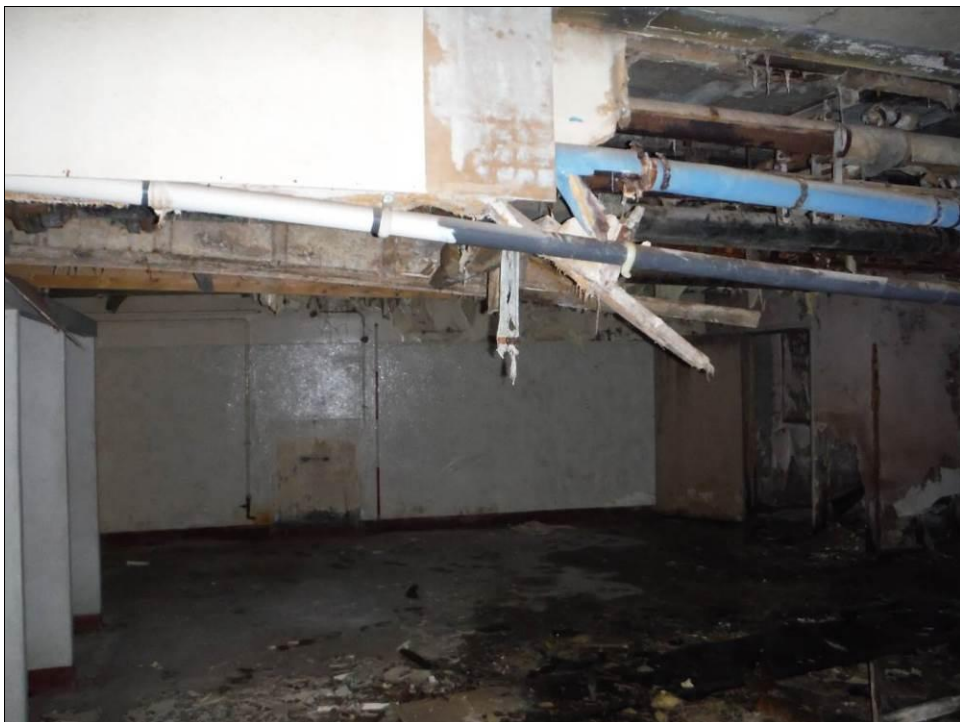
Figure 107: South wall of Room B5, Building B (Scale = 2m).
