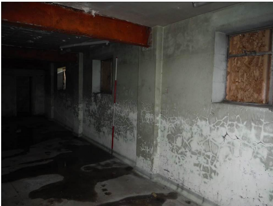
Figure 102: South wall of Room B2, Building B (Scale = 2m).
