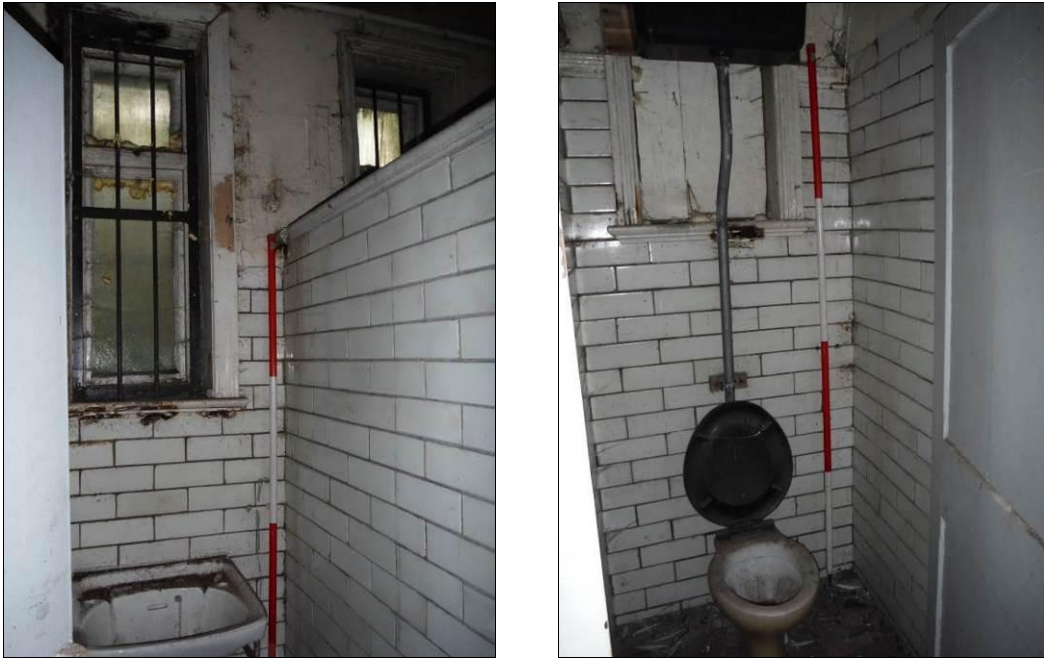
Figure 40: North facing views of Room G4, Building A (Scale = 2m).
