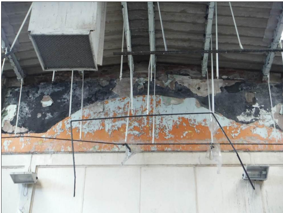
Figure 31: Detail of blocked Diocletian window in the east wall of Room G1 in Building A.
