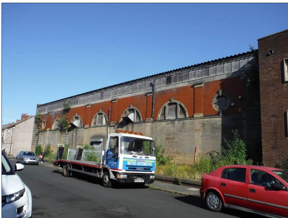
Figure 13: West North West facing oblique view of the South East elevation of Building A (Scale = 2 x 2m).
