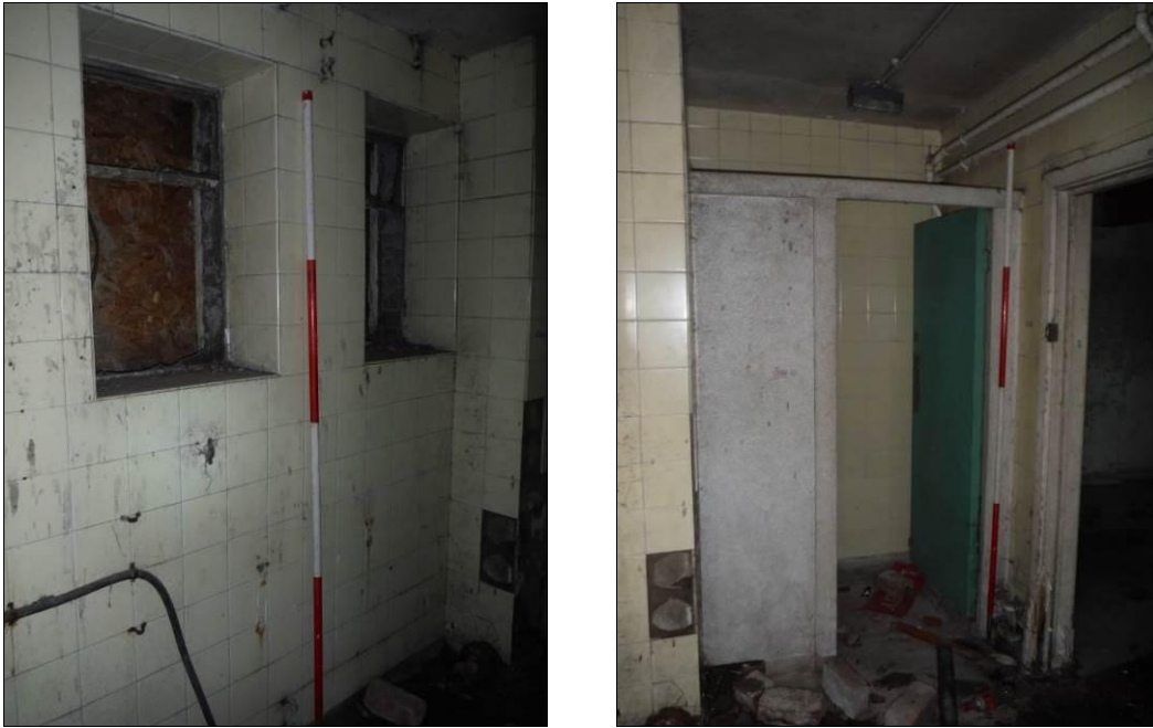
Figure 103: Room B4, Building B (Scale = 2m).
