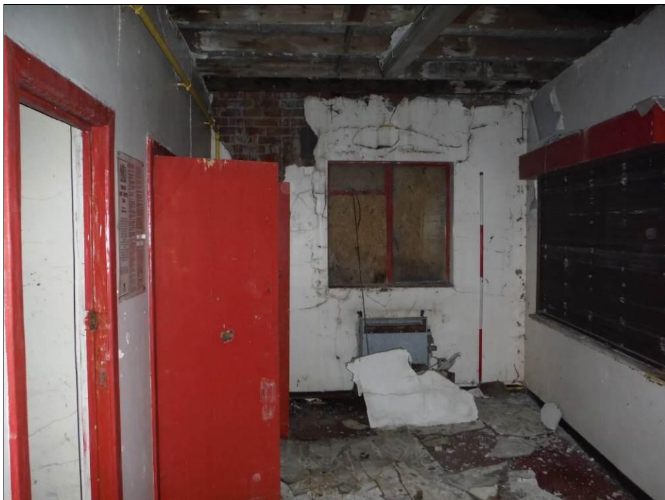
Figure 125: East wall of Room F5, Building B (Scale = 2m).
