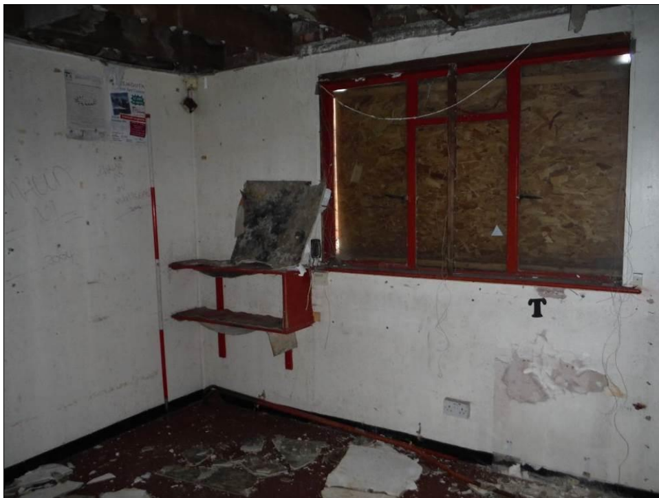
Figure 133: West and north walls of Room F8, Building B (Scale = 2m).
