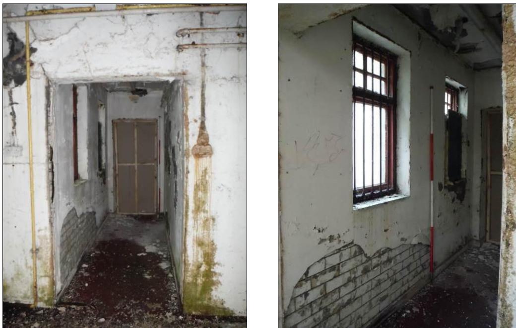
Figure 47: South and west walls of Room G6, Building A (Scale= 2m).
