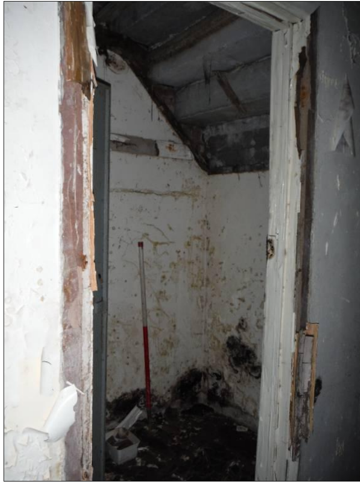
Figure 65: Room G14, Building A (Scale = 1m).
