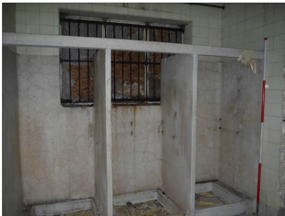
Figure 73: Room G1, Building B (Scale = 2m).
