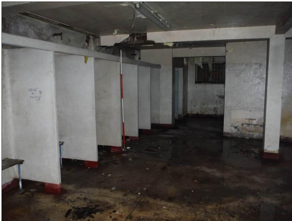
Figure 105: North and west walls of Room B5, Building B (Scale = 2m).
