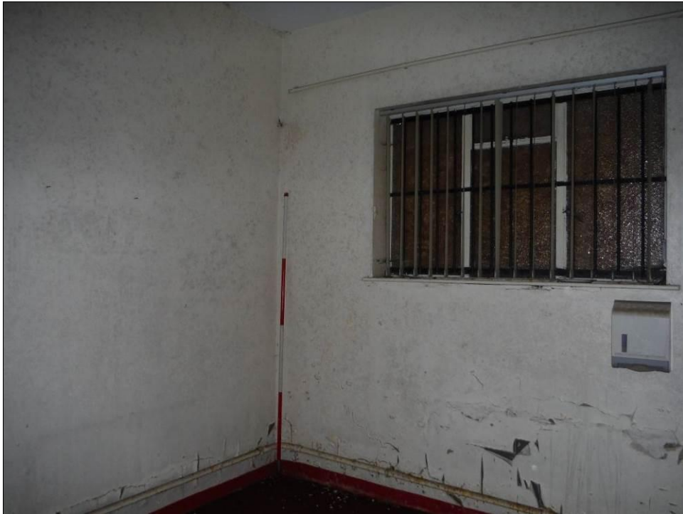
Figure 63: North and east walls of Room G13, Building A (Scale = 2m).
