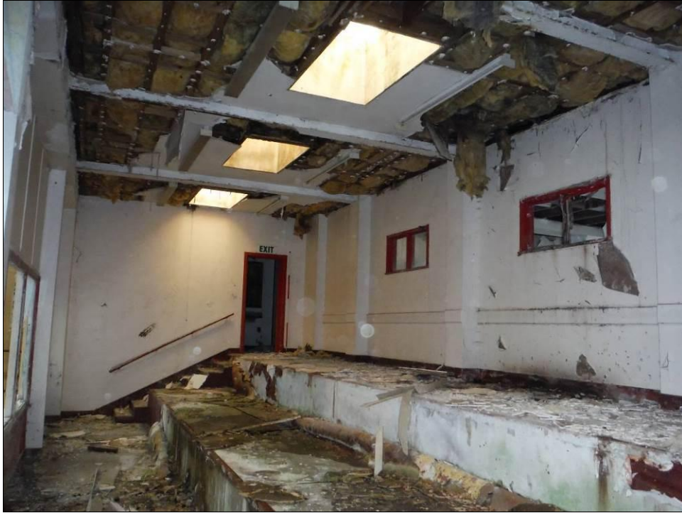
Figure 128: North wall of Room F6, Building B (Scale = 2m).
