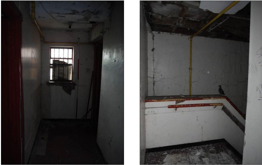
Figure 132: Room F7, Building B (Scale = 2m).
