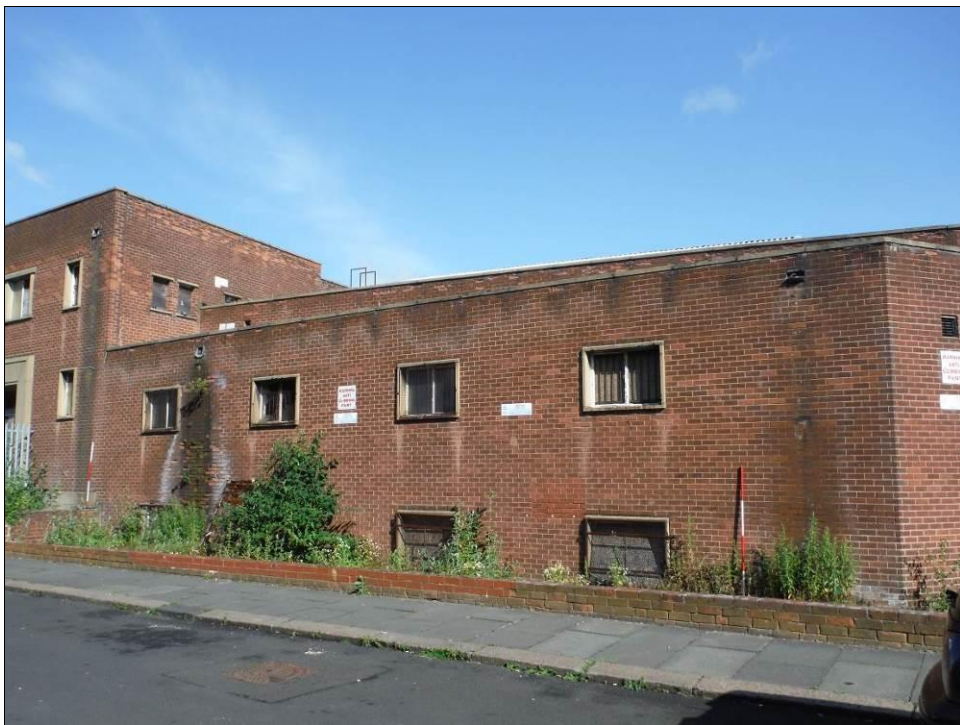
Figure 67: South East elevation of Building B (Scale = 2 x 2m).
