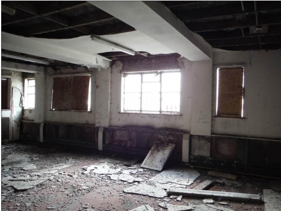
Figure 121: East wall of Room F4, Building B (Scale = 2m).
