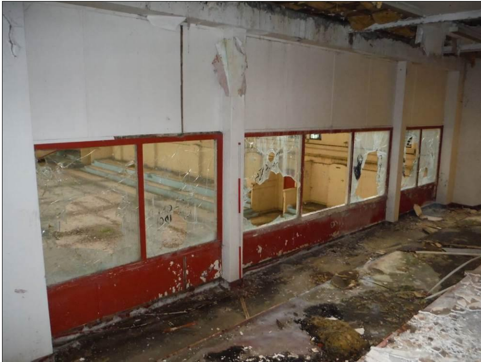
Figure 130: West wall of Room F6, Building B (Scale = 2m).
