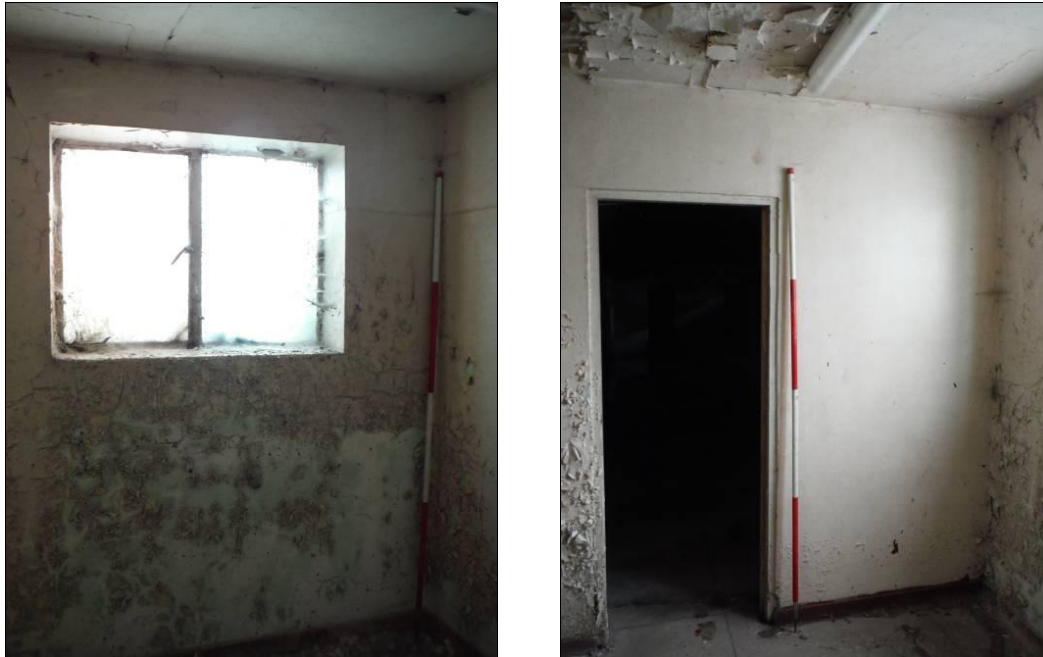
Figure 98: Room B1, Building B (Scale = 2m).
