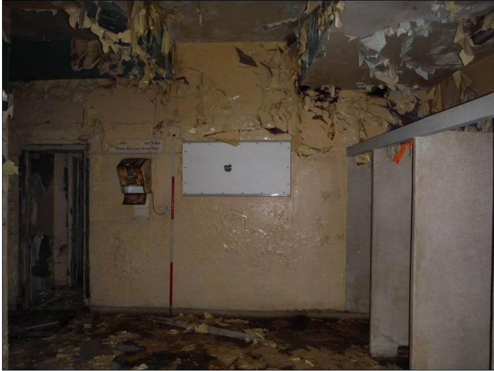
Figure 81: South wall of Room G3, Building B (Scale = 2m).
