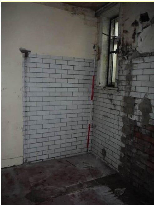
Figure 60: West wall of Room G12, Building A (Scale= 2m).
