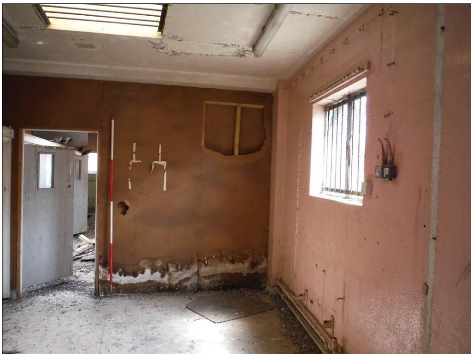
Figure 91: South and east walls of Room G10, Building B (Scale = 2m).
