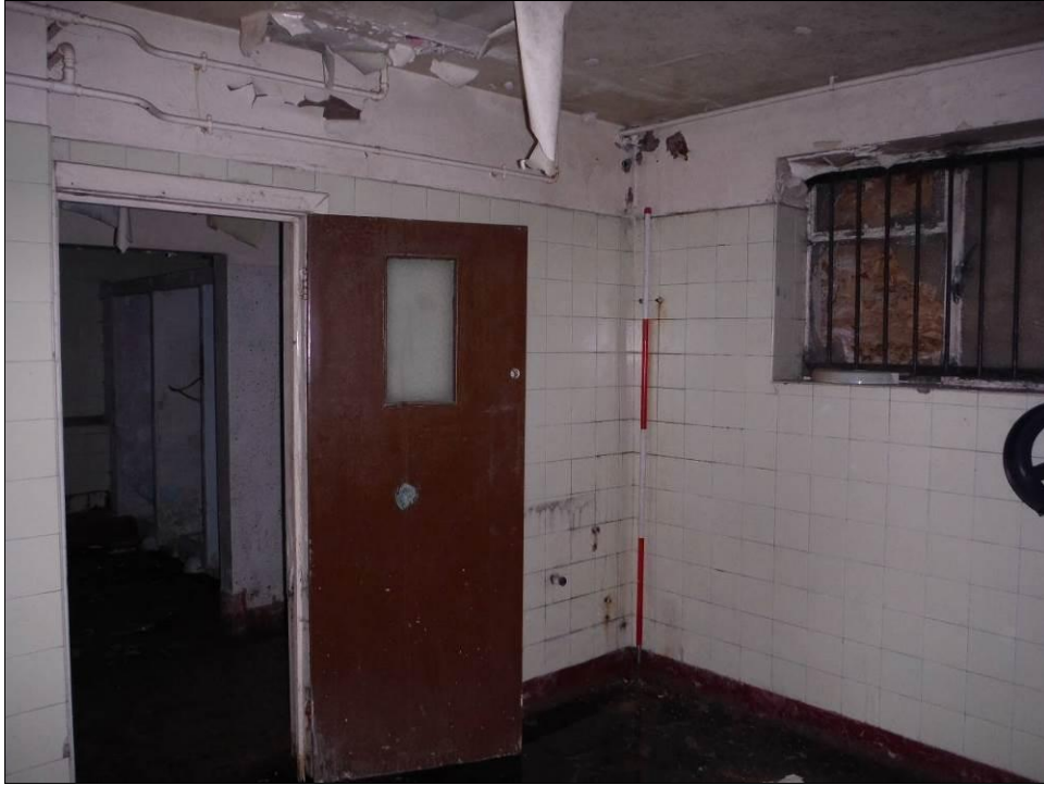
Figure 111: Room B6, Building B (Scale= 2m).
