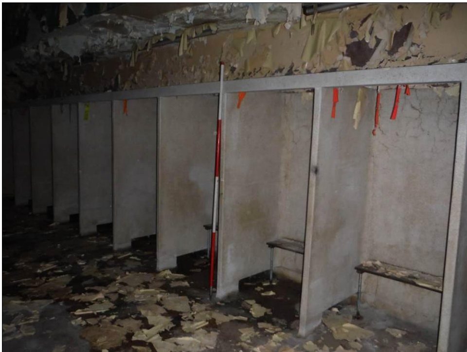
Figure 78: East wall of Room G3, Building B (Scale = 2m).
