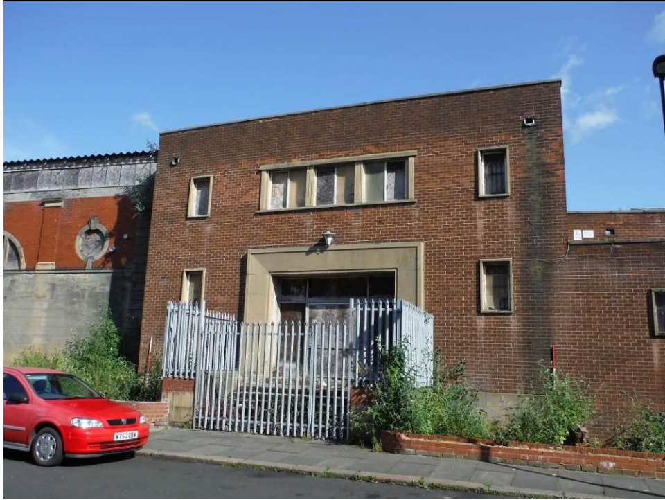
Figure 66: South-east elevation of the two-storey entrance block on Building B (Scale = 2 x 2m).
