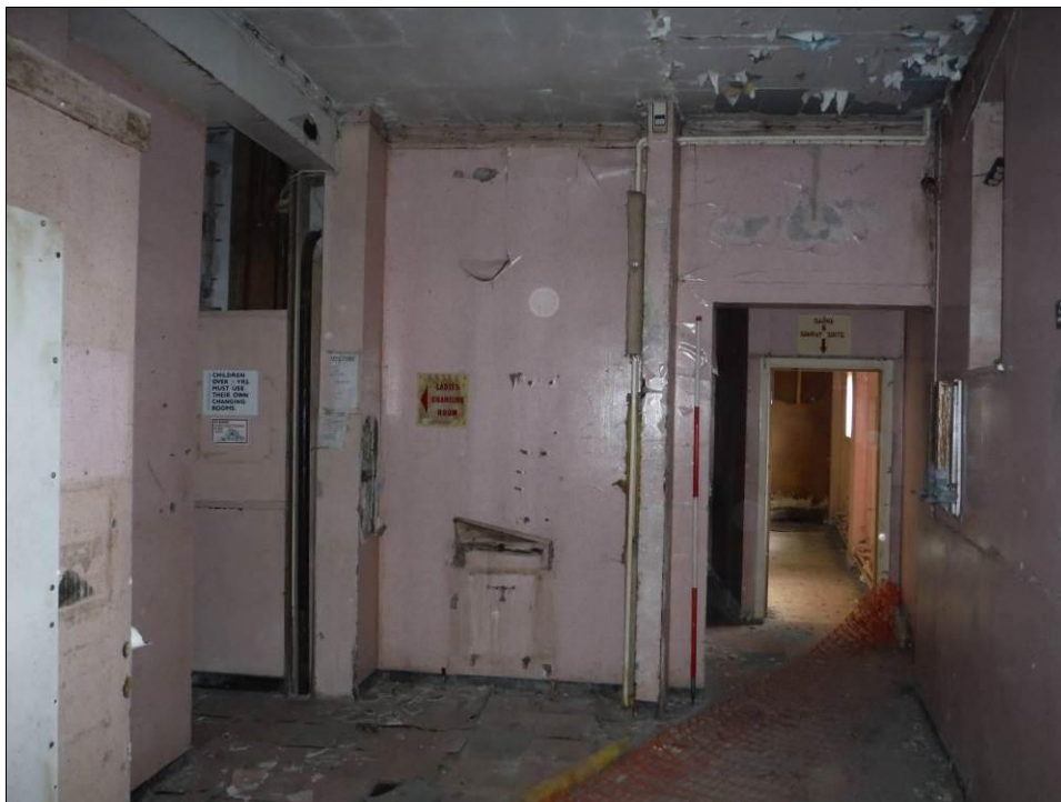
Figure 87: East wall of Room G5, Building B (Scale = 2m).
