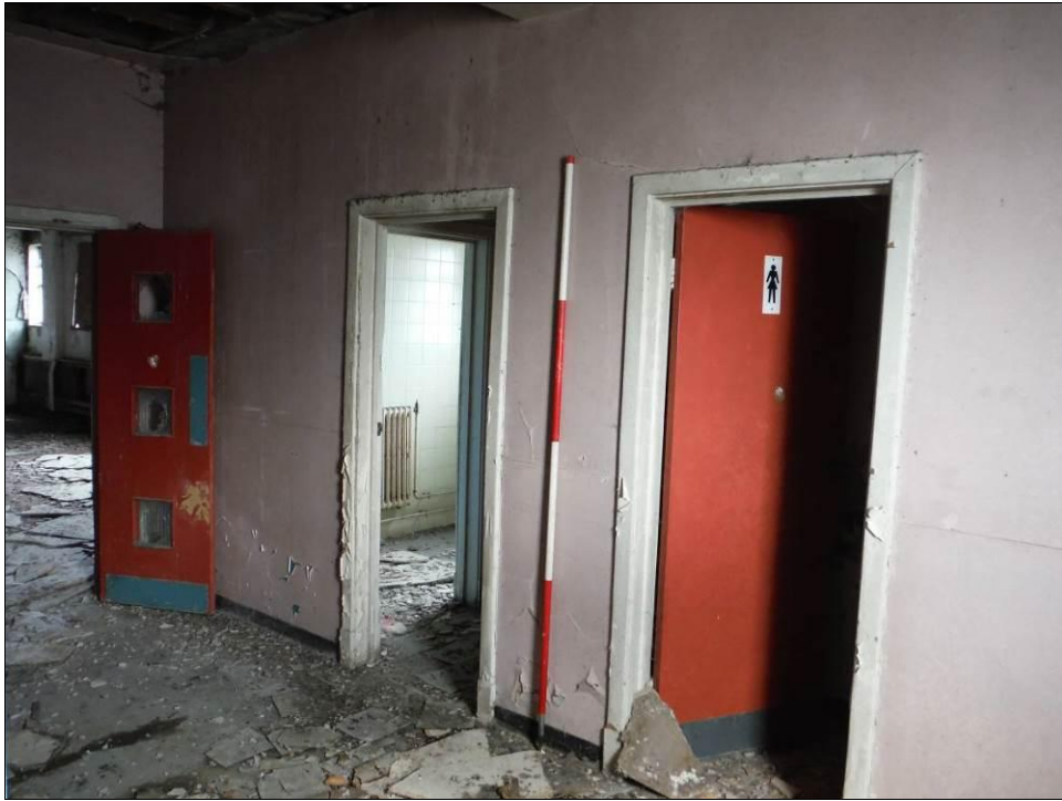
Figure 117: East wall of Room F1, Building B1 (Scale = 2m).
