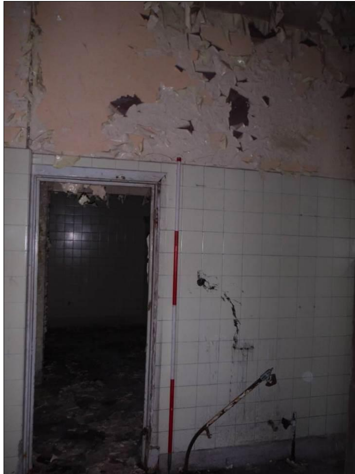
Figure 74: West wall of Room G2, Building B (Scale= 2m).
