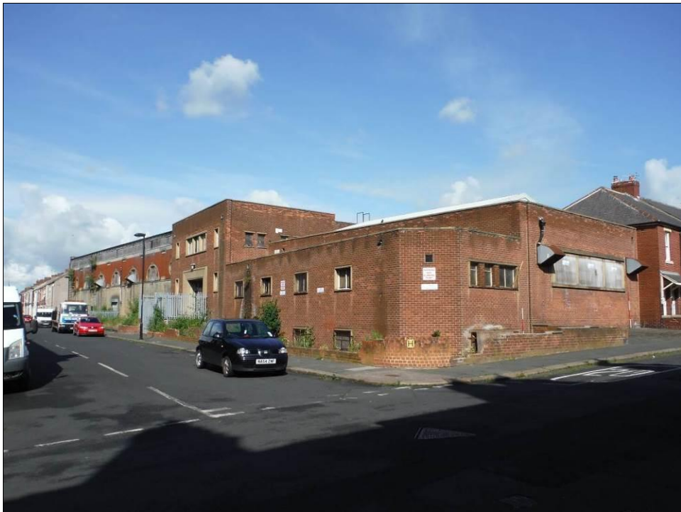
Figure 71: East facing oblique view of South East and North East elevations of Building B (Scale = 2 x 2m).
