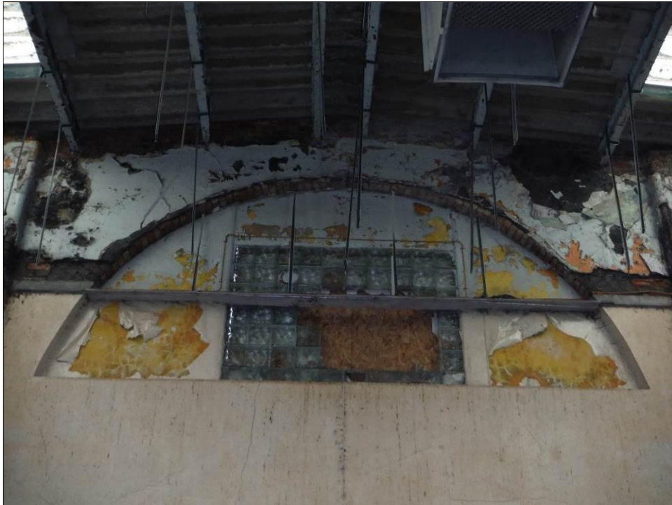
Figure 26: Detail of Diocletian window in the west wall of Room G1 in Building A.
