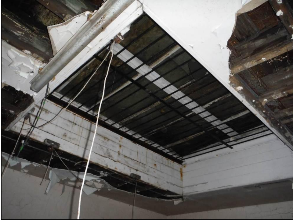
Figure 59: Detail of skylight in Room G9, Building A.
