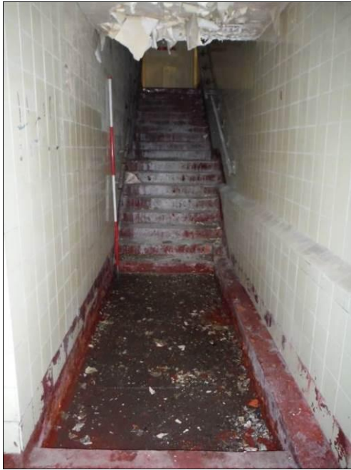
Figure 113: Detail of stairway in Room B7, Building B (Scale = 2m).
