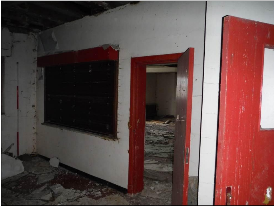
Figure 124: South wall of Room F5, Building B (Scale = 2m).
