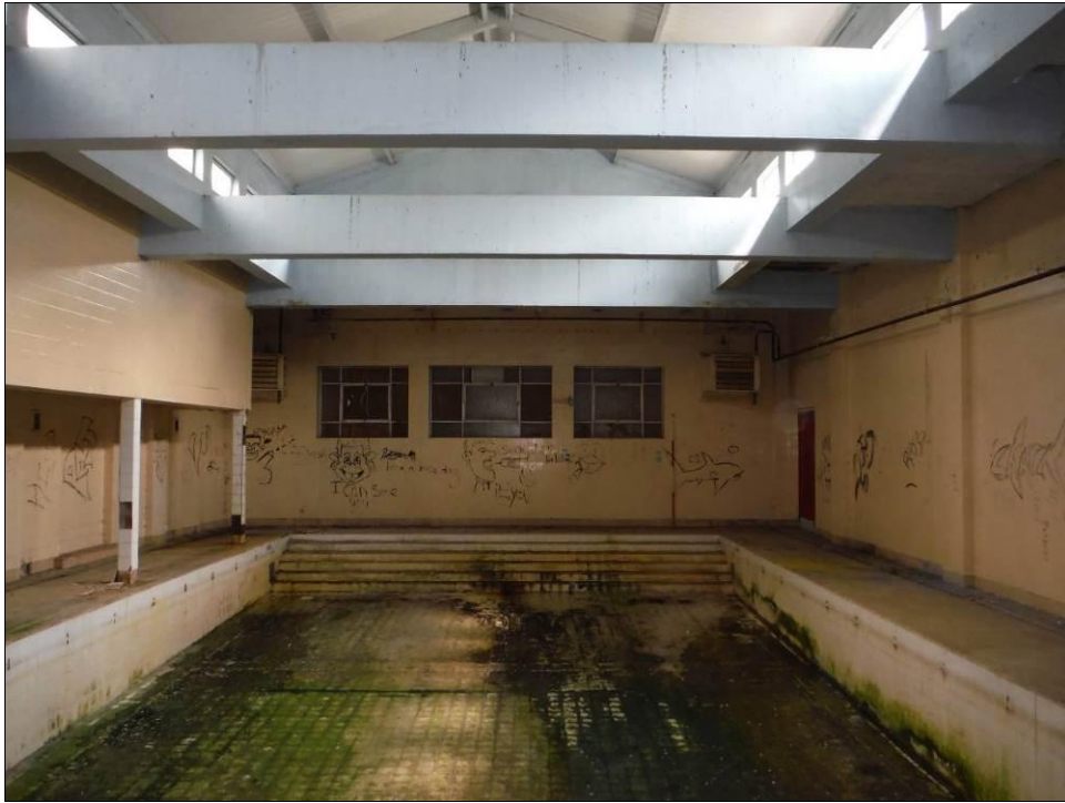
Figure 96: East wall of Room G12, Building B (Scale = 2m).
