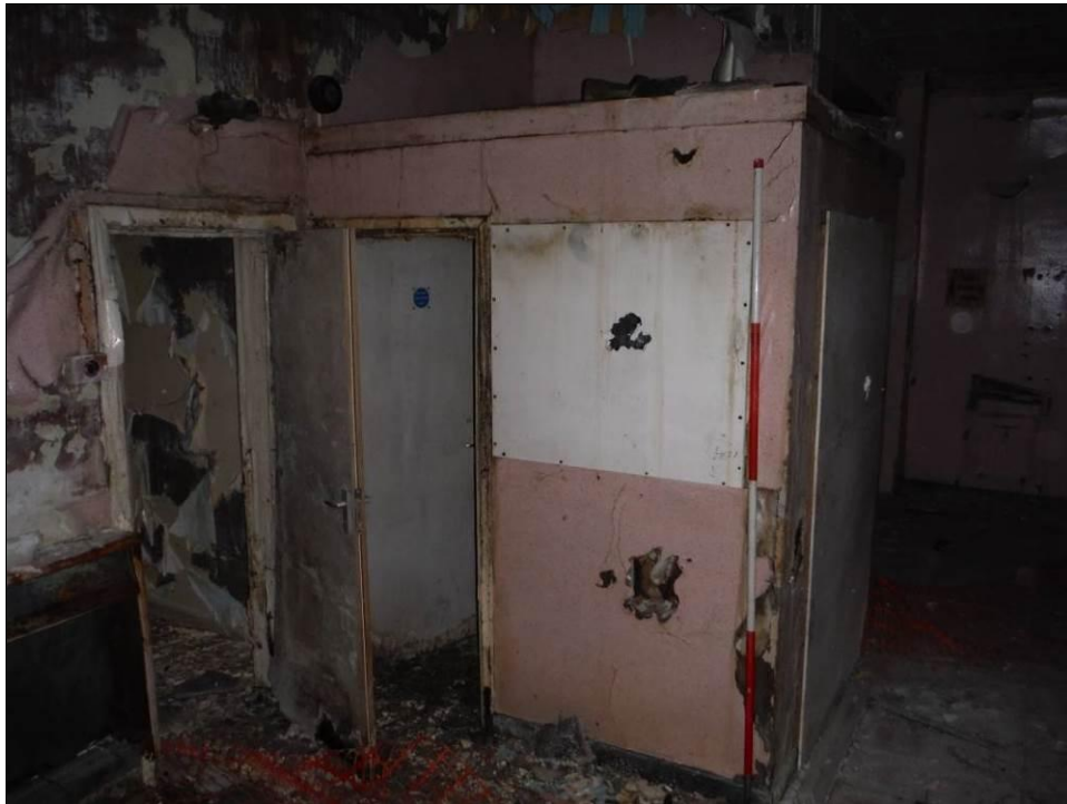
Figure 85: Exterior of Room G6 in Room G5, Building B (Scale = 2m).
