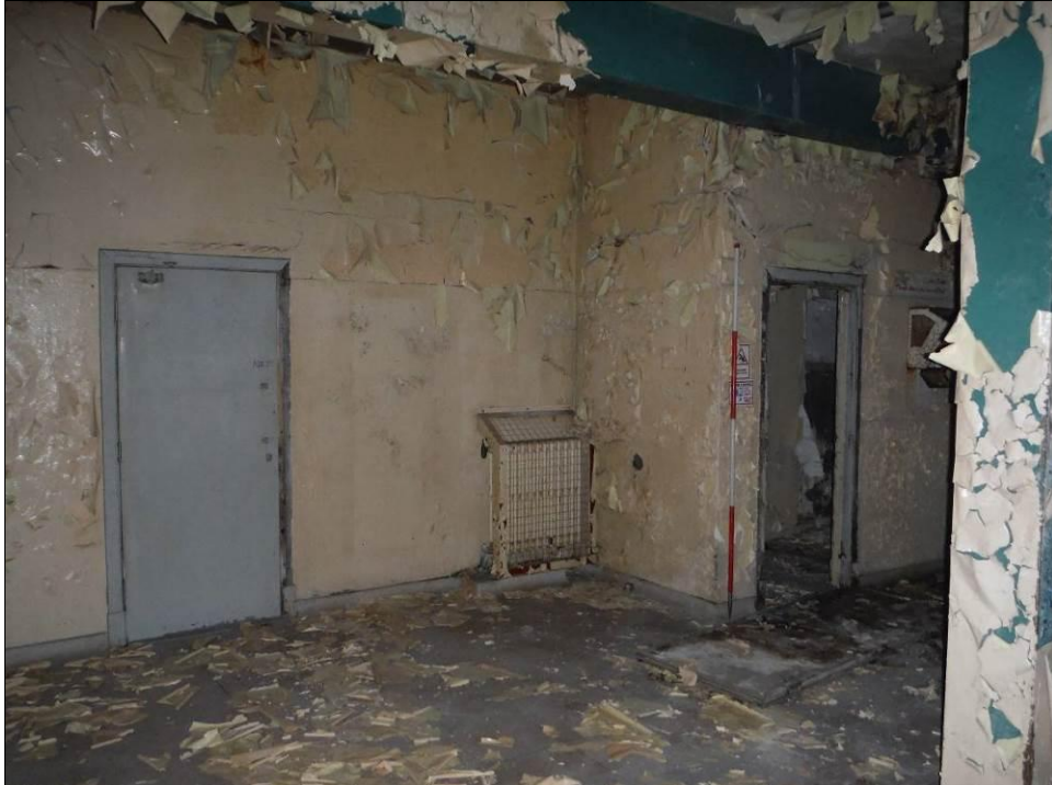
Figure 80: South wall of Room G3, Building B (Scale = 2m).
