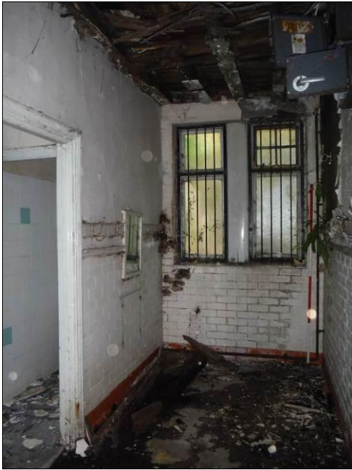
Figure 51: Room G8, Building A (Scale = 2m).
