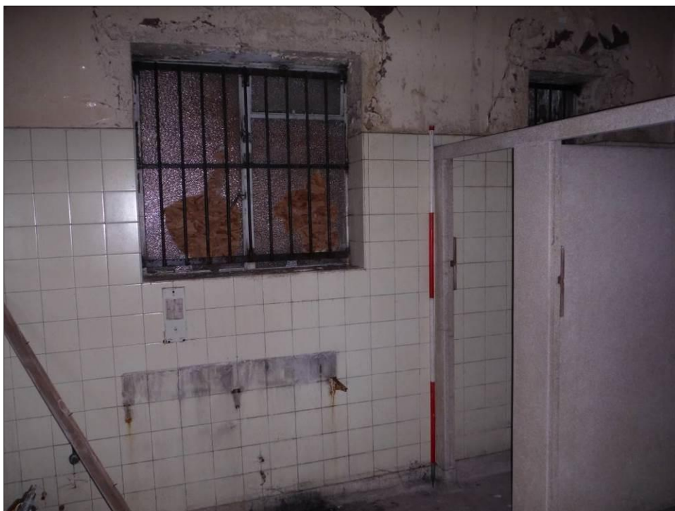
Figure 75: North wall of Room G2, Building B (Scale = 2m).
