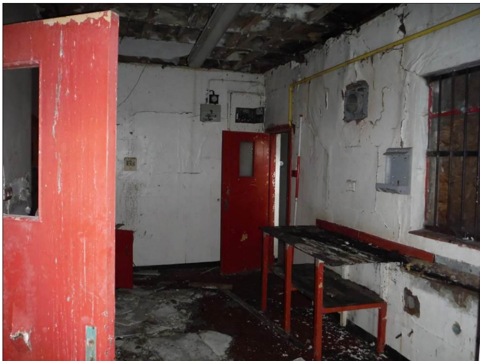
Figure 127: West wall of Room F5, Building B (Scale = 2m).
