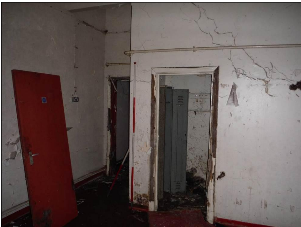
Figure 64: South and west walls of Room G13, Building A (Scale = 2m).
