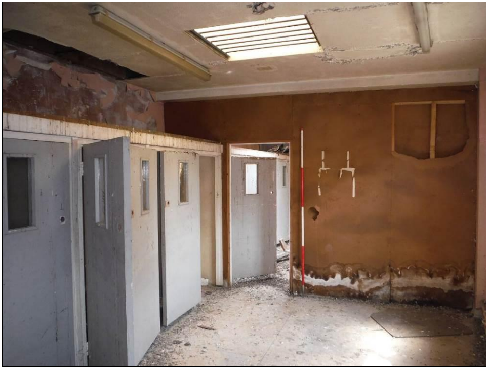
Figure 90: North and east walls of Room G10, Building B (Scale = 2m).
