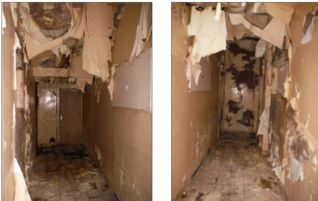
Figure 83: Room G4, Building B looking west (left) and east (right) (Scale = 2m).
