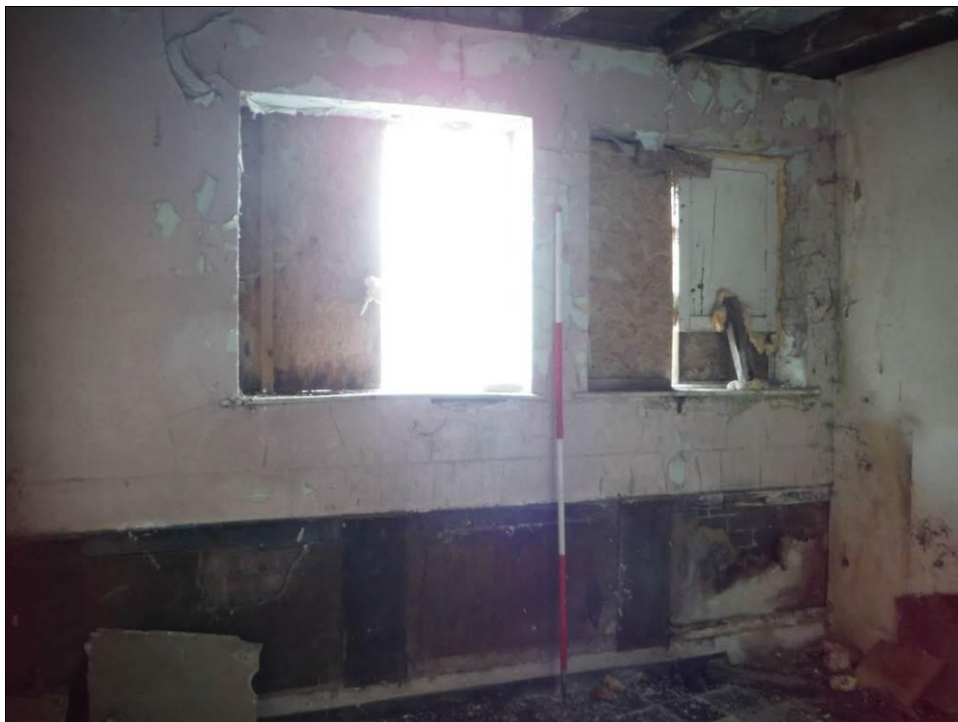
Figure 116: South wall of Room F1, Building B (Scale = 2m).
