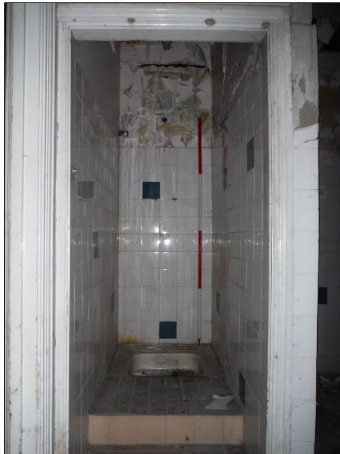
Figure 53: Room G11, Building A (Scale = 2m).
