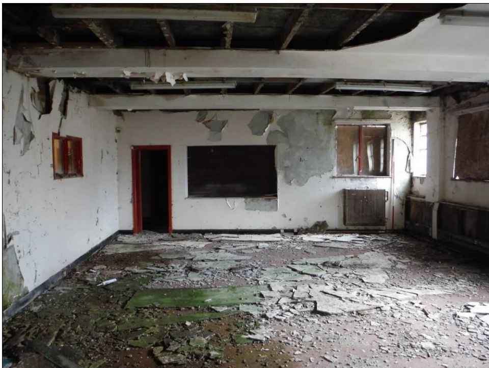
Figure 122: North wall of Room F4, Building B (Scale = 2m).
