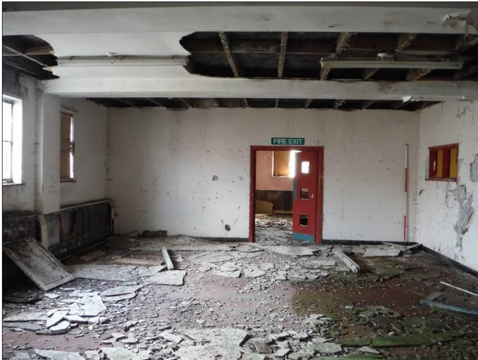
Figure 120: South wall of Room F4, Building B (Scale = 2m).
