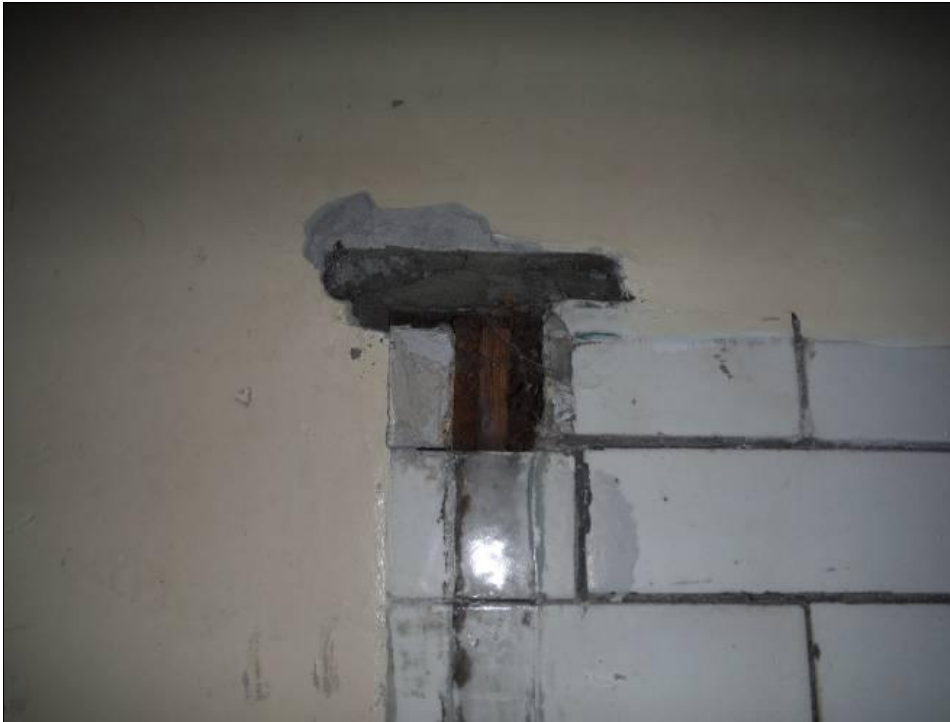
Figure 62: Detail of timber moulded corning from Room G4 in west wall of G12, Building A.
