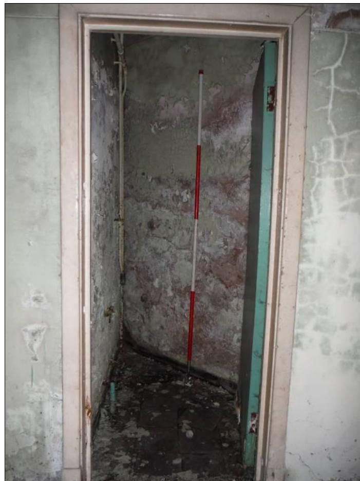
Figure 104: Room B3, Building B (Scale = 2m).
