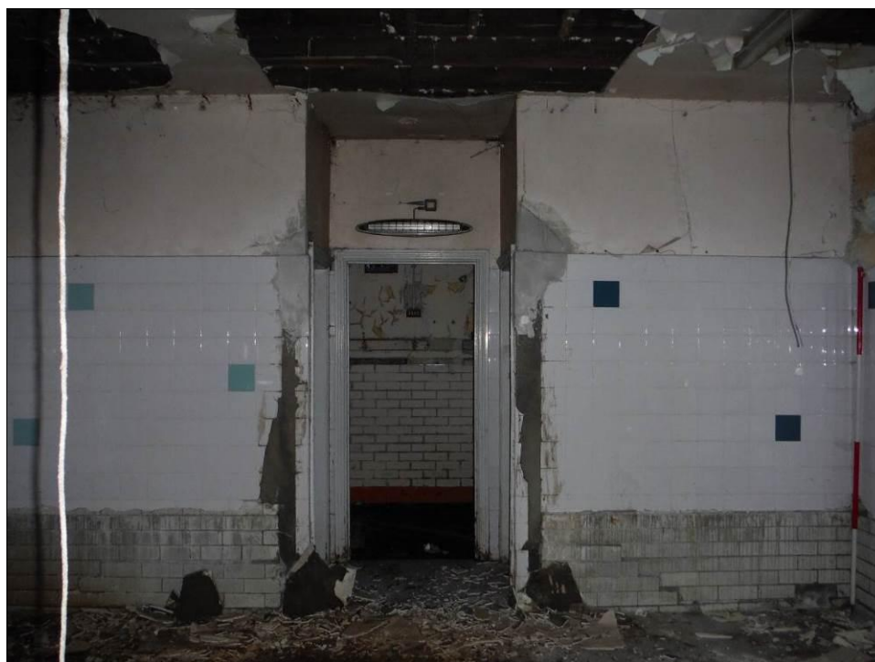
Figure 54: West wall of Room G9, Building A (Scale = 2m).
