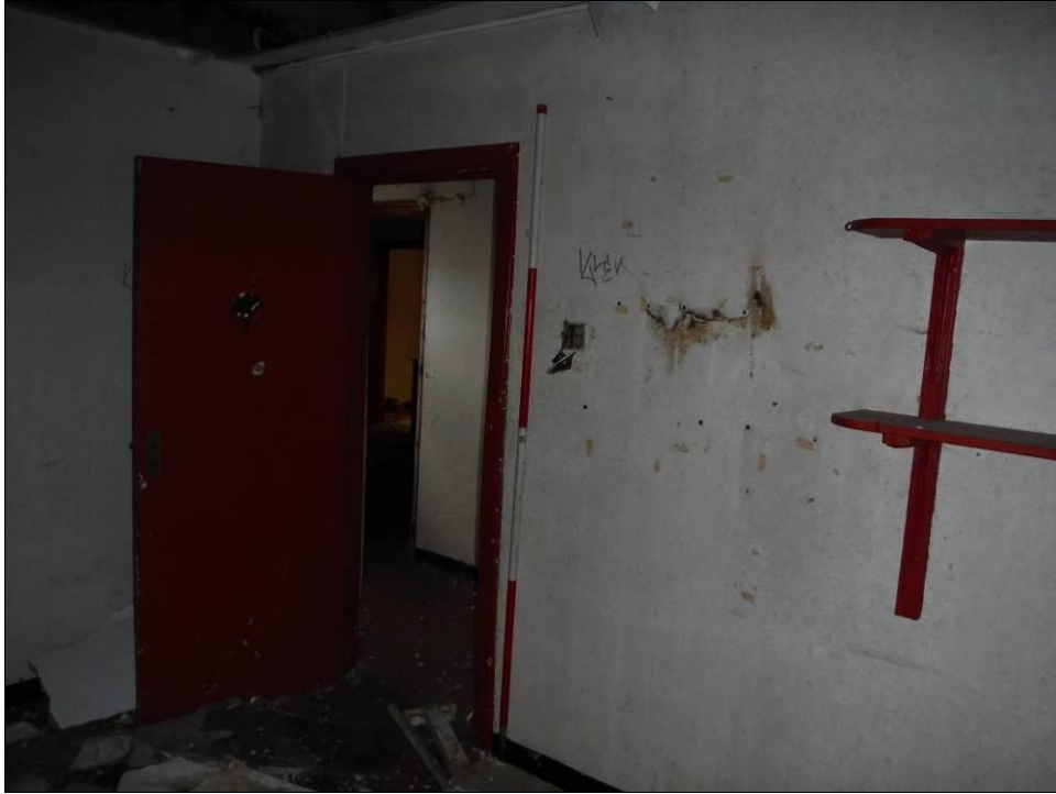
Figure 134: South wall of Room F8, Building B (Scale = 2m).
