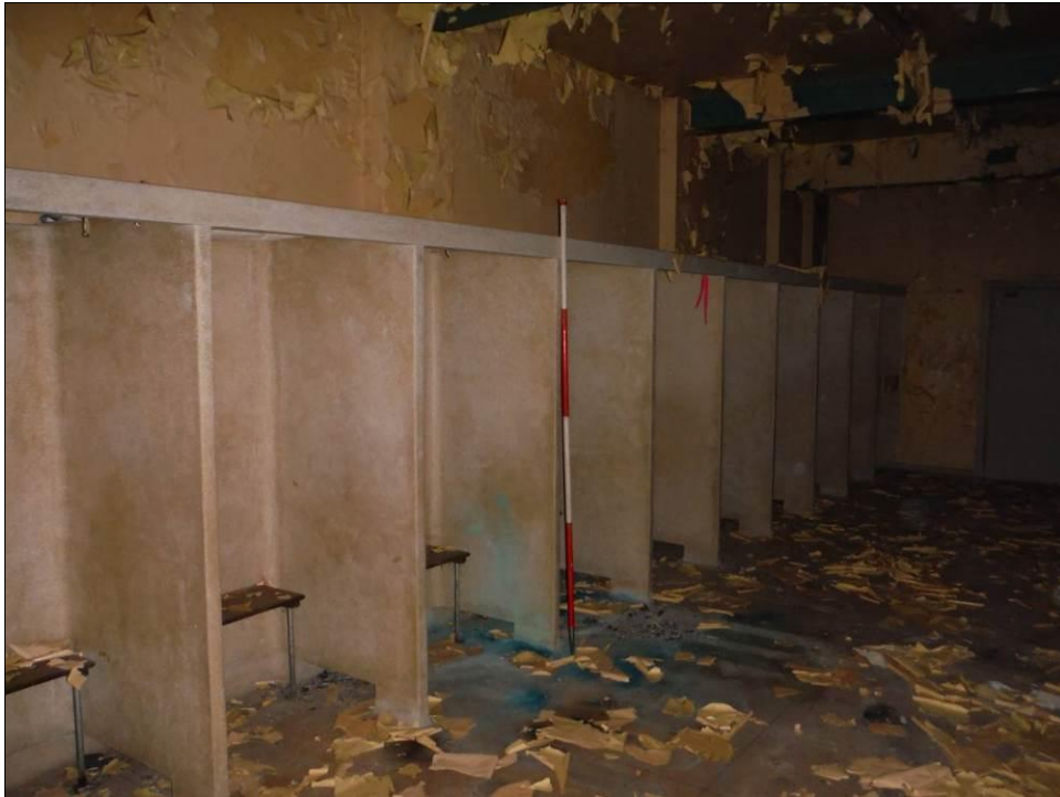
Figure 79: East wall of Room G3, Building B (Scale = 2m).
