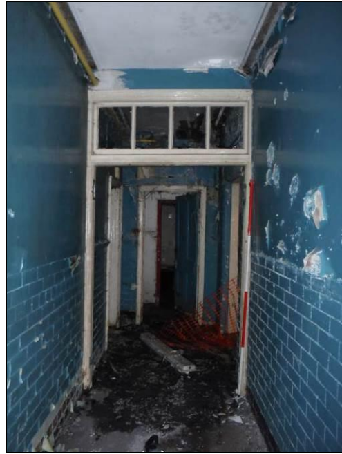
Figure 37: Detail of transom doorway in Room G2, Building A (Scale= 2m).
