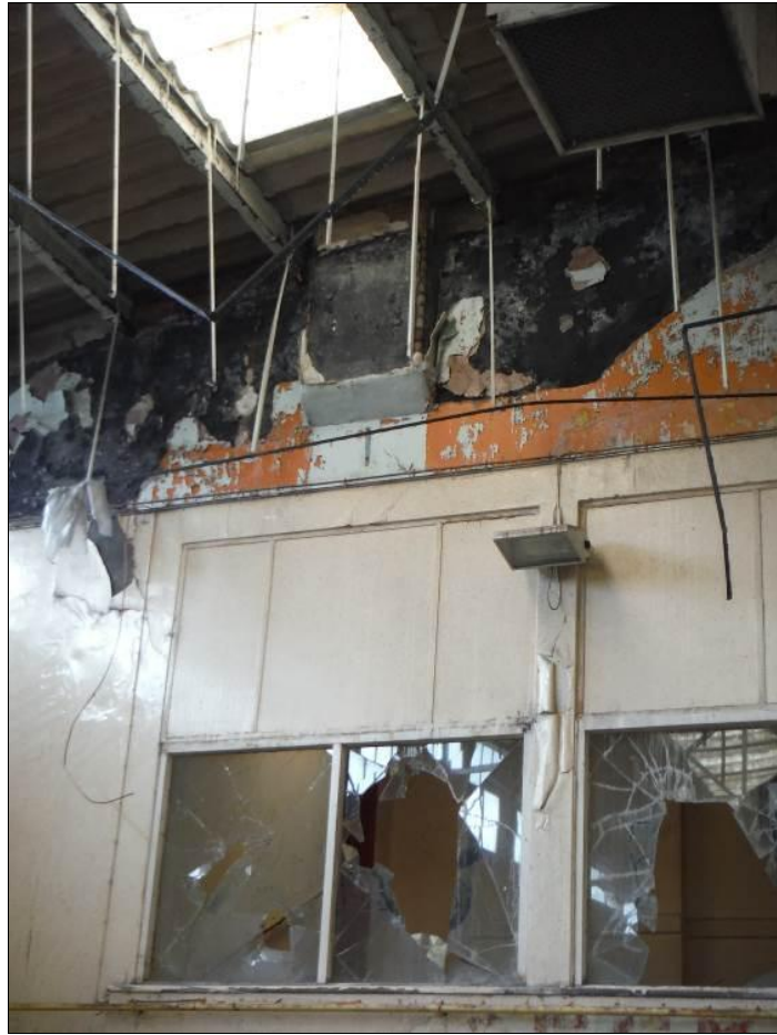
Figure 32: Surviving upper portion of the original pilasters on the west wall.
