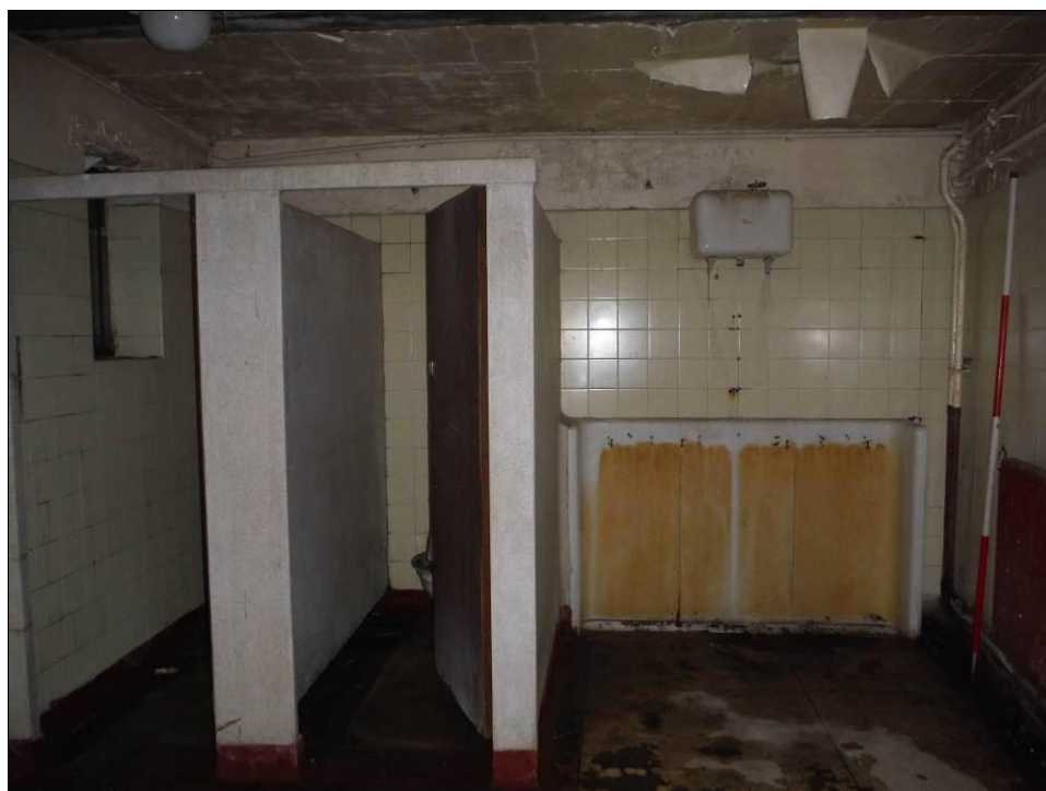
Figure 110: Room B6, Building B (Scale = 2m).
