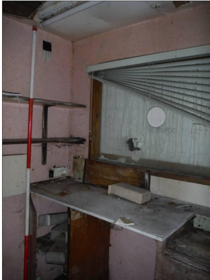
Figure 86: Interior of Room G6, Building B (Scale = 2m).
