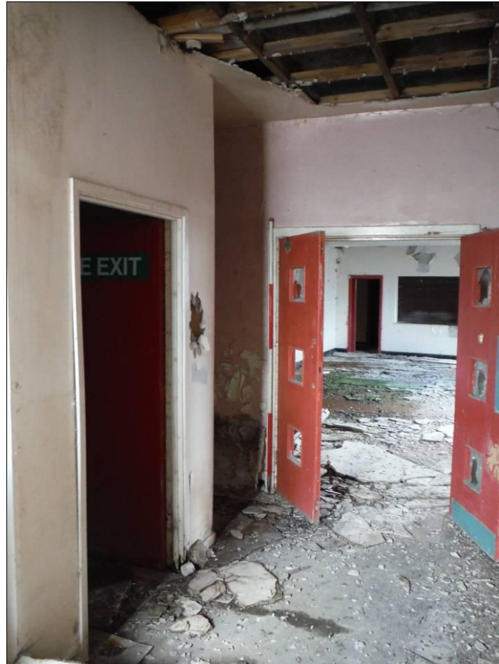
Figure 115: North and west walls of Room F1, Building B (Scale = 2m).
