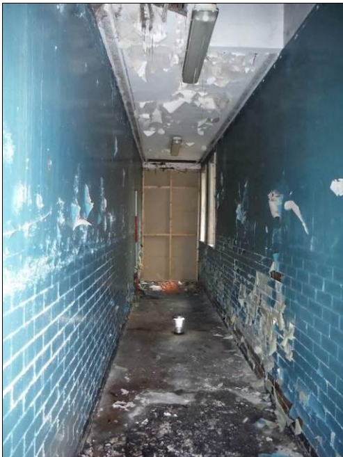
Figure 34: West wall of Room G2, Building A (Scale = 2m).
