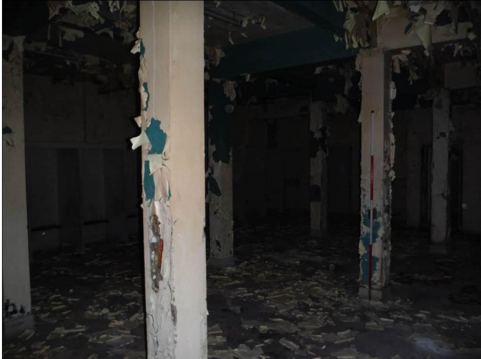
Figure 82: Detail of concrete pillars in Room G3, Building B (Scale = 2m).
