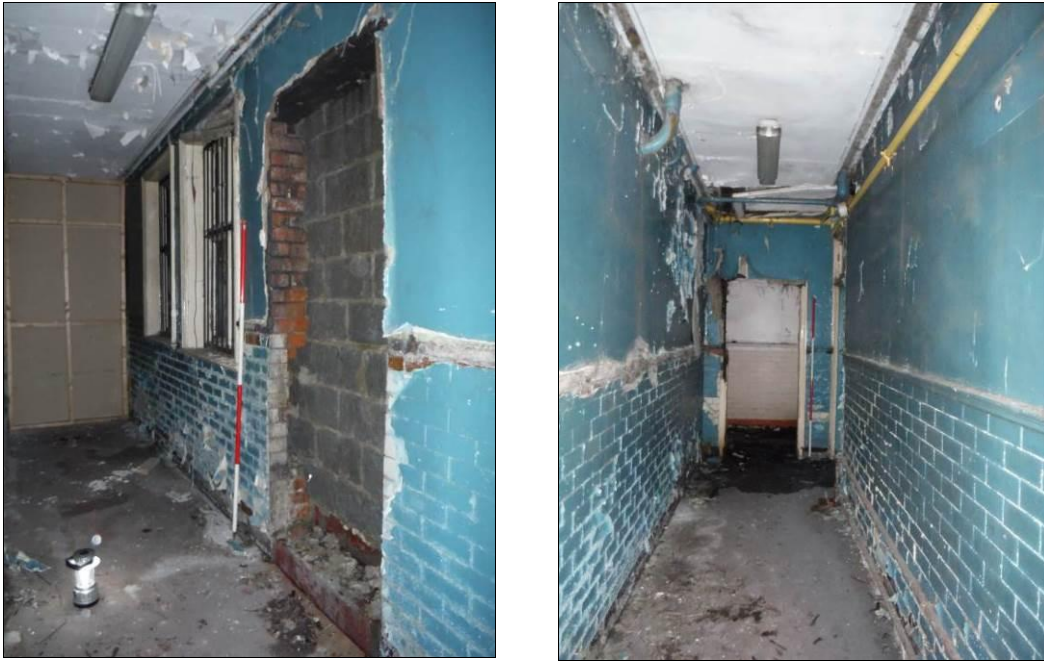
Figure 48: Room G7, Building A (Scale = 2m)
