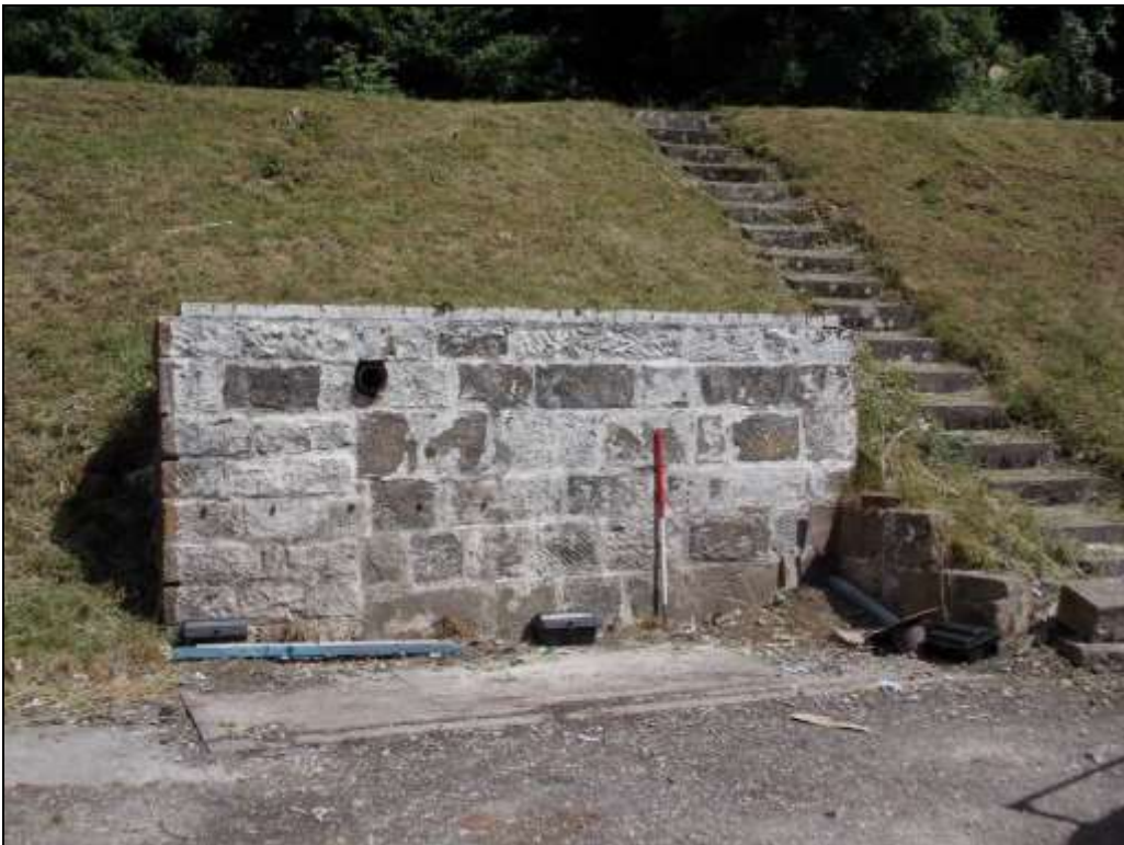
Plate 41: Detail of standing boundary wall, looking north-east.
