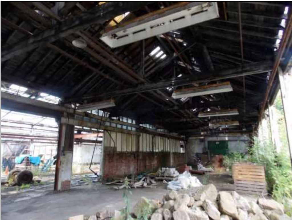
Plate 76: Internal view of Unit 18, looking north.
