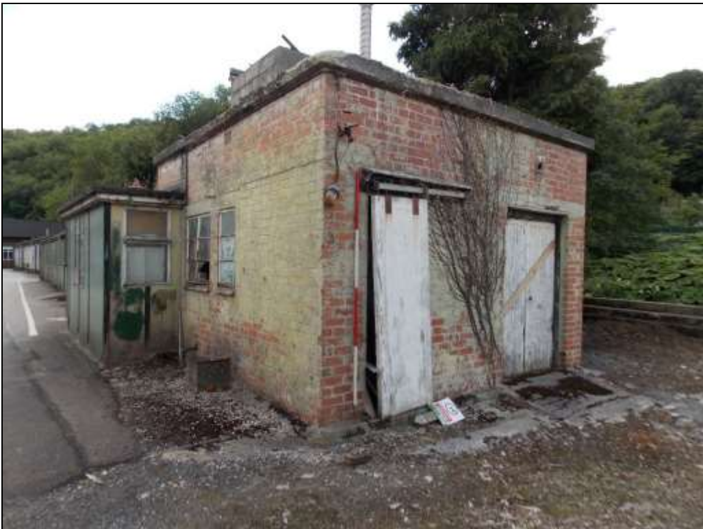
Plate 64: Plant room within the western end of Unit 22, looking south-east.
