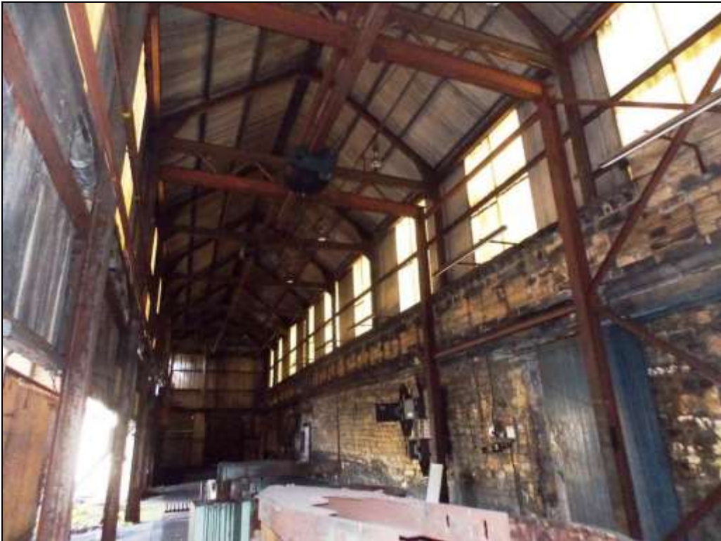
Plate 82: Internal view of Unit 2, looking north-east.
