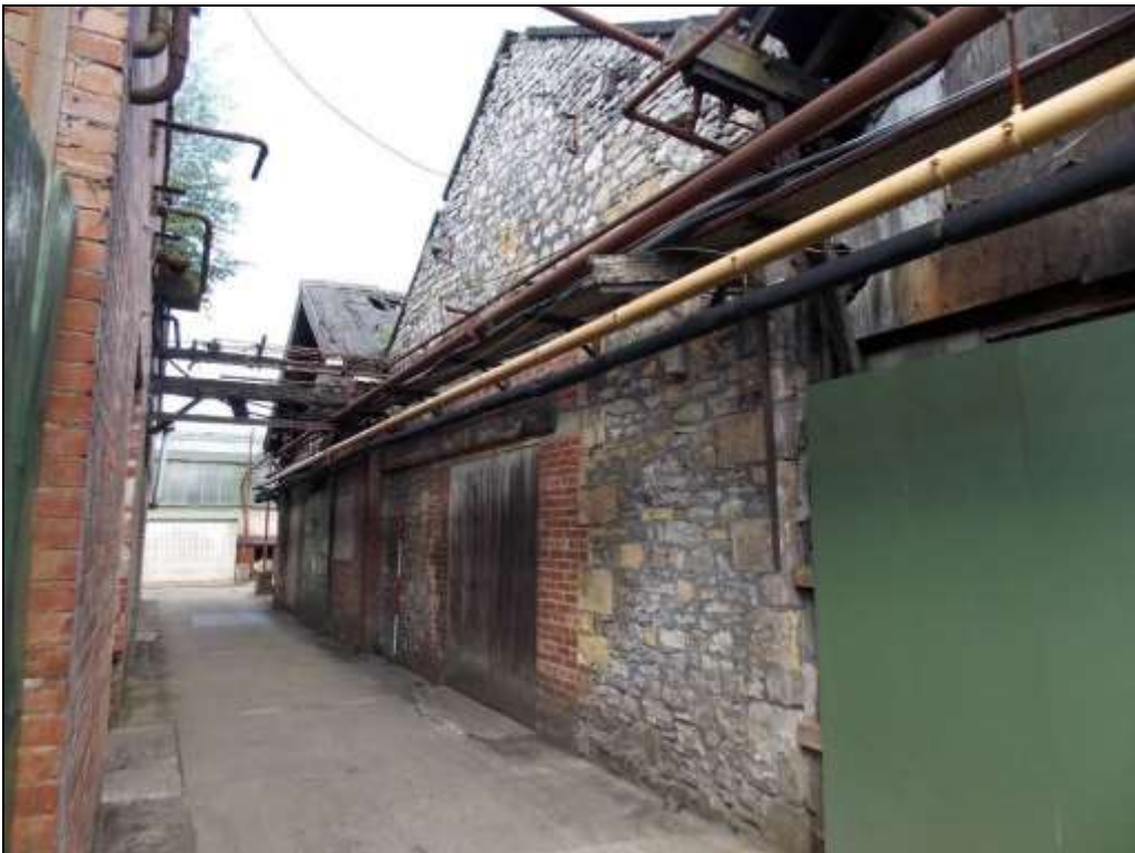
Plate 47: South elevation of Units 7a – c, looking north-west.
