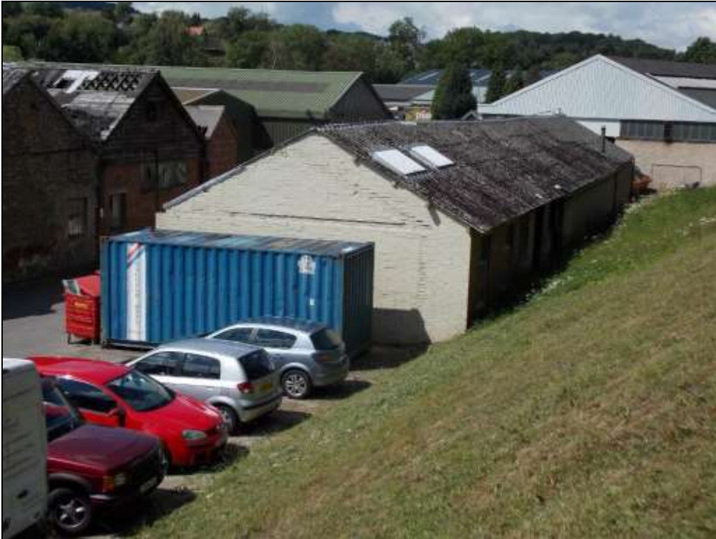
Plate 43: Eastern gable wall showing scars of already demolished extension, looking west.
