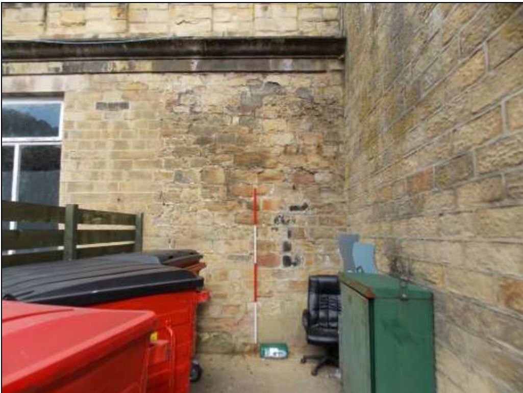
Plate 9: Detail of the extant original wall with soot stain, looking west.
