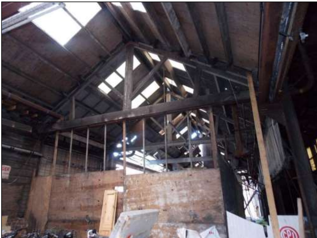
Plate 79: Internal view of Unit 17, looking north.
