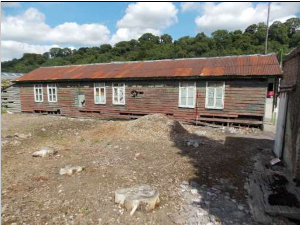
Plate 61: South elevation of Unit 21, looking north-east.
