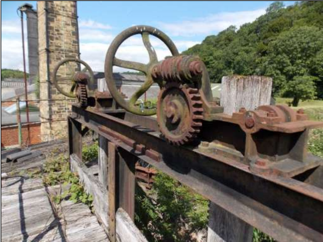
Plate 12: Detail of gate's ratchet wheels, looking north-west.
