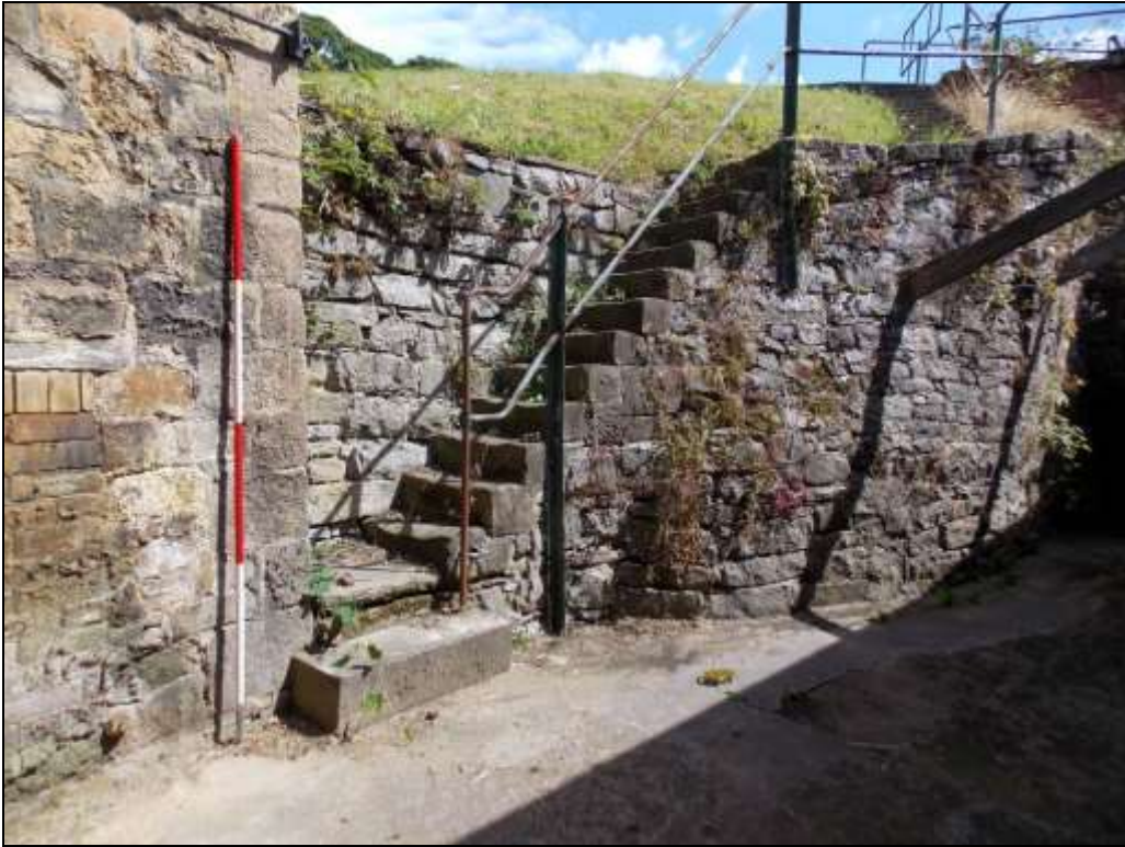
Plate 14: Primary staircase to the former water wheel housing, looking north-east.
