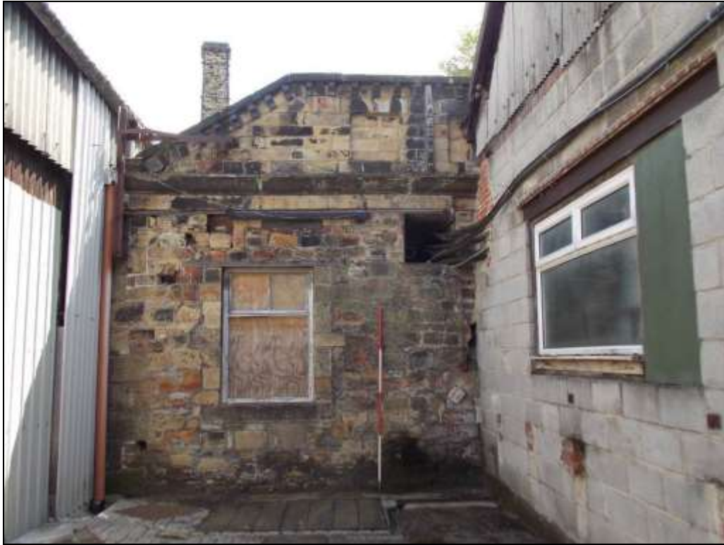
Plate 20: Northern end of the west elevation with sloping parapet, looking east.
