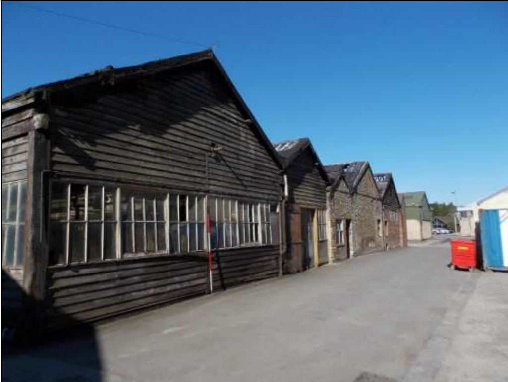
Plate 46: North elevation of Units 7a – c, looking west.
