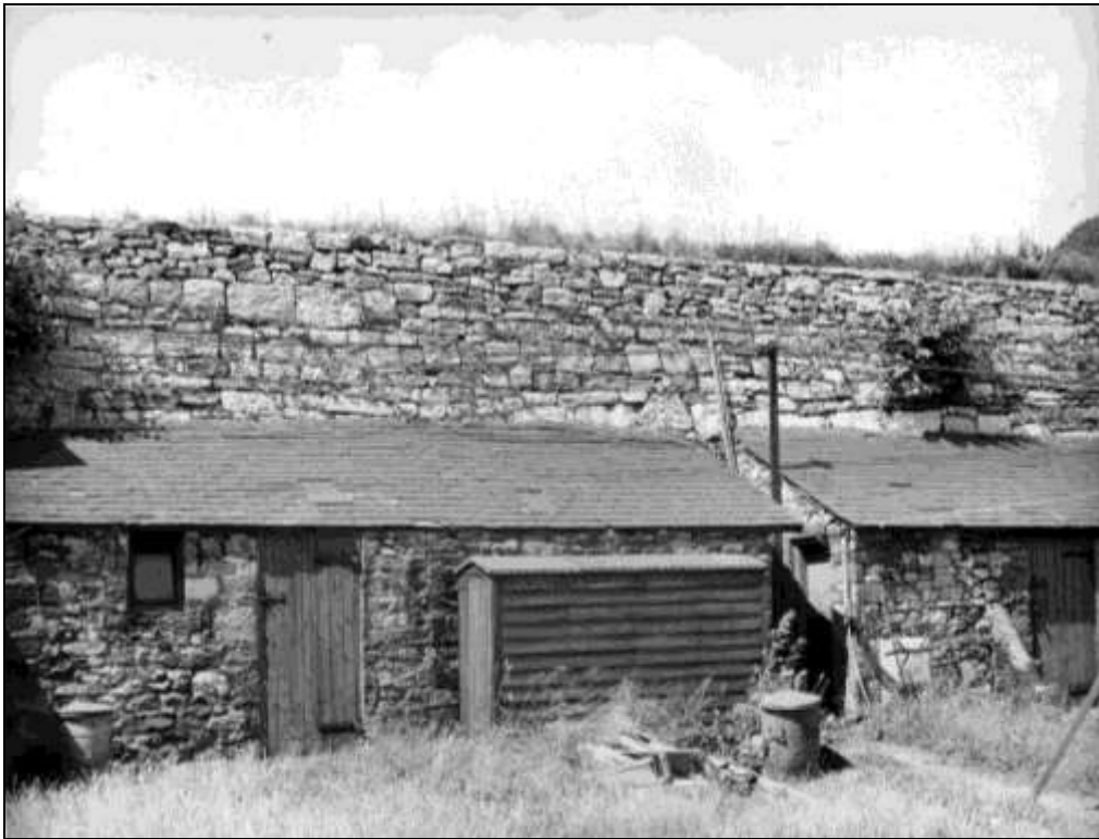
Plate 31: Historical photograph showing former lean-to outbuildings against the retaining wall.
