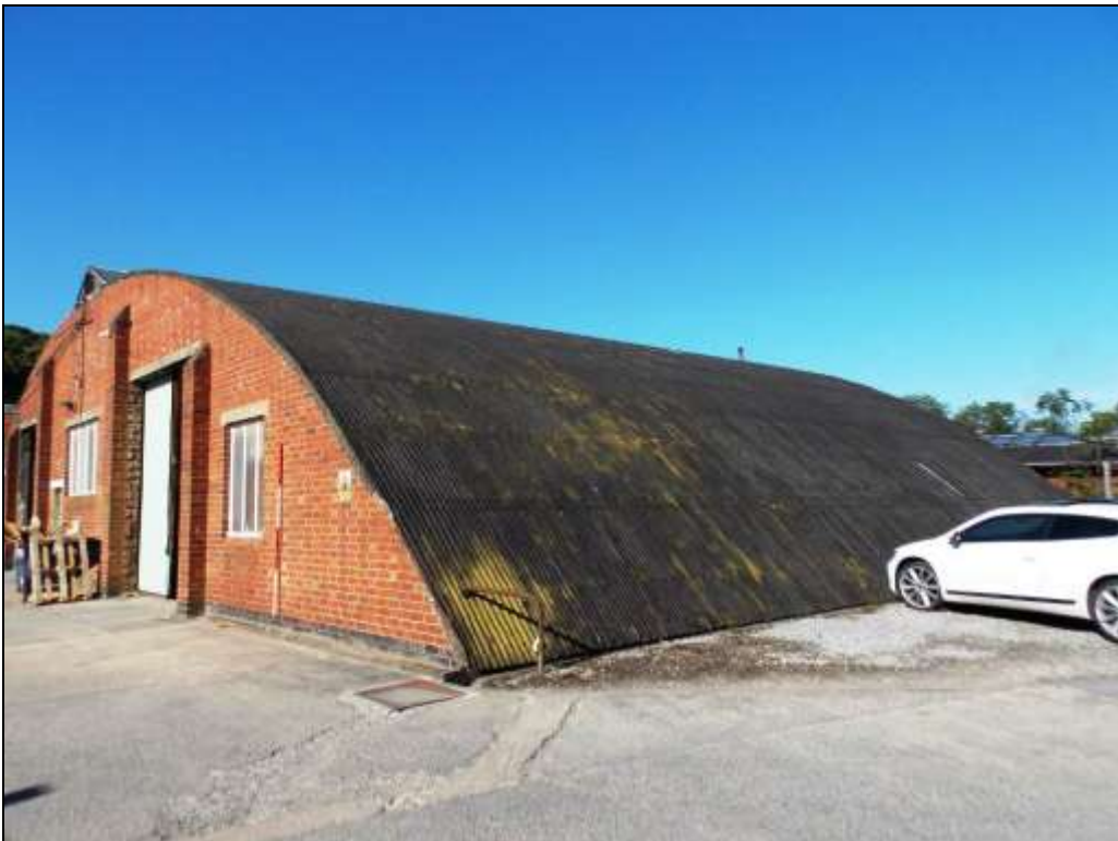
Plate 58: Detail of roof structure, looking south-west.
