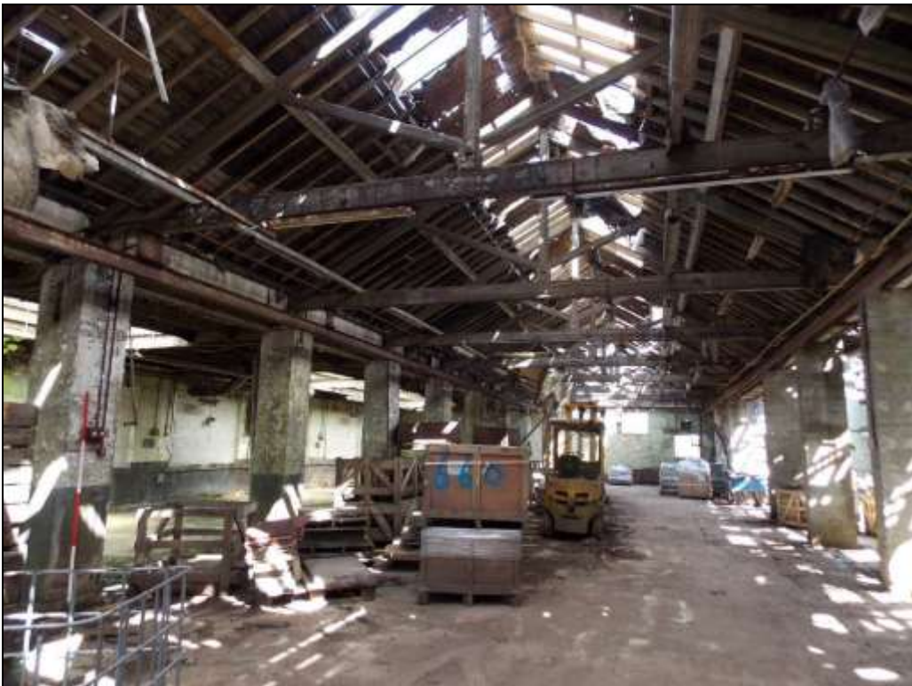
Plate 51: Internal view of Unit 7c, looking north.
