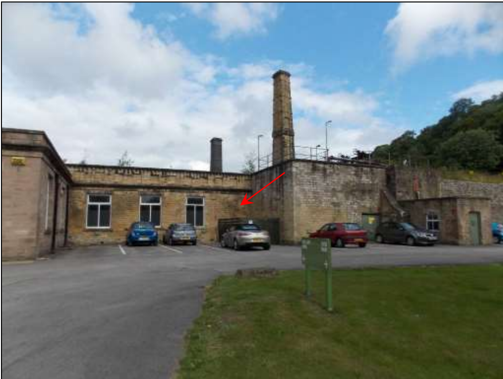
Plate 8: Northern side of the east elevation with surviving masonry of the primary mill (arrow).
