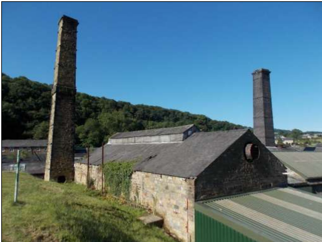
Plate 32: General view of the Retort House, looking south-west.
