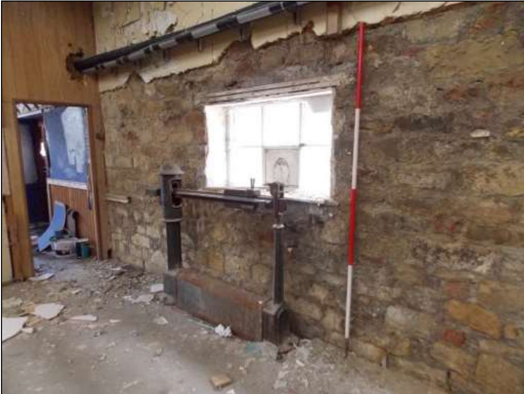
Plate 24: Detail of the weighing scale, looking south-east.
