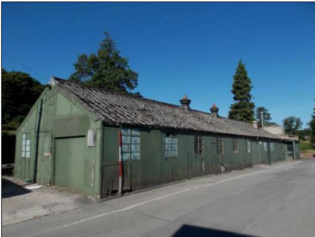
Plate 62: North elevation of Unit 22 along the access road of the works, looking west.
