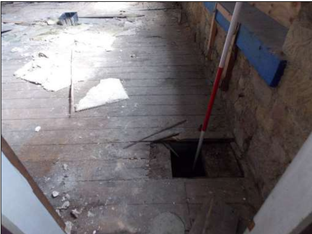
Plate 25: Timber floor with cavity within the office block, looking north.
