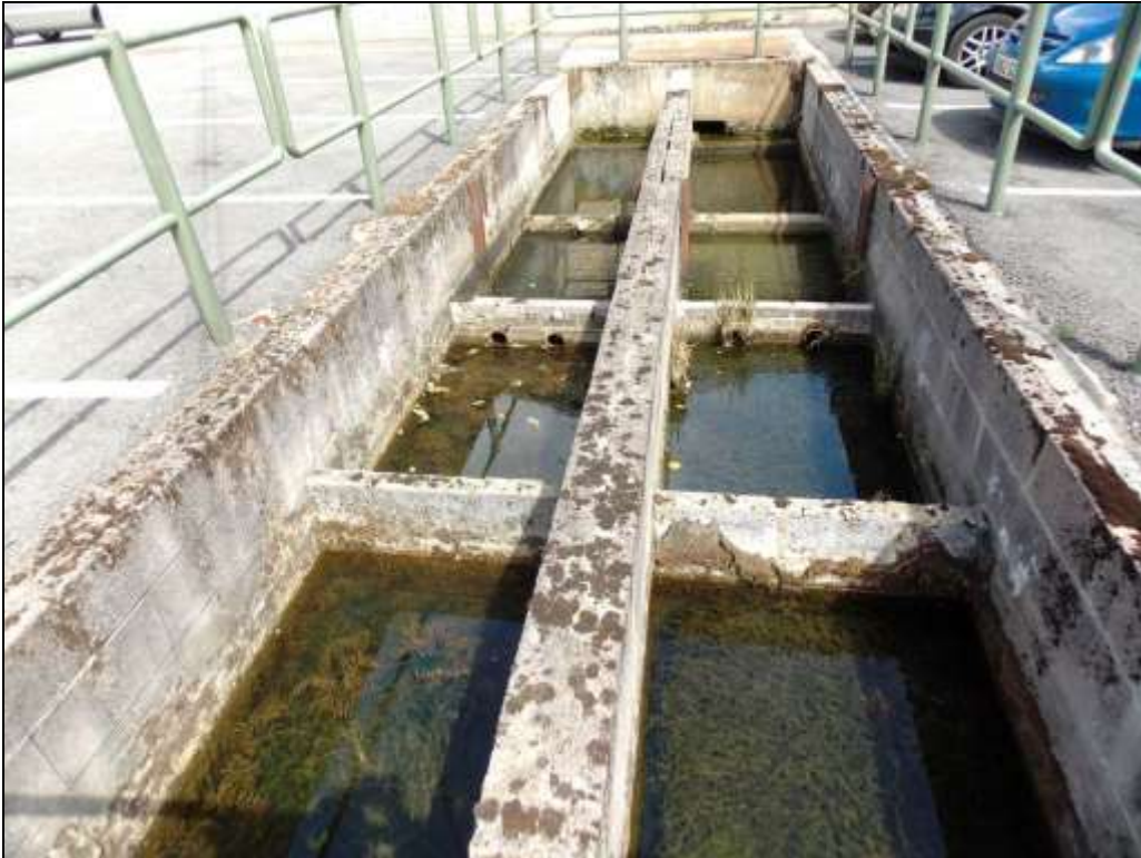
Plate 55: Settling tanks outside the south elevation of the main range of Unit 8, looking north.
