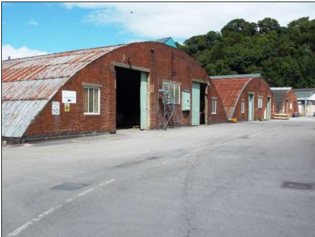
Plate 56: General view of the Nissen huts (Units 10 – 12), looking north.
