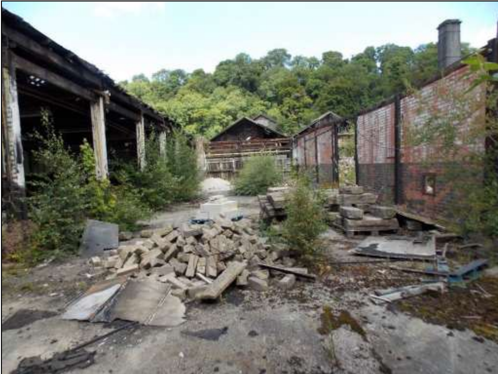
Plate 72: Internal view of Unit 14, looking south.
