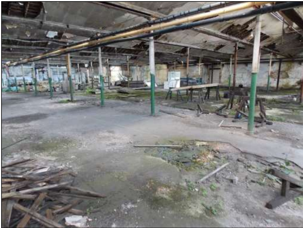
Plate 21: Internal view of the former Mule Spinning Shed, looking south-west.
