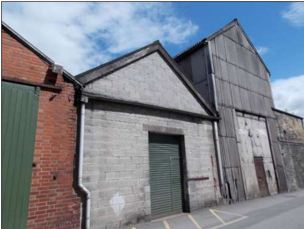
Plate 77: South gable wall of Unit 17, looking north-east.
