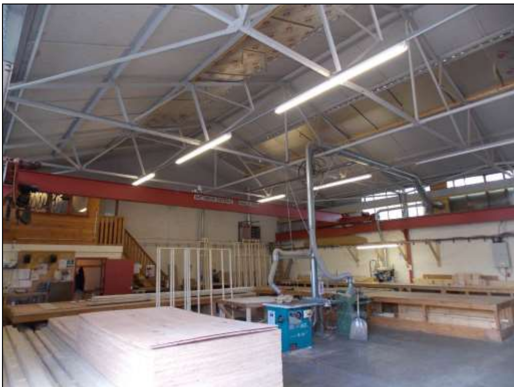
Plate 54: Internal view of Unit 8, looking north-east.
