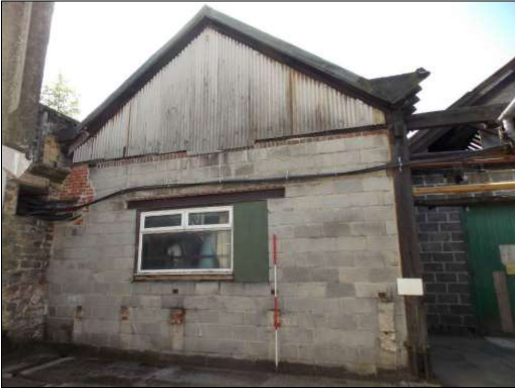
Plate 81: North gable wall of Unit 2, looking south.
