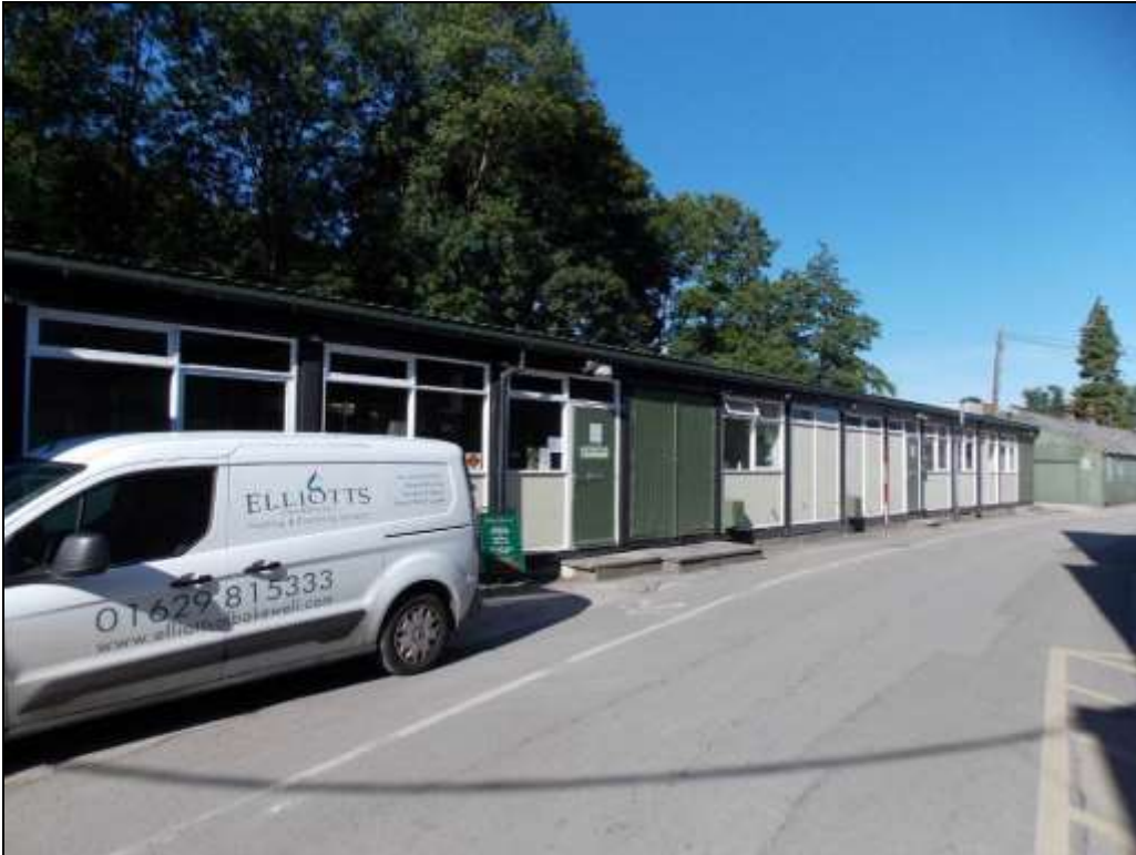
Plate 66: General view of Units 11 and 12, looking west.
