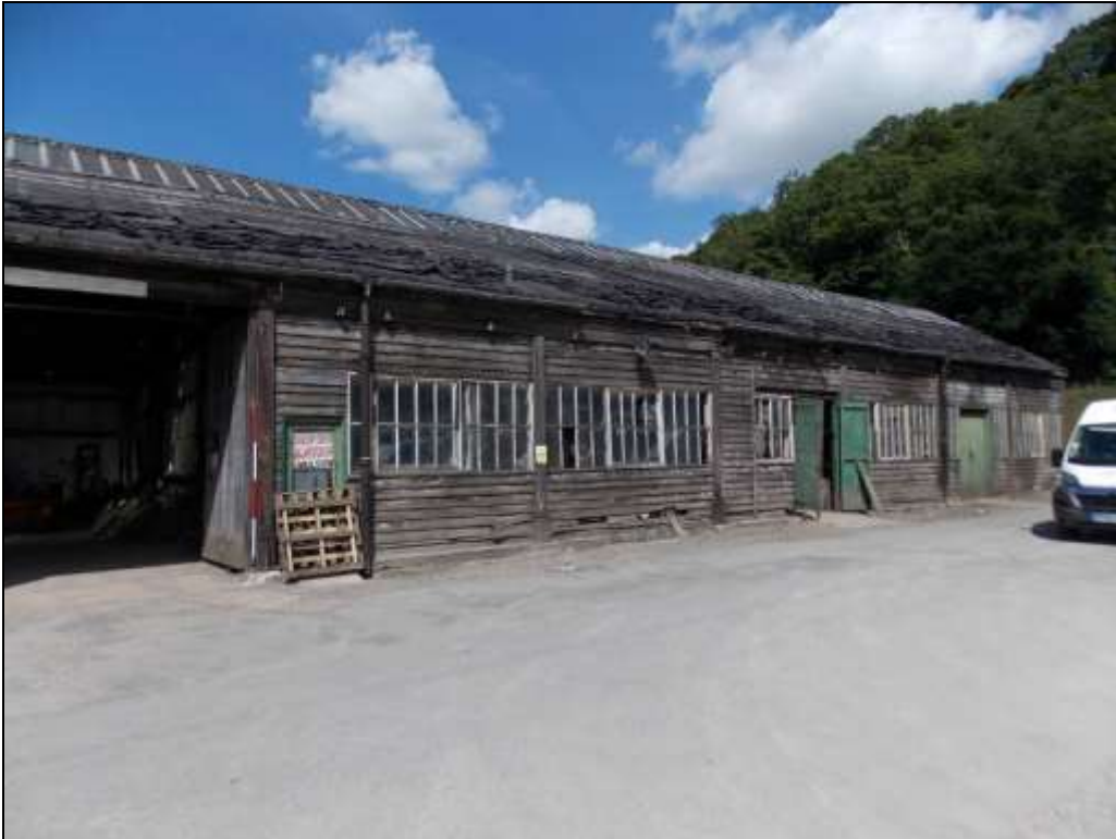
Plate 48: East elevation of Unit 7a, looking north-west.
