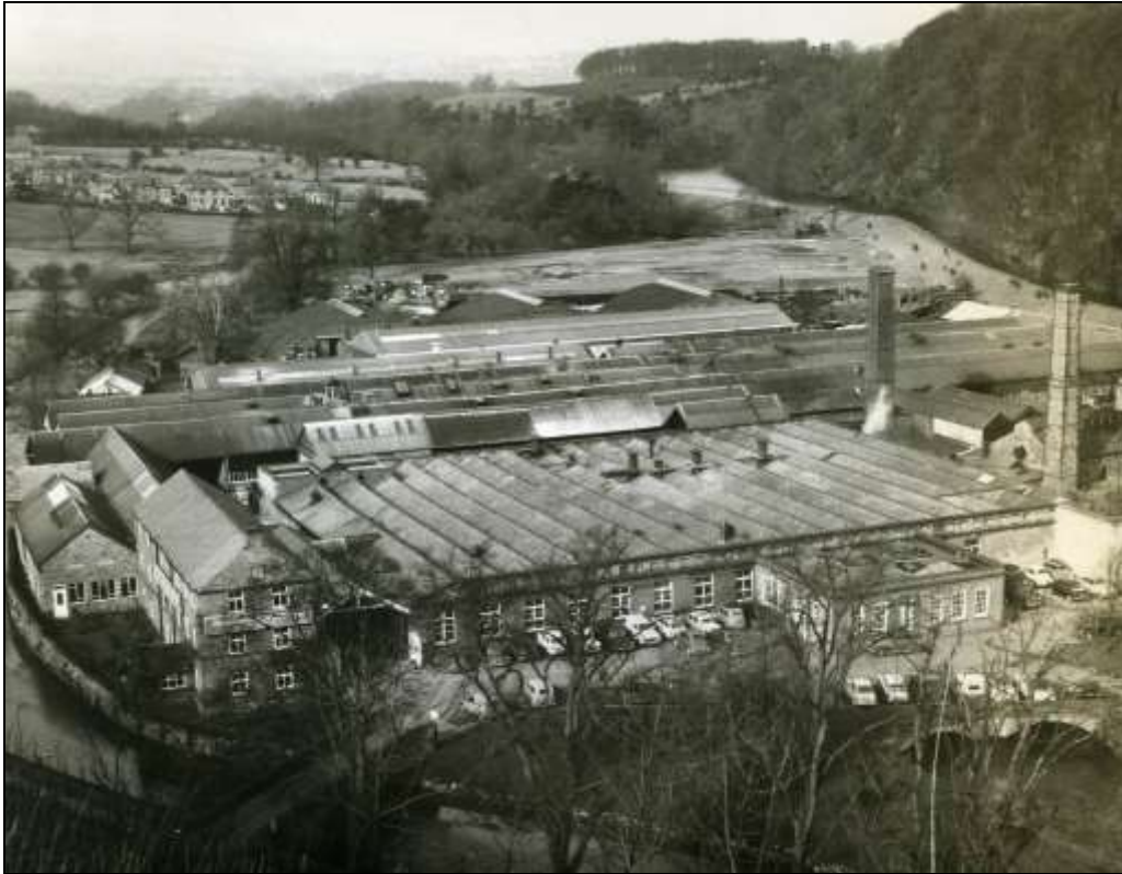
Plate 4: Historical photograph (post 1950) of the works showing the former Mule Spinning Shed.
