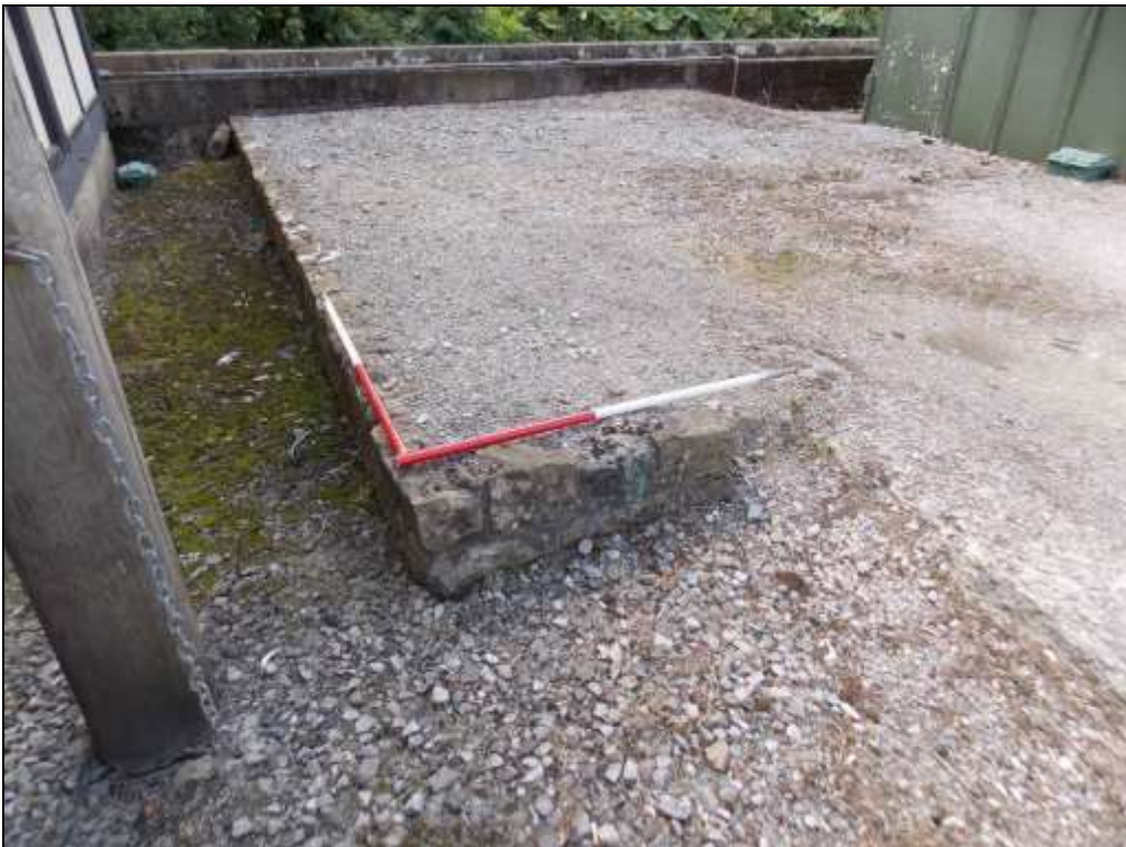
Plate 67: Structural remains adjacent to the west elevation of Units 11 and 12, looking south-west.
