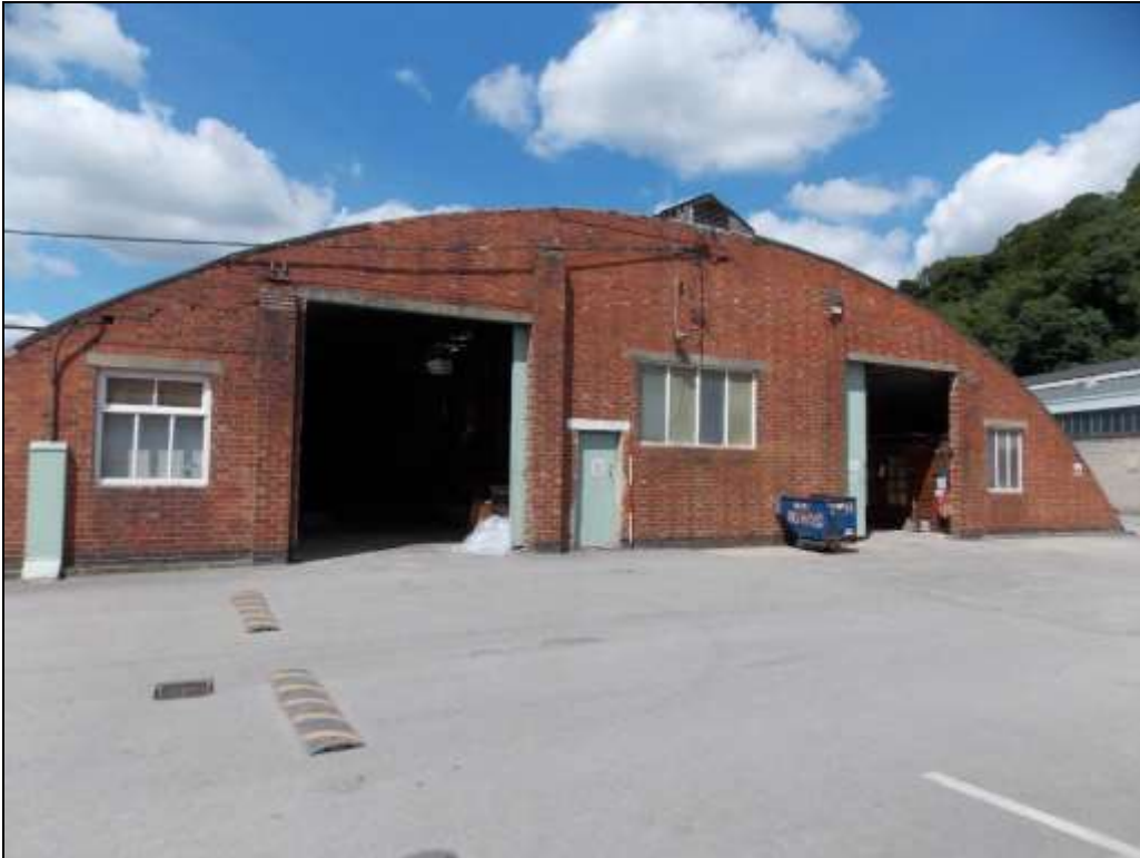
Plate 57: Front elevation of Unit 10, looking west.
