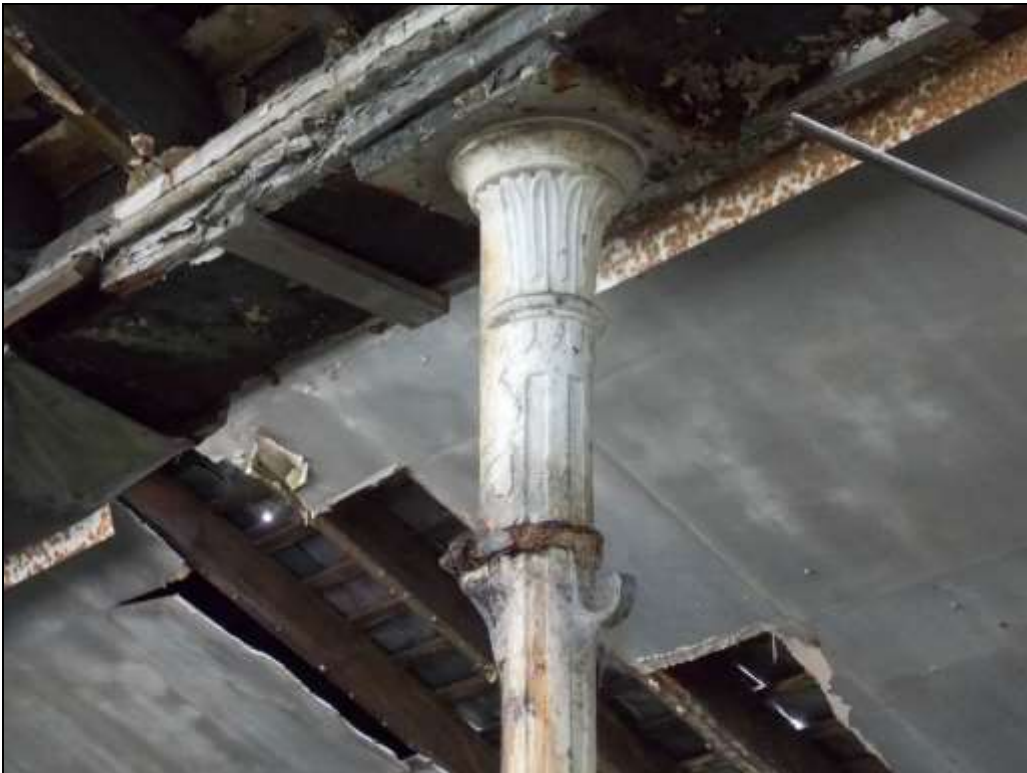
Plate 22: Detail of cast-iron column's capital.
