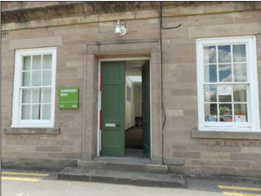
Plate 7: Doorway of Fearnough House, looking west.
