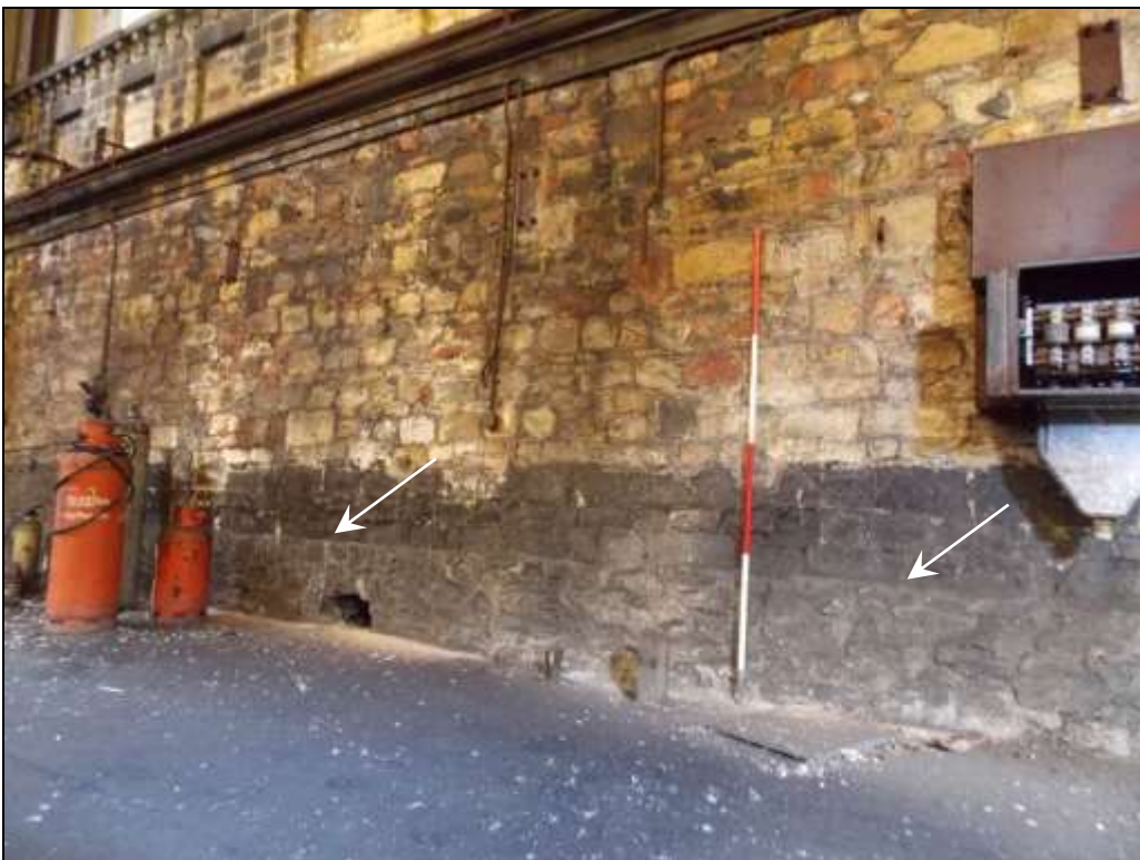
Plate 19: Northern side built over an earlier lower wall (arrows), looking north-east.
