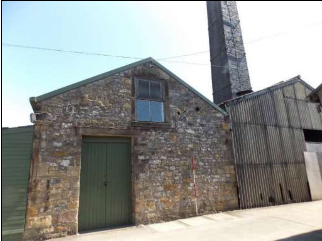
Plate 36: West elevation of Units 16b – d, looking east.
