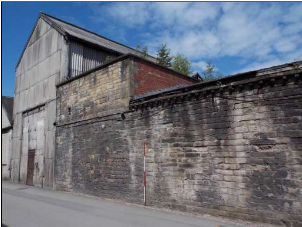
Plate 80: South gable wall of Unit 2, looking north-west.
