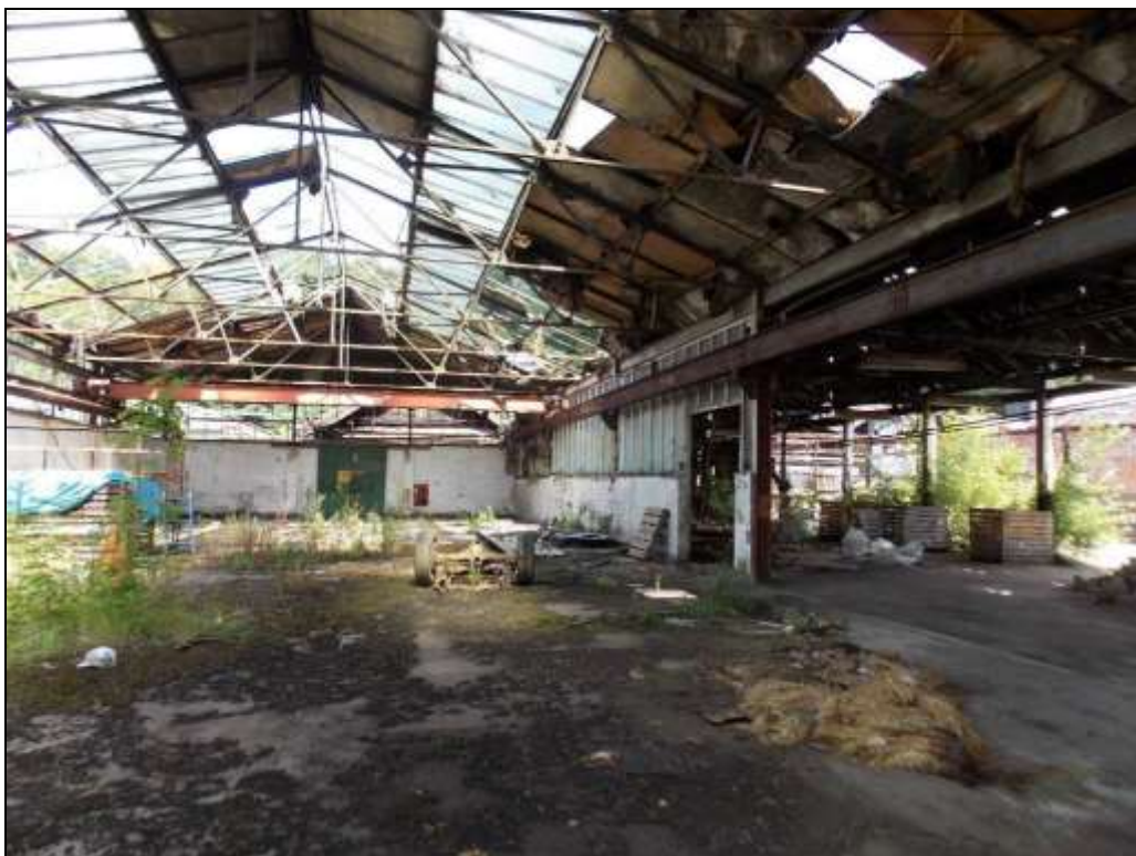
Plate 70: Internal view of Units 5a (right) and 5b (left), looking north.
