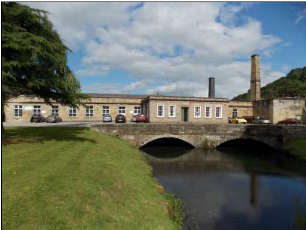
Plate 5: East elevation viewed from the mill stream.
