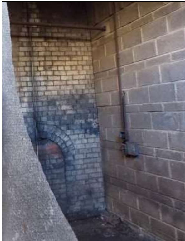
Plate 38: Detail of flue opening, looking east.
