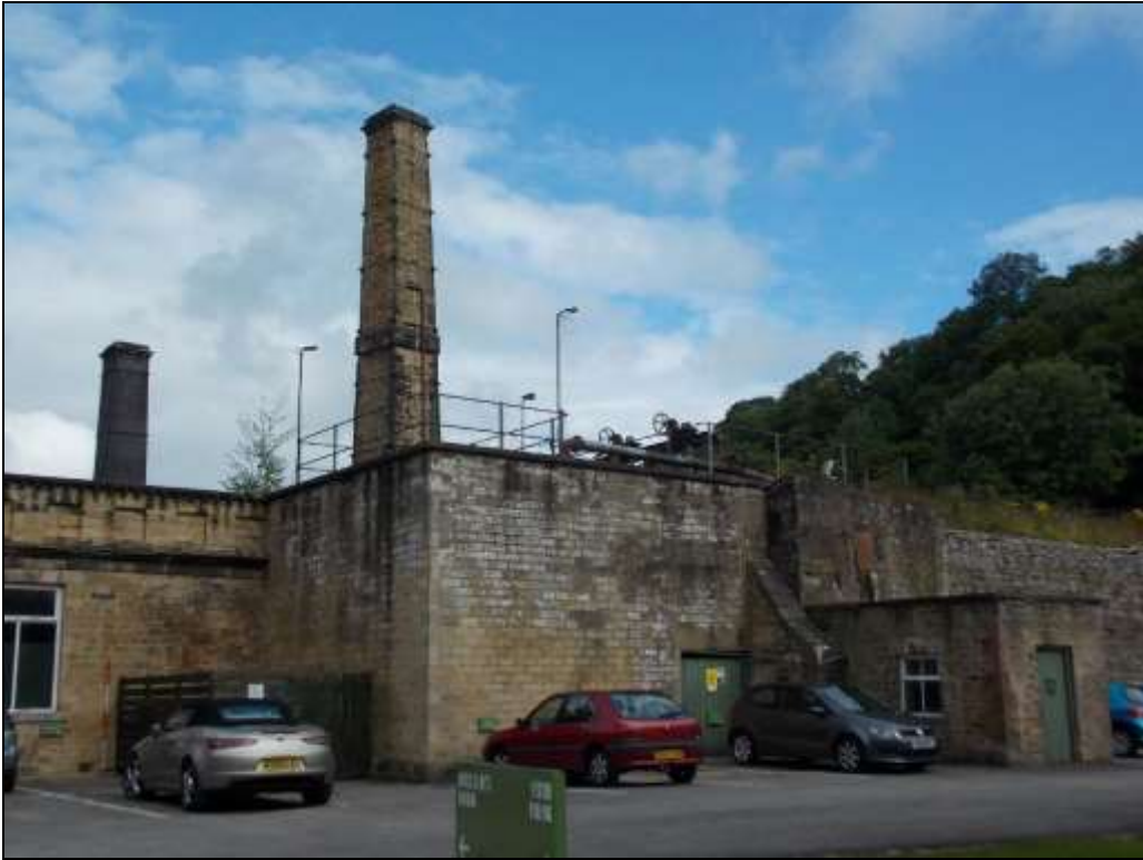
Plate 10: Projecting water wheel housing, looking north-west.
