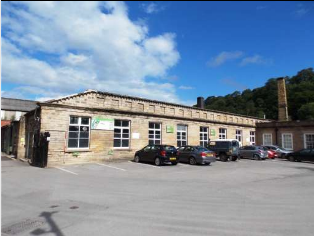
Plate 6: Southern side of the east elevation, looking north-west.
