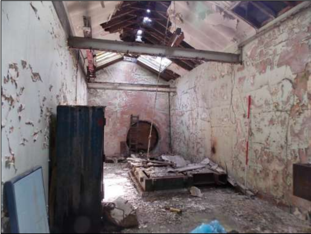
Plate 26: Plant room with circular hole of former turbine, looking east.
