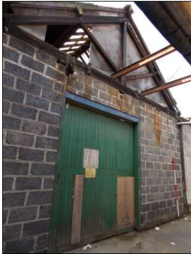
Plate 78: North gable wall of Unit 17, looking south-west.
