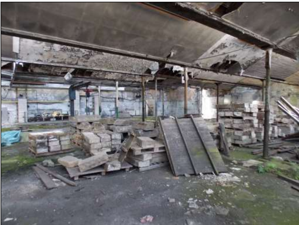
Plate 23: Reclaimed masonry stored within the main workshop, looking east.
