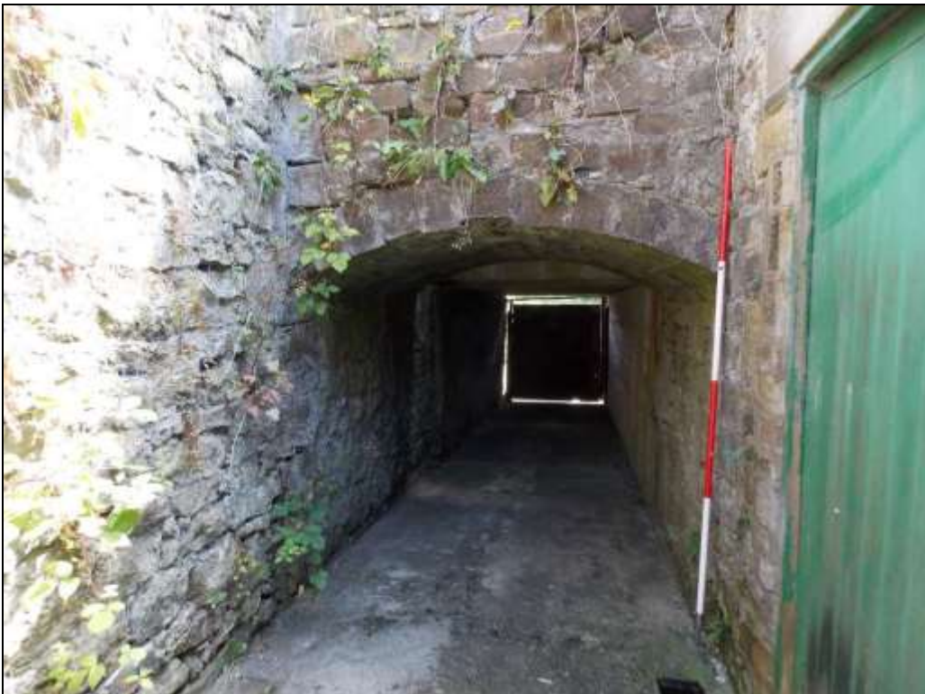
Plate 13: Original archway beneath the former water wheel housing, looking east.
