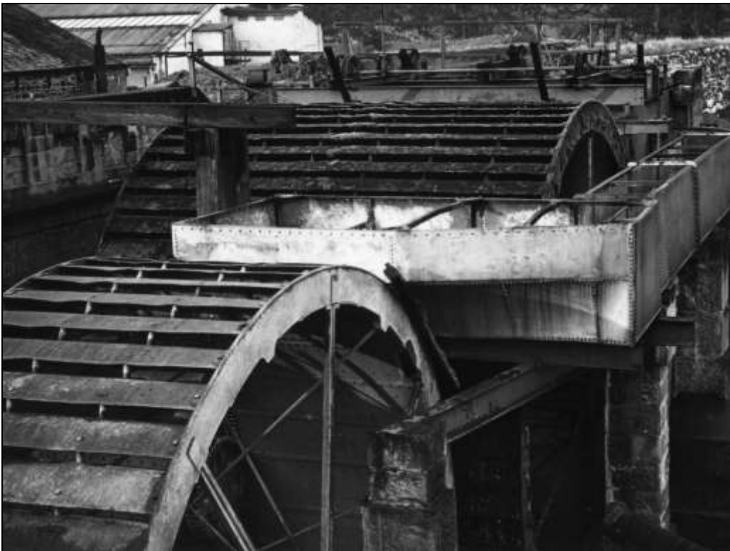
Plate 15: Historical photograph showing the former wheels with a metal launder for the small wheel.
