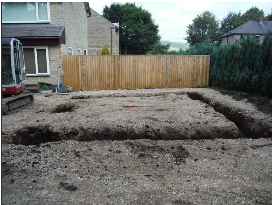
Figure 6. The excavation facing north. Scale 1m.
