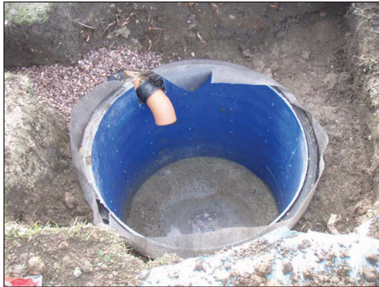
Figure 3. View of completed soakaway four.
