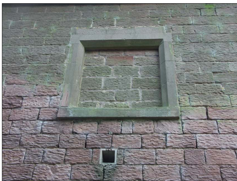
Fig. 12 Blocked up window at eastern end of north-east facing elevation
