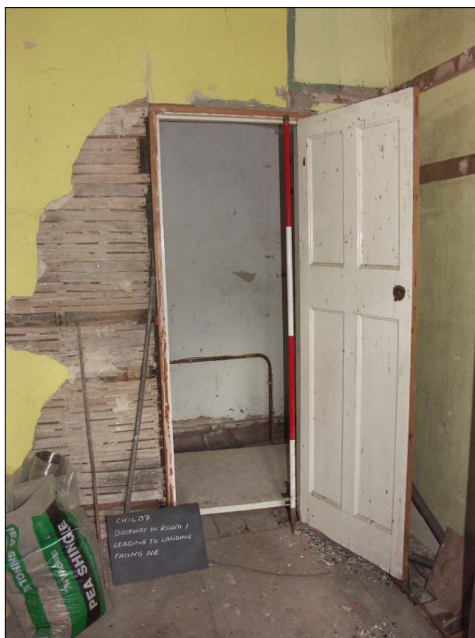
Fig. 40 Room One doorway showing lath and plaster construction, scale 2m
