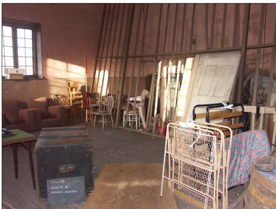
Fig. 44 Room Four facing north, the wooden fram is a laundry drying rack, scale 2m
