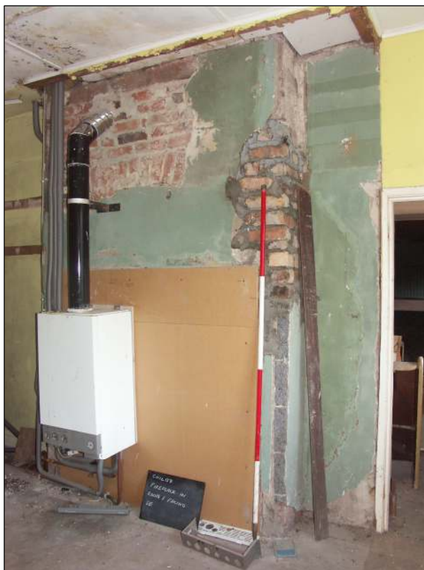
Fig. 41 Fireplace in Room One showing brick construction, scale 2m
