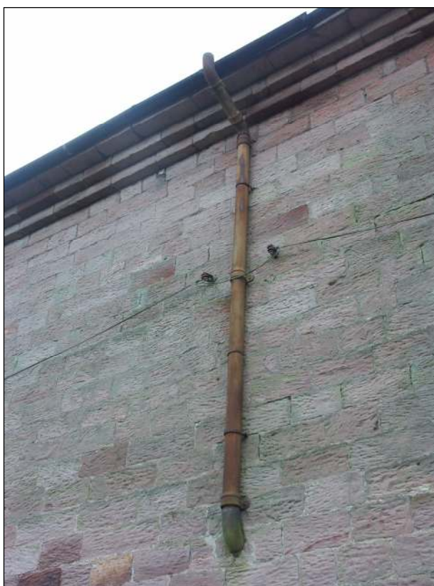
Fig. 8 Ventilation flue at west end of north-east facing elevation
