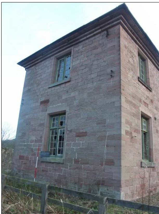
Fig. 24 North-west facing elevation, scale 2m
