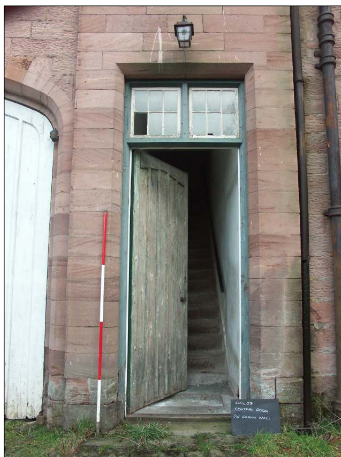
Fig. 20 East central doorway in south-west facing elevation, scale 2m
