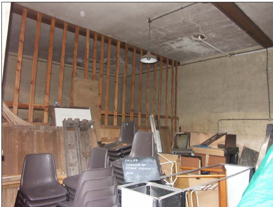
Fig. 28 The stables facing north-west
