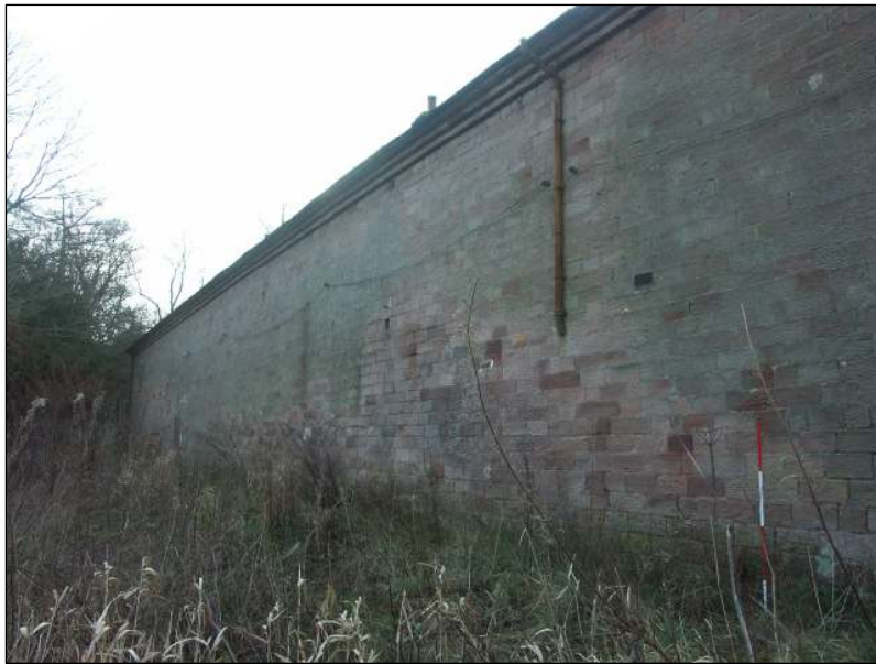
Fig. 5 North-east facing elevation looking south, scales 2 x 2m
