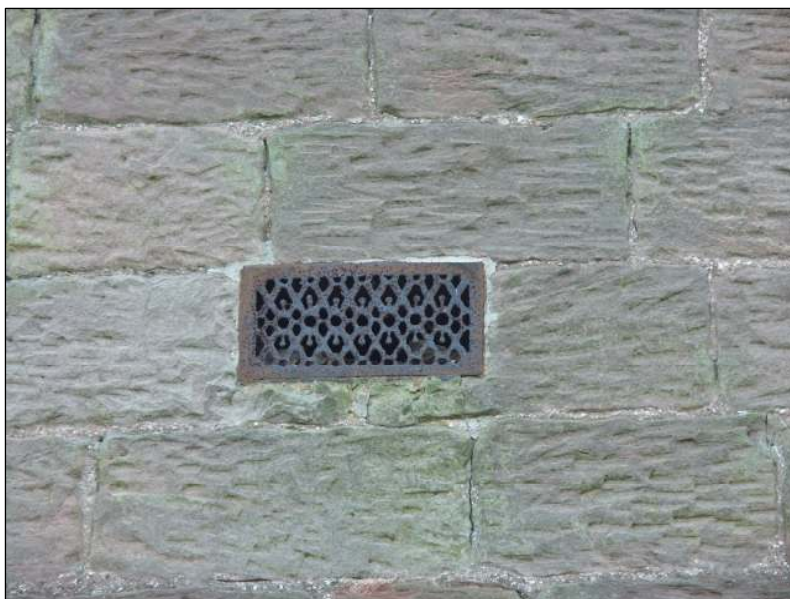
Fig. 7 Air ventilation grate at west end of north-east facing elevation
