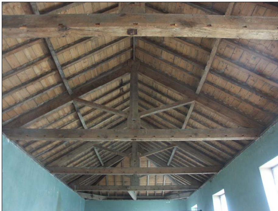
Fig. 39 Roof construction viewed from the gallery, looking South-east
