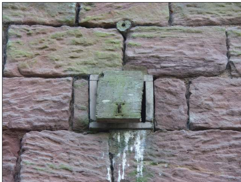
Fig. 10 Pigeon trap at eastern end of north-east facing elevation
