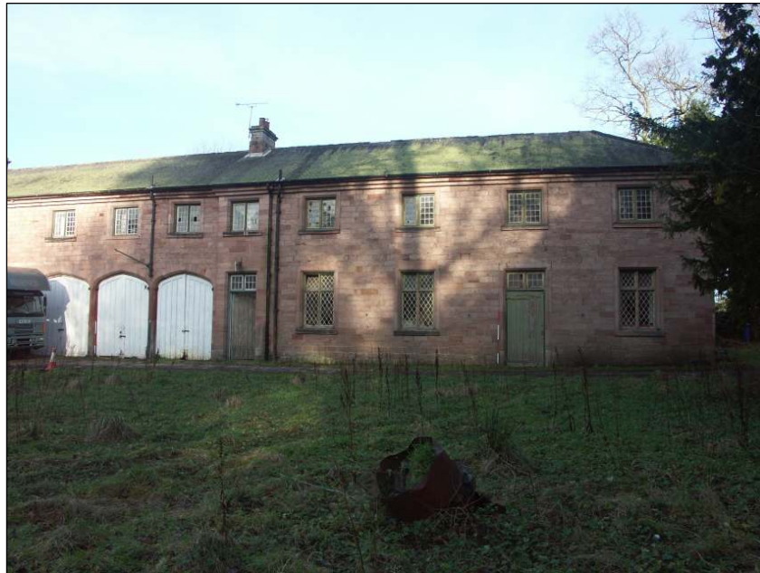
Fig. 14 South-west facing elevation looking north-east, scale 2 x 2m
