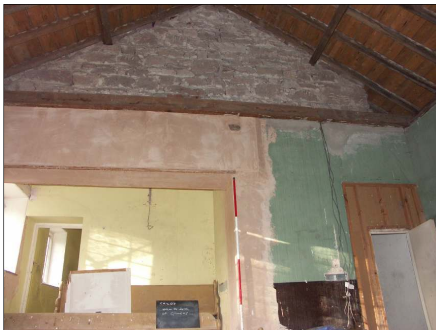
Fig. 38 Rear gallery wall showing sandstone block wall construction, scale 2m
