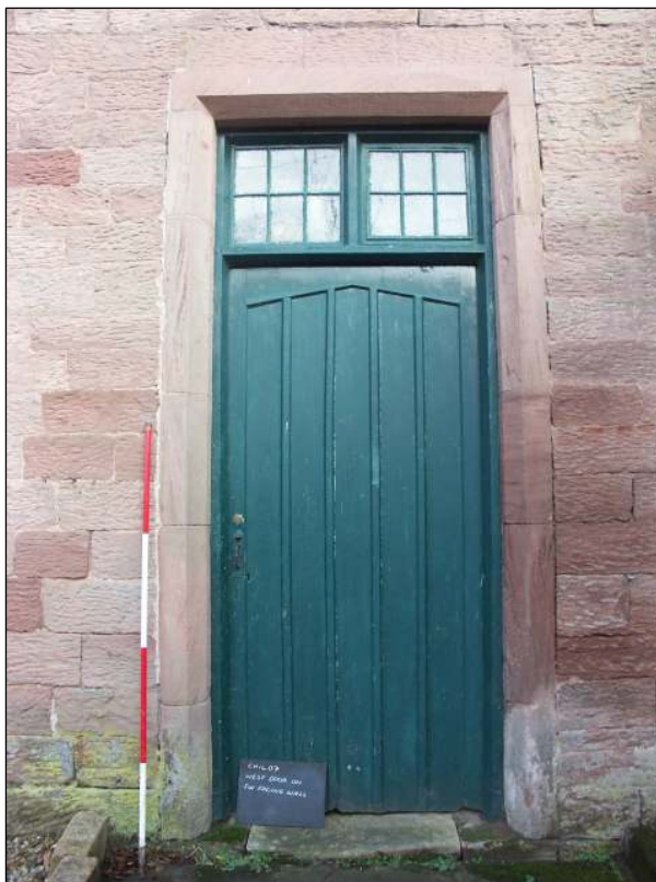
Fig. 23 Western doorway in south-west facing elevation, scale 2m
