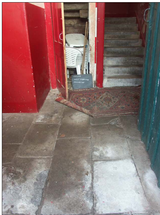
Fig. 32 Stone slab flooring in the western passageway, scale 2m
