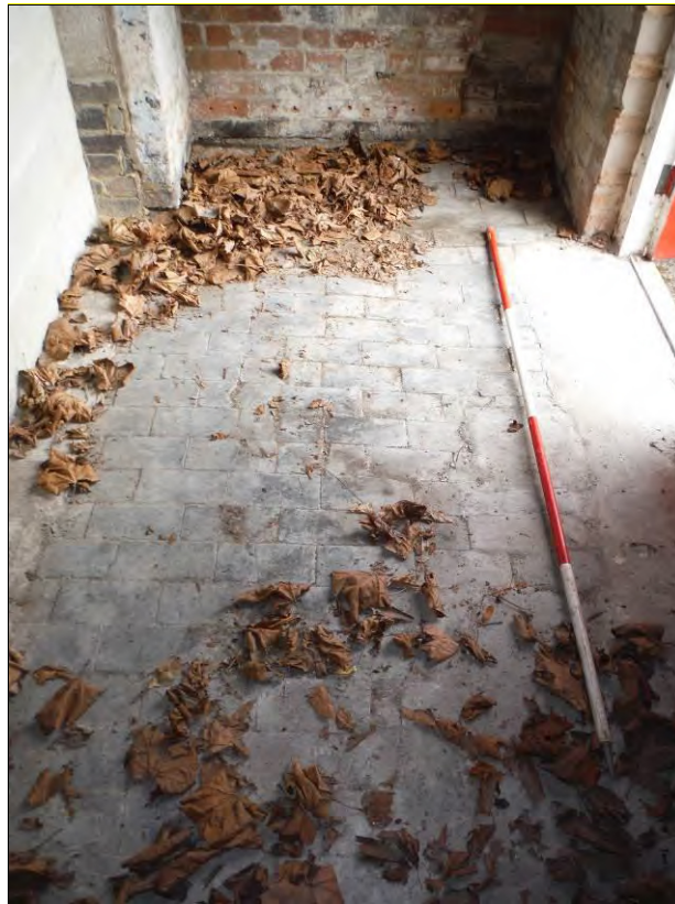
Figure 41: Detail of the brick floor in Room G10 (Scale = 2m).
