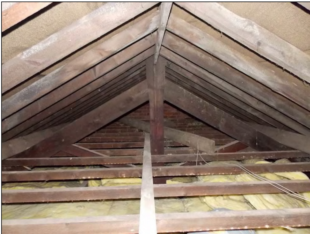
Figure 88: King-post truss over Room F7.
