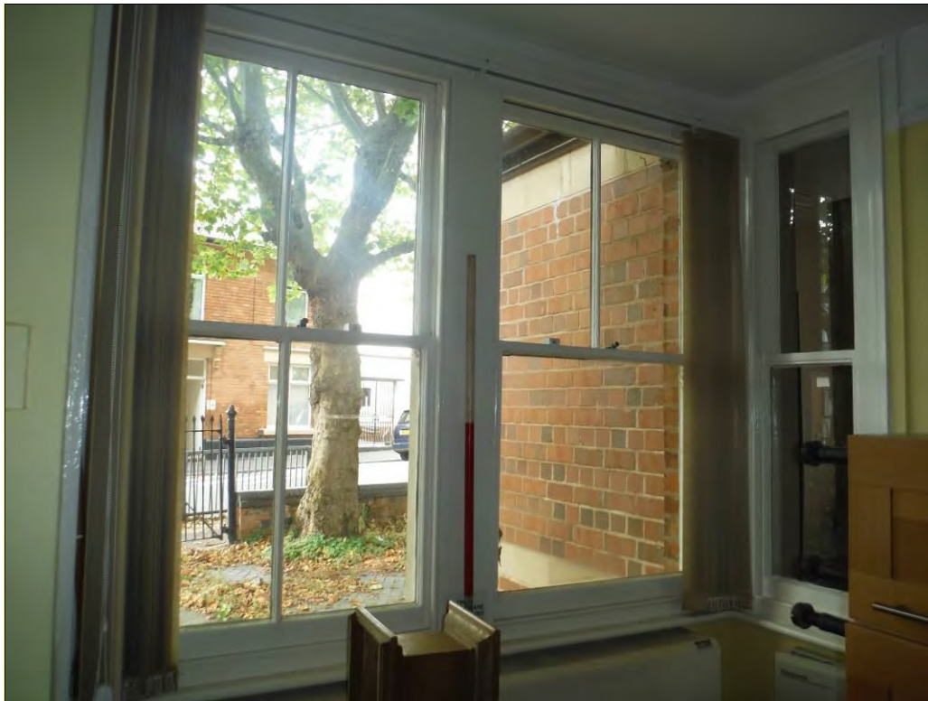
Figure 28: Detail of the inserted three-light bay window in the south wall of Room G2 (Scale = 1m).
