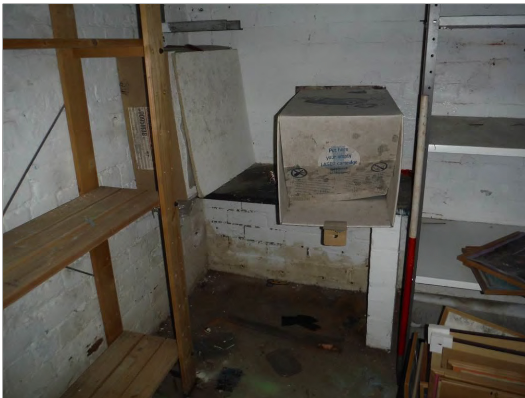
Figure 64: Inserted workbench in the south-west corner of Room B2 (Scale = 1m).
