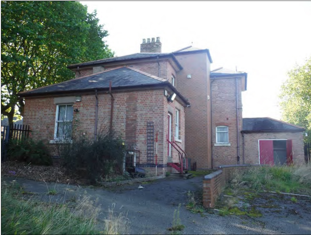
Figure 23: East elevation, looking west (Scale = 2m).
