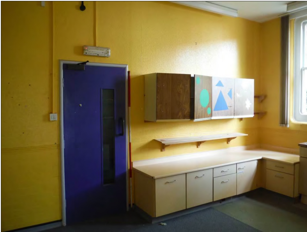
Figure 55: View south-west within Room G16 (Scale = 2m).
