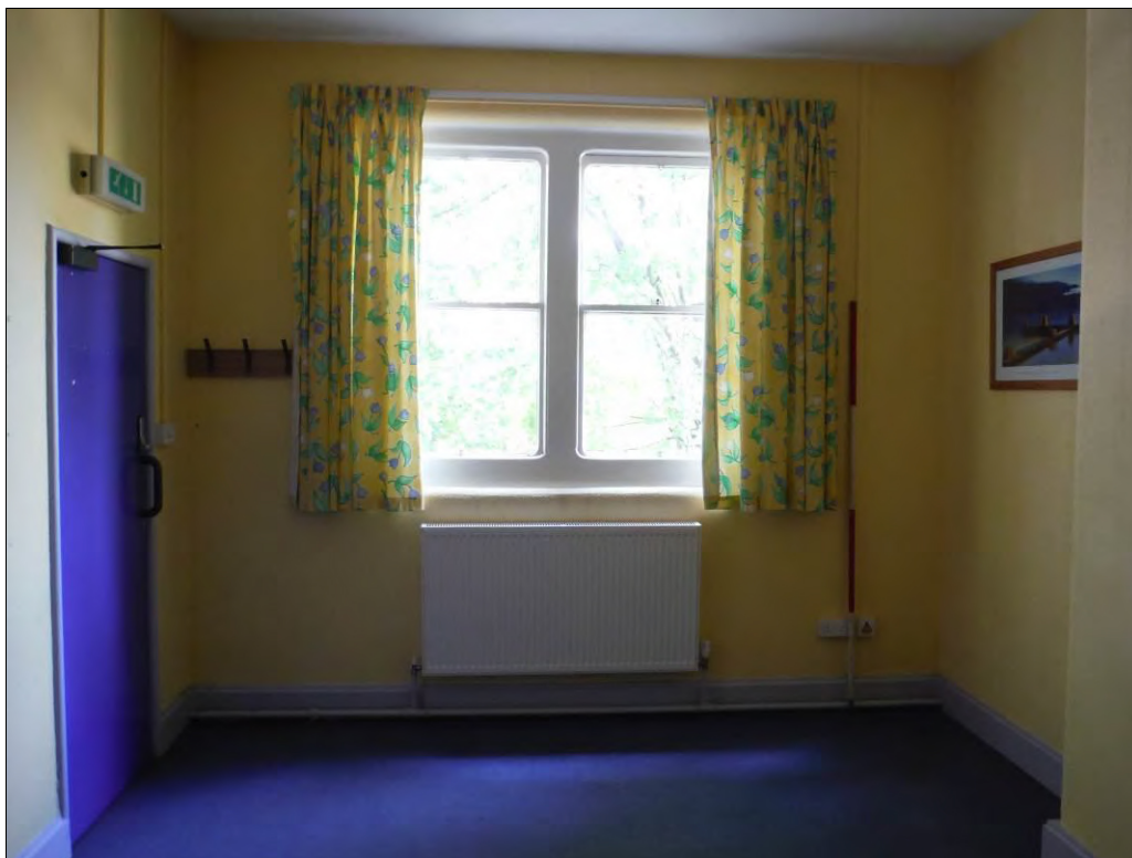
Figure 83: West wall of Room F12 (Scale = 2m).
