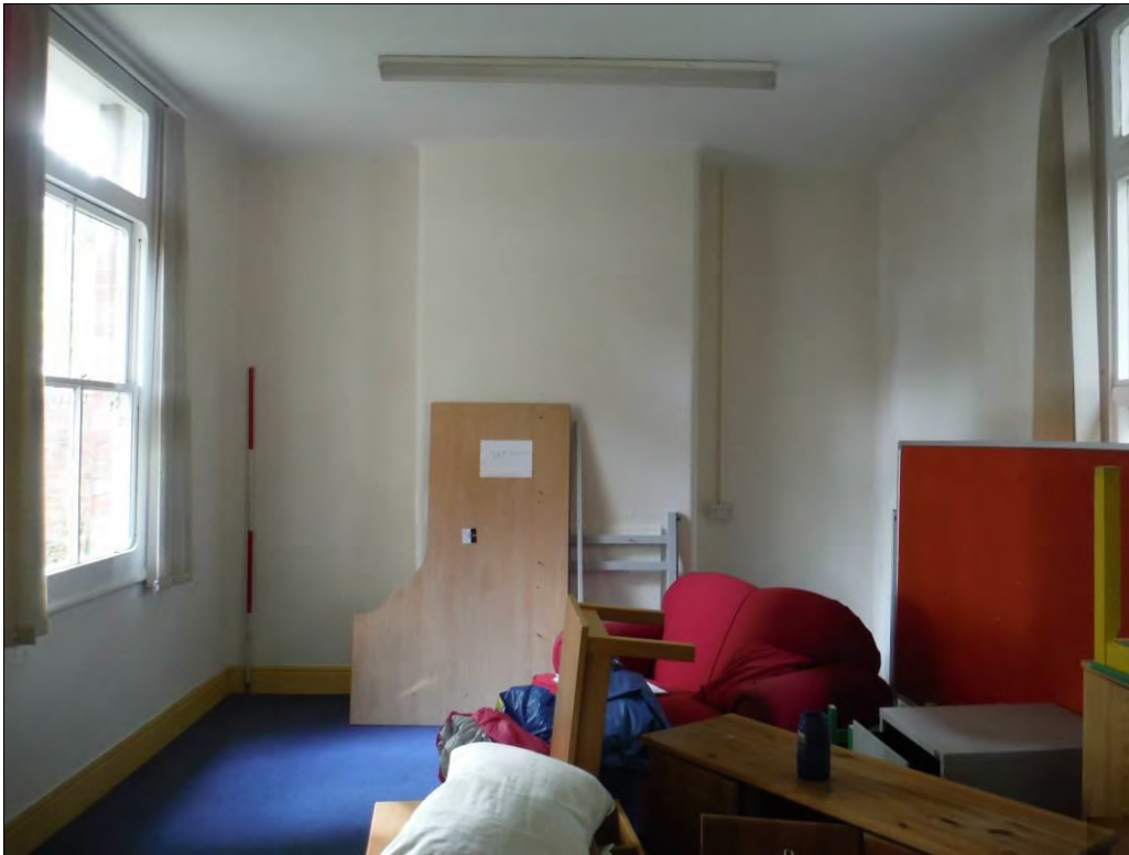
Figure 51: South wall of Room G14 (Scale = 2m).
