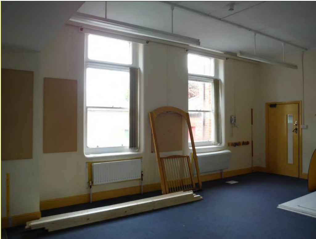
Figure 47: North wall of Room G13a (Scale = 2m).
