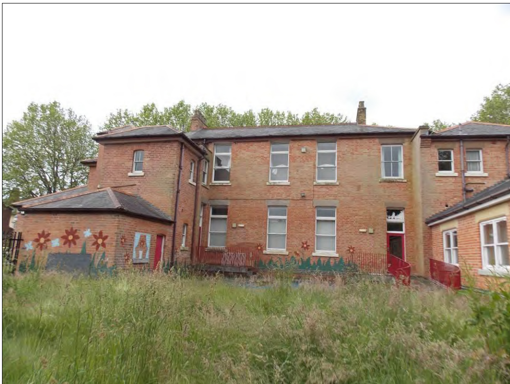
Figure 10: General view of the north elevation of the Sanatorium building, particularly showing the style of its roof, looking south.
