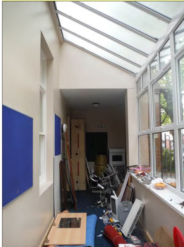
Figure 24: View east within Room G1 looking towards the porch (Scale = 2m).
