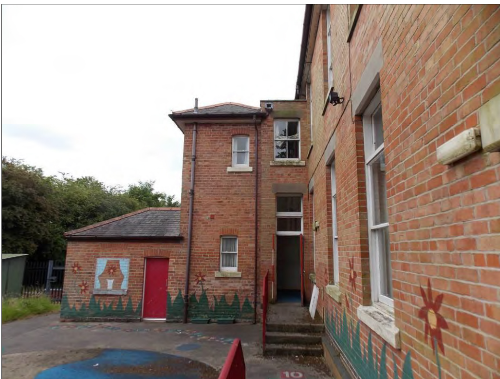
Figure 22: West elevation of the crossing, looking east (Scale = 2m).
