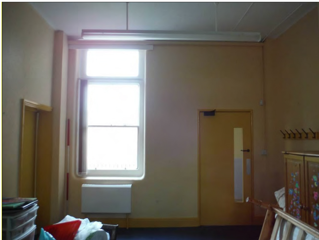
Figure 43: North wall of Room G12 (Scale = 2m).
