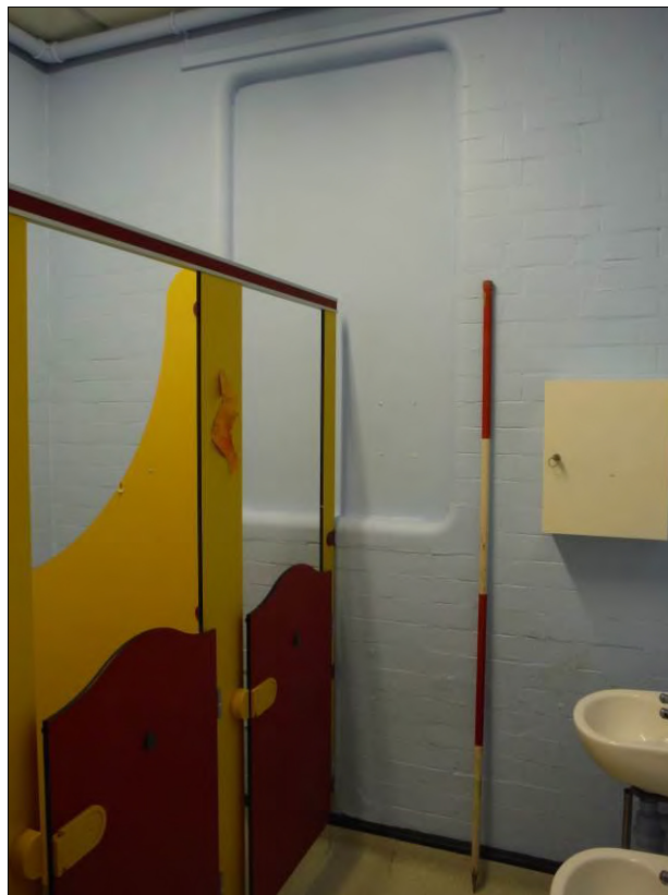
Figure 57: North wall of Room G18 showing blocked original window (Scale = 2m).
