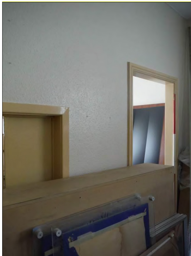
Figure 35: North wall of Room G5 (Scale = 2m).
