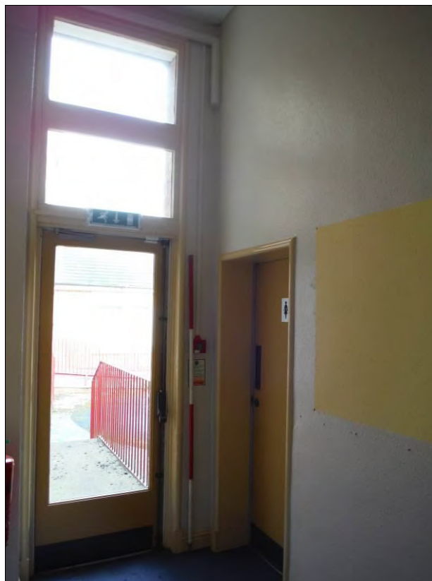
Figure 37: View north-west within Room G7 (Scale =2m).
