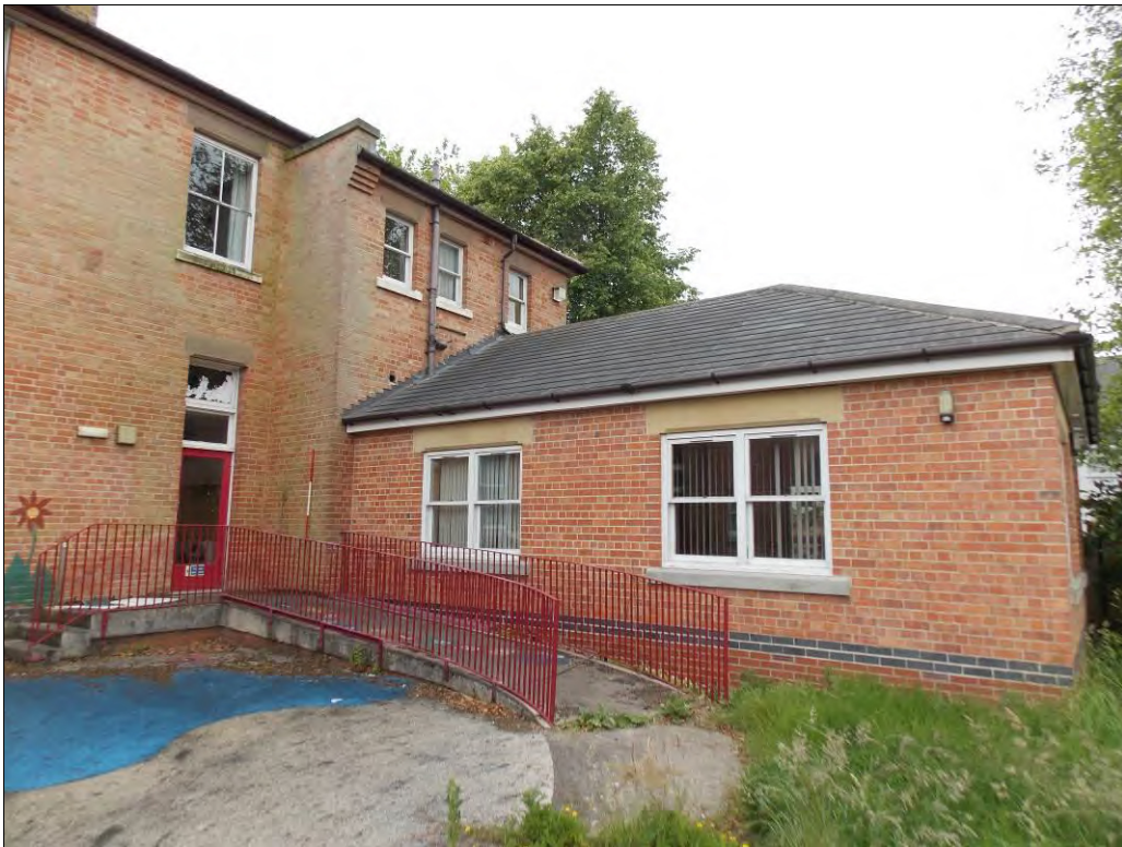
Figure 21: North elevation, looking south-west (Scale = 2m).
