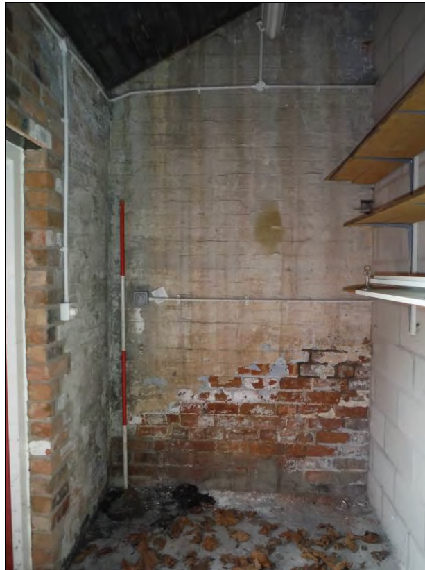
Figure 40: View south within Room G10 (Scale = 2m).
