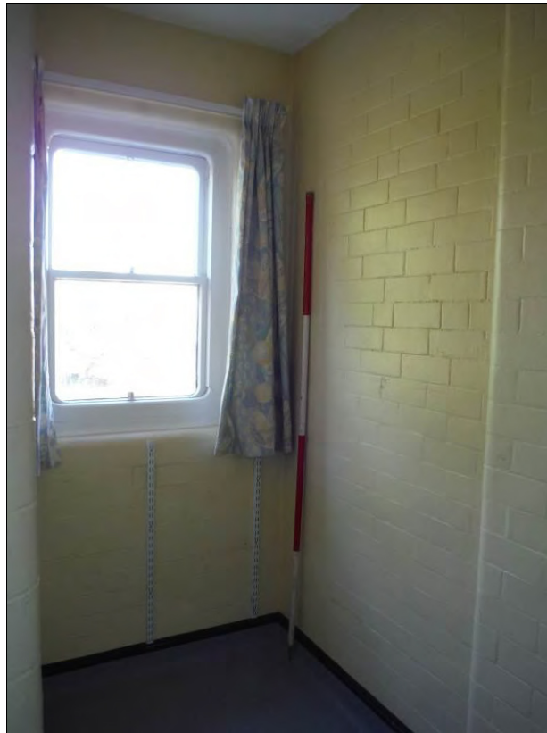
Figure 79: North wall of the east side of Room F9 (Scale = 2m).
