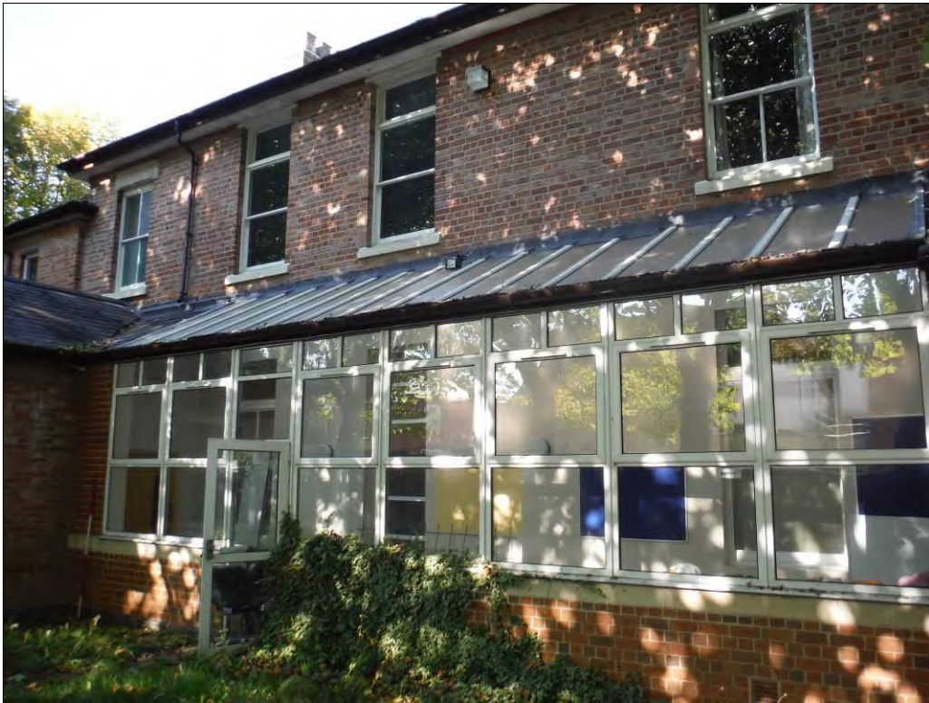
Figure 12: Central section of the south elevation, looking north-west (Scale = 2m).
