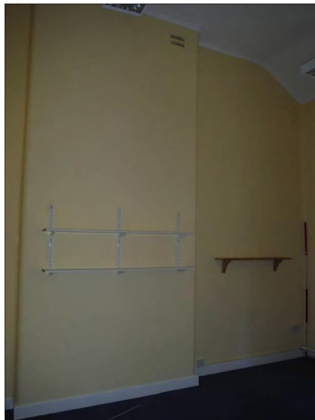
Figure 72: East wall of Room F5 (Scale = 2m).
