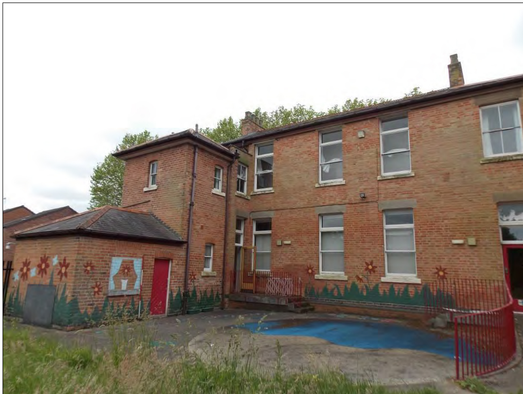
Figure 20: North elevation, looking south-east (Scale = 2m).
