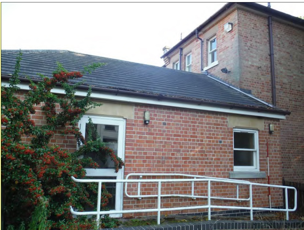
Figure 18: West elevation of northwards extension, looking south-east (Scale = 2m).
