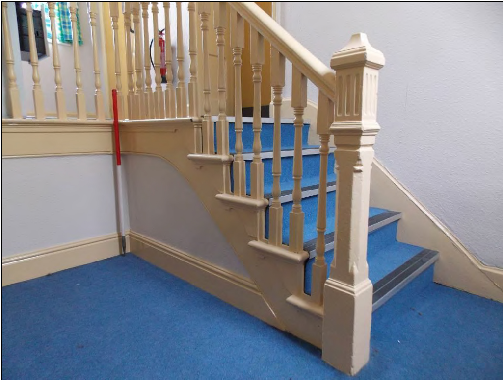
Figure 77: Detail of truncated staircase in Room F8 (Scale = 1m).
