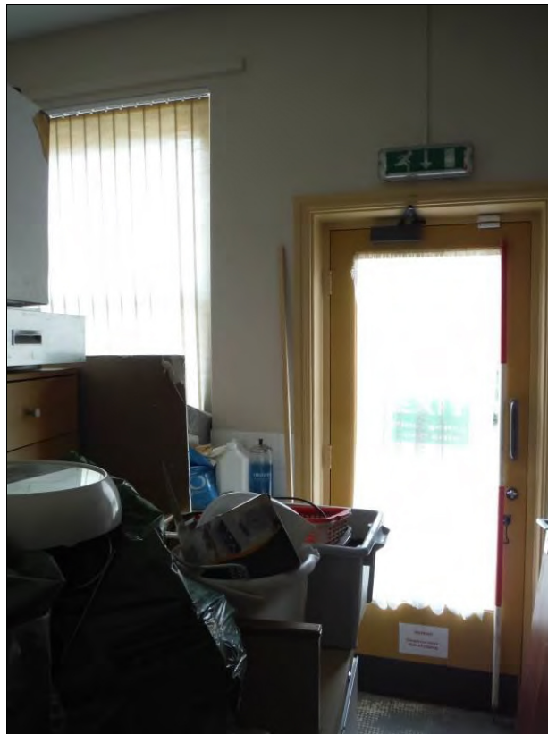
Figure 36: North wall of Room G6 (Scale = 2m).
