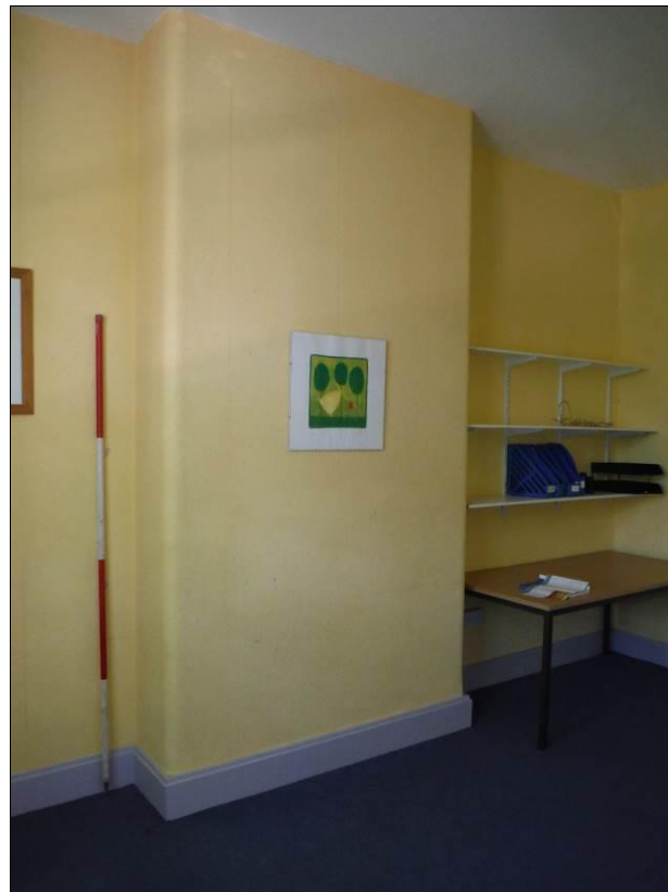
Figure 82: Chimney breast in the north wall of Room F12 (Scale = 2m).
