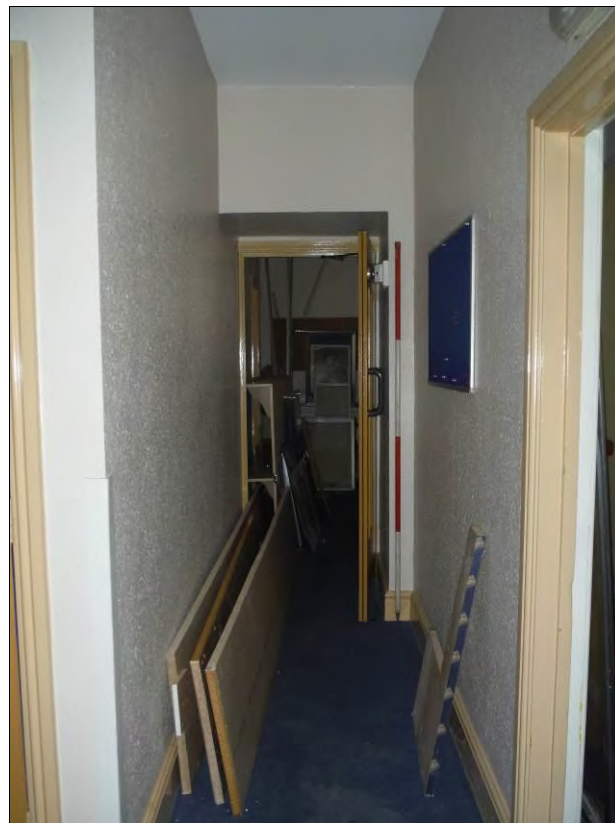
Figure 29: View east within Room G3 along the inserted corridor to Room G5 (Scale = 2m).
