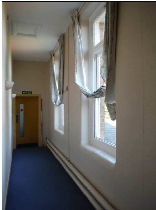
Figure 71: View west within Room F6 (Scale= 2m).
