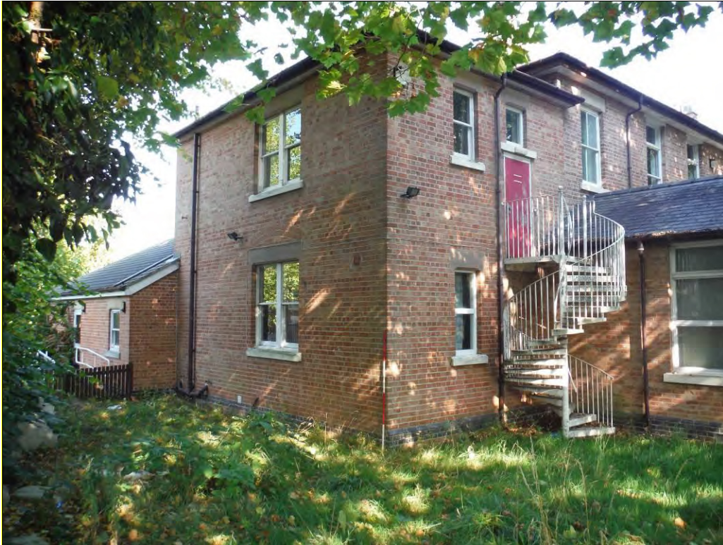
Figure 17: West elevation, looking north-east (Scale = 2m).
