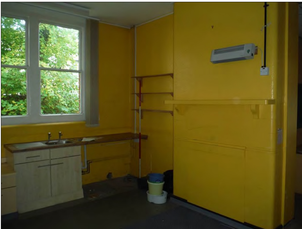
Figure 54: View north-west within Room G16 (Scale = 2m).
