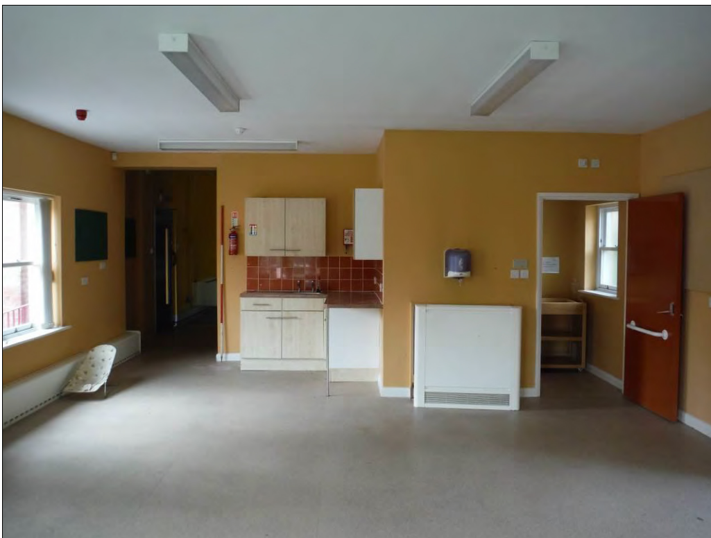
Figure 59: View south within Room G19, showing the partitioned off toilet cubicle, Room G20, in the south-west corner with its western window (Scale = 2m).
