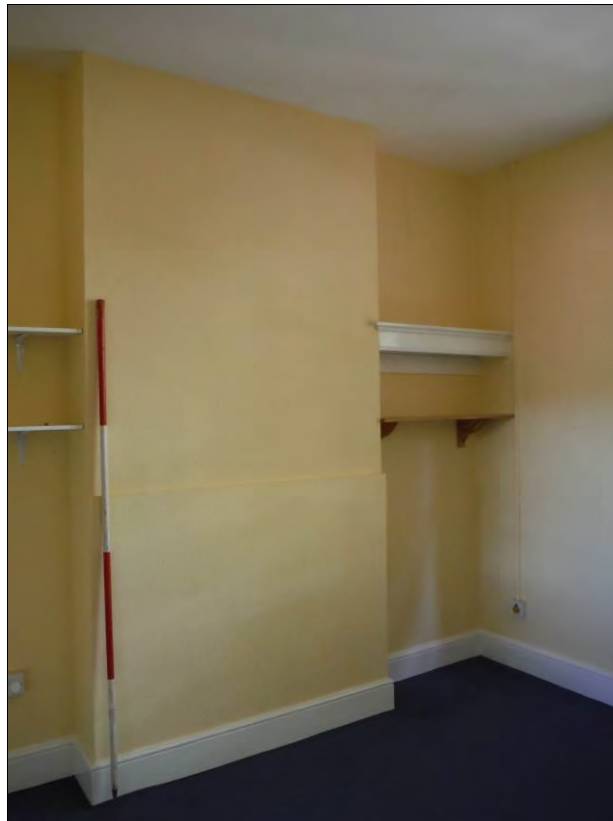
Figure 86: East wall of Room F14 (Scale = 2m).
