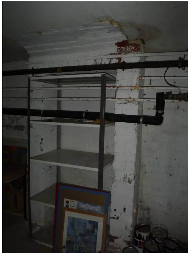
Figure 63: Brick piers against the east wall of Room B2 supporting the fireplace and hearth in Room G2 above.
