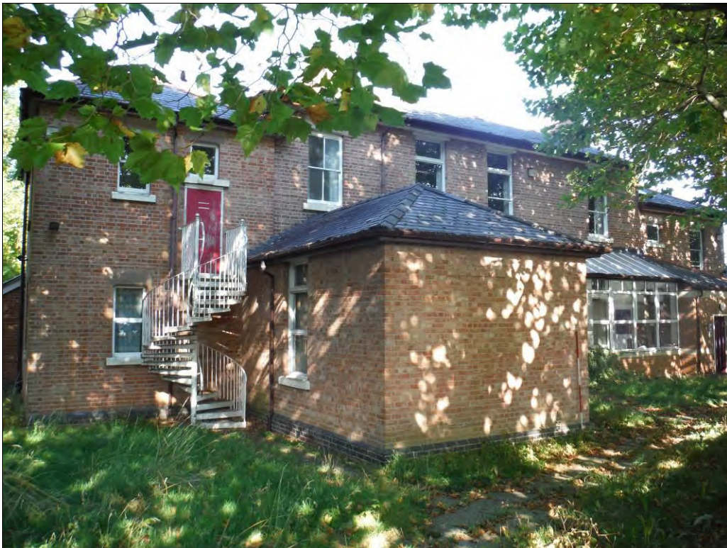
Figure 13: West end of the south elevation, looking north-north-east (Scale = 2m).
