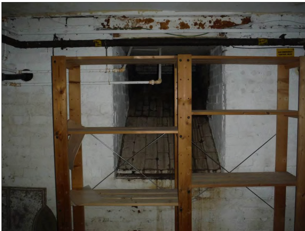
Figure 62: Coal chute in the south wall of Room B2.
