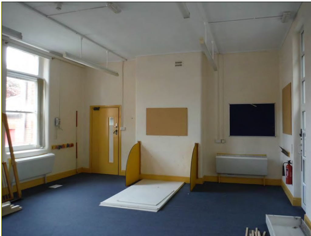
Figure 44: West wall of Room G13a (Scale = 2m).
