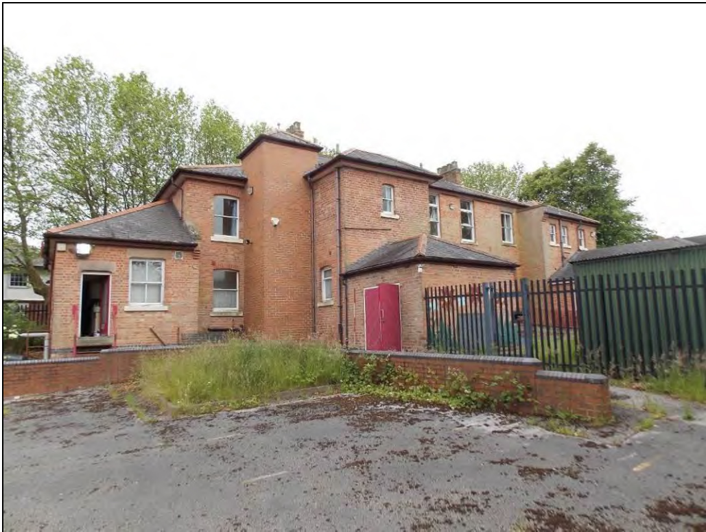
Figure 19: East end of the north elevation, looking south-west (Scale = 2m).
