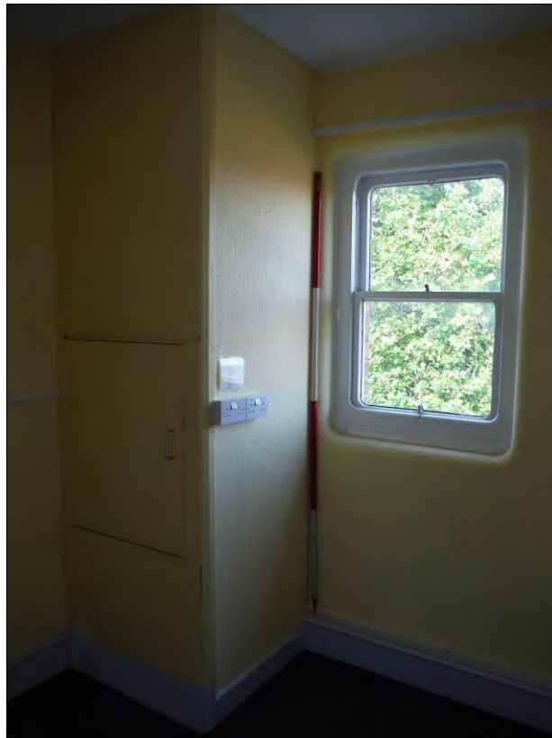
Figure 80: North wall of Room F10 showing inserted boiler cupboard (Scale = 2m).
