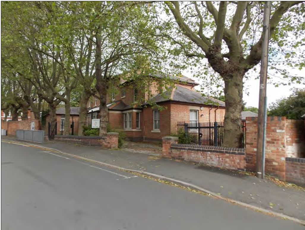
Figure 9: General view of the Sanatorium Building from Stepping Lane, looking north-west.
