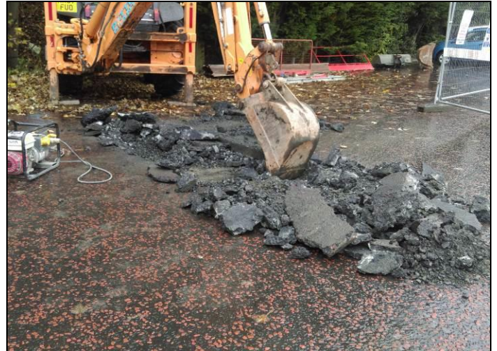
Excavation of the trench through the car park tarmac.
