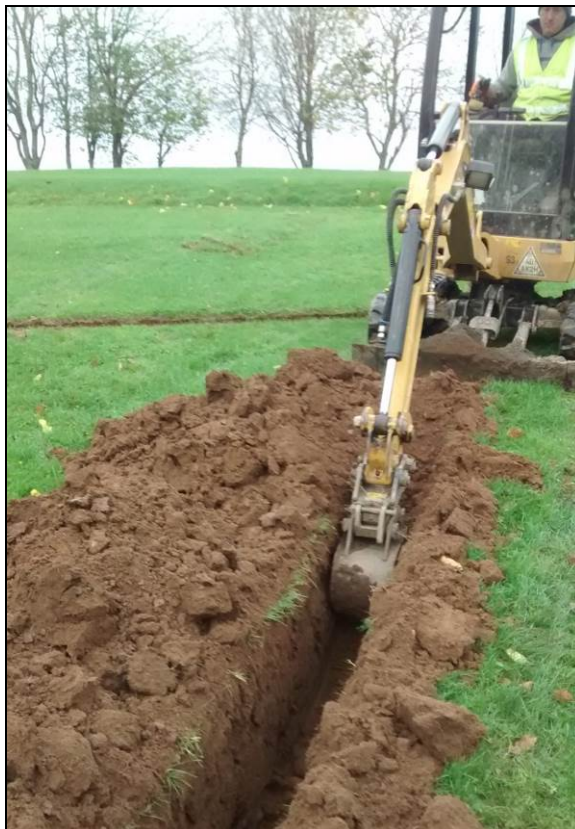
Figure 3. Excavation of electricity cable trenches. Phase A.
