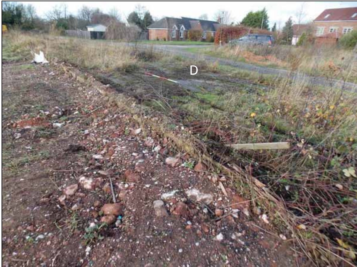
Figure 14: Structure D adjacent to the main east/west trackway, looking north-east (scale 2m).
