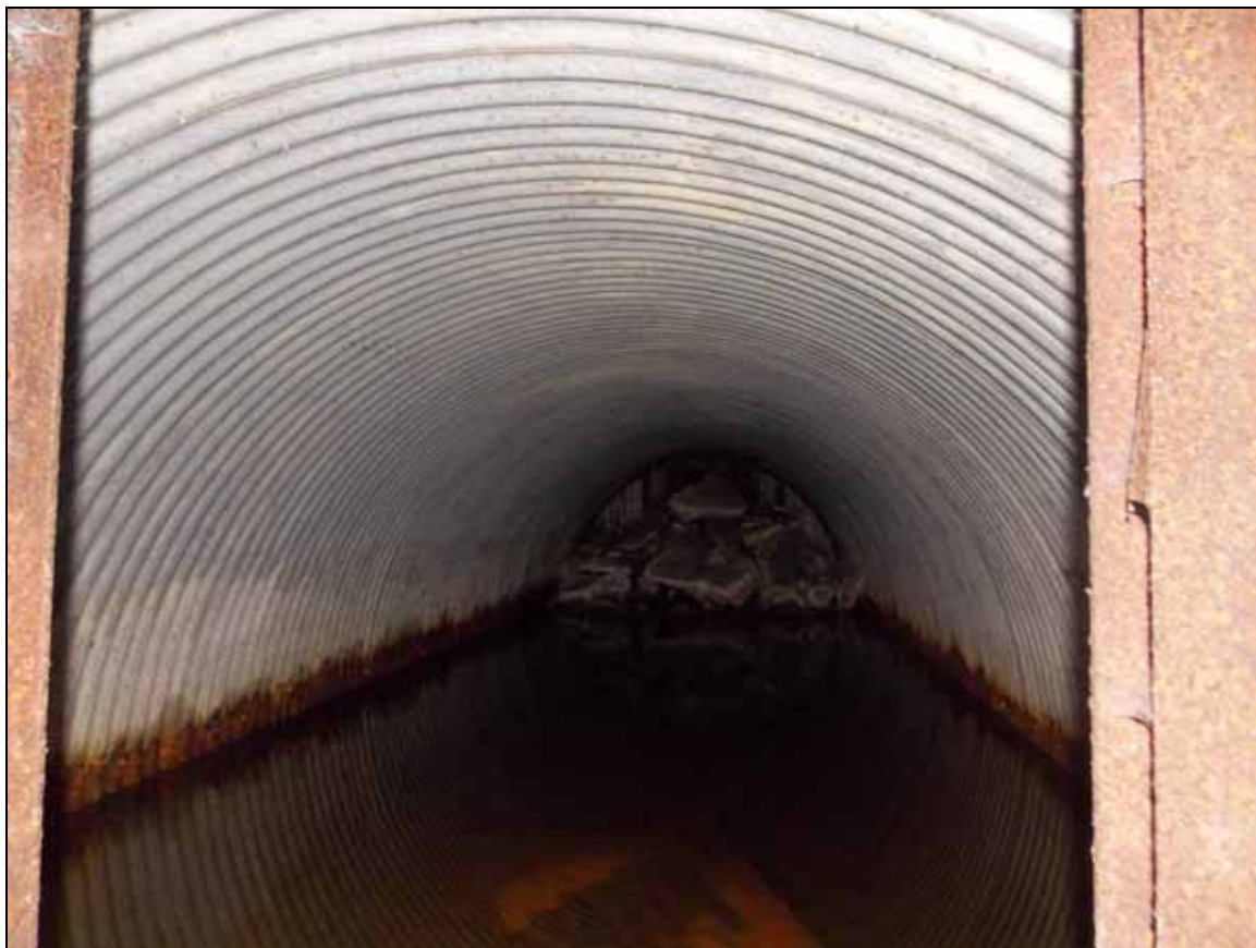
Figure 13: Internal view of the air-raid shelter Structure C, looking east.
