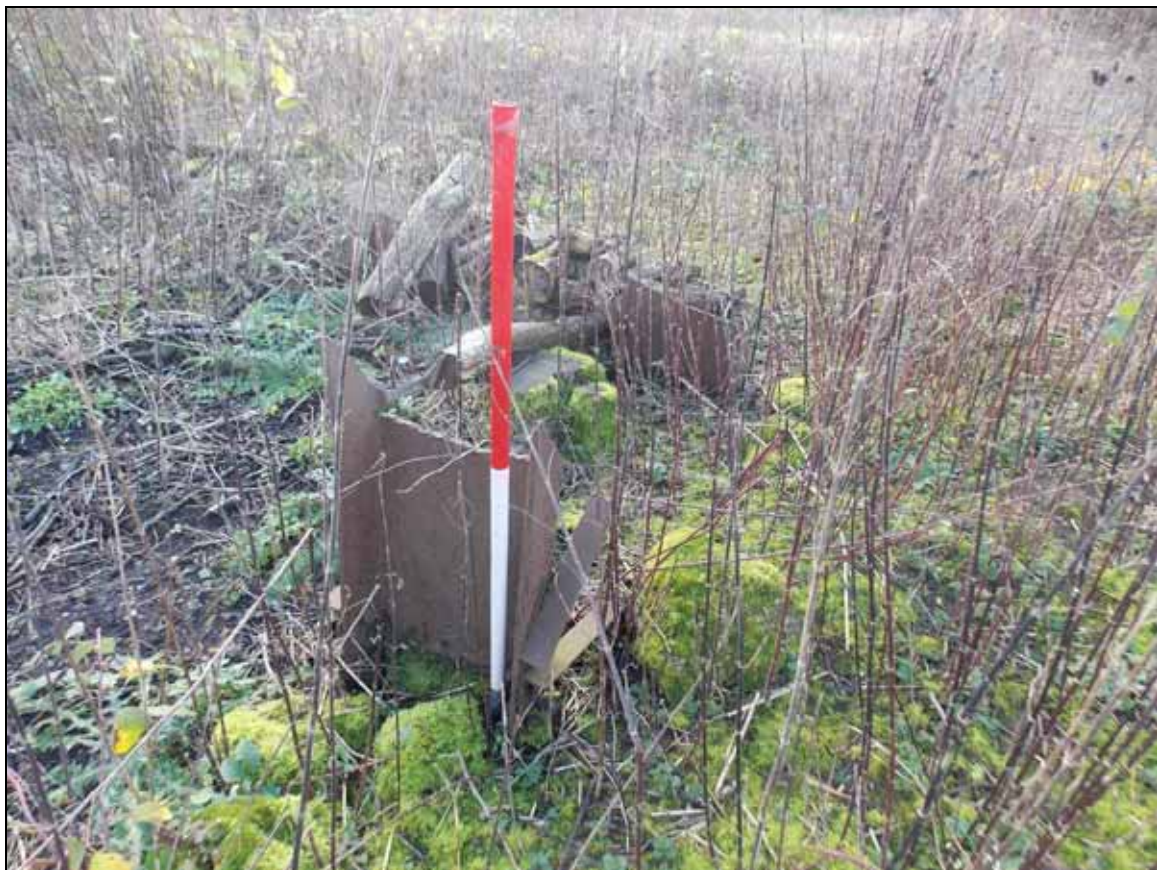
Figure 42: Base of steel SW stanchions of Structure O, looking south-west (scale 1m).
