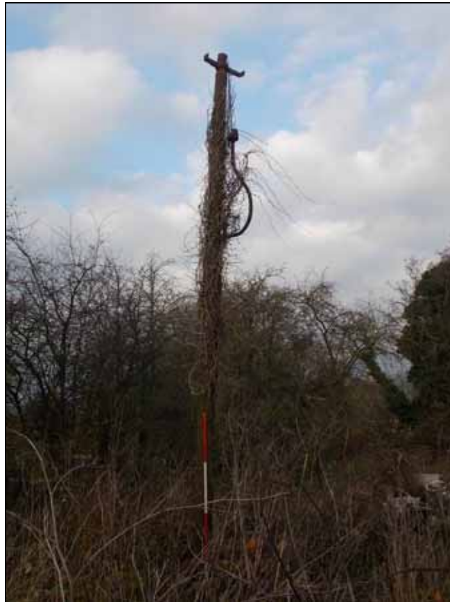
Figure 32: Structure J, looking south-west (scale 2m).
