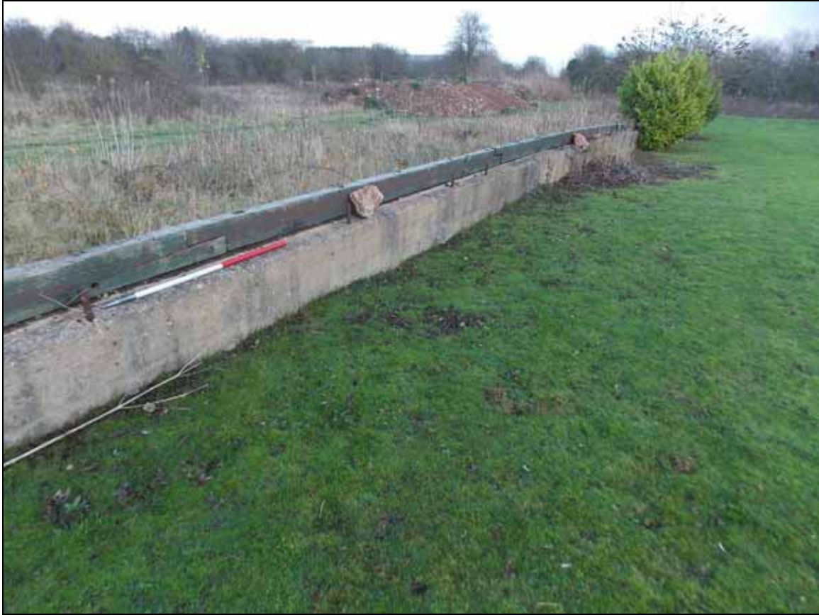
Figure 20: Eastern section of the northern plinth with timber sill, looking north-east (scale 1m).
