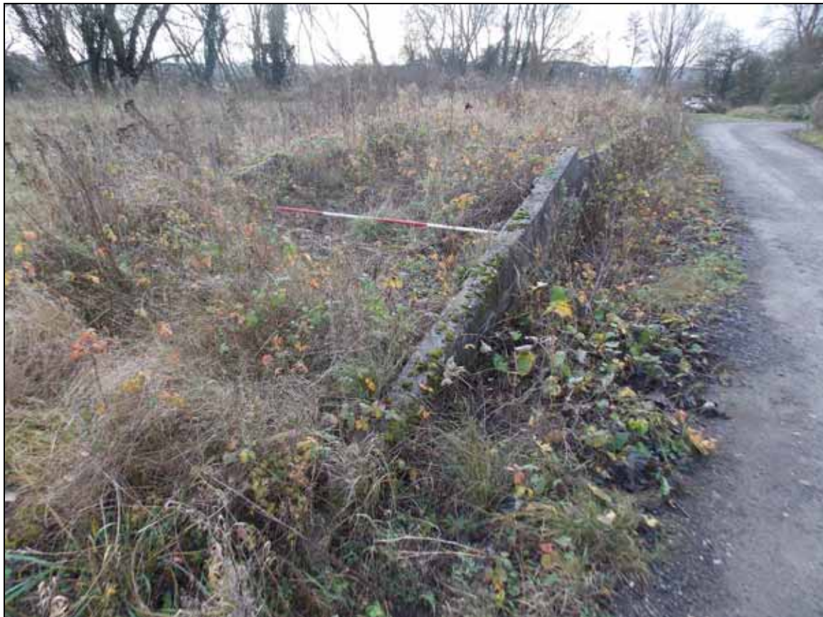
Figure 28: North-eastern end of the former platform Structure I, looking south-west (scale 2m).
