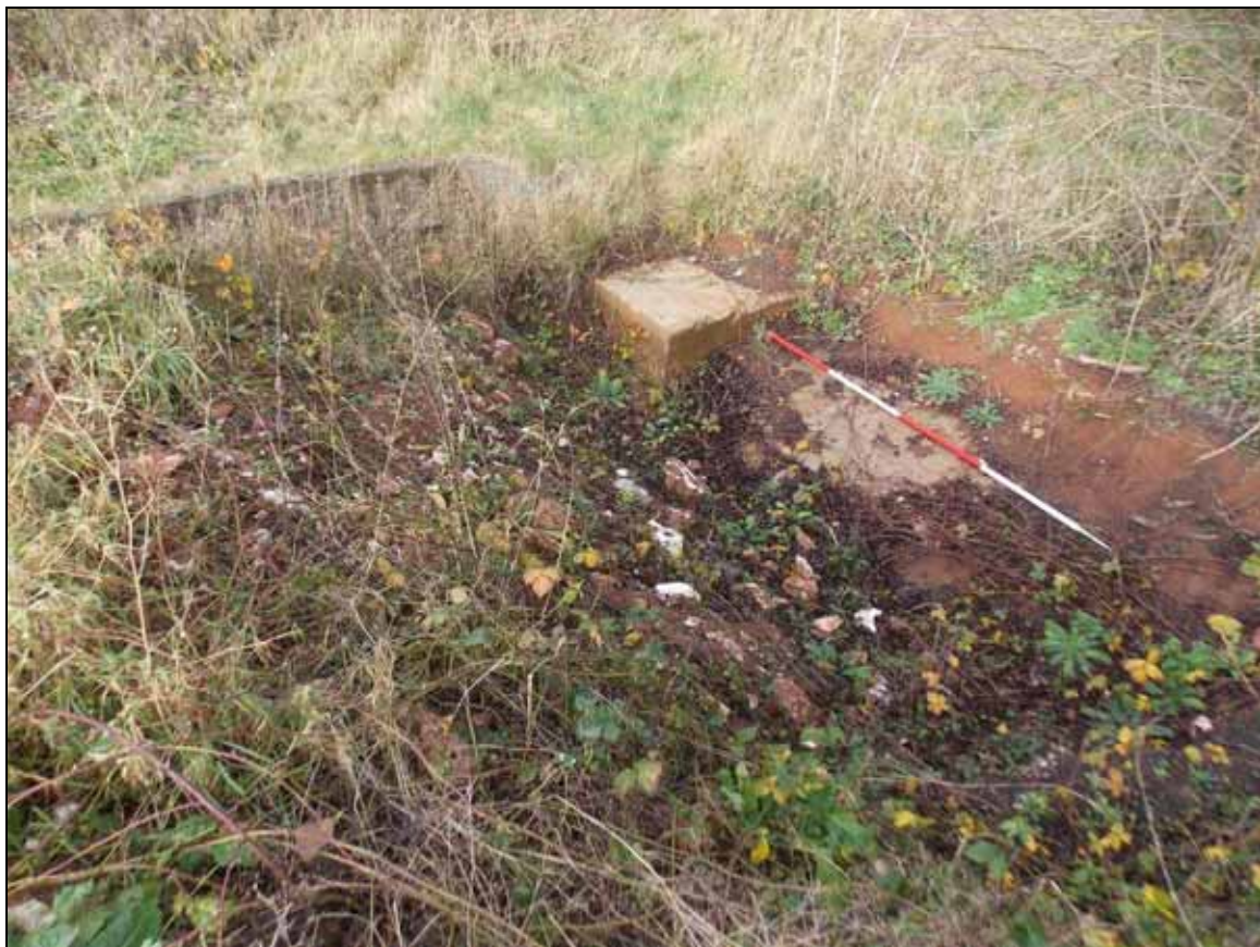
Figure 10: Concrete roof of Structure B, looking north-west (scale 2m).
