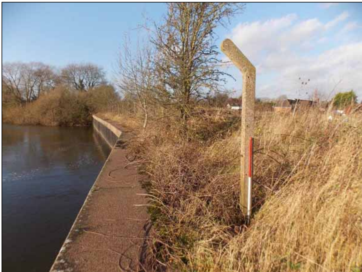
Figure 39: Detail of concrete fence post, looking west (scale 1m).
