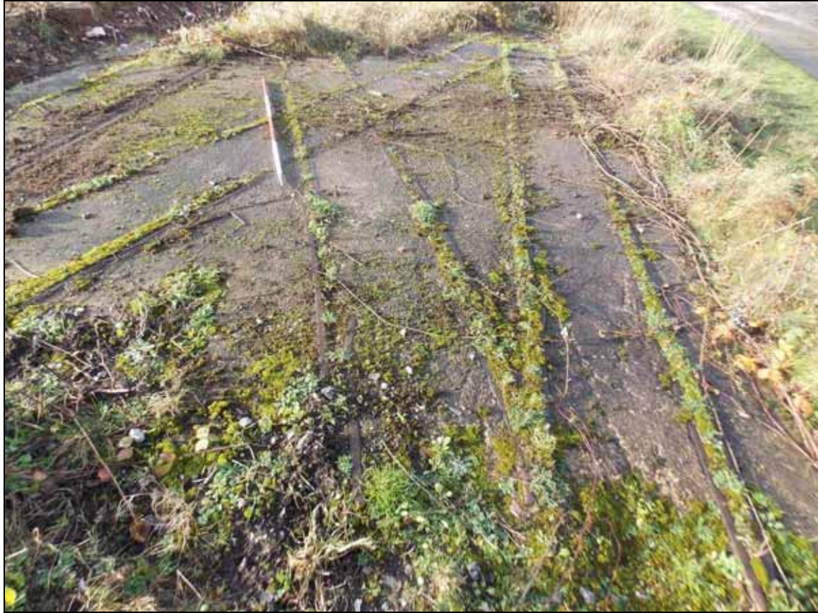
Figure 15: Structure D with railway lines set within a concrete base, looking east (scale 2m).
