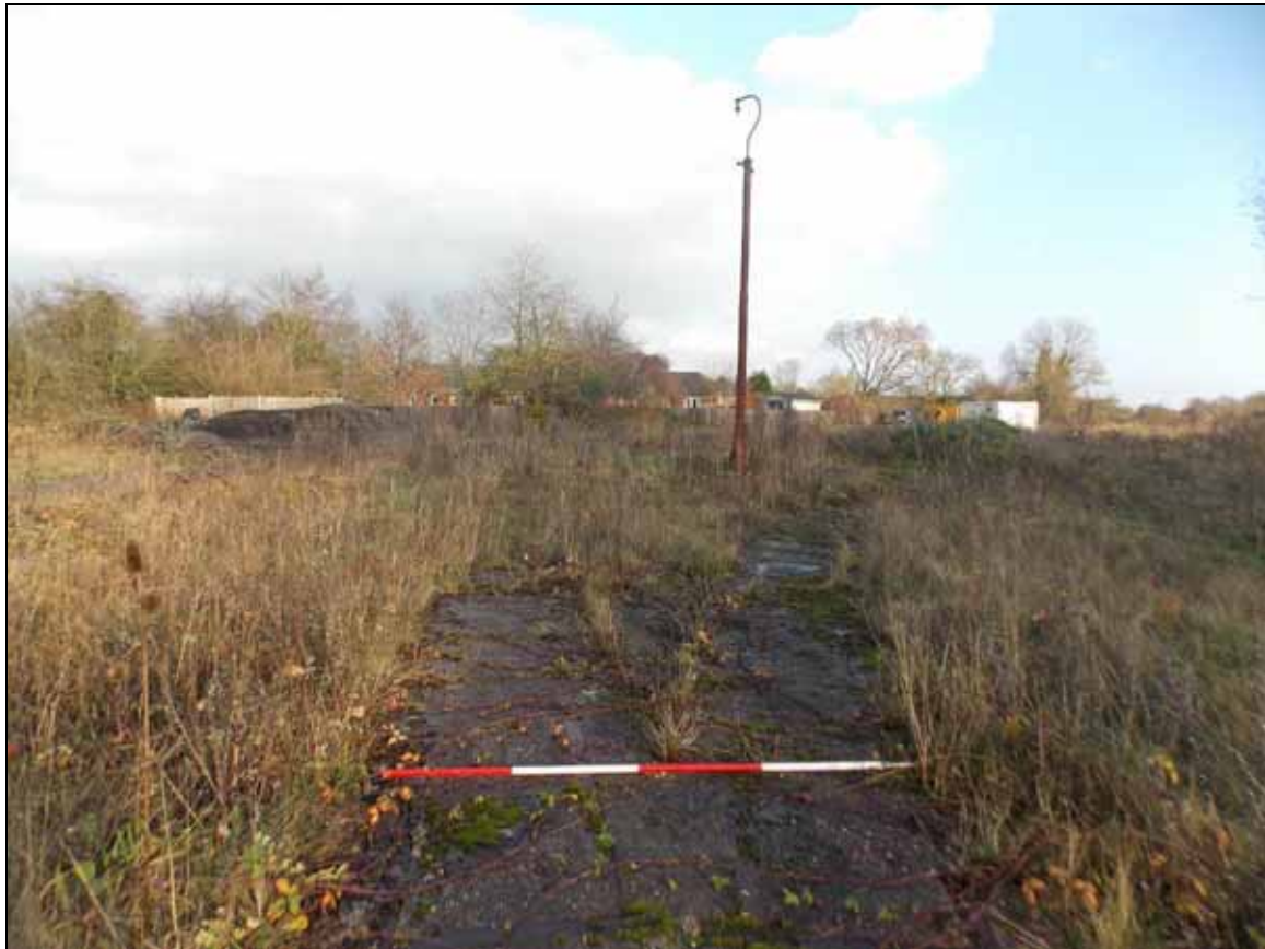
Figure 26: Structure H and adjacent lamp post Structure G, looking north-east (scale 2m).
