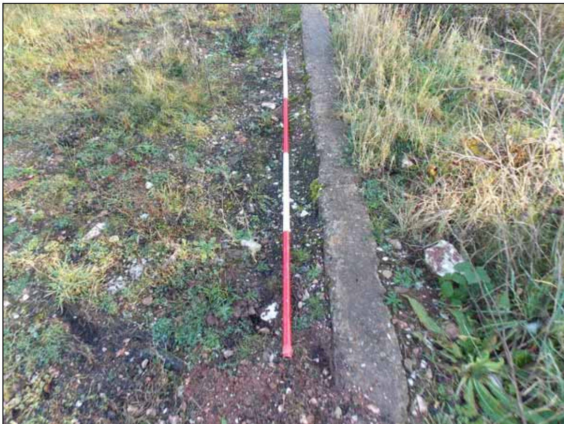
Figure 24: Detail of the concrete wall, looking east (scale 2m).
