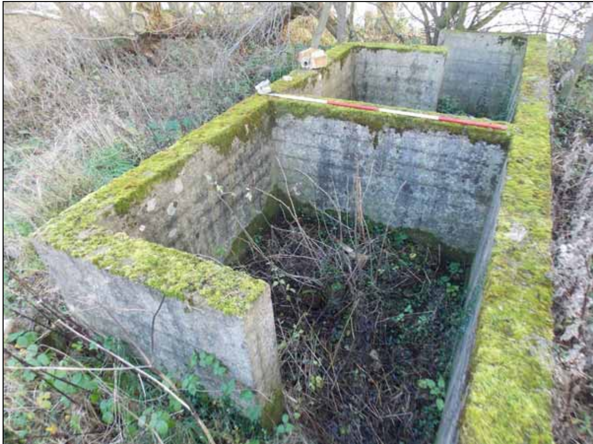
Figure 35: General view of Structure L, looking south-east (scale 2m).
