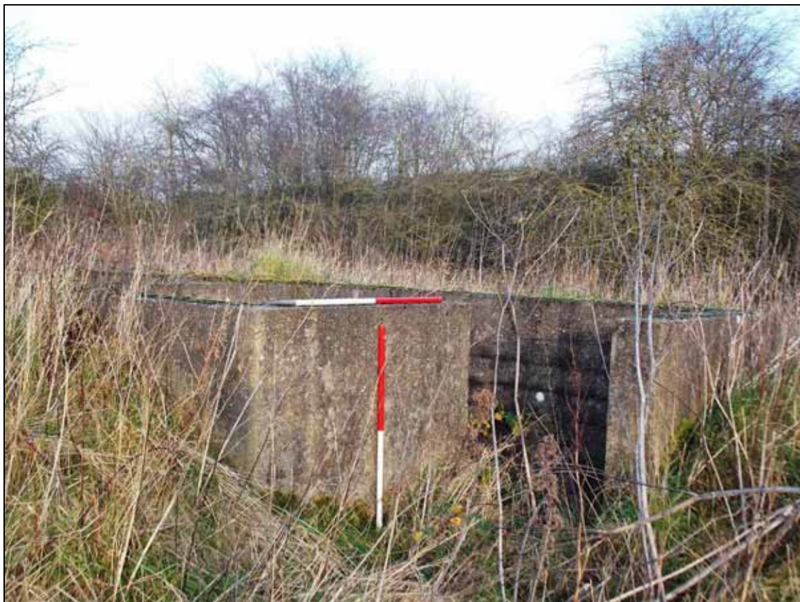
Figure 46: Southern blast entrance of Structure Q, looking north-east (scale 2 x 1m).
