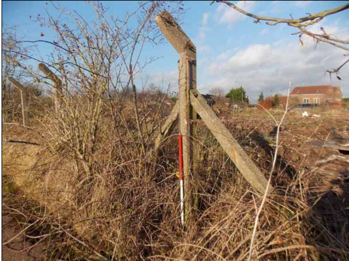
Figure 40: Fence post with angled struts and traces of the wire mesh, looking north-west (scale 1m).
