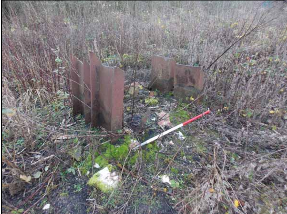
Figure 43: Base of NE stanchions of Structure O, Looking north-east (scale 1m).
