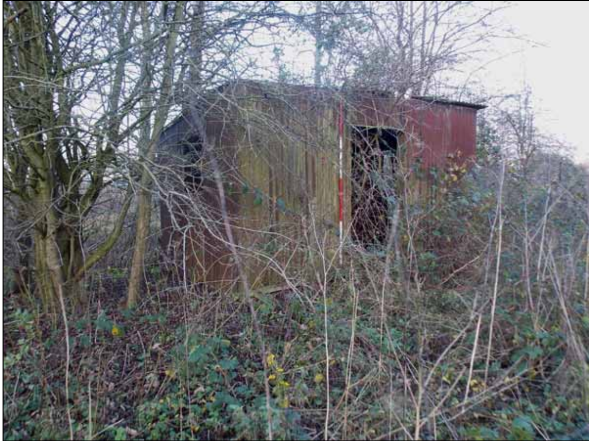
Figure 47: Structure R, looking north-east (scale 2m).
