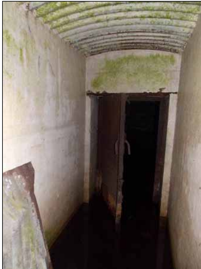
Figure 12: Blast door of Structure C, looking east.
