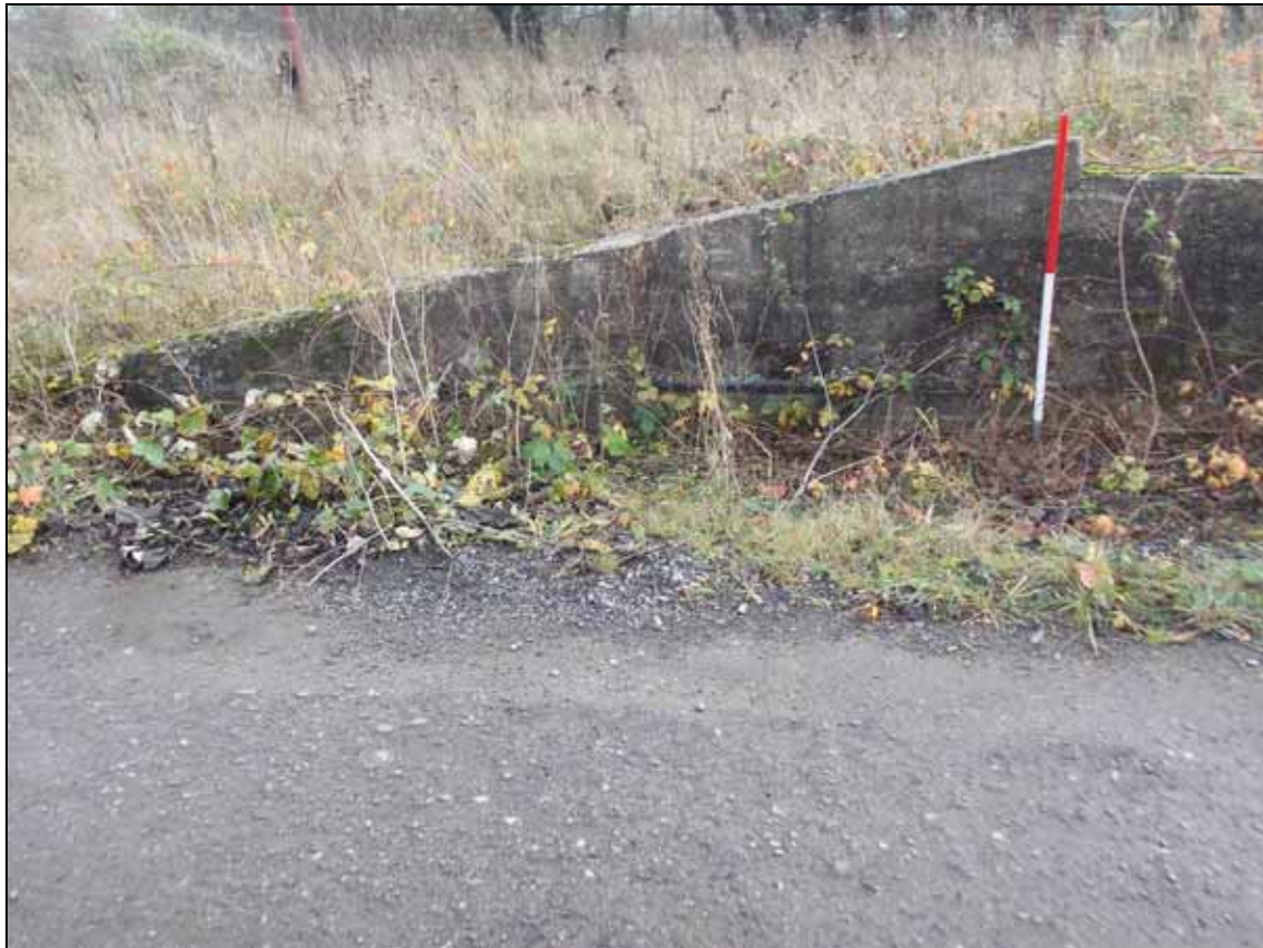
Figure 29: Detail of the sloped north-eastern end, looking south-east (scale 1m).
