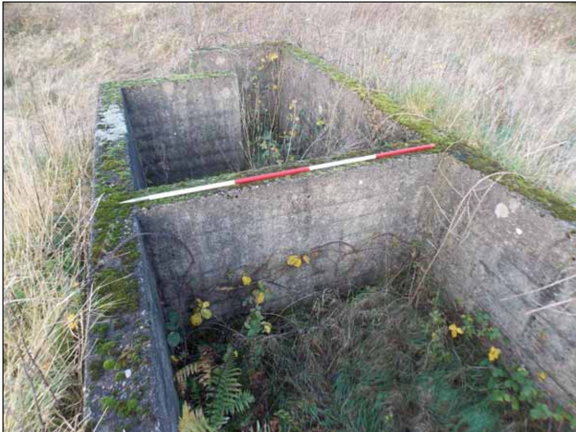
Figure 45: General view of Structure Q, looking north (scale 2m).
