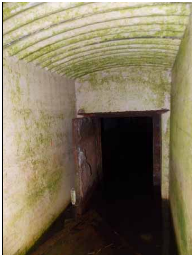
Figure 8: Blast door of Structure B, looking east.
