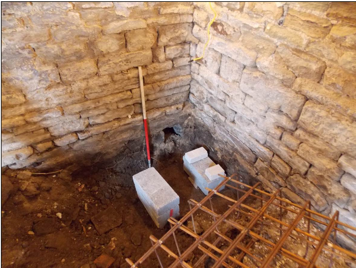
Figure 24: Underpinning trench within the north-eastern corner of the barn (scale 1m).
