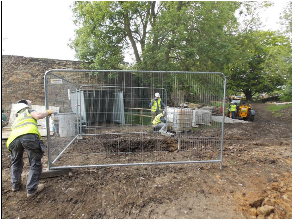
Figure 16: Location of soak-away test pit, looking south-west.
