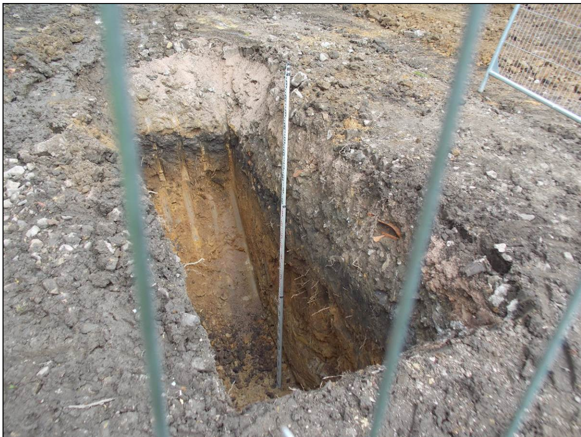
Figure 17: Soak-away test pit, looking north-west (scale 3m).
