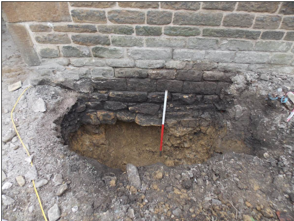
Figure 28: Underpinning trench against the external north wall (scale 1m).
