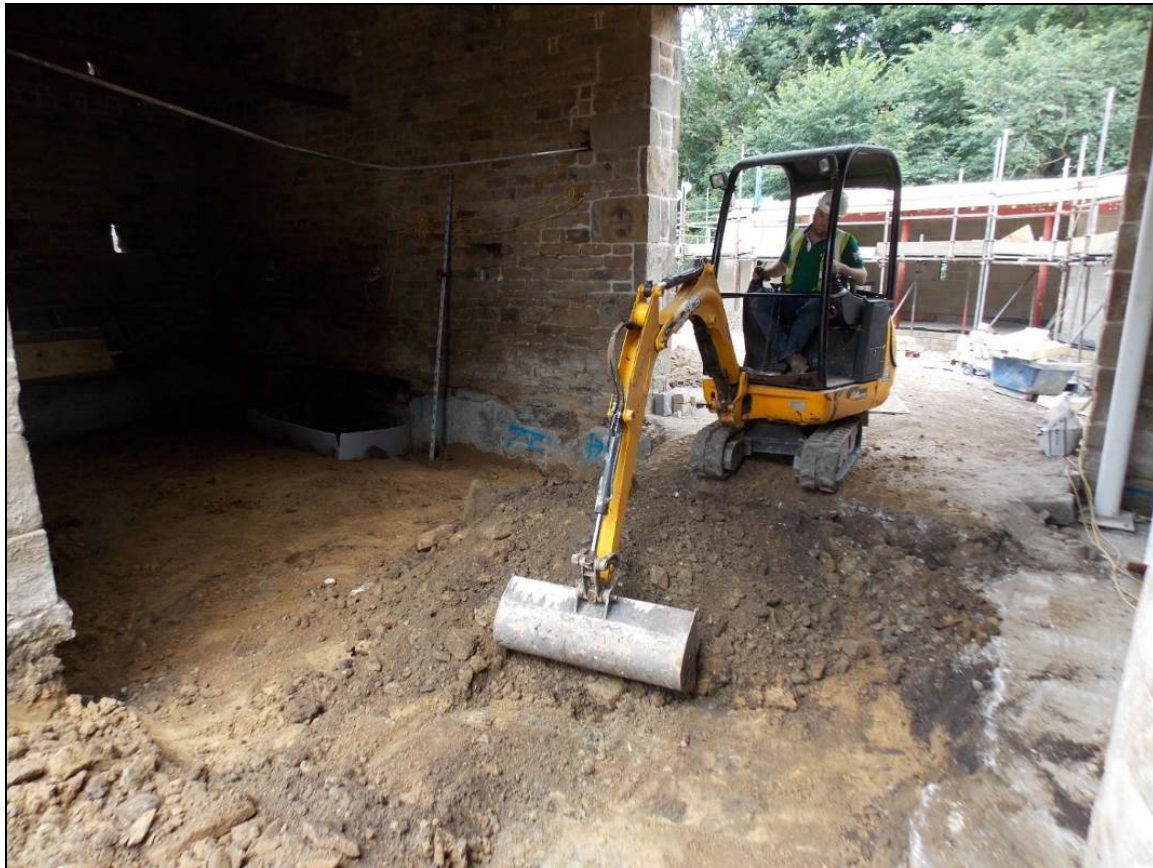
Figure 35: Excavation down to the natural clay, looking north.
