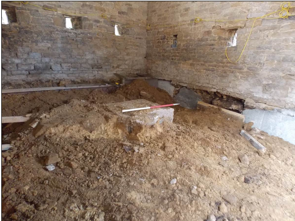
Figure 37: Excavated western area with a concrete back-filled test pit, looking north-west (scale 1m).
