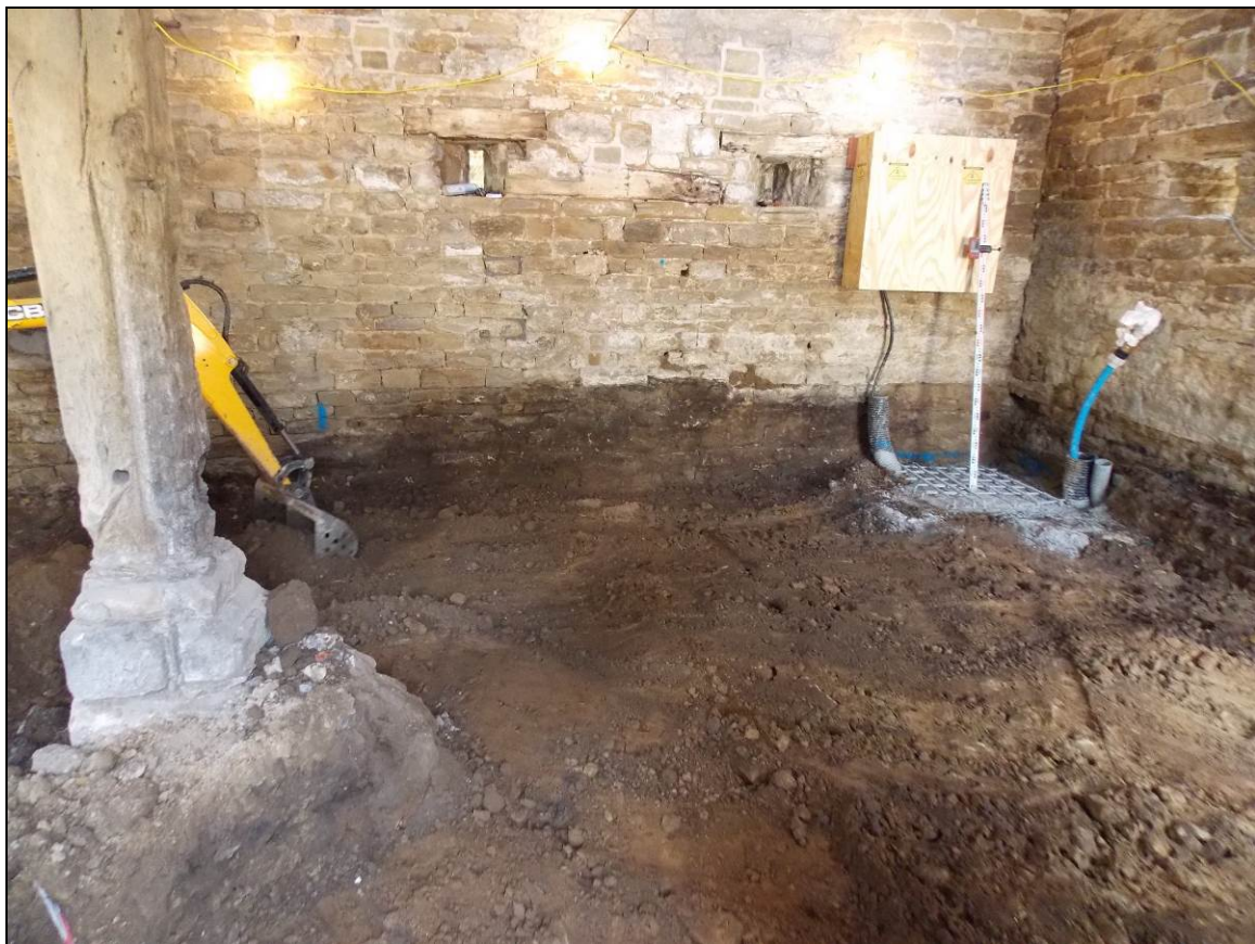
Figure 32: Excavation within the eastern area of the Old Barn, looking north-east.
