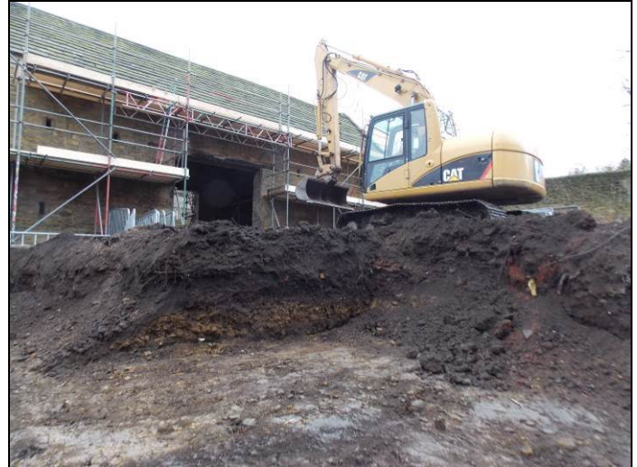
Groundworks to the rear of the Old Barn, Dronfield
