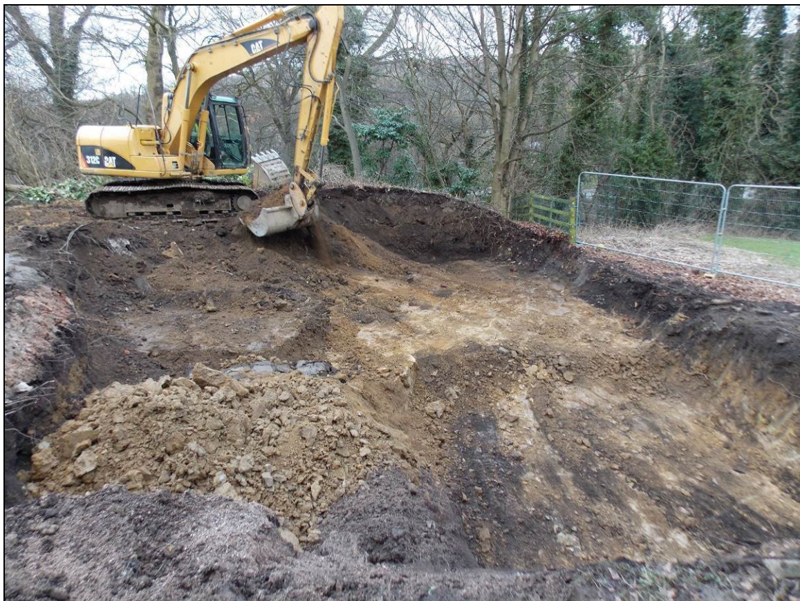
Figure 6: Northern area under excavation, looking north.
