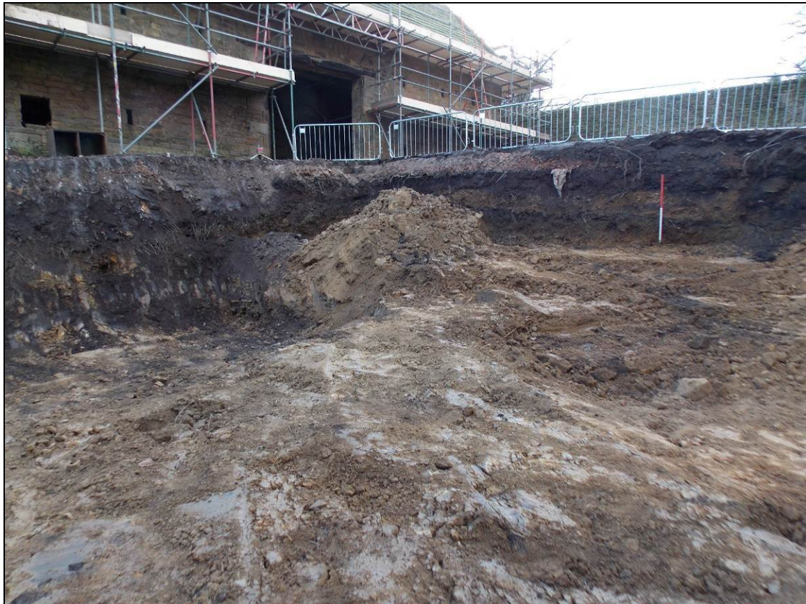
Figure 5: East facing section through the excavation, looking south-west (scale 1m).
