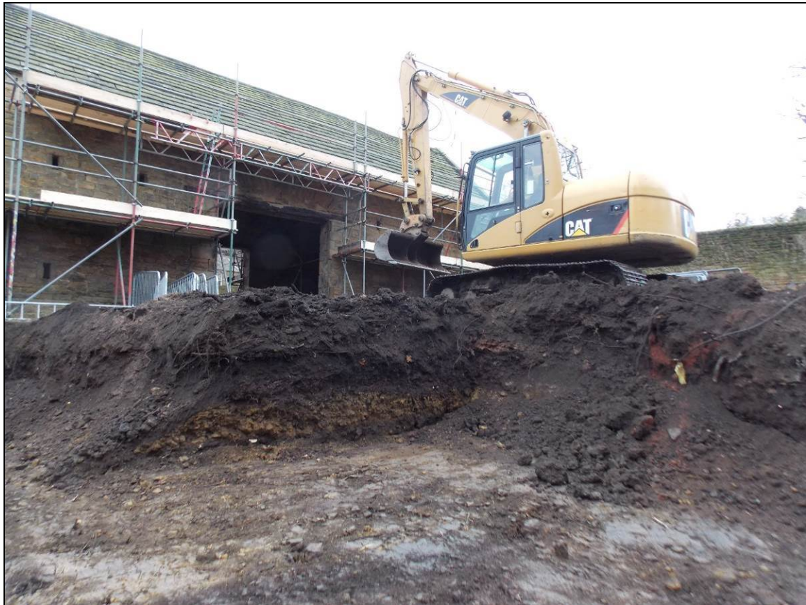
Figure 3: Excavation to the rear of the Old Barn, looking south-west.
