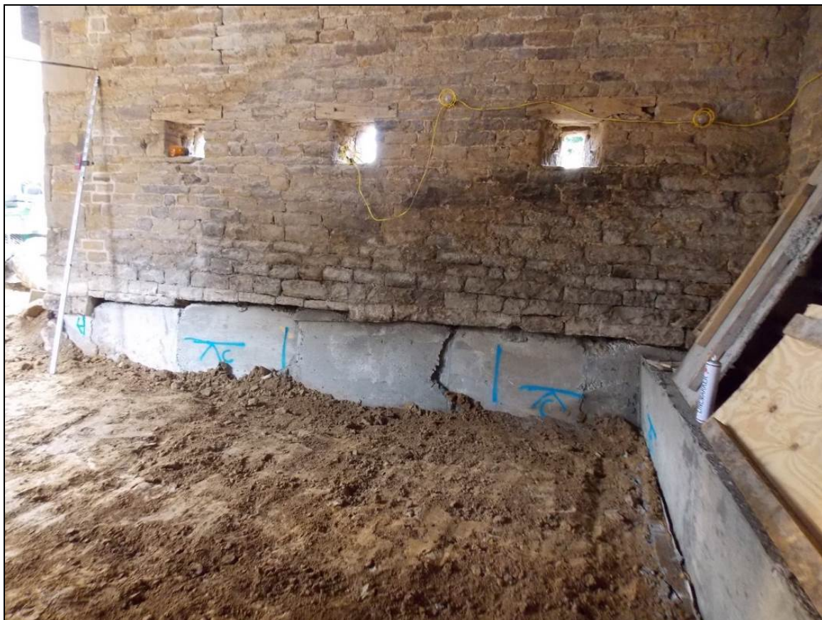
Figure 38: Full excavation within the western area, looking south.
