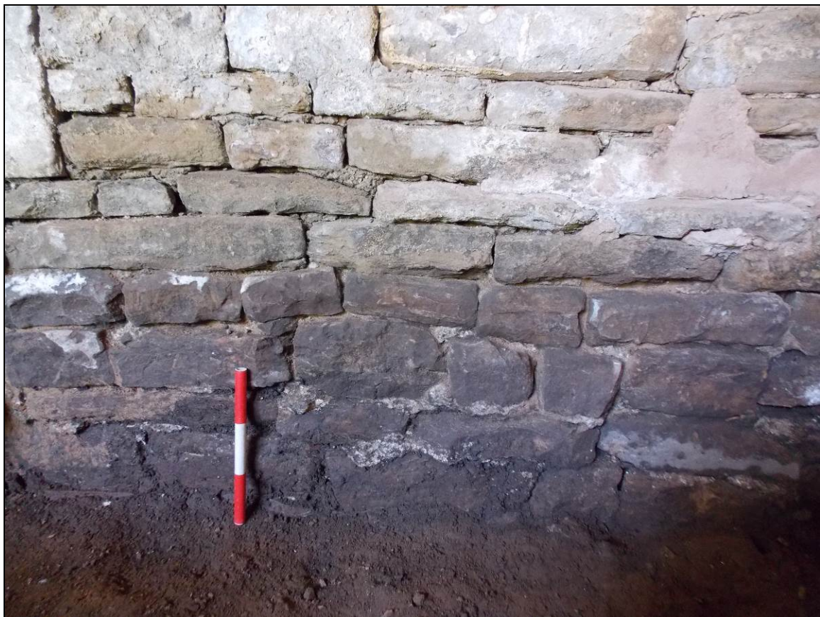
Figure 20: Detailed view of northern wall (221) following the removal of the later abutment (scale 300mm).
