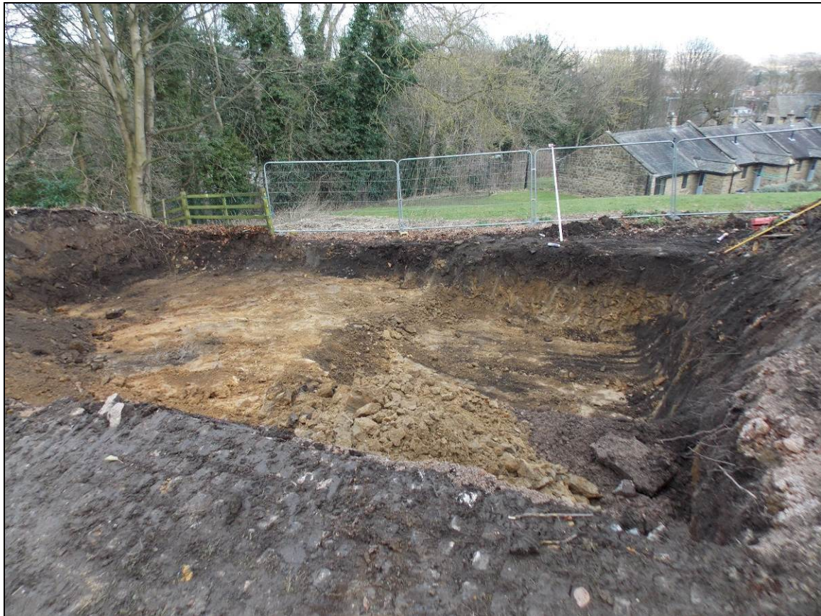
Figure 9: Excavation area, looking north-east.
