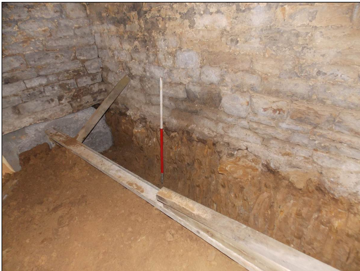
Figure 26: Underpinning trench along the west wall, looking south-west (scale 1m).
