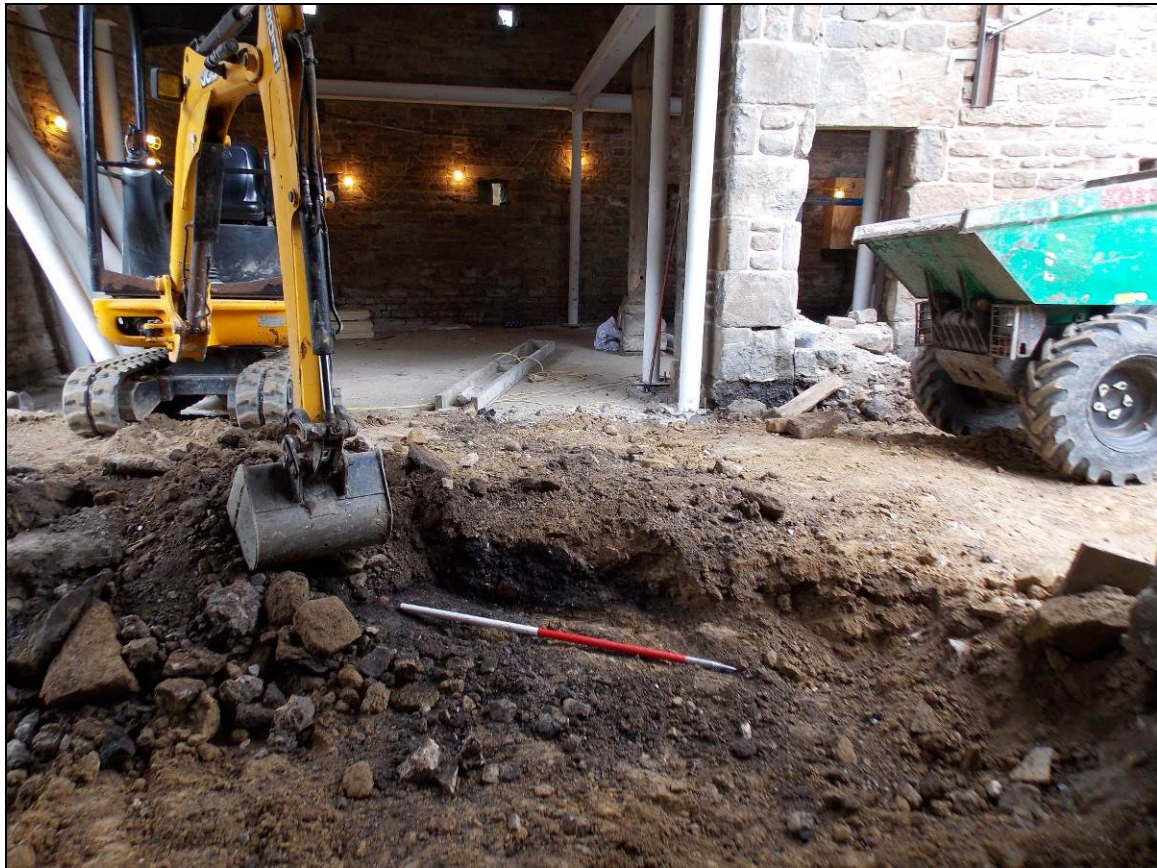
Figure 33: Excavation of the central paving area, looking east (scale 1m).
