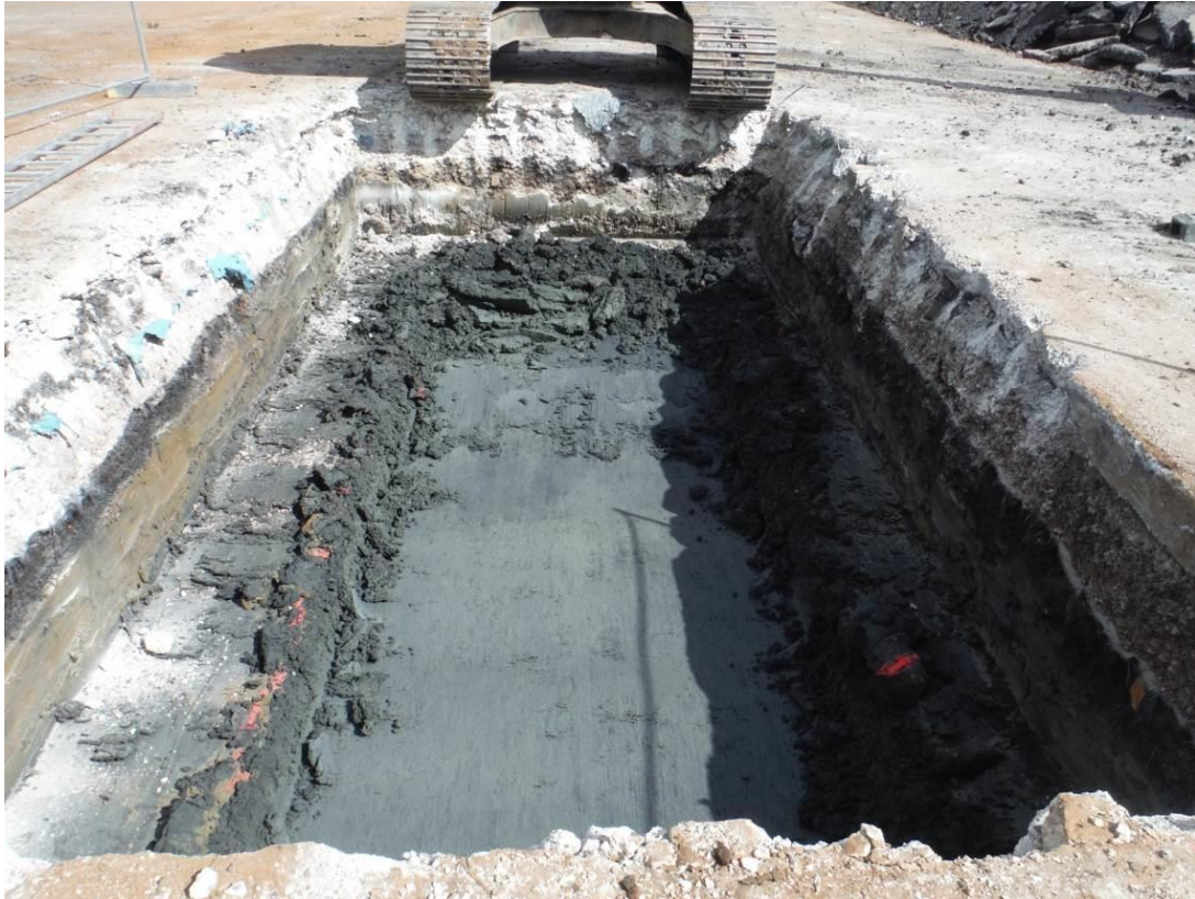
Figure 7. Trench 1 looking east, showing clean and uniform surface of upper alluvial clay.
