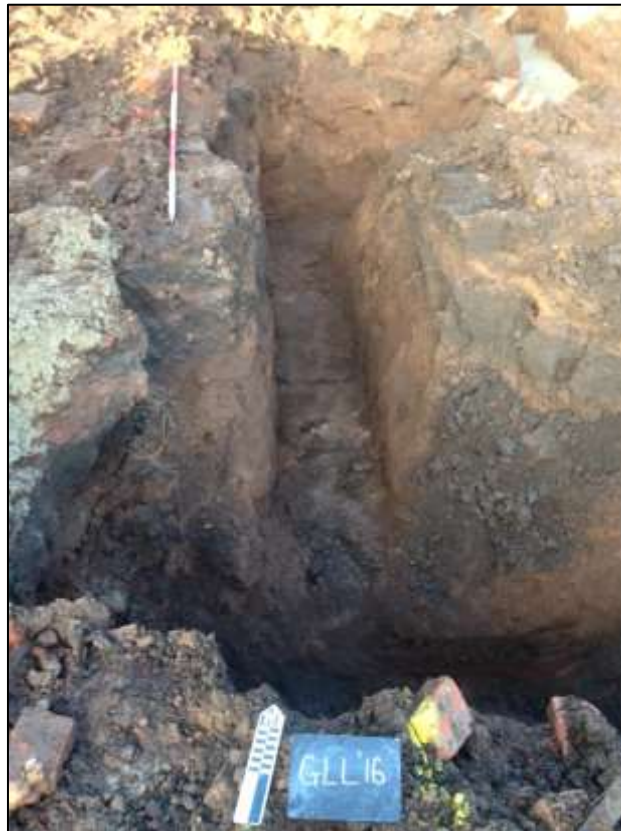
Figure 5. View north of the foundation trenching (scales = 0.5m graduations).
