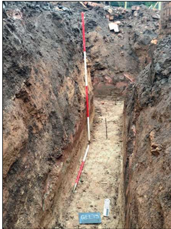
Figure 3. View north of foundation trench (scales = 0.5m graduations).
