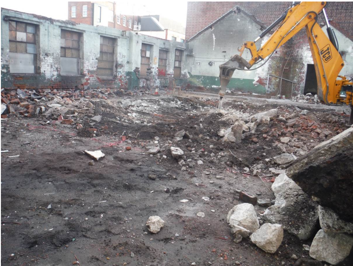
Figure 2. Initial stripping of the evaluation trench, looking south-east.
