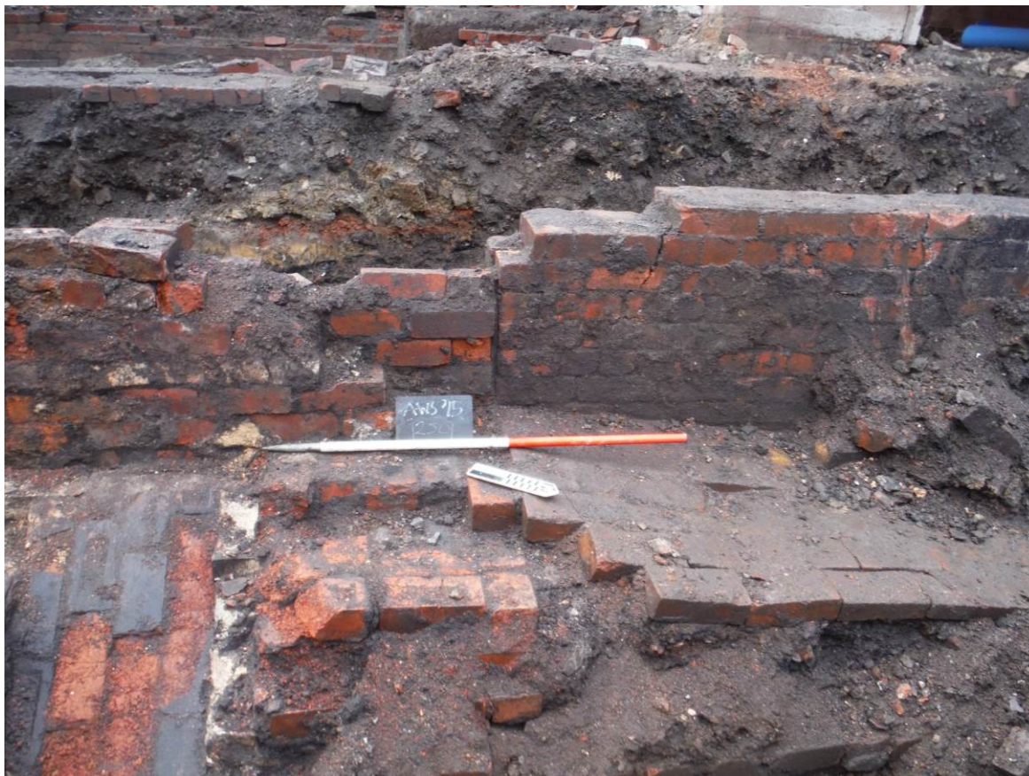
Figure 11. Floor surface (250) (right hand side) rising up over the south-west side of the boiler house (scale = 1m).
