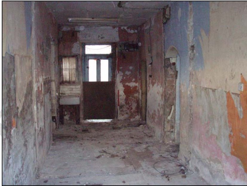
Fig. 57. Ground floor hall of Unit one (facing south-west) (scale = 2m).
