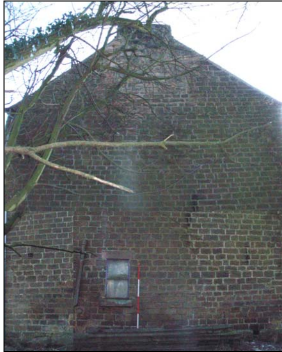
Fig. 33. Photograph of the north-west façade of the house (facing south-east).
