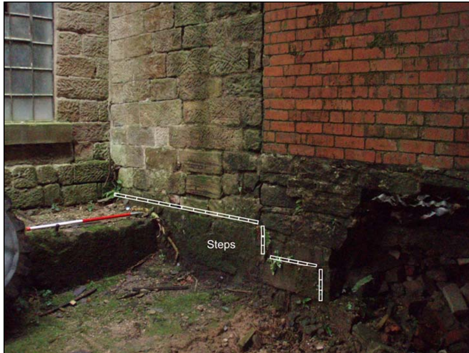
Fig. 16. Photograph of the original steps which led up to the arched entranceway in phase one (facing north-east) (scale = 1m).
