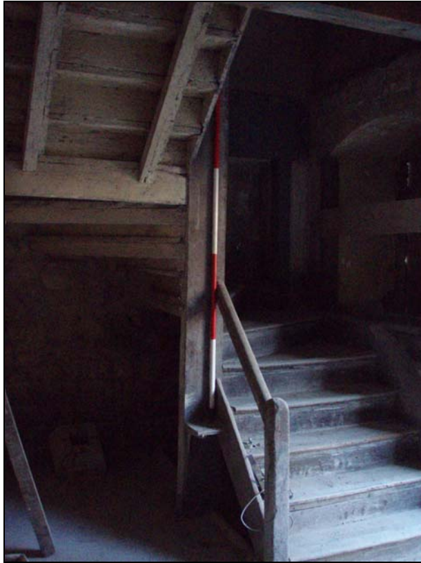
Fig. 46. Photograph of the staircase in the mill (facing north) (scale = 2m).
