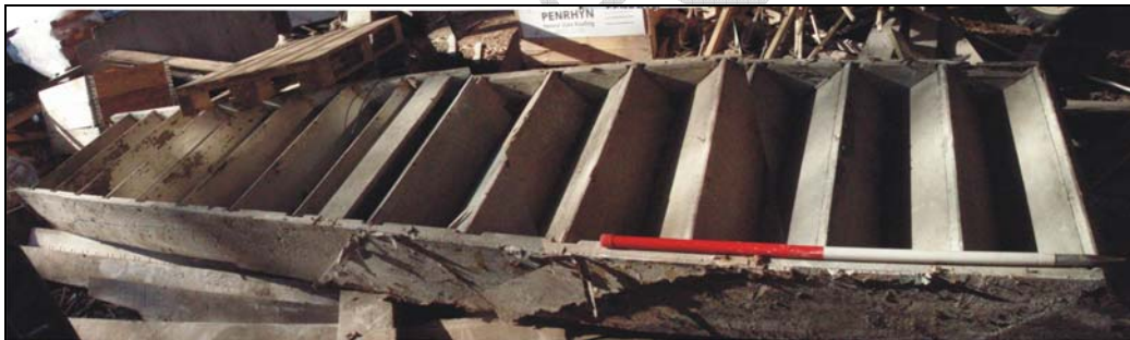
Fig. 51. Photograph of original staircase from the second floor of the mill (facing south-west) (scale = 1m).
