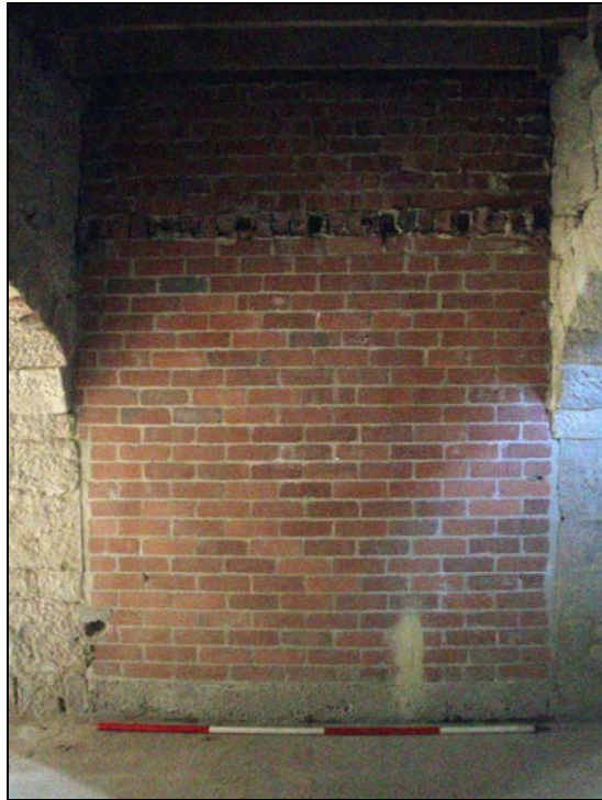
Fig. 45. Photograph of the brick wall which blocks the original entrance to the mill (facing south-west) (scale = 2m).
