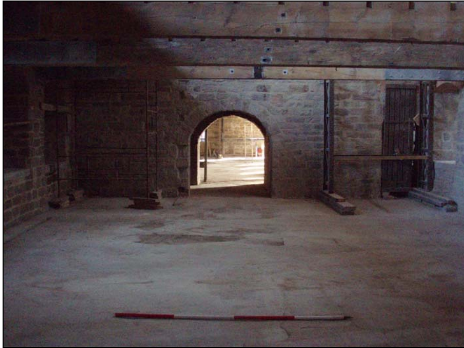
Fig. 36. Photograph of the partition wall and arches on the ground floor of the mill (facing south-east) (scale = 2m).
