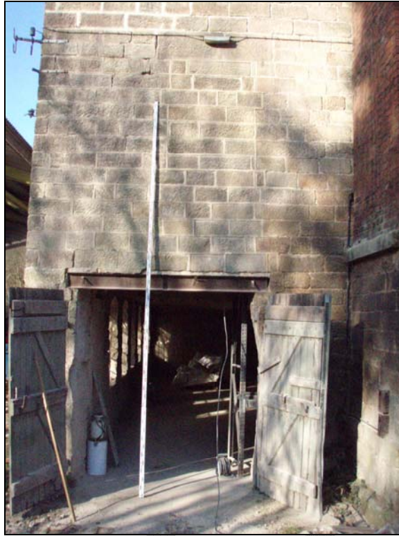
Fig. 7. Photograph of infilled window and doorway of later construction than the mill in the south-east façade of the mill (facing north-west) (scale = 5m)
