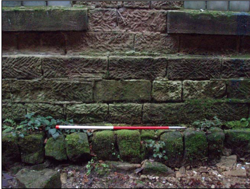
Fig. 5. Photograph of the rougher courses of stone forming the foundations (facing north-east) (scale = 1m).
