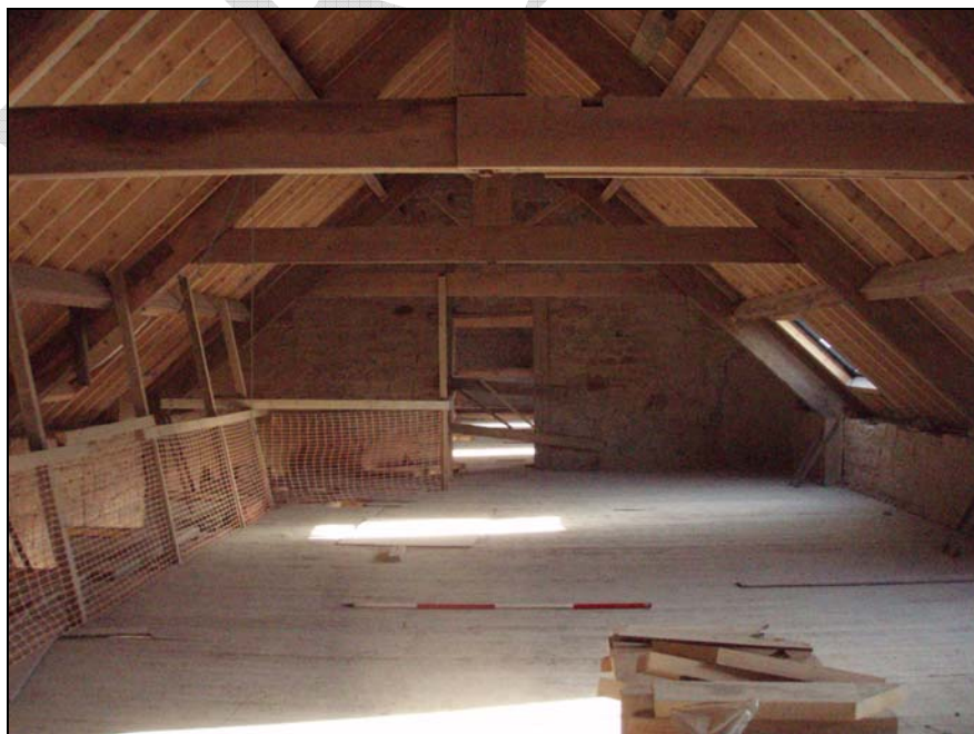
Fig. 54. Photograph of the attic of the mill (facing south-east) (scale = 2m).
