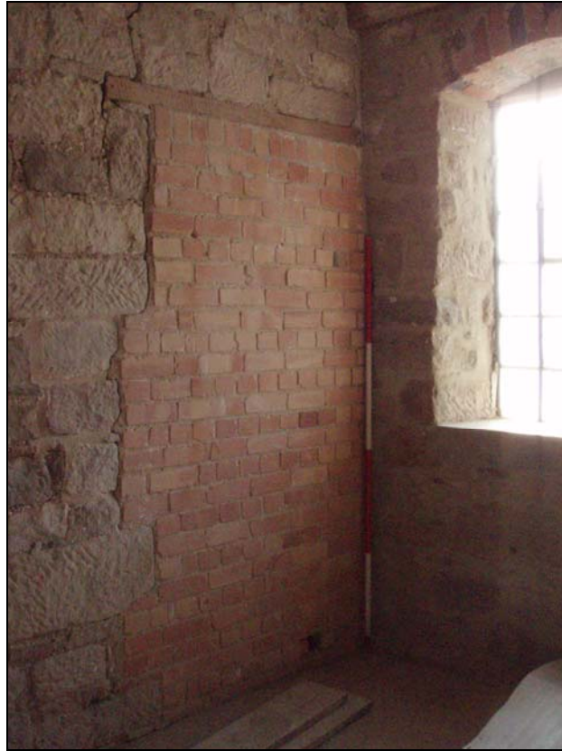
Fig. 49. Photograph of infilled door on second floor of mill (facing south).
