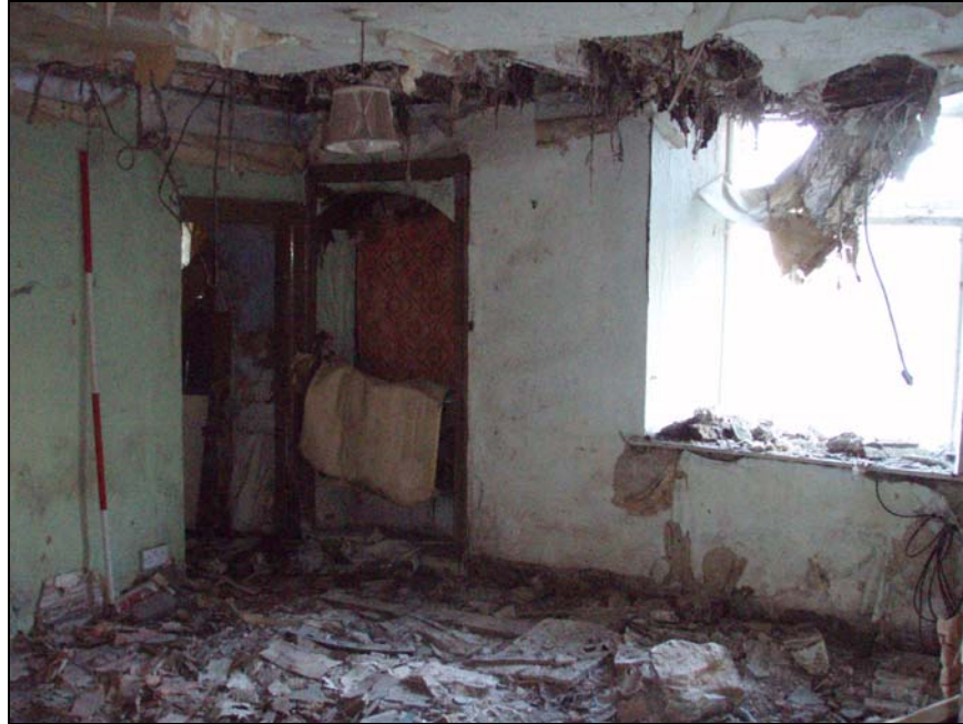
Fig. 60. Photograph of the front room of unit two showing the infilled back door (facing north) (scale = 2m).
