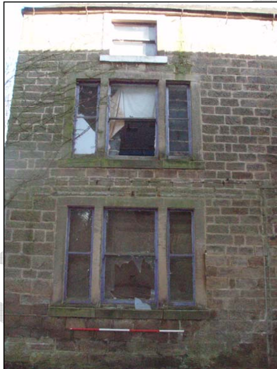
Fig. 25. Photograph of a standard window (ground and first floor) and small window (second floor) of the south-west façade of the house (facing north-east)
