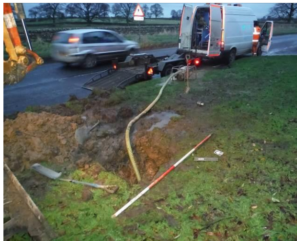
View looking north-east towards Trench 1 and the B6318 trunk road
