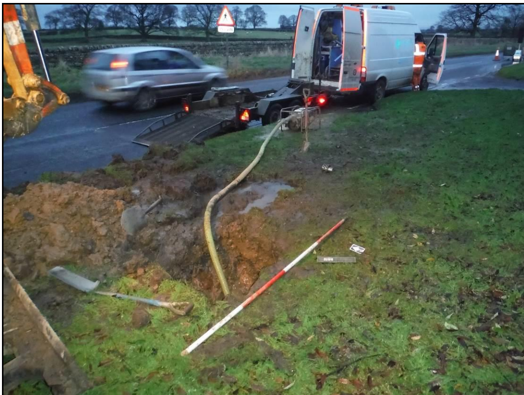
Figure 5. View of Trench 1 looking north-east towards the B6318 (scale = 0.5m graduations).
