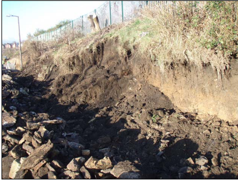
Fig. 5 View of the wall after demolition, looking north-west.
