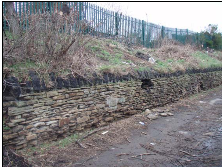
Fig. 3 View of the sandstone revetment wall looking west.
