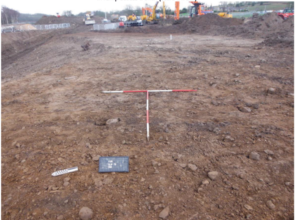
Figure 7. View looking east of 10m strip (scale= 2 x 1m).
