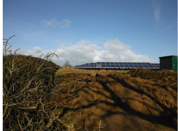
View of the Solar farm from the southern edge of the site
