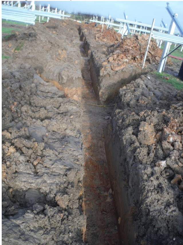
Figure 6 Course of the Primary Cable Trench looking north
