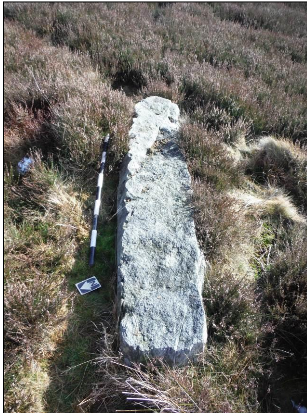
Figure 16. Possible collapsed boundary marker stone or gate post F009, looking south-east. Scale = 1m.
