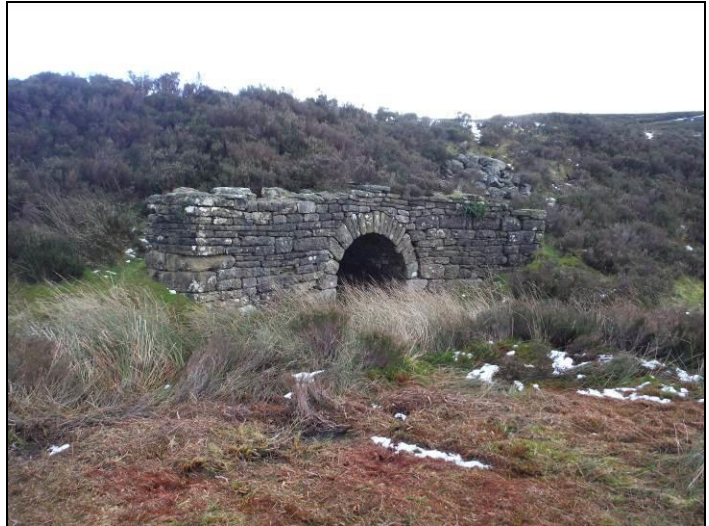
HER 7530, Bridge over Blaeberry Cleugh
