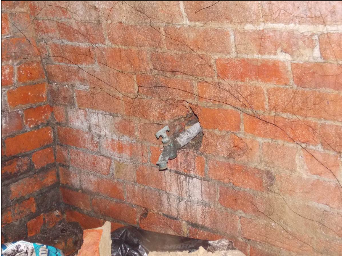
Figure 16: Detailed view of the tap, looking south.
