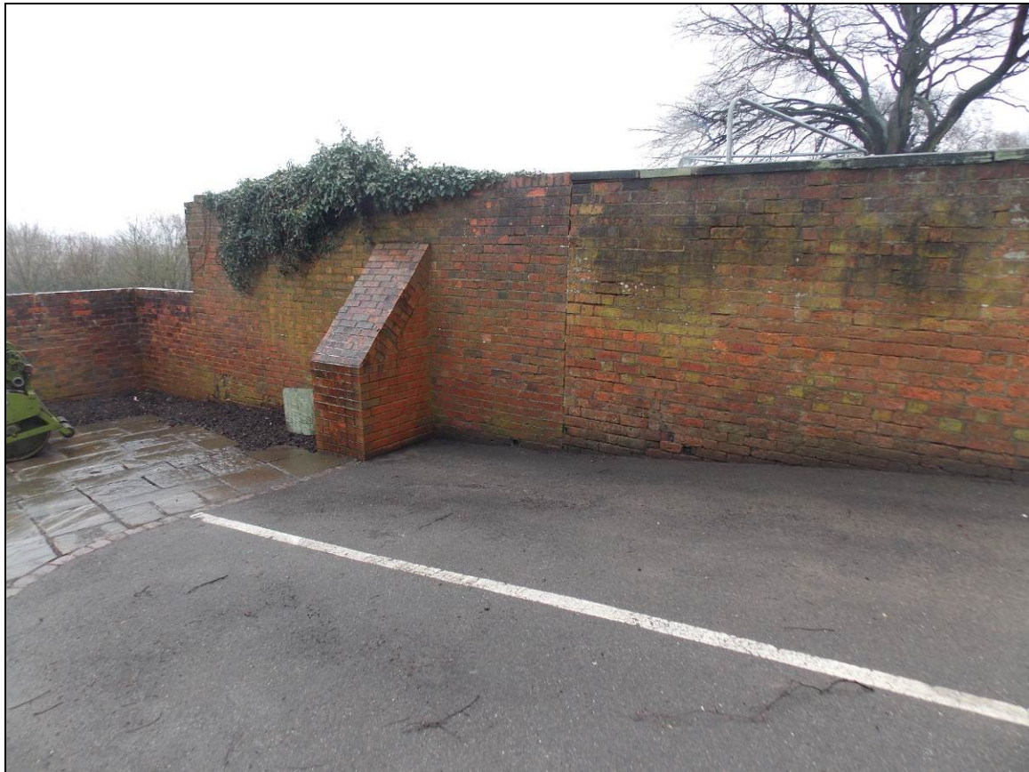
Figure 10: North-western retaining wall of the Appel Store with buttress.
