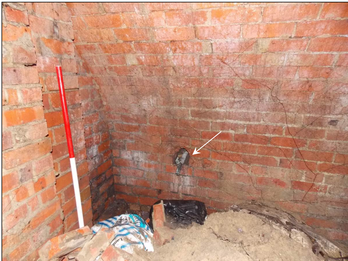
Figure 15: Water tap (arrow) within the south-western longitudinal wall (scale 1m).
