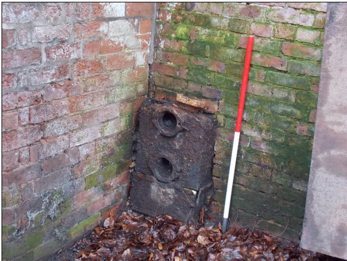
Figure 13: Detail of former pipe housing, looking north-east (scale 1m).
