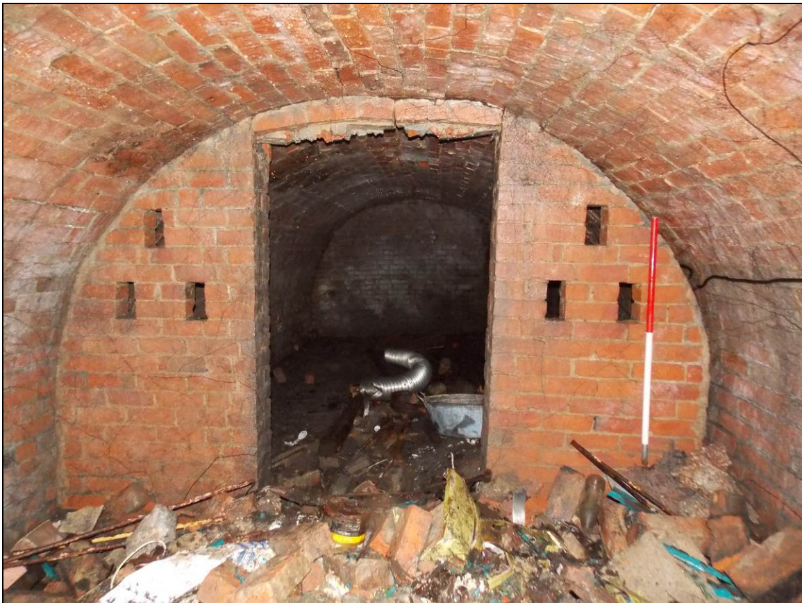
Figure 17: Partition wall with doorway opening across the south-eastern chamber (scale 1m).
