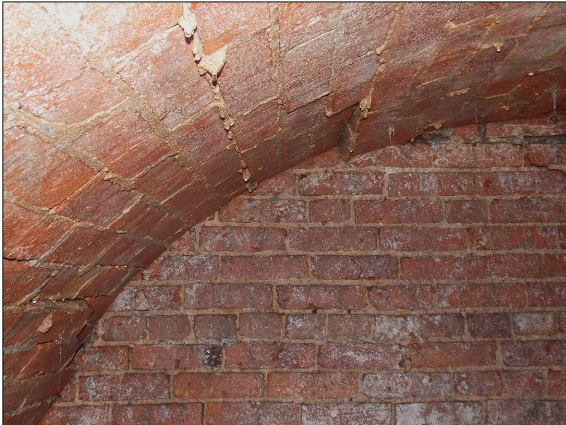
Figure 20: Primary brickwork of the cross wall and later arched brick vault.
