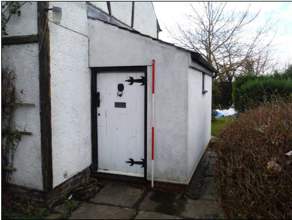
Figure 16. North-east elevation of the northern pitched roof extension (scale = 1 x 2m).
