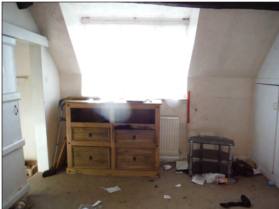
Figure 56. South-west wall of Room F5 (scale = 1 x 1m).
