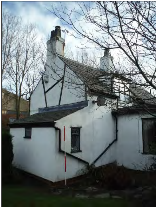
Figure 20. North-west and south-west elevations on the north-westward extension (scale = 1 x 2m).
