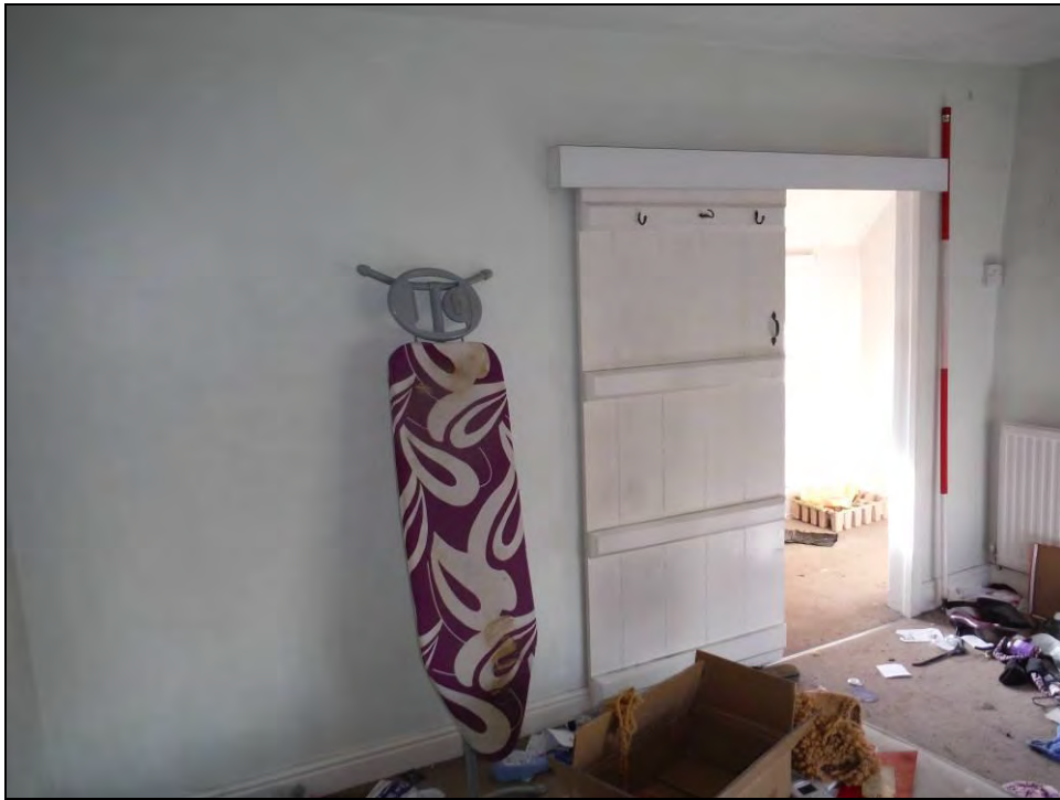
Figure 51. South-west wall of Room F4 (scale = 1 x 2m).
