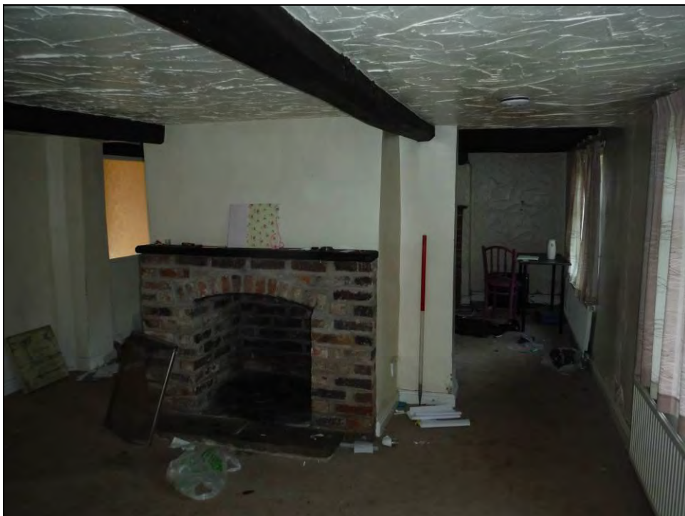
Figure 28. View facing north-west of Room G4 (scale = 1 x 1m)
