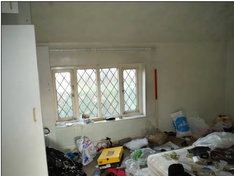
Figure 52. North-east wall of Room F4 (scale = 1 x 1m).
