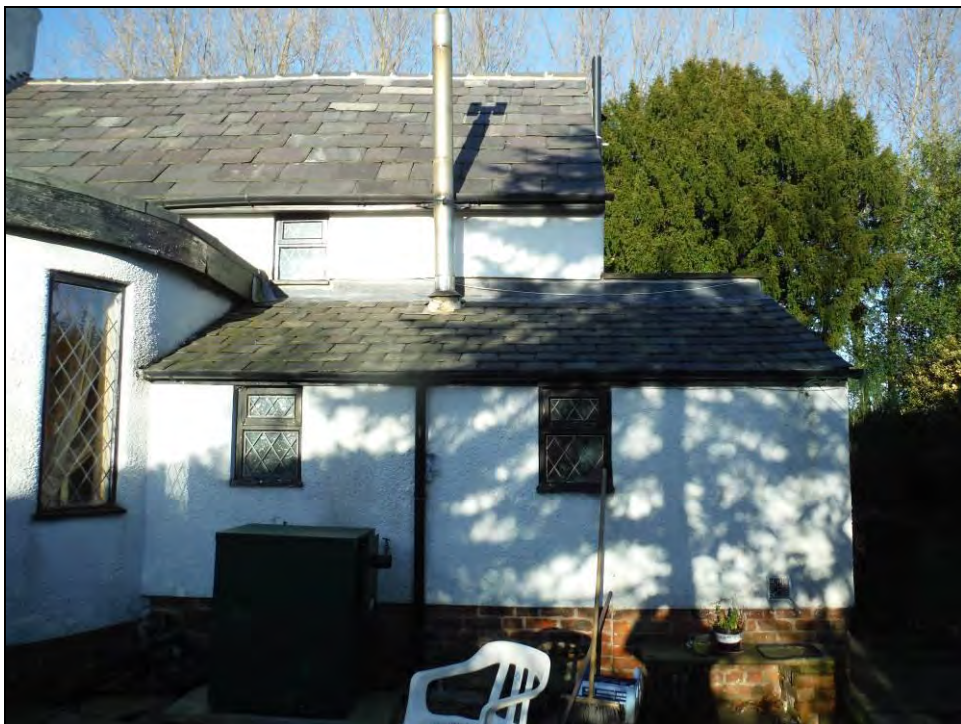
Figure 19. South-east end of the south-west elevation.
