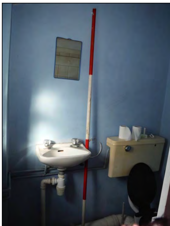
Figure 24. View facing east of Room G2 (scale = 1 x 2m).
