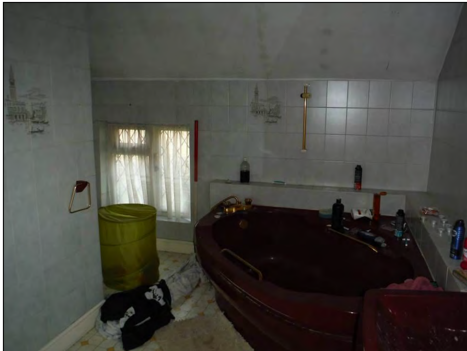
Figure 46. North-east wall of Room F2 (scale = 1 x 1m).
