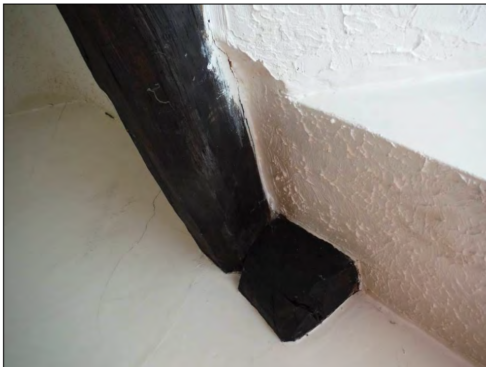
Figure 58. Detail of through-purlin and cleat in the south-east wall of Room F5.
