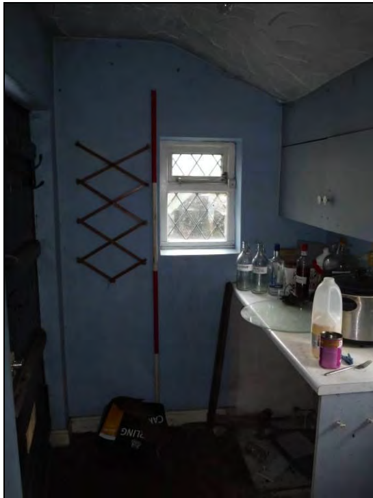
Figure 22. View looking south-east in Room G1. (scale = 1 x 2m).
