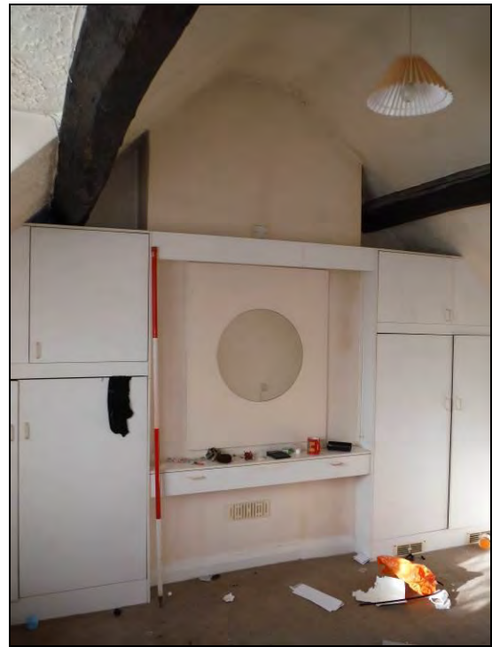
Figure 55. North-west wall of Room F5 (scale = 1 x 2m).
