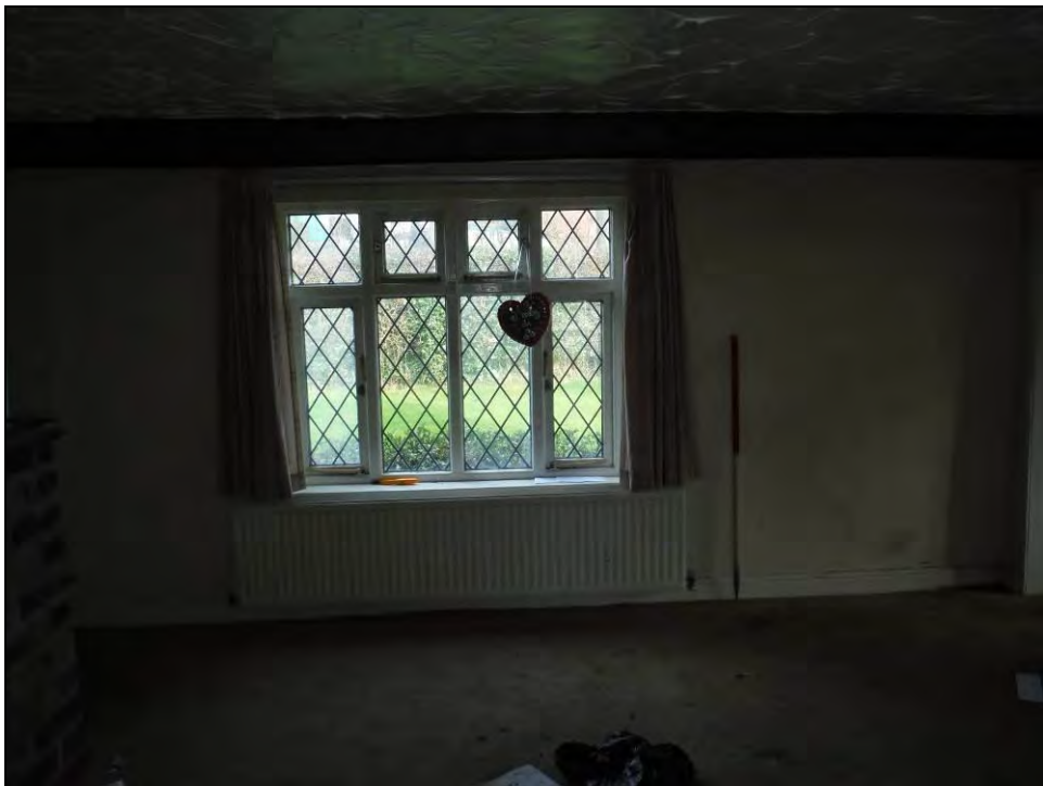
Figure 30. North-east wall of Room G4 with eight-light window (scale = 1 x 1m).
