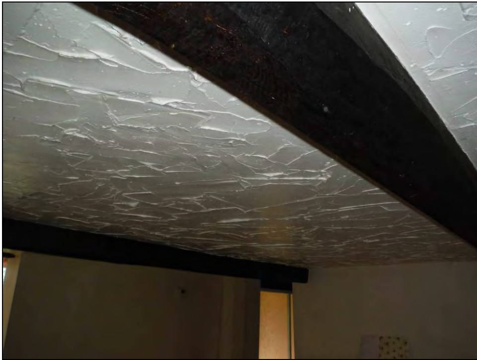
Figure 33. Detail of binder beams in Room G4.
