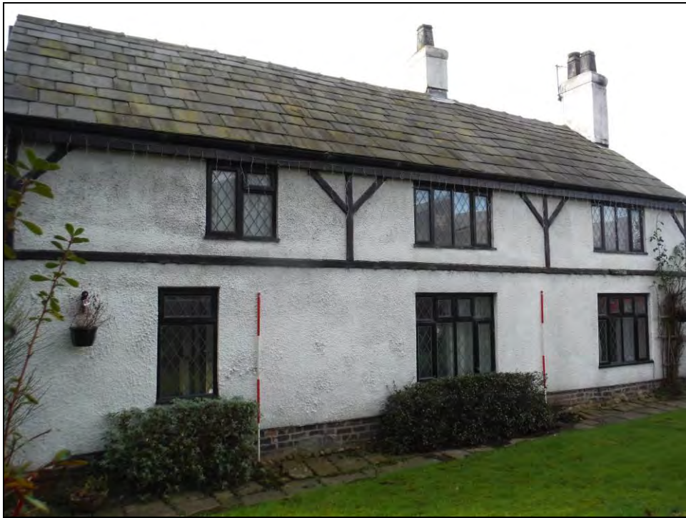
Figure 14. North-east elevation with rough-cast render and mock-Tudor decoration (scale – 2 x 2m).
