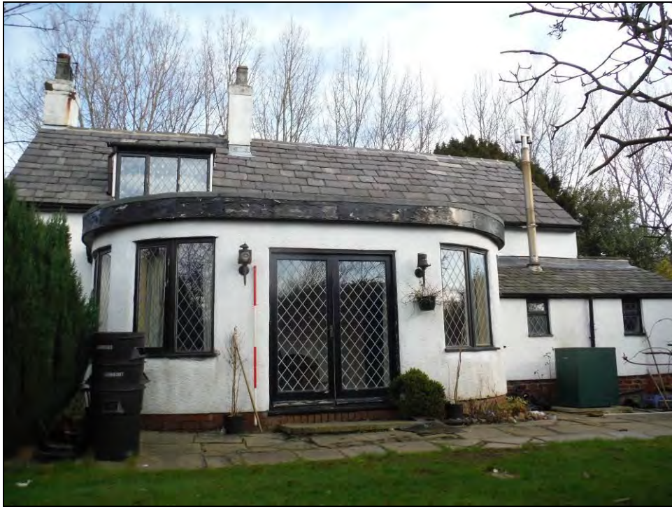
Figure 18. South-west elevation with the curved sun room extension (scale = 1 x 2m).
