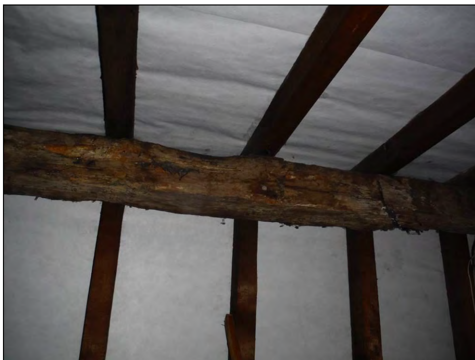
Figure 60. Carved, timber ridge-purlin with modern, replacement common rafters.
