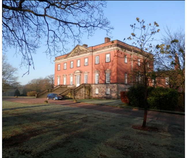
View west of Radbourne Hall.
