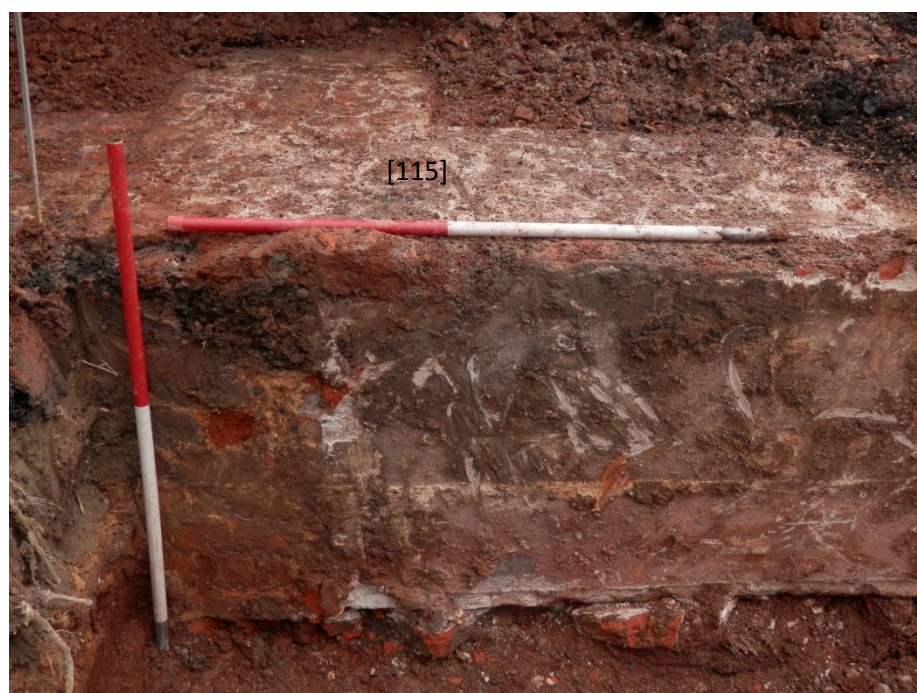
Figure 8: Limewashed mortar on the south-west facing elevation of [115] (scale 1m).
