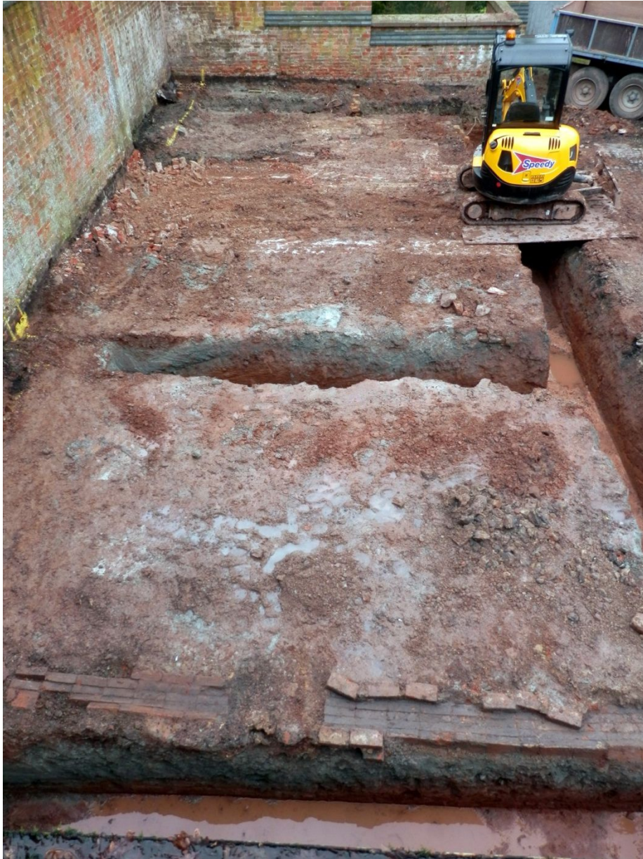
Figure 2: Excavation Area from the south-east, Note drain [120] at bottom of frame.
