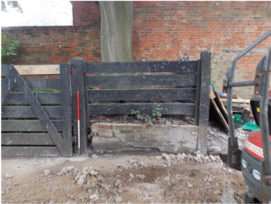
Figure 4. Ground level around the tree adjacent to the development area shows a previous reduction in the ground level, prior to the deposition of made ground deposits.
