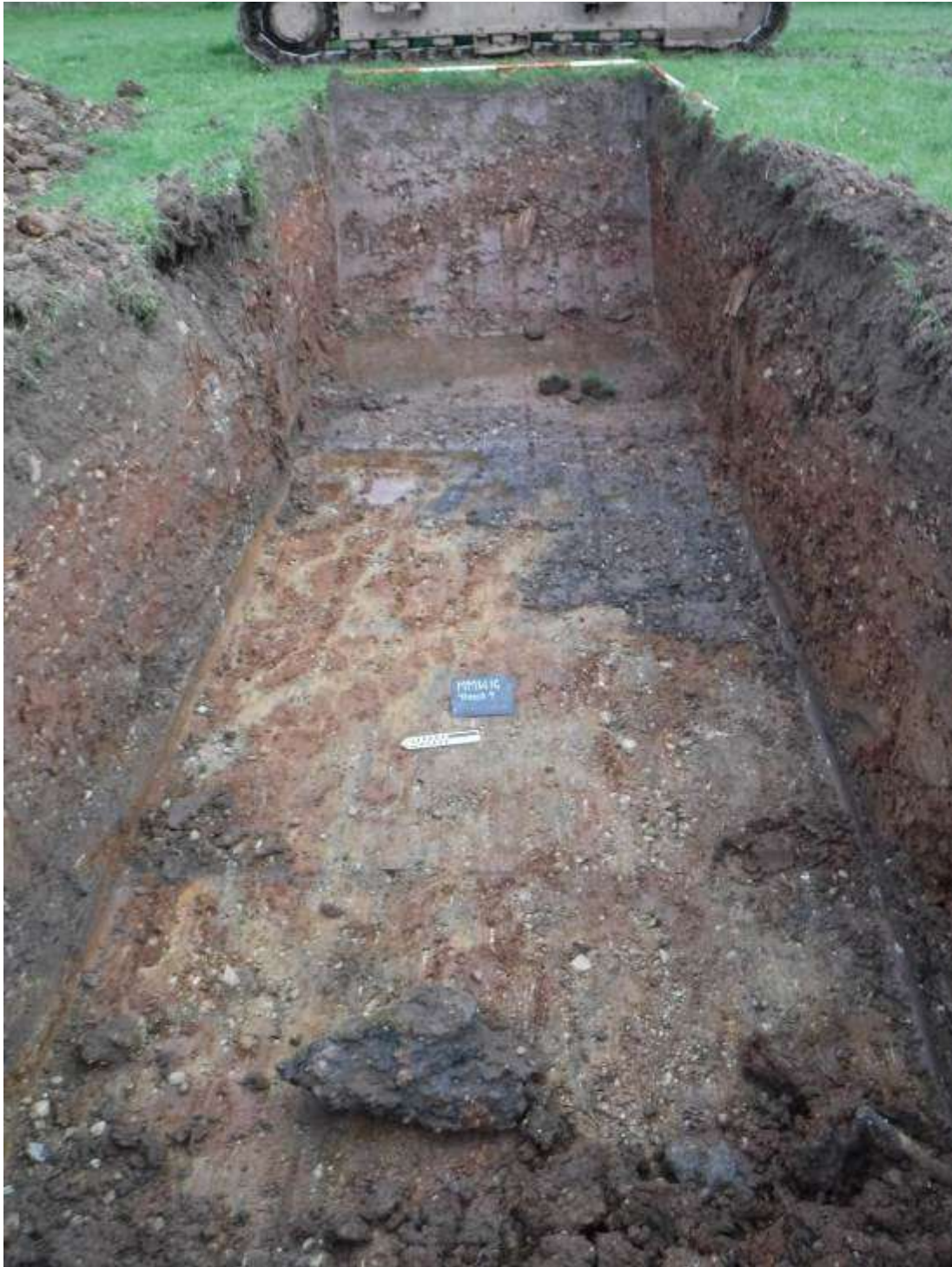
Figure 26: The eastern end of Trench 9 demonstrating depth of made ground prior to backfilling. Note cloth bag in north facing section (scale 2m).
