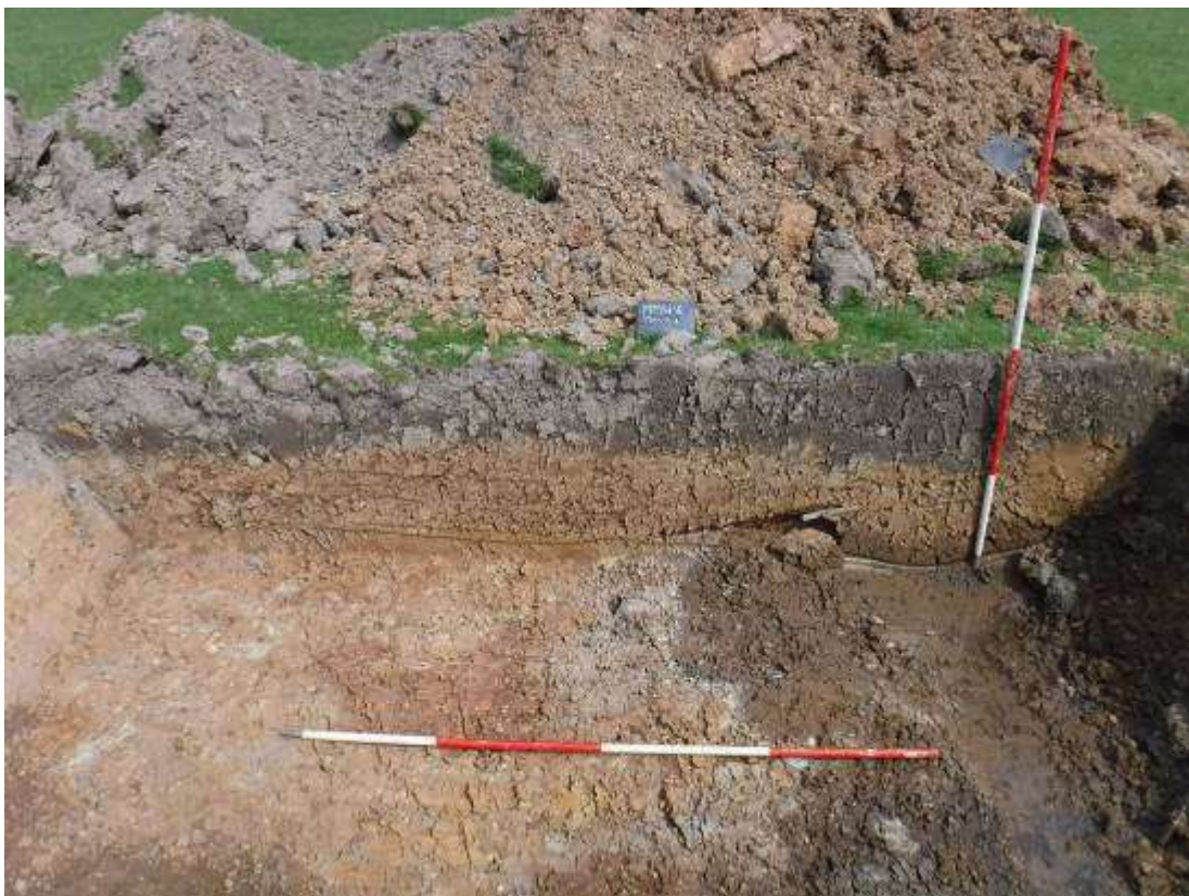
Figure 18: South-eastern end of Trench 6 looking north-east showing levelling up (602) with asphalt and polyethylene pipe (scale 2m).
