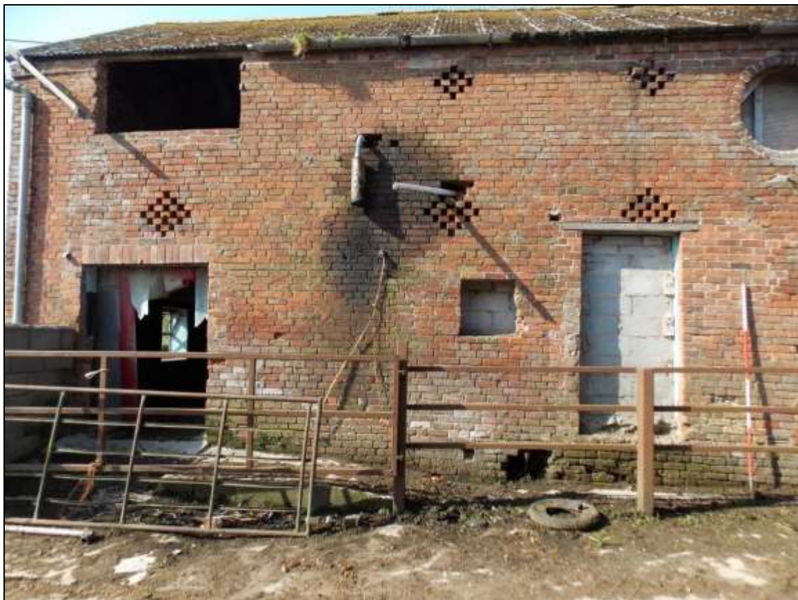
Plate 41: South-east end of the north-eastern elevation (scale 2m).
