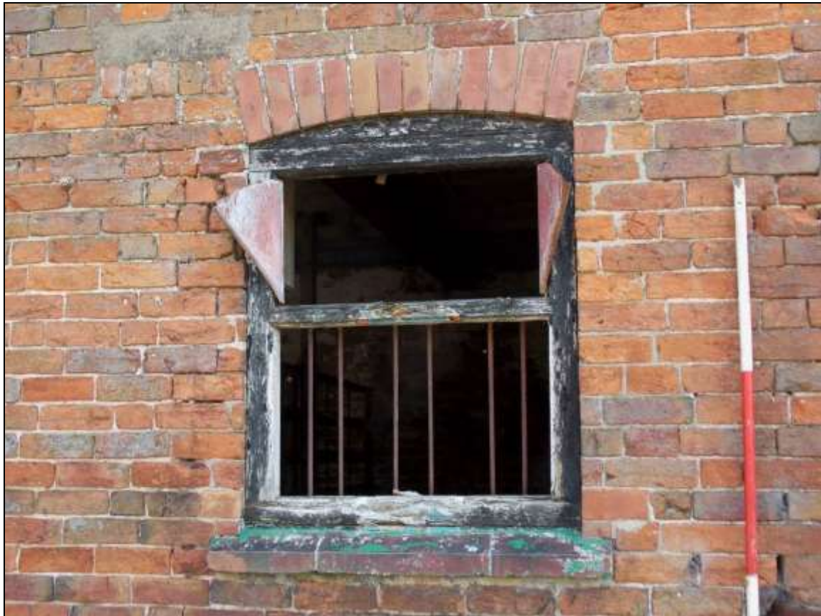
Plate 30: Detail of window opening (scale 2m).
