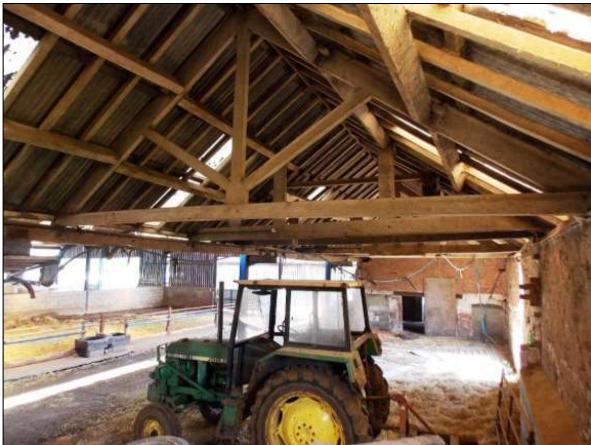
Plate 65: North-eastern king-post truss with pegged joints, looking north-east.
