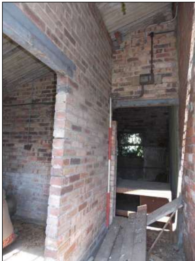
Plate 87: Passageway of Building I, looking north-west (scale 2m).
