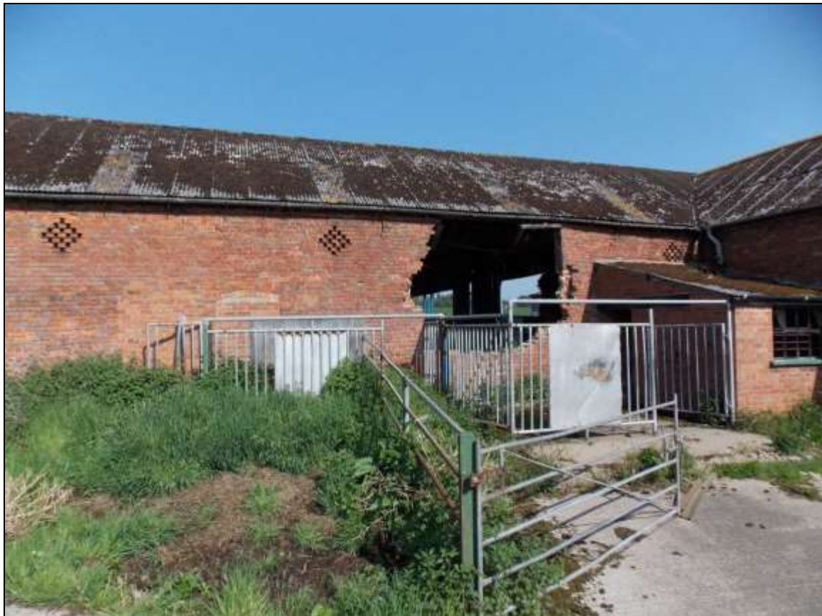
Plate 70 South-eastern elevation of Building G facing onto the courtyard.
