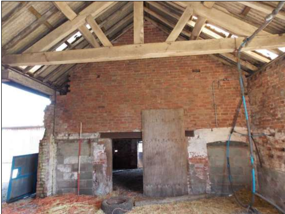
Plate 8: Doorways within the south-western gable wall, looking north-east (scale 2m).
