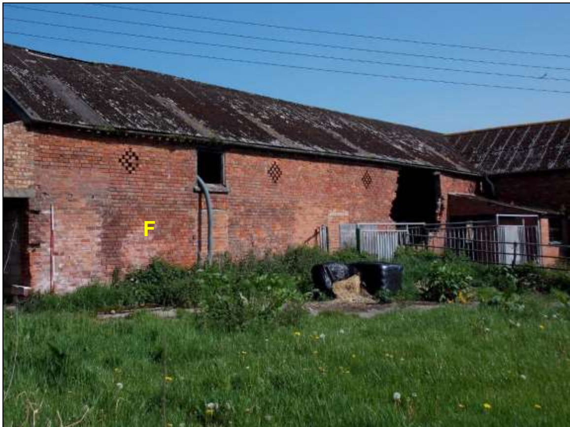
Plate 60: South-east elevation of Building F facing onto the courtyard (scale 2m).
