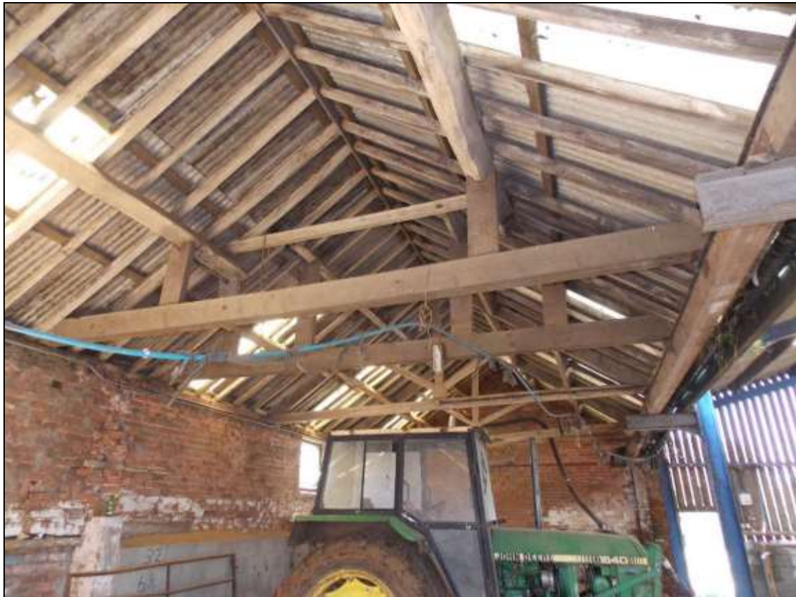
Plate 64: Internal view of Building F, looking south-west.
