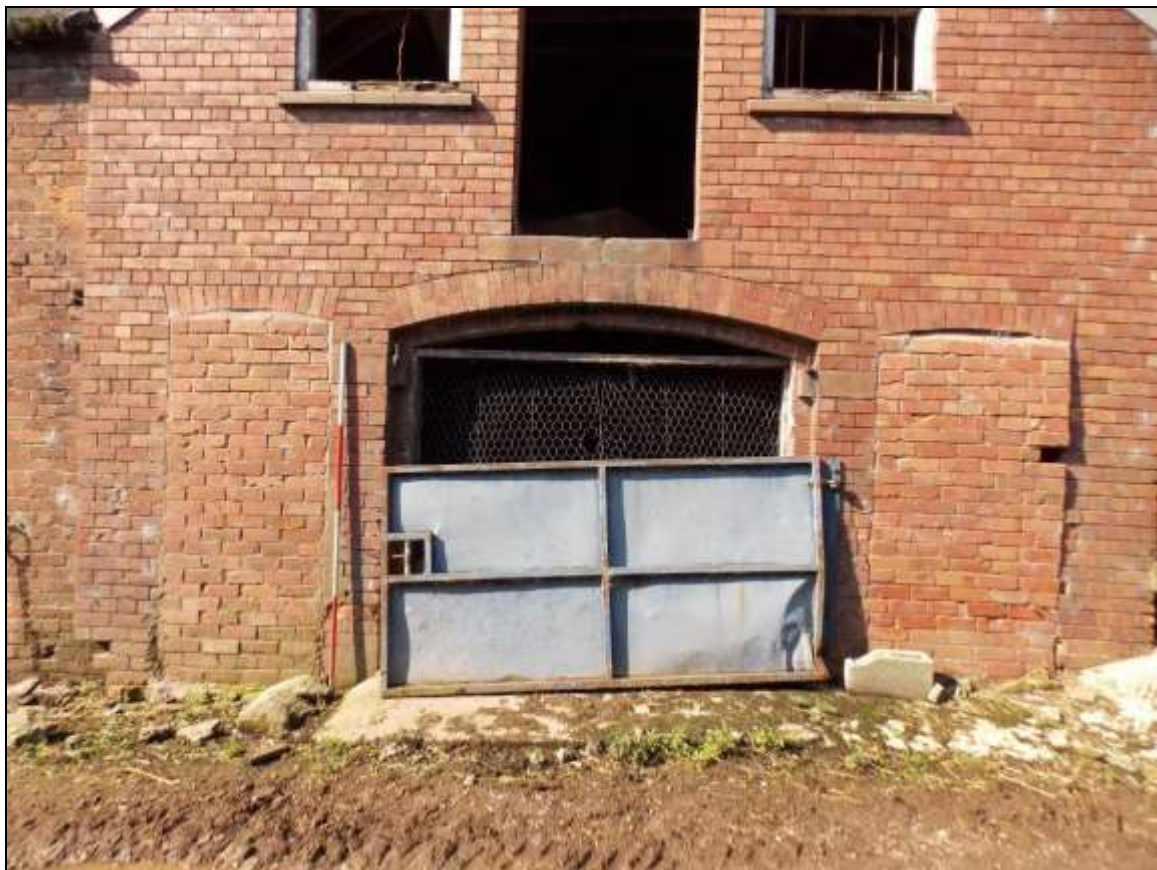
Plate 5: Detail of central doorway flanked by blocked-up side doorways, looking south-west (scale 2m).
