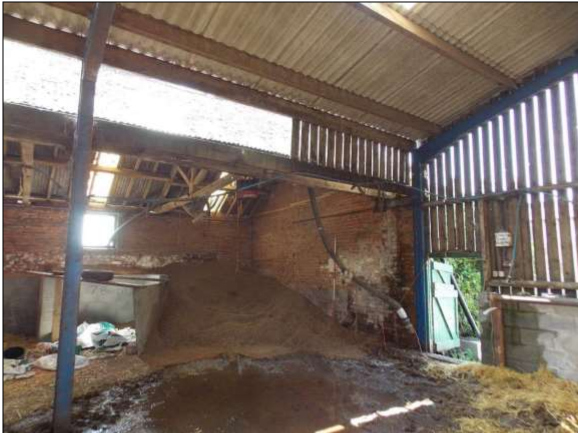
Plate 63: South-western end of Building F, looking south (scale 2m).
