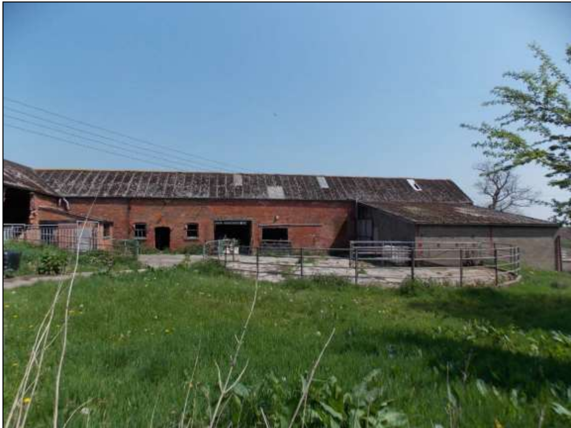
Plate 58: Building E projecting into the courtyard, looking north-east.
