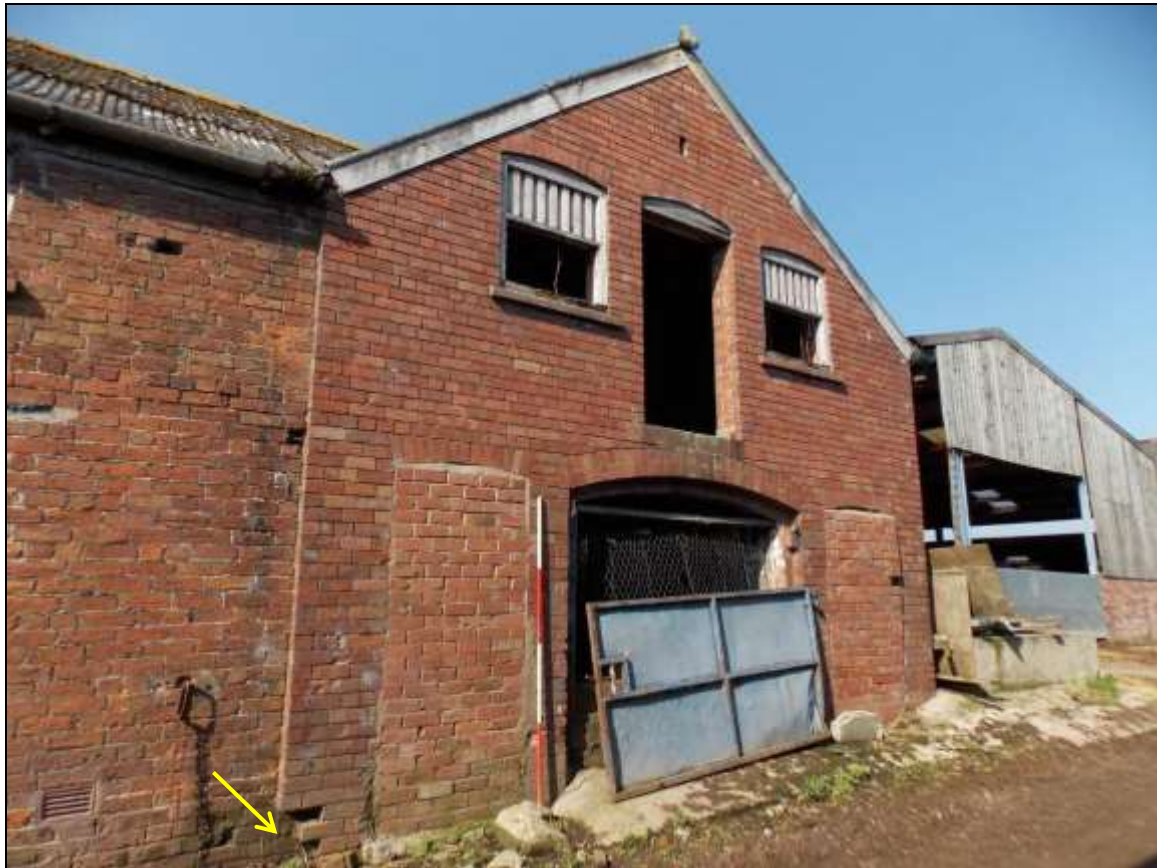
Plate 4: Front elevation of Building A covering earlier brickwork (arrow), looking north-west (scale 2m).
