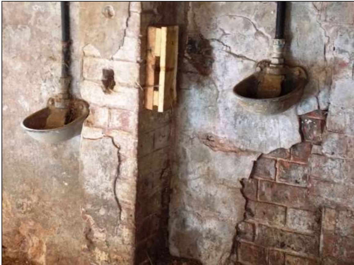
Plate 23: Detail of troughs on the south-western wall.
