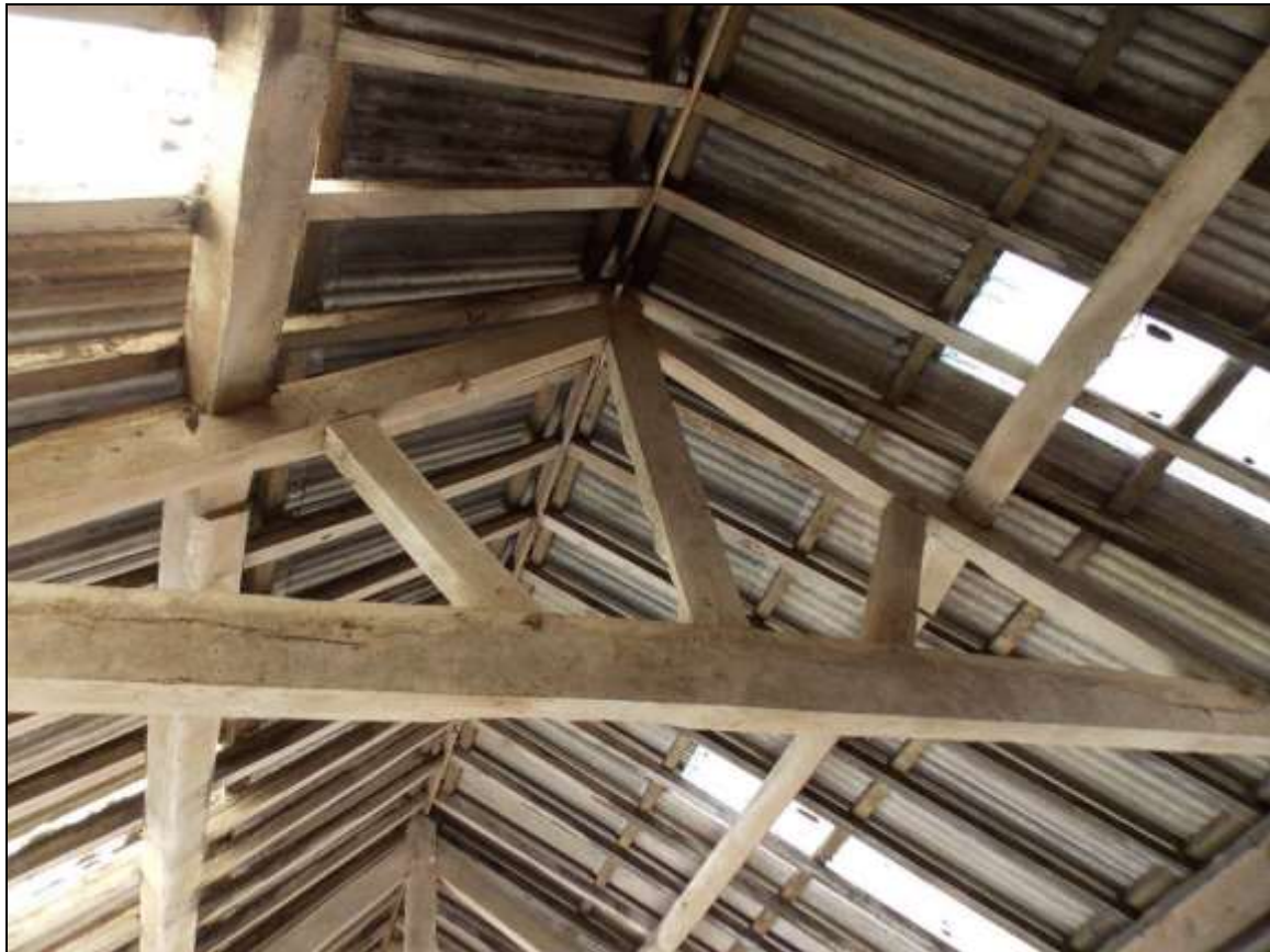
Plate 78: North-eastern king-post truss with pegged joints, looking south-west.
