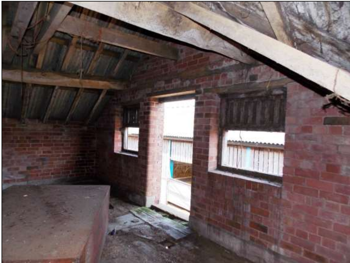
Plate 12: First floor of Building A, looking north-west.
