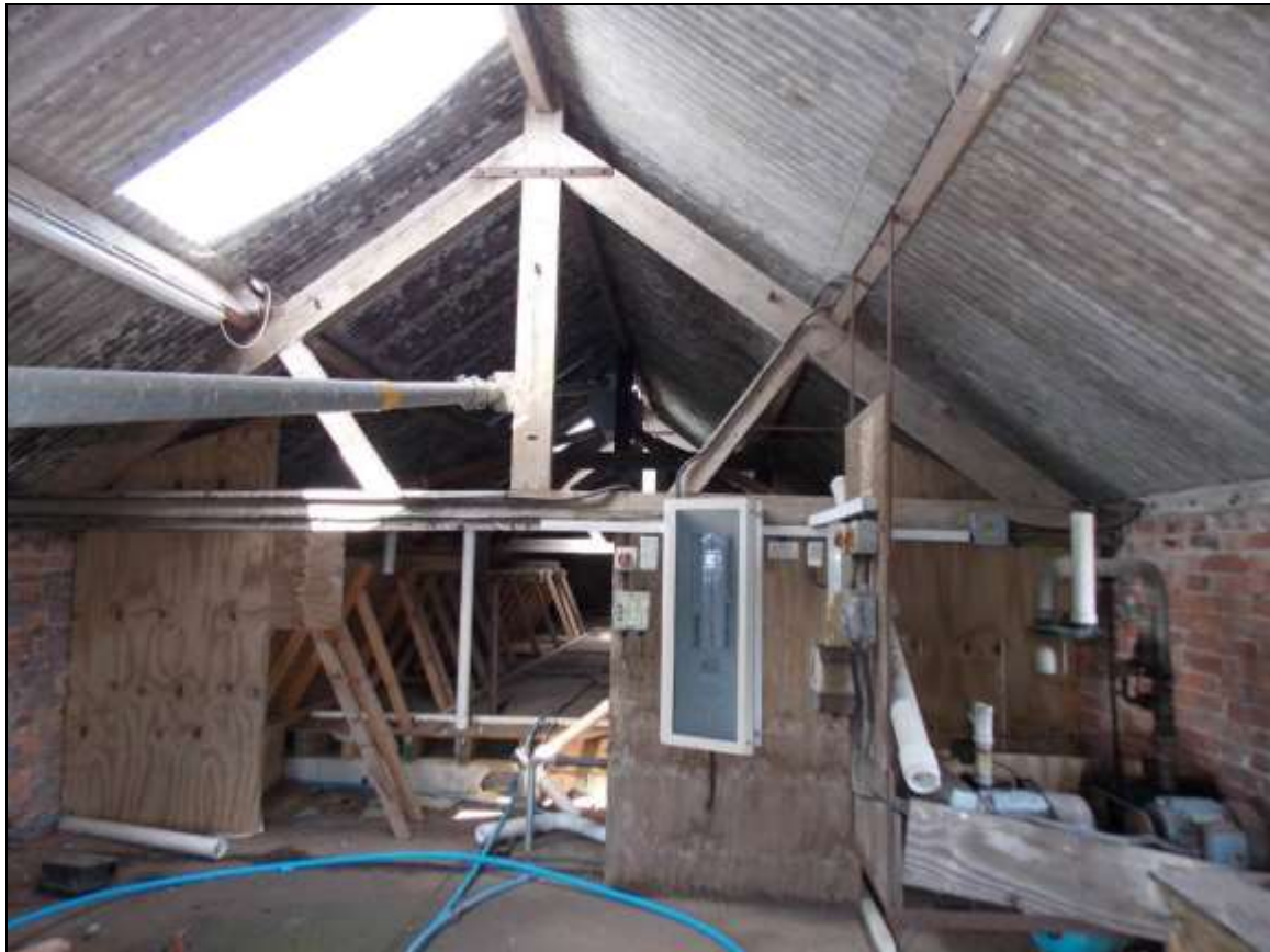
Plate 53: South-eastern end of the loft storey, looking north-west.
