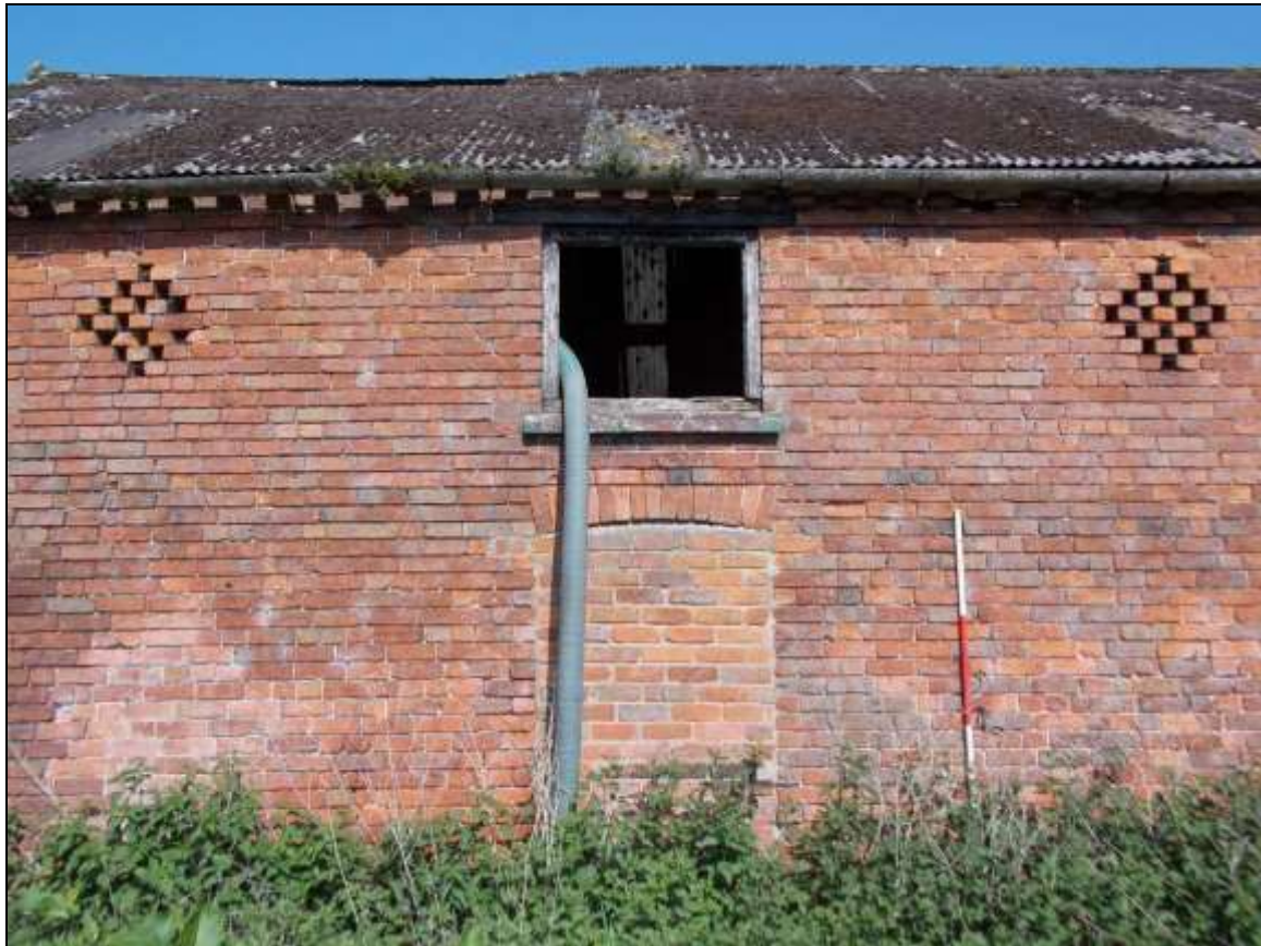
Plate 61: Blocked-up central doorway, looking north-west (scale 2m).
