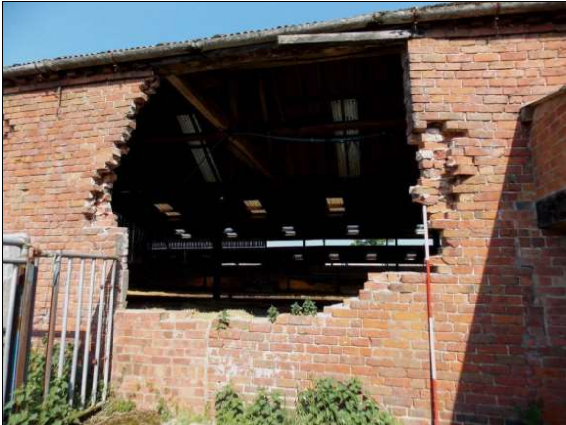
Plate 71: Partially destroyed wall with remnants of a former window and a blocked-up doorway (scale 2m).
