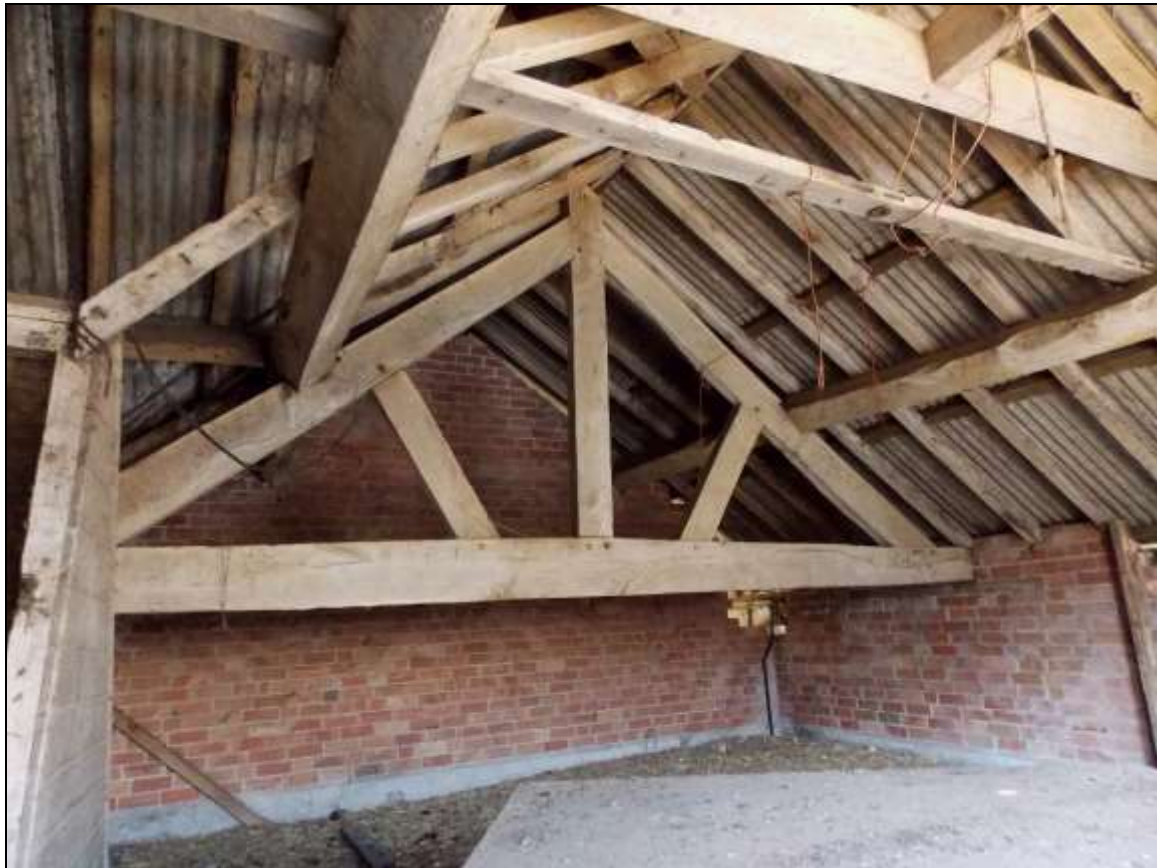
Plate 14: King-post timber truss with pegged joints, looking south-west.
