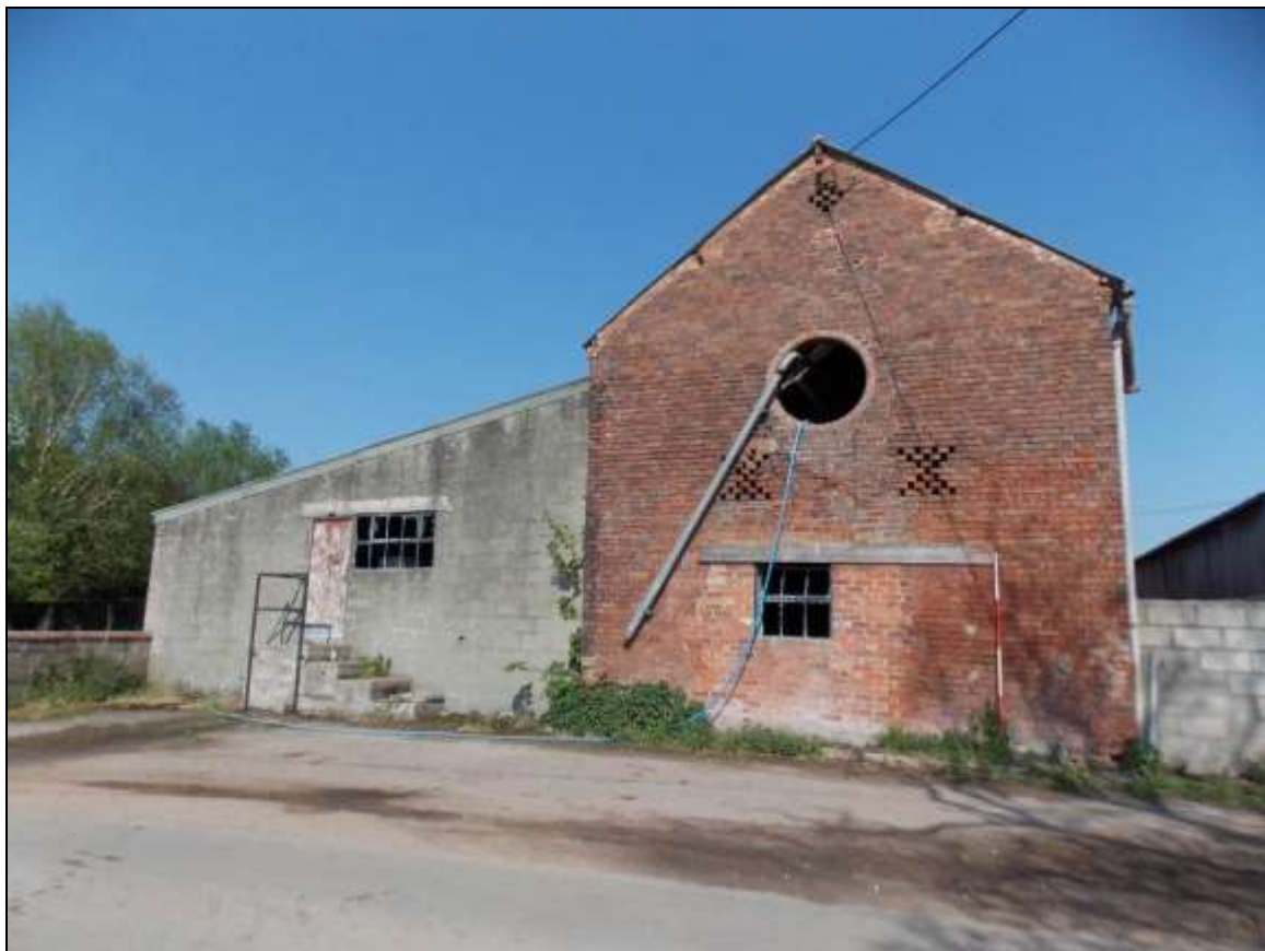
Plate 39: Gable wall facing onto Black Park Road (scale 2m).
