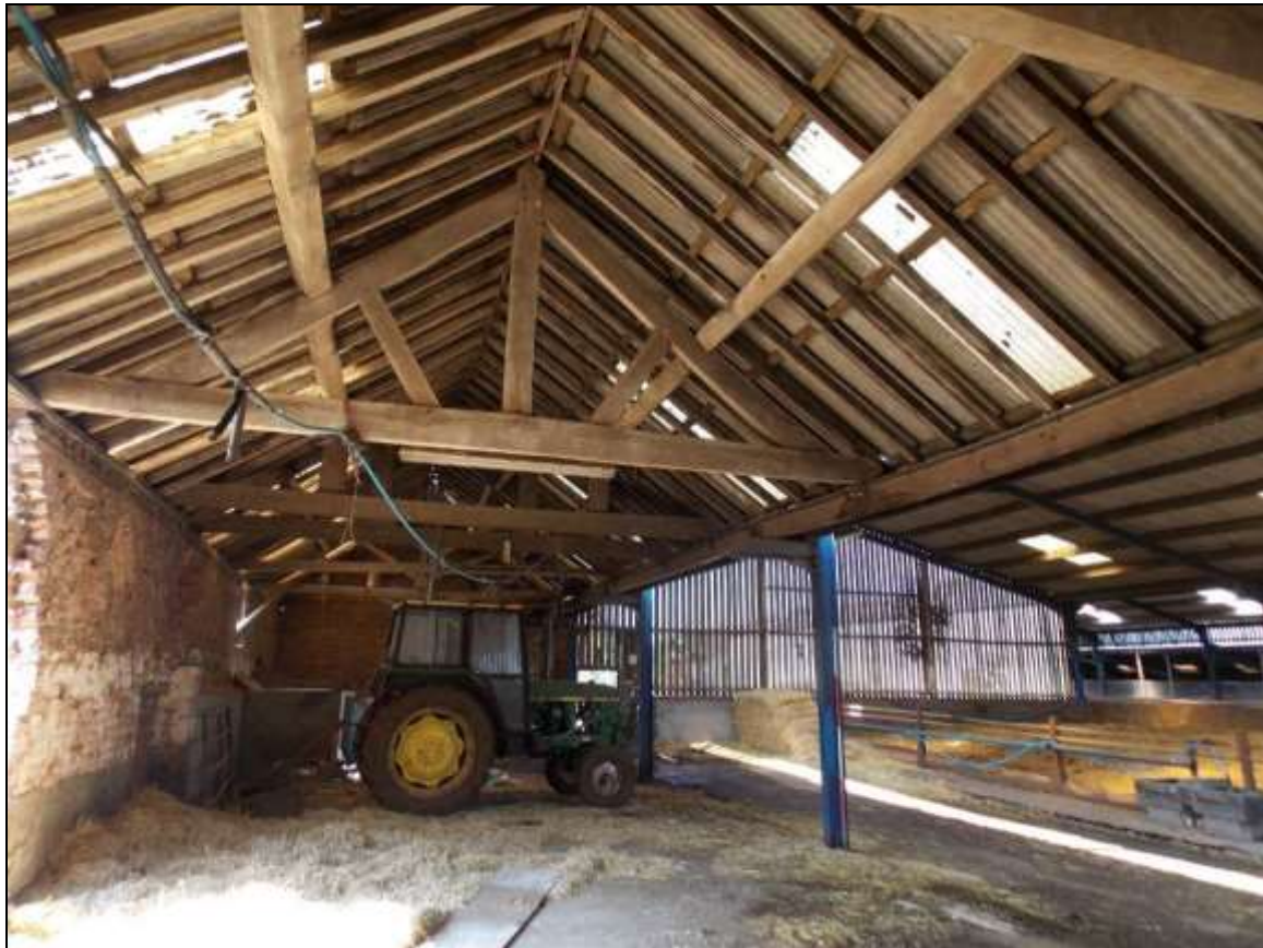
Plate 80: South-western king-post truss of Building G, looking south-west
