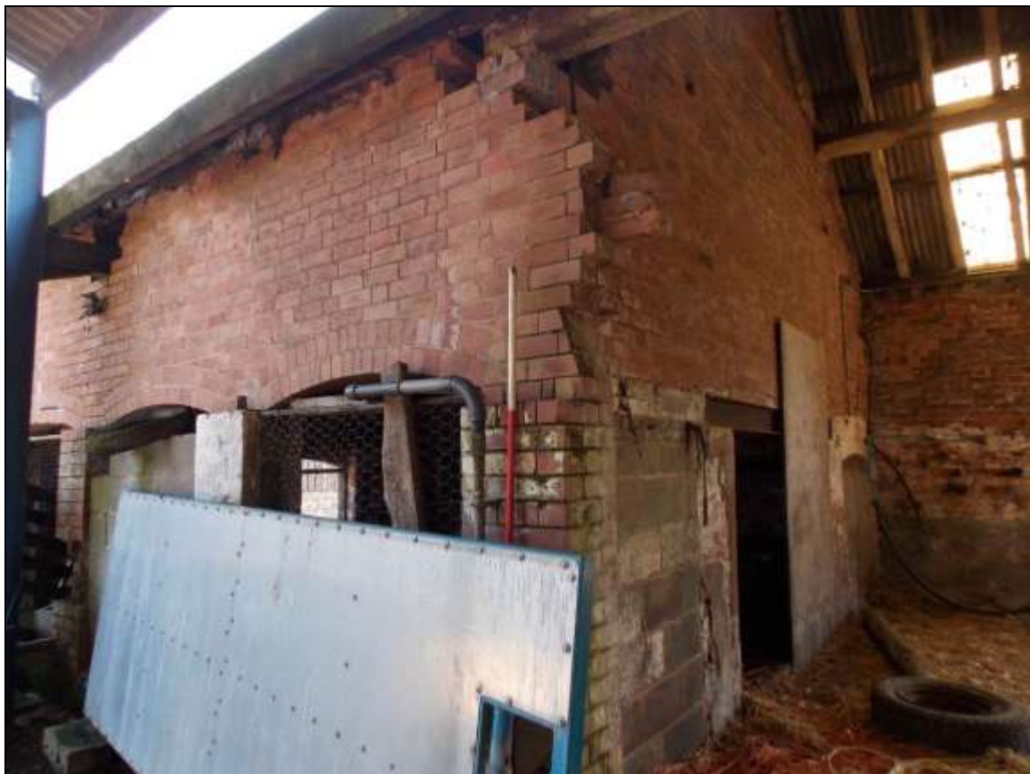
Plate 7: Detail of truncated arcade, looking north-east (scale 2m).
