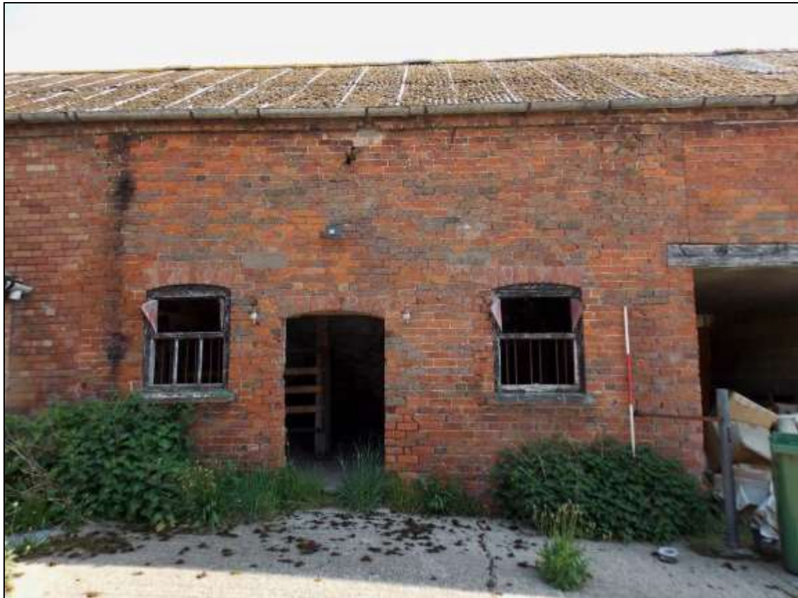
Plate 28: South-western elevation facing onto the courtyard (scale 2m).
