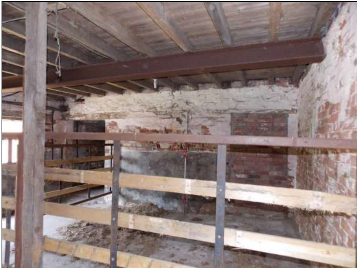
Plate 32: Ground floor of Building C, looking north-west (scale 2m).
