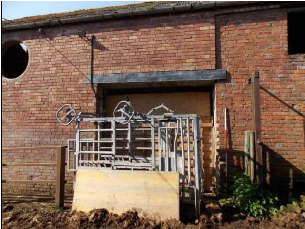
Plate 44: Gate for livestock leading to a large inserted passageway, looking south-west (scale 2m).
