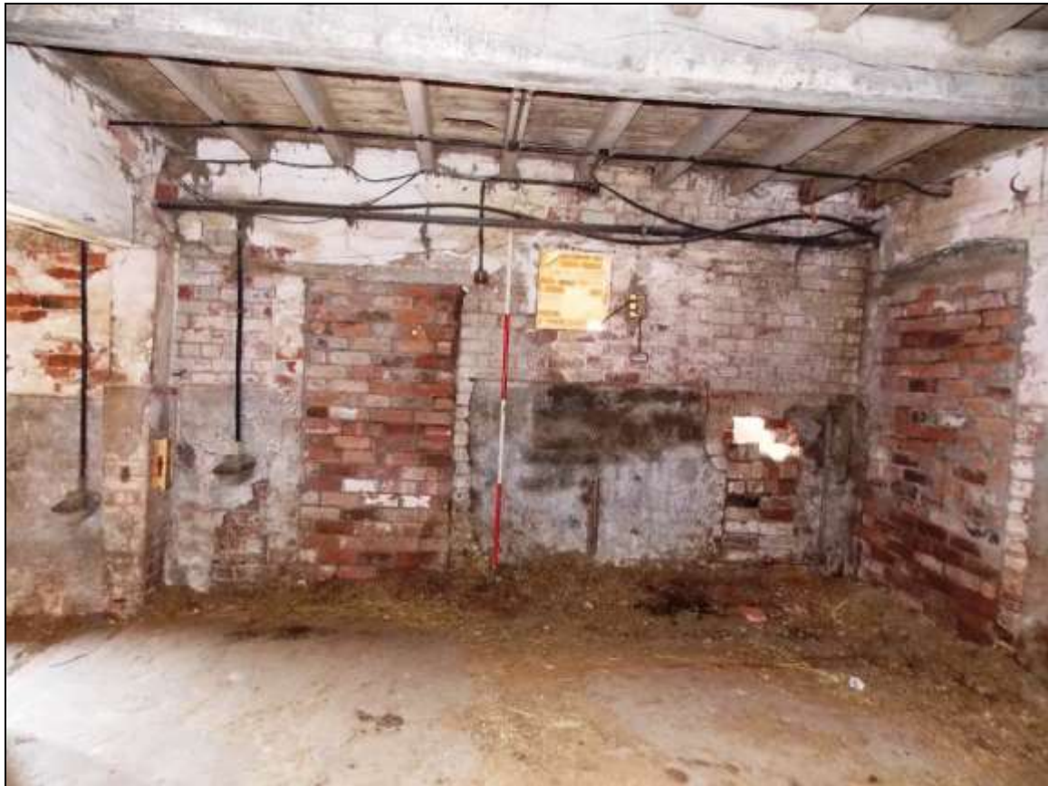
Plate 21: South-western wall with blocked-up openings (scale 2m).
