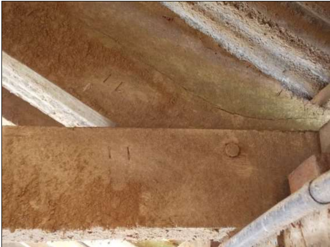
Plate 68: Upper face of truss with peg's heads and associated carpenter's assembly marks.
