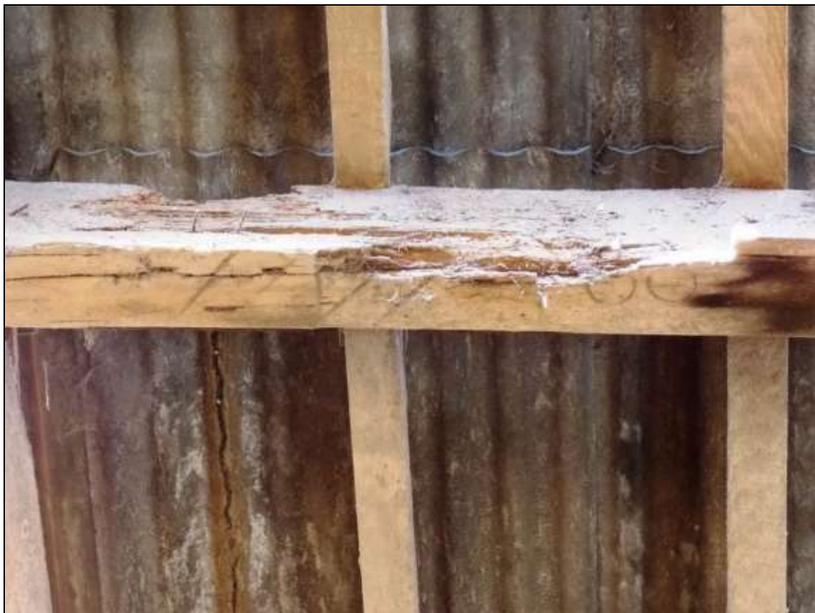
Plate 69: Shipping mark within a side purlin of Building F.
