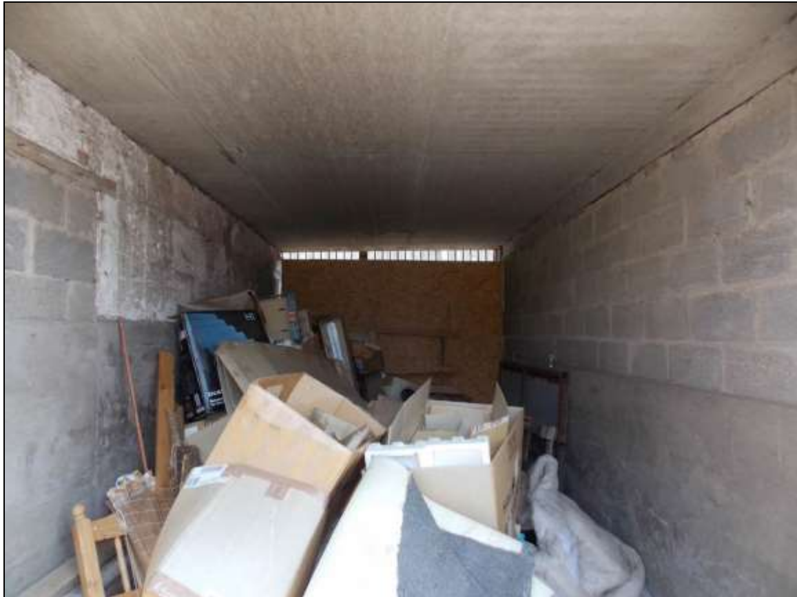
Plate 48: Internal view of the passageway of Building D, looking north-east.
