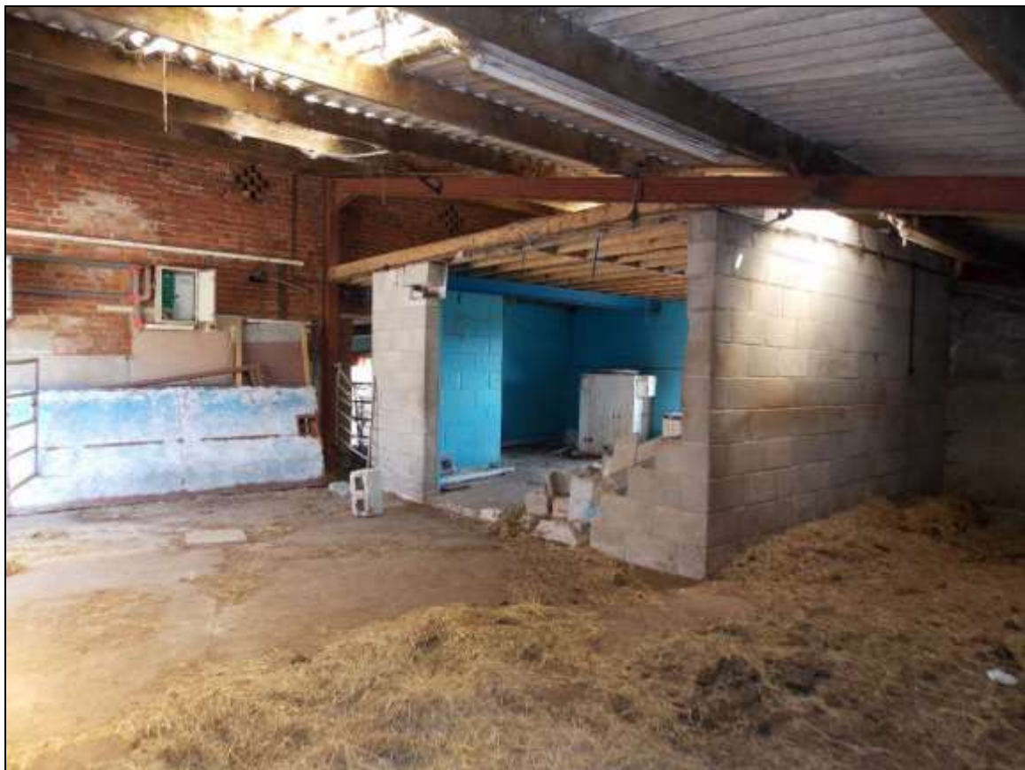
Plate 59: Internal view of Building E, looking east.
