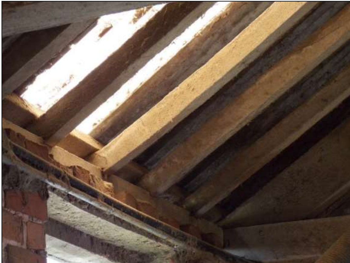
Plate 66: Common rafters with bird mouth joints attaching the south-eastern wall plate.
