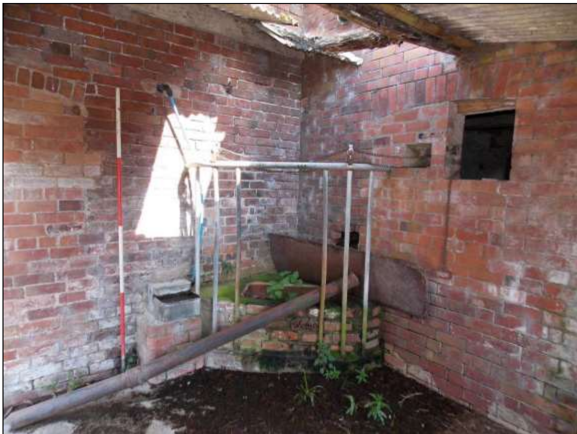
Plate 84: Internal view of Building H, looking north (scale 2m).
