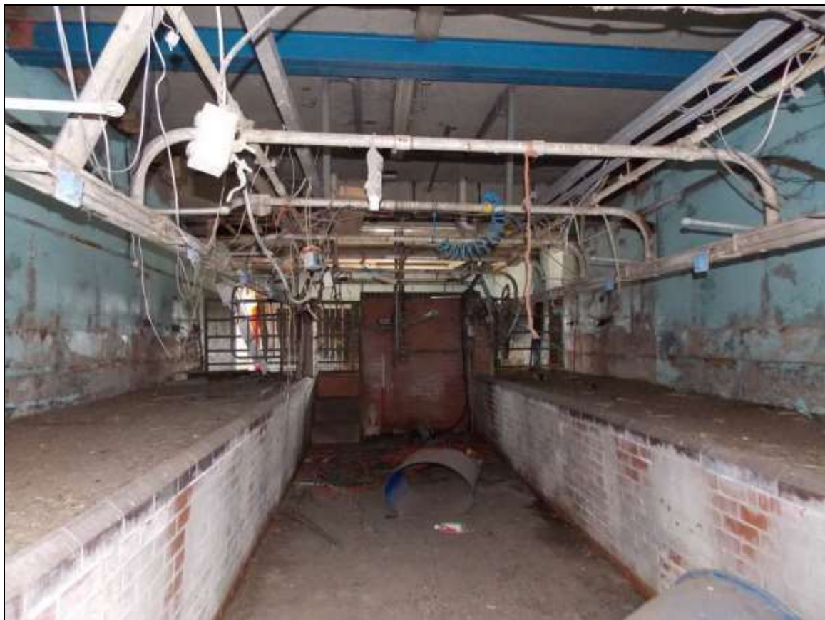
Plate 50: Detail of central pit of the milking parlour, looking south-east (scale 1m).
