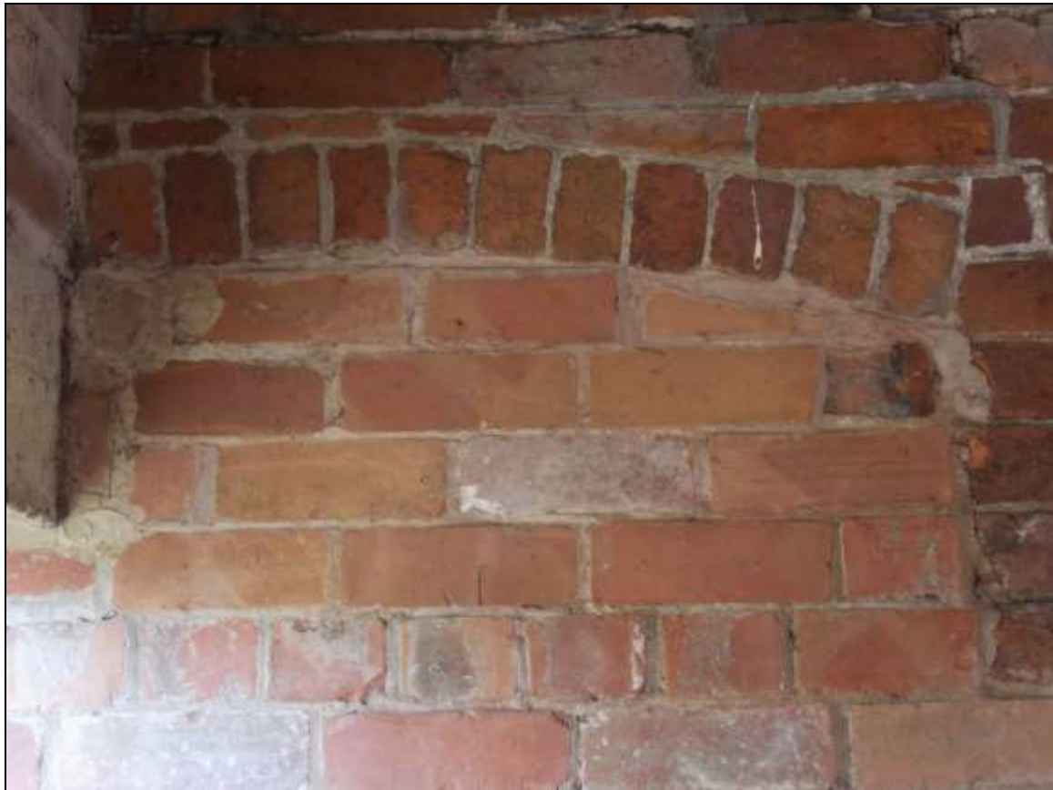
Plate 73: Blocked-up window opening abutted by Building H, looking north-west.
