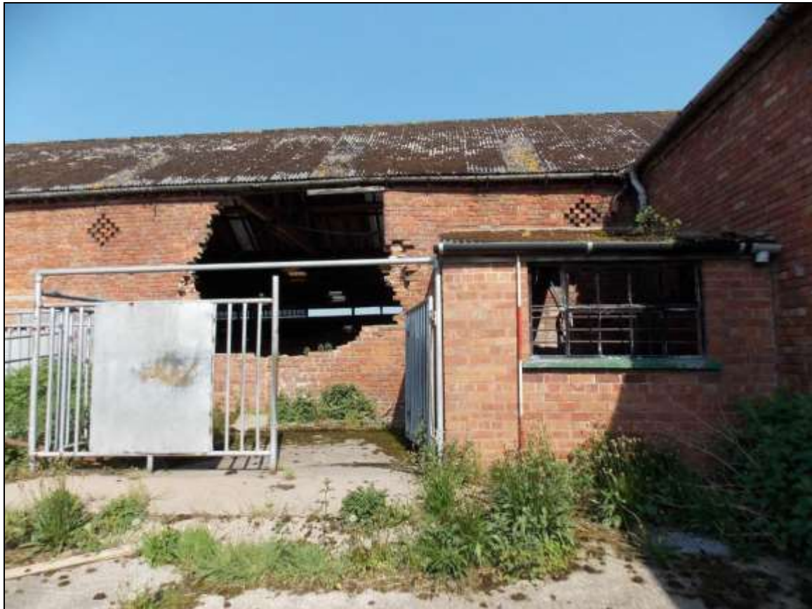
Plate 83: South-eastern wall of Building H (scale 2m).
