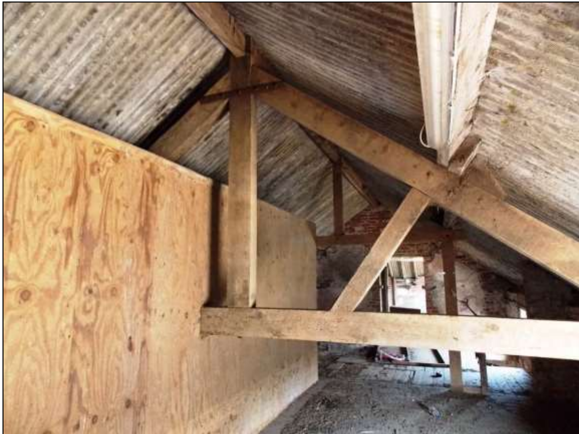
Plate 35: Loft storey of Building C with bolted king-post truss, looking north-west.
