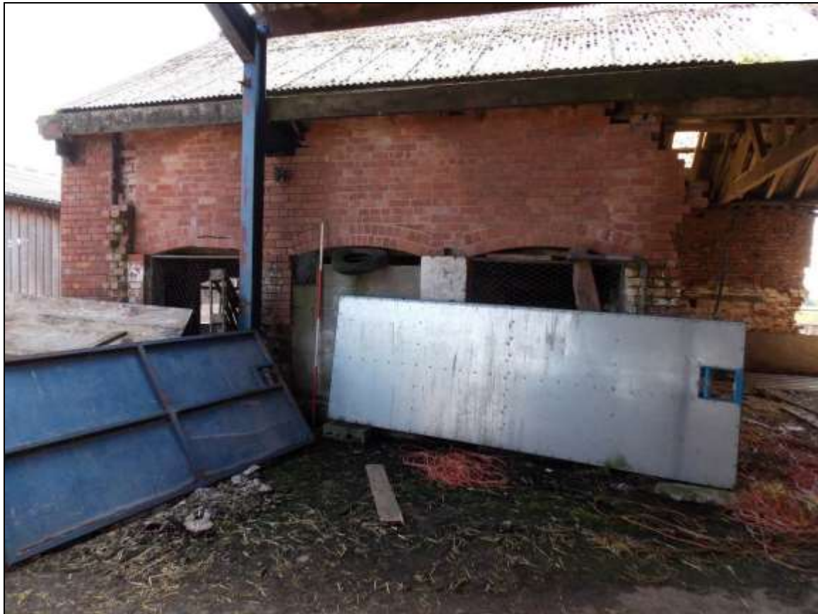
Plate 6: Arcaded elevation of Building A, looking south-east (scale 2m).
