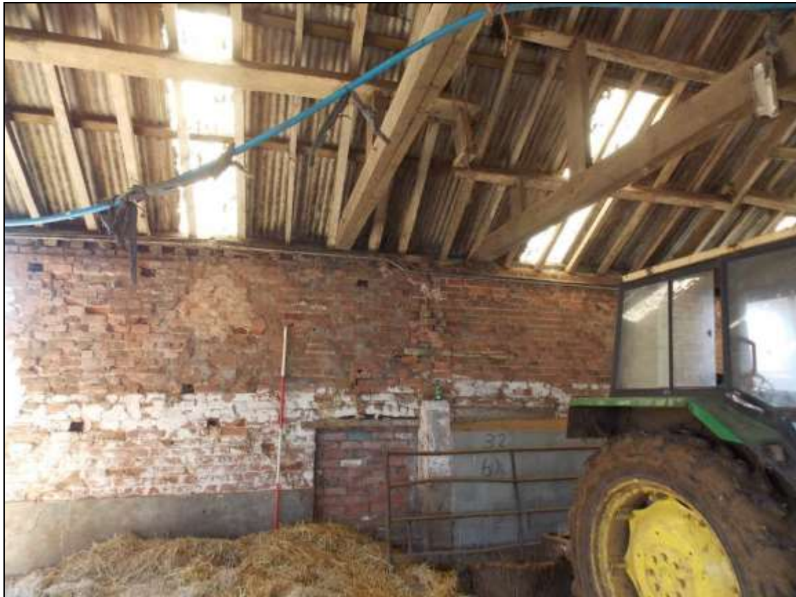
Plate 76: Vertical construction scar (arrow) and improvised trusses above it, looking south-east.
