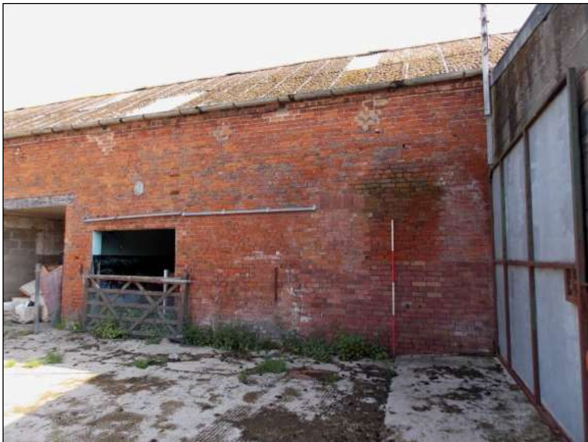
Plate 47: South-western elevation with blocked-up vents and a doorway (scale 2m).
