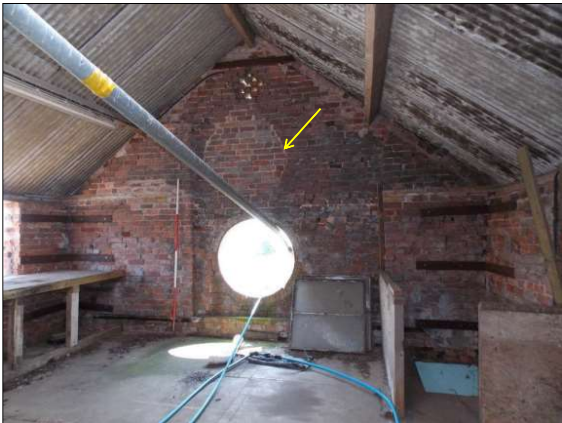
Plate 56: Gable wall with an inserted oculus which substituted a comparable opening above it (arrow).
