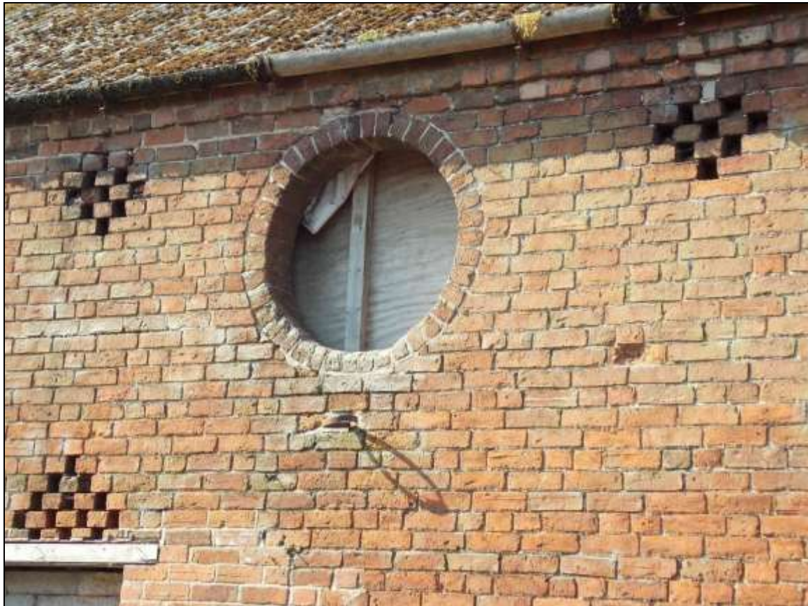
Plate 42: Detail of oculus and diamond-shaped vents within the north-eastern elevation.
