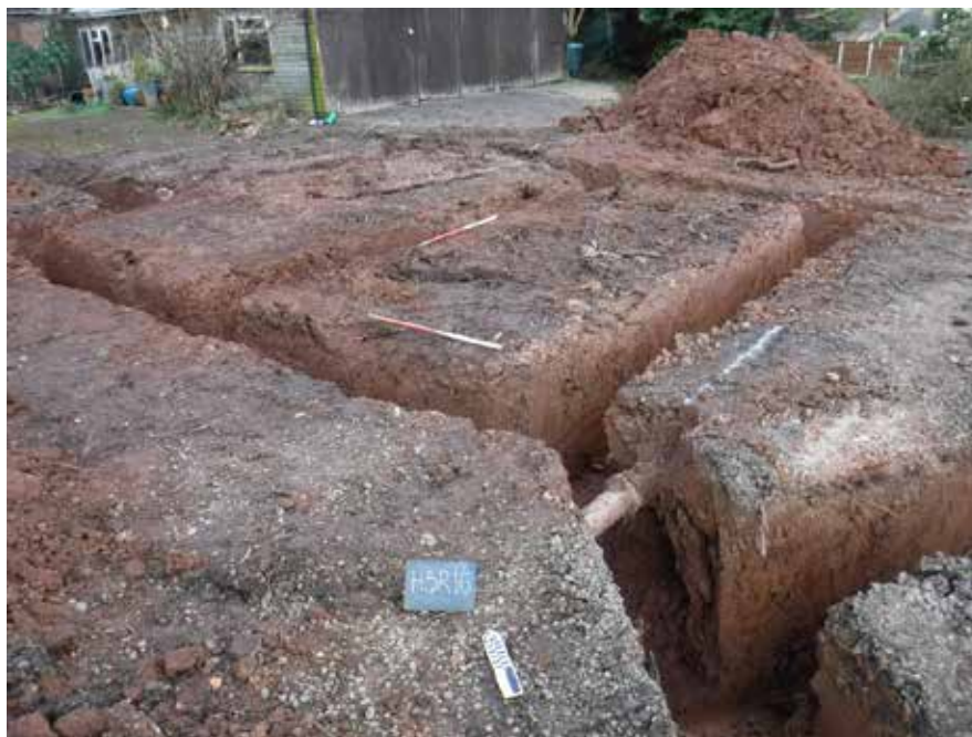
Figure 4. View north across the footing trenches (scale = 0.5m graduations)
