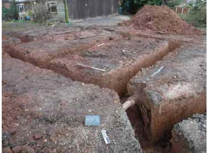
View north overlooking groundworks.
