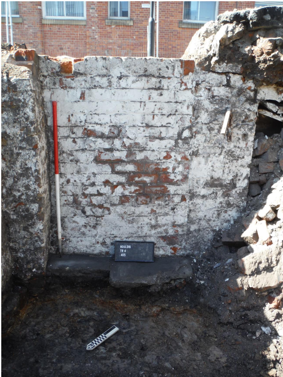
Figure 26. Walls F405 & F407, and flagstones (404), looking southwest (scale 1m)
