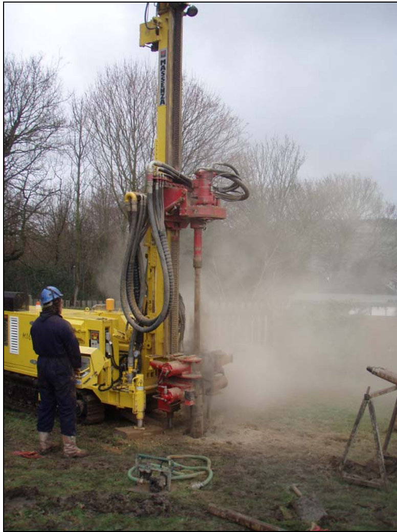
Figure 4. Rotary bore hole 1 under excavation.
