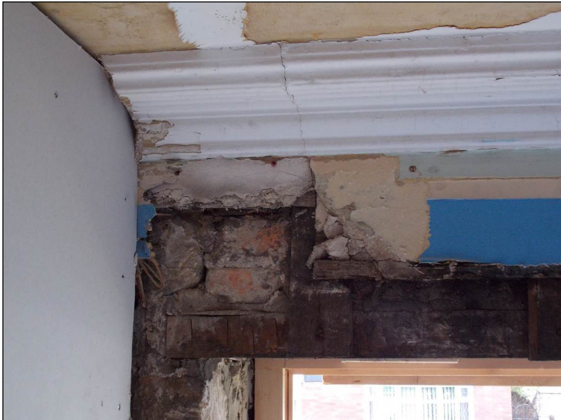
Figure 7: Detail of original timber lintel and brickwork above it.
