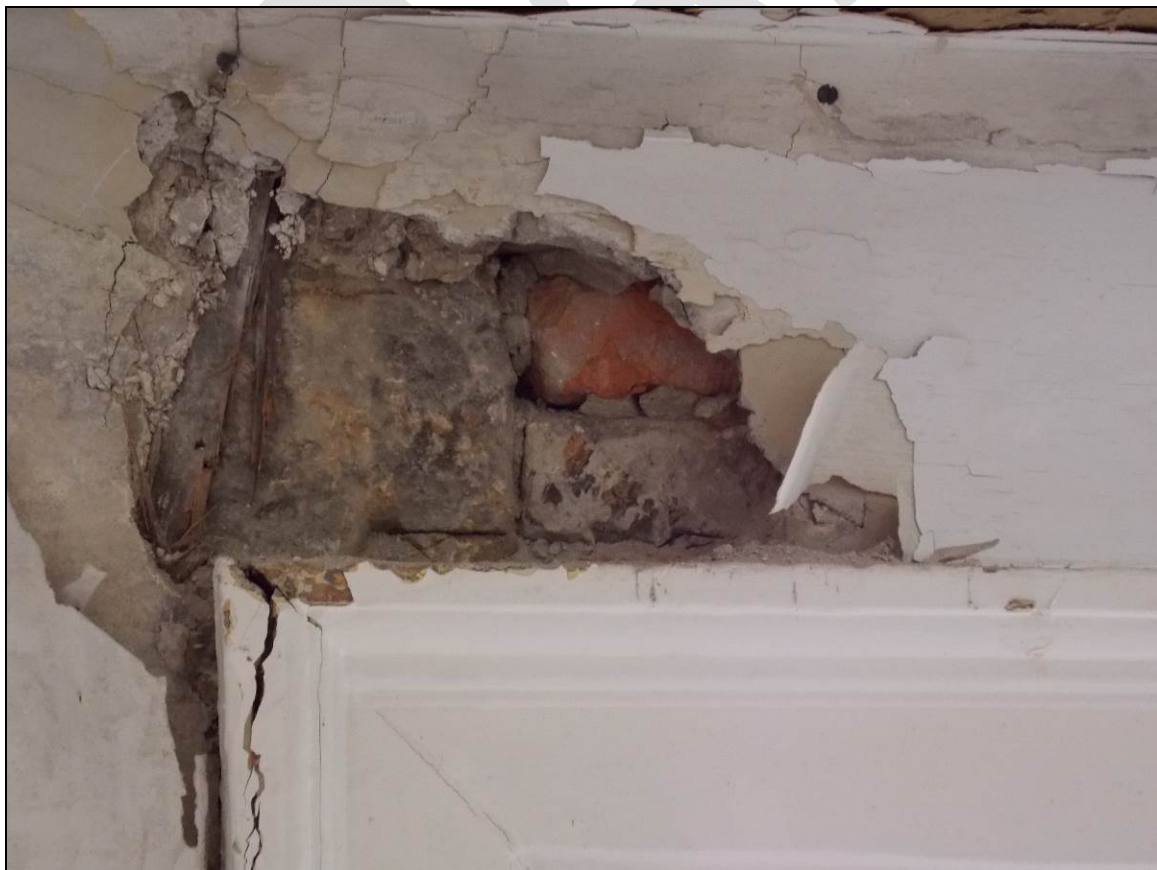
Figure 10: Detail of brickwork above window lintel within room G2.
