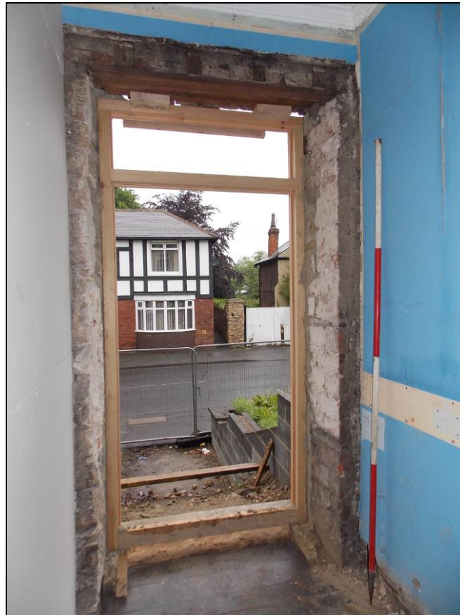
Figure 5: Internal view of the inserted doorway (scale 2m).
