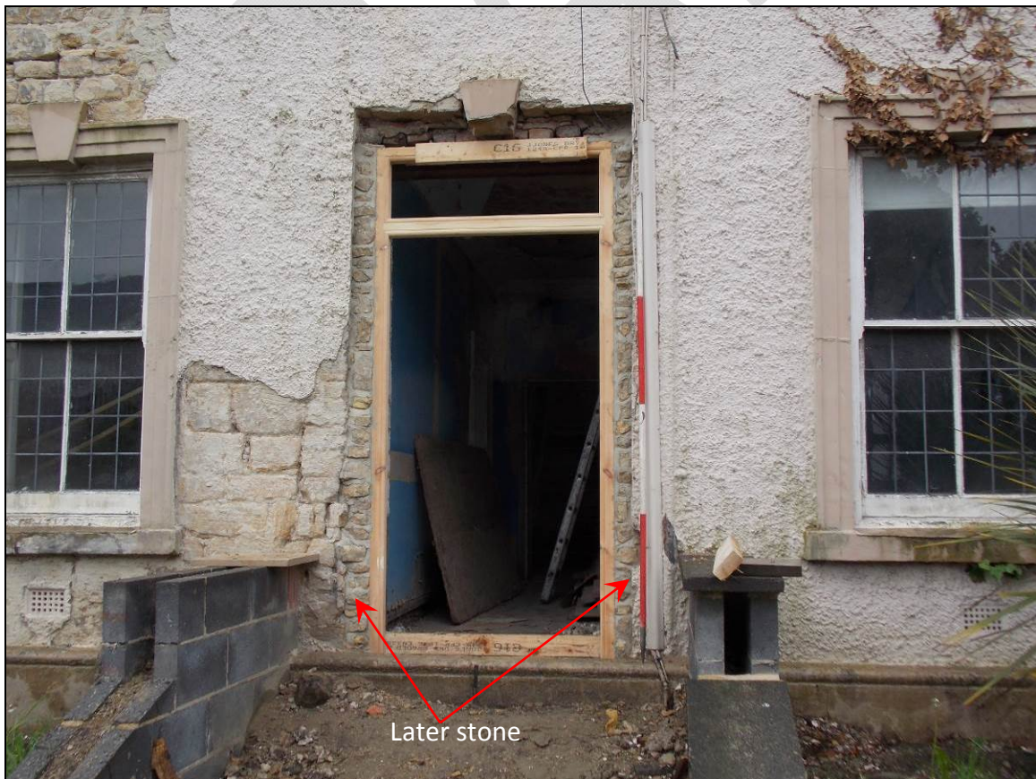
Figure 4: Detail of the central window opening modified into a doorway (scale 2m).
