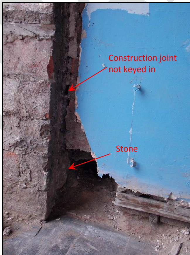
Figure 8: Brick jamb and later brick wall abutting the stone north wall.
