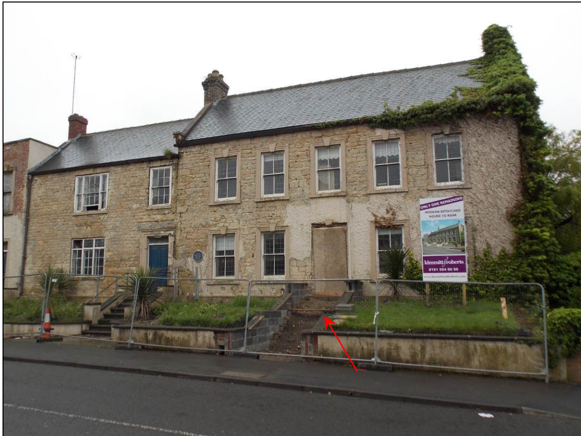
Figure 3: Front facade of Hetton House with inserted doorway and stairwell (arrow).
