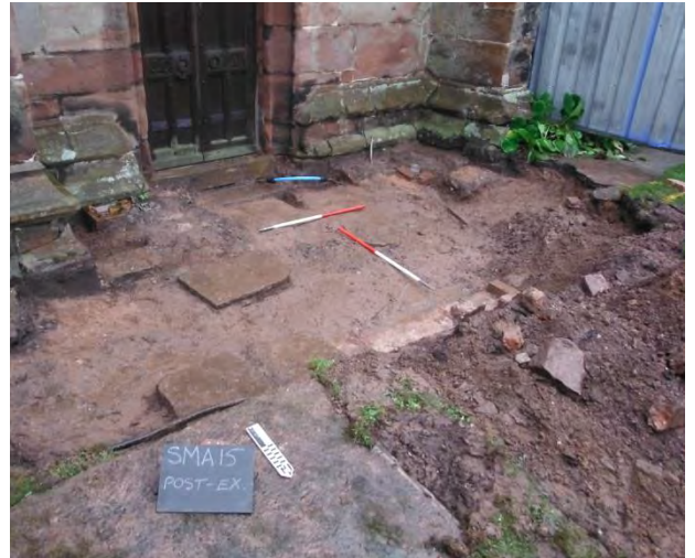
Post excavation view of trench, looking south-west.
