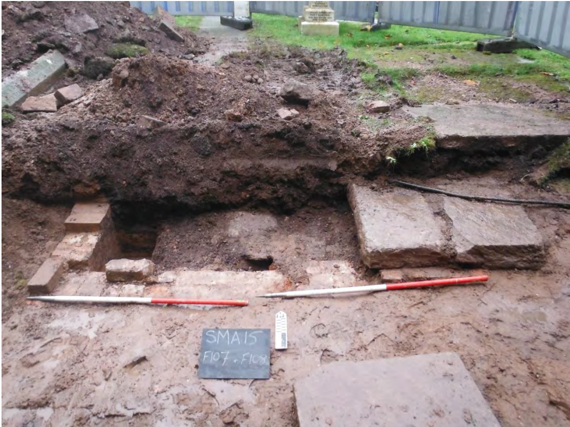
Figure 8. View looking north of the brick-built grave/crypt structure (F107) with overlying capping stones (F108) at the northern extent of the trench. Scale = 0.5m graduations.
