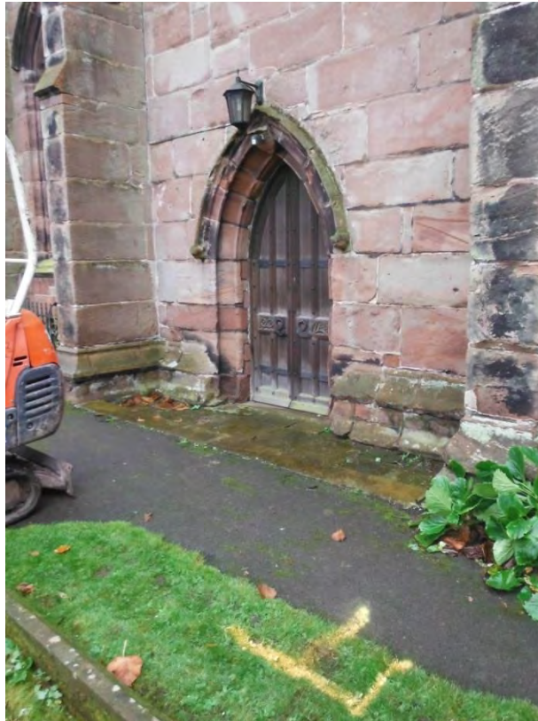
Figure 3. View of the development area looking south-east prior to excavation. Yellow paint marks the north-western corner of the trench.
