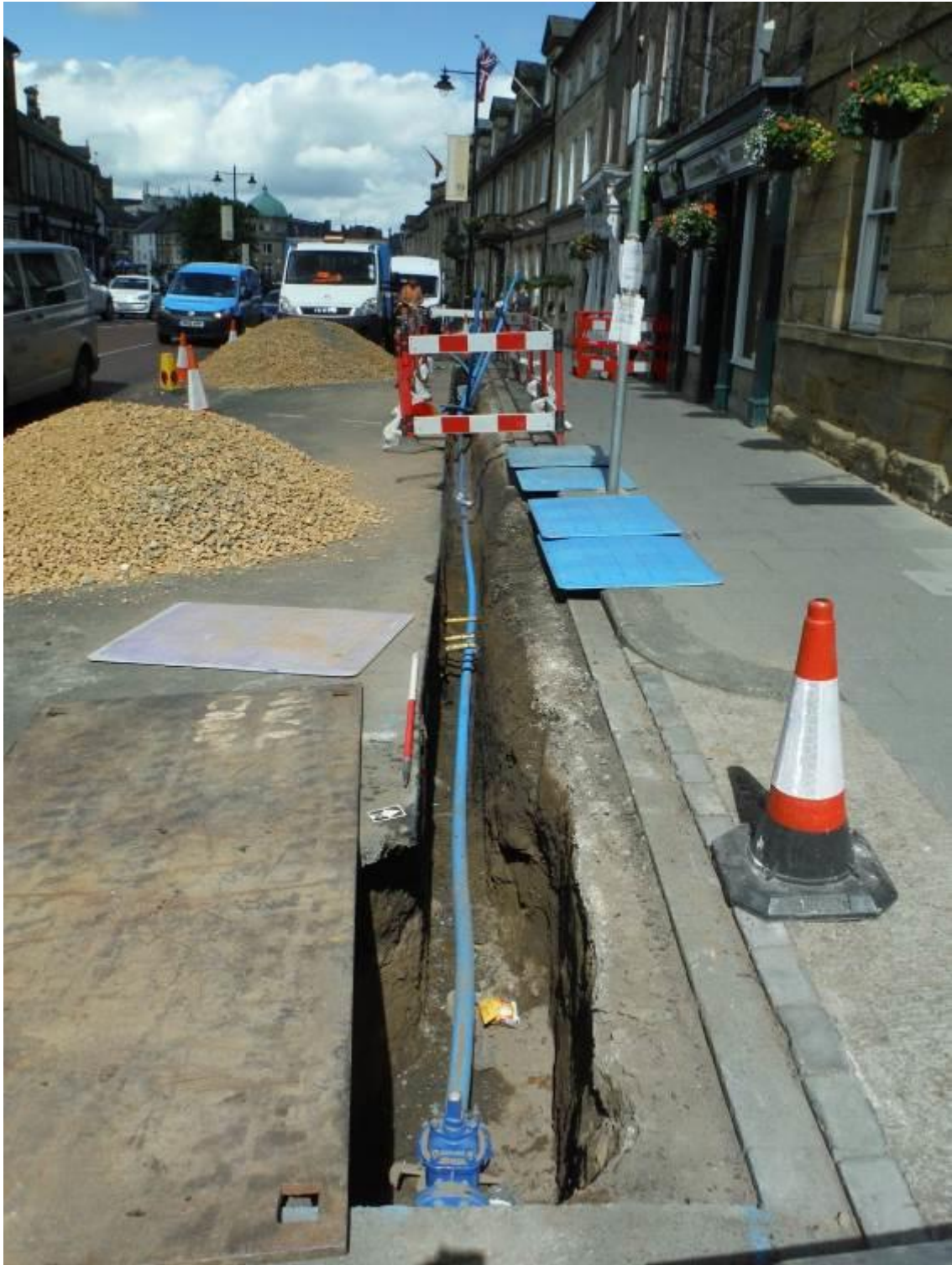
Figure 9: View of the trench looking north west (scale = 1 x 1m).
