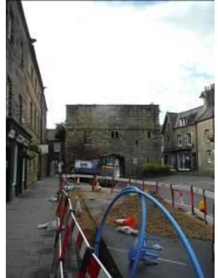
View looking south east towards Bondgate Tower.
