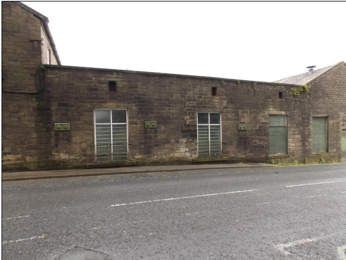
Plate 20: Building 3 facing onto Bolton Road North, looking south-east.
