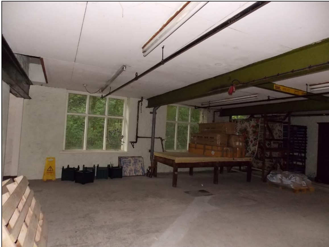
Plate 53: Ground floor of Building 12, looking south-east.
