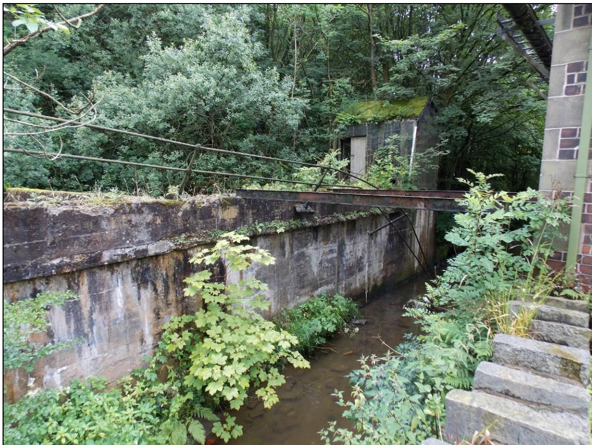
Plate 64: The tanks and shed along Dearden Brook, looking south-west.
