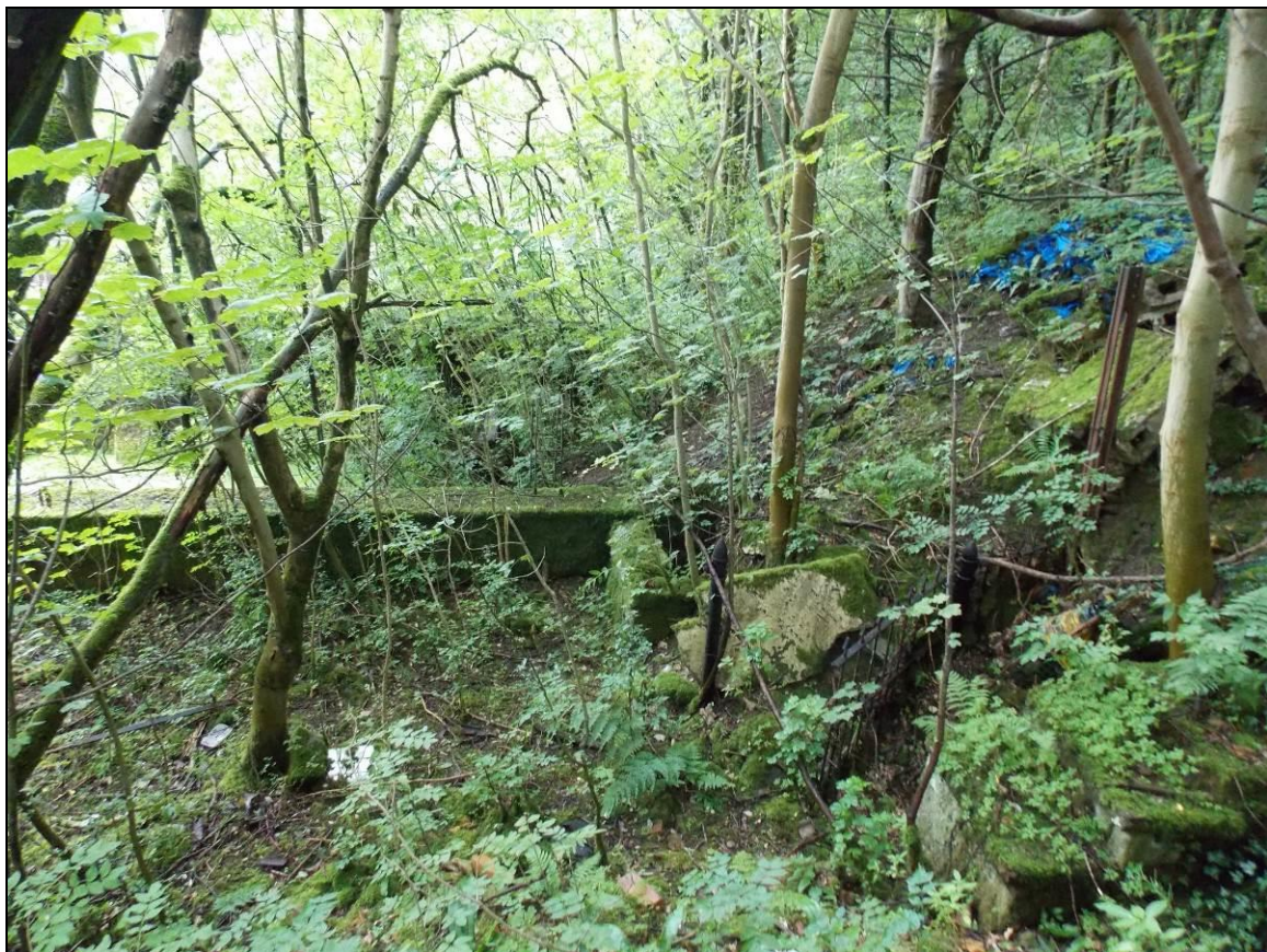
Plate 62: Settling tanks and iron railings, looking north-east.
