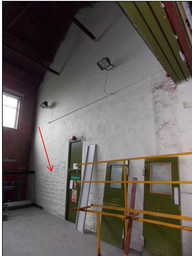
Plate 47: South-east wall with remnants of earlier stonework (arrow), looking west.
