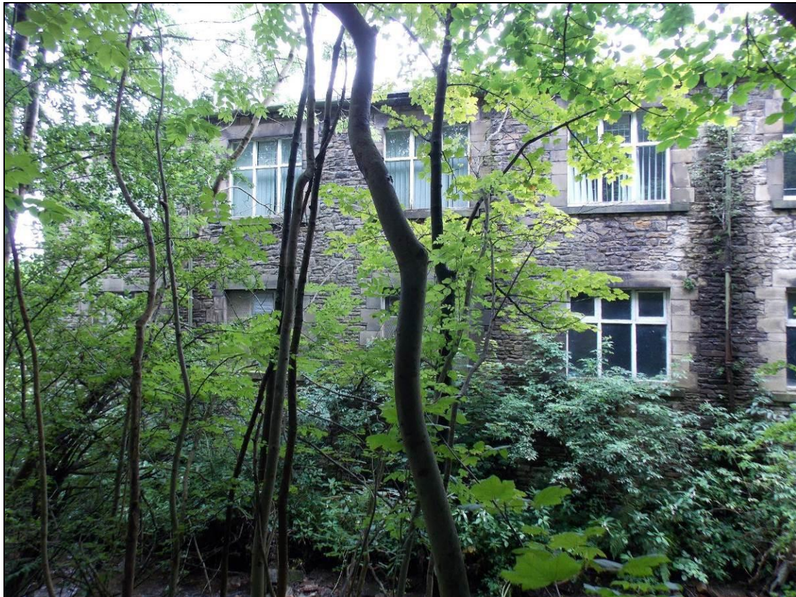
Plate 34: Rear elevation of Building 7 along Dearden Brook, looking north-west.
