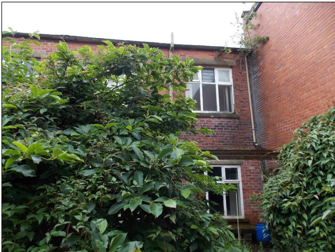
Plate 52: South-west elevation of Building 13, viewed from the courtyard.
