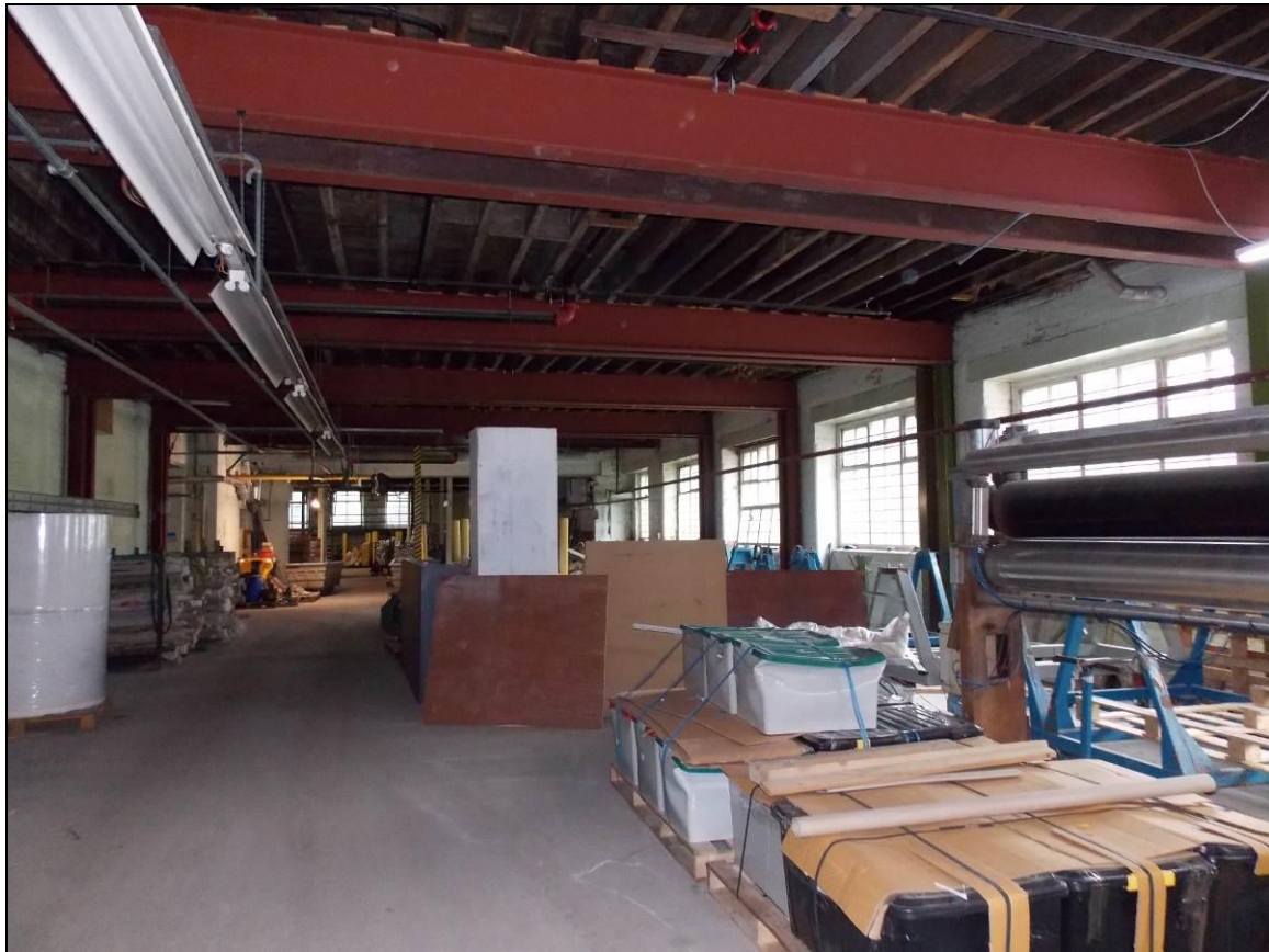
Plate 15: Internal view of Building 2A, looking north-west.
