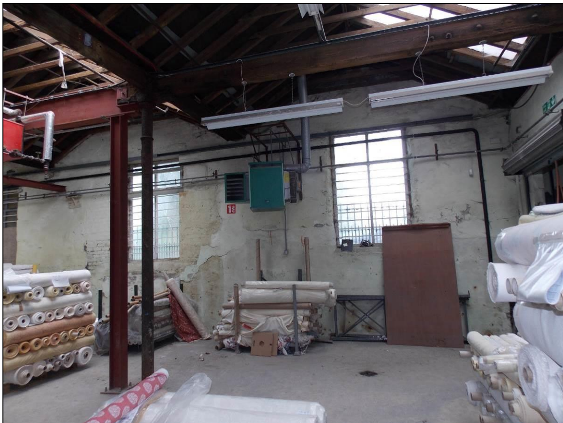
Plate 22: Window openings along Bolton Road North, looking north-west.
