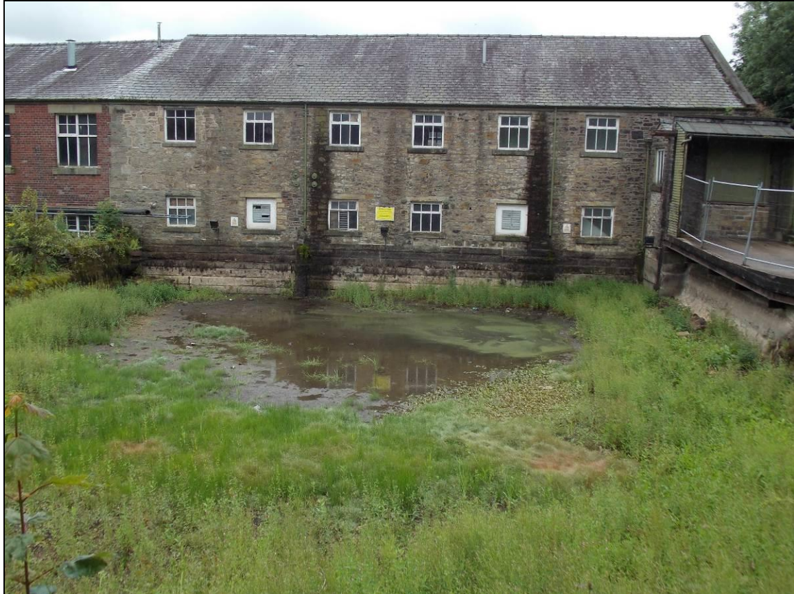
Plate 7: North-east elevation of Building 2 and adjacent reservoir, looking south-west.
