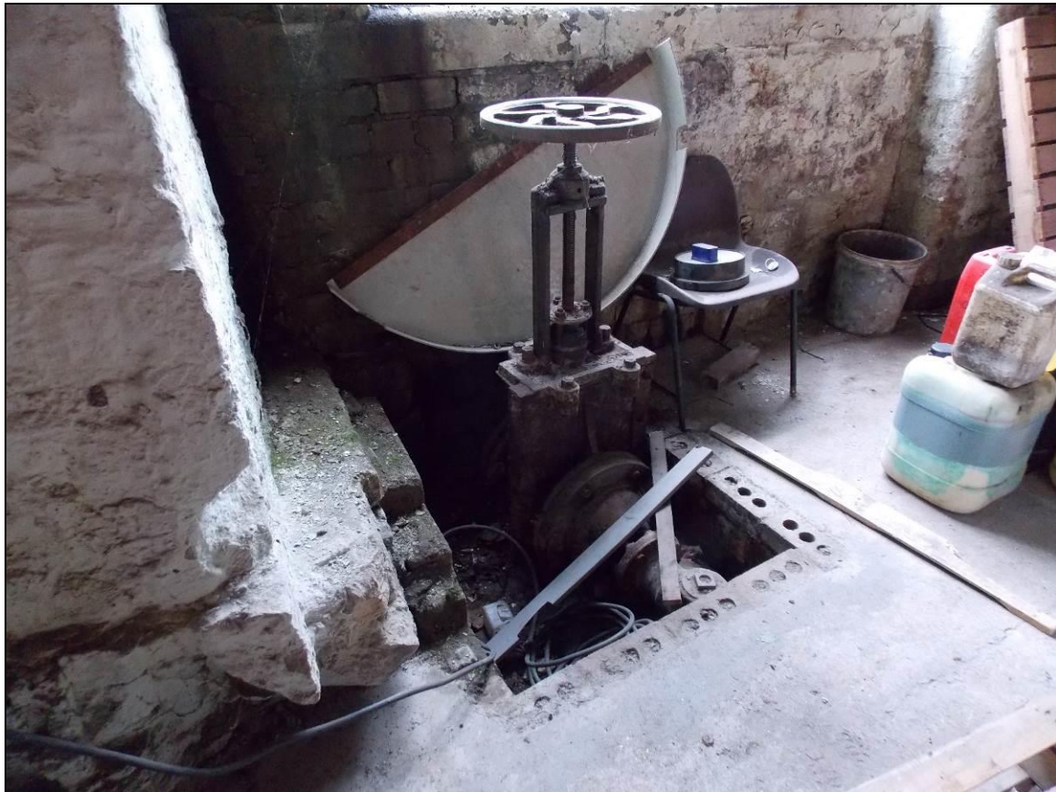
Plate 17: Sluice gate adjacent to Building 2, looking north-east.
