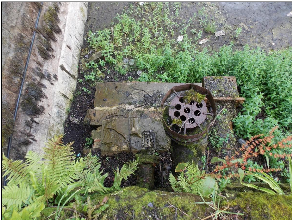
Plate 60: Detail of iron pipes with filters, looking north-east.
