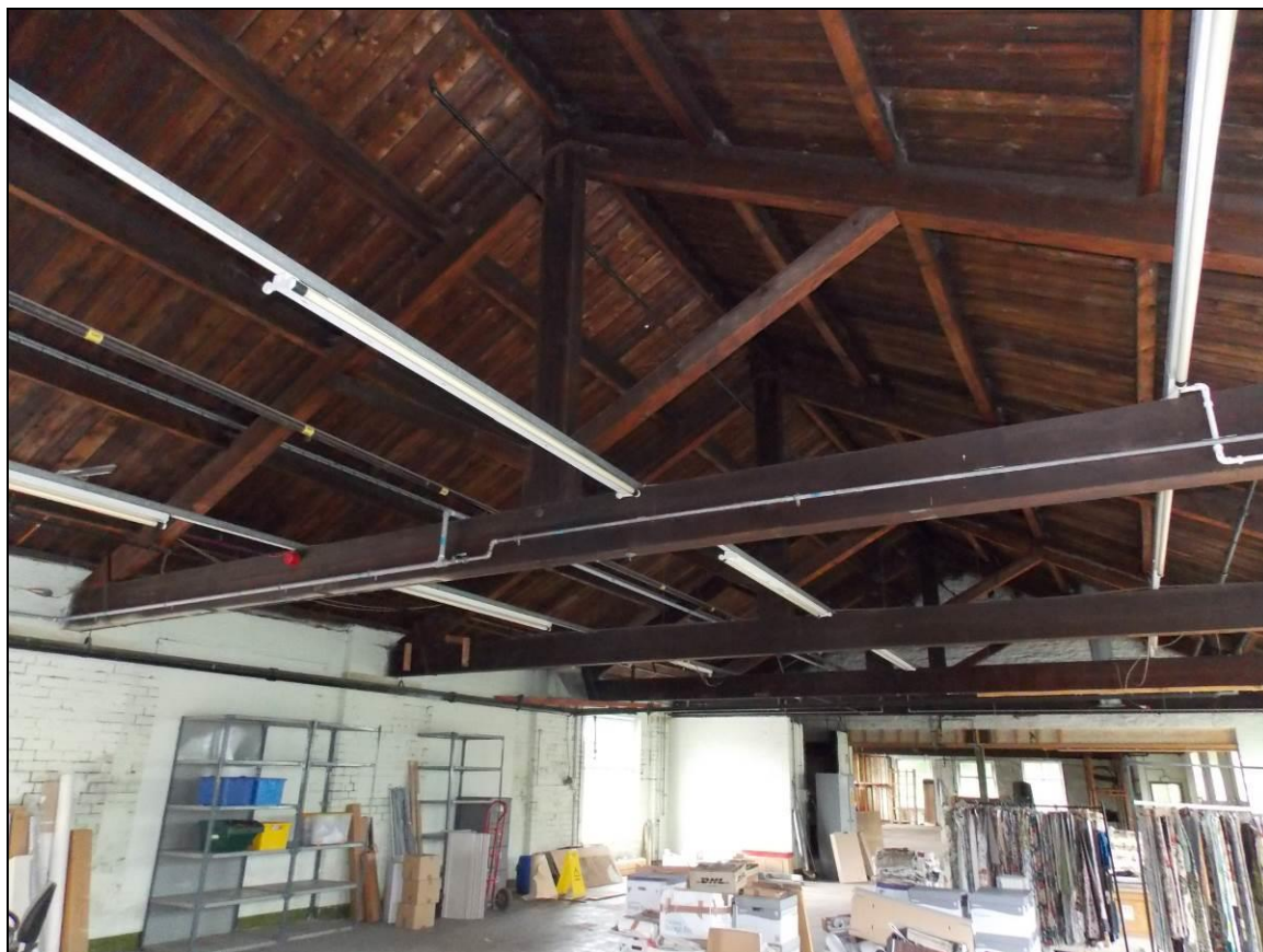
Plate 19: Roof structure of Building 2A, looking north-west.
