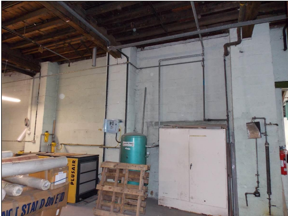
Plate 11: Concrete block pilasters encasing cast-iron columns, looking south-west.
