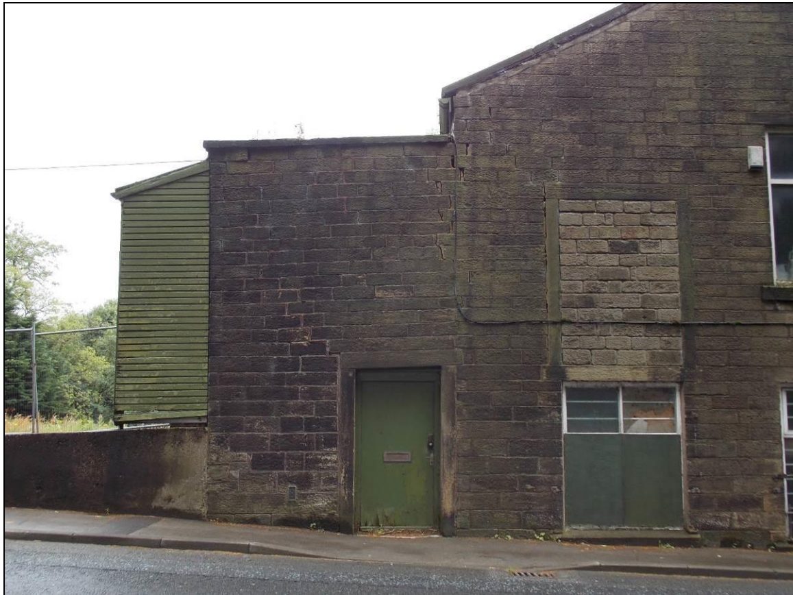
Plate 4: Building 1 facing onto Bolton Road North, looking south-east.
