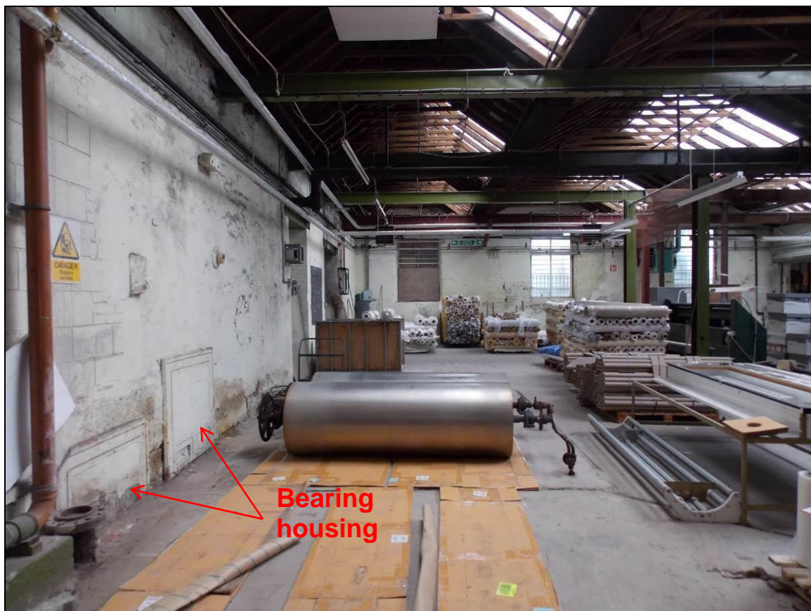
Plate 46: North-east wall with bearing housing (arrows), looking north-west.
