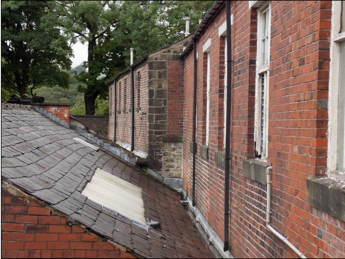
Plate 9: Brick-built south-west elevation and stone south-east gable wall, looking north-west.
