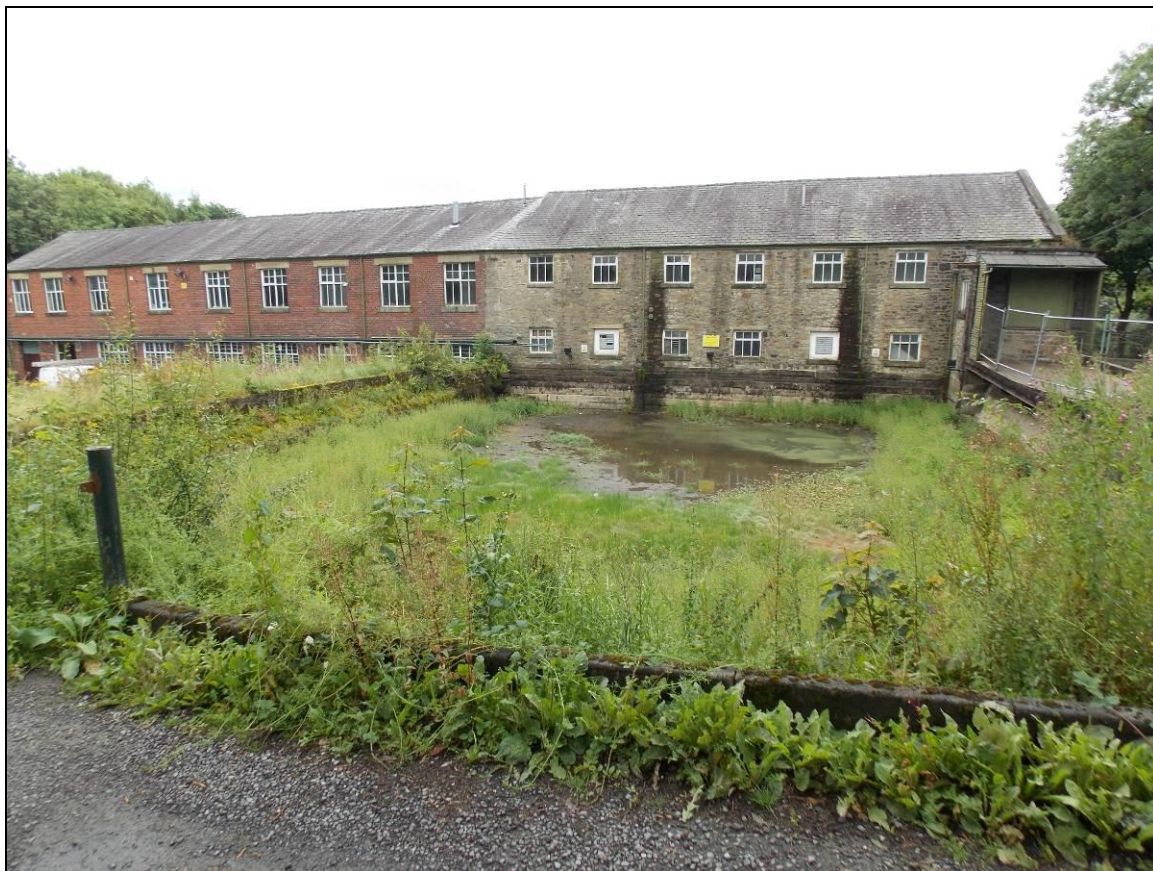
Plate 58: General view of the reservoir, looking south-west.
