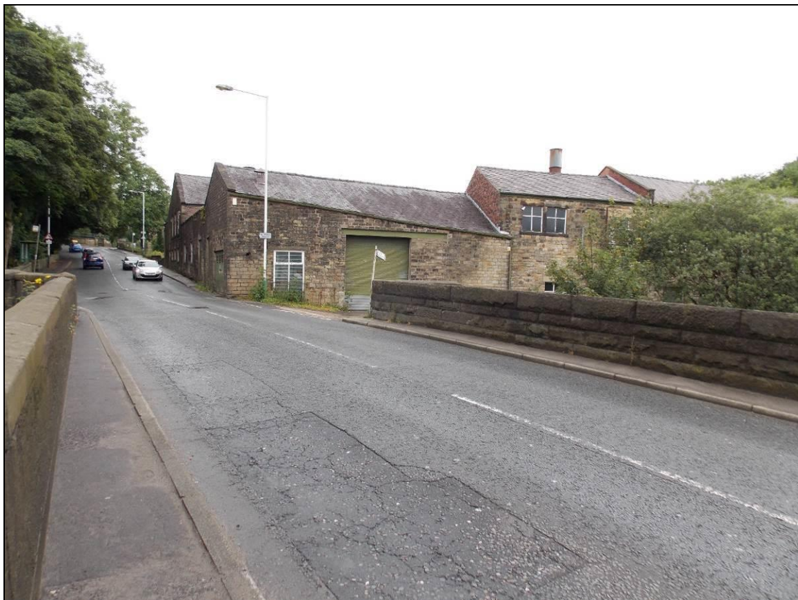
Plate 69: Croft End Mill facing onto Bolton Road North viewed from Stubbins Bridge, looking north-east.
