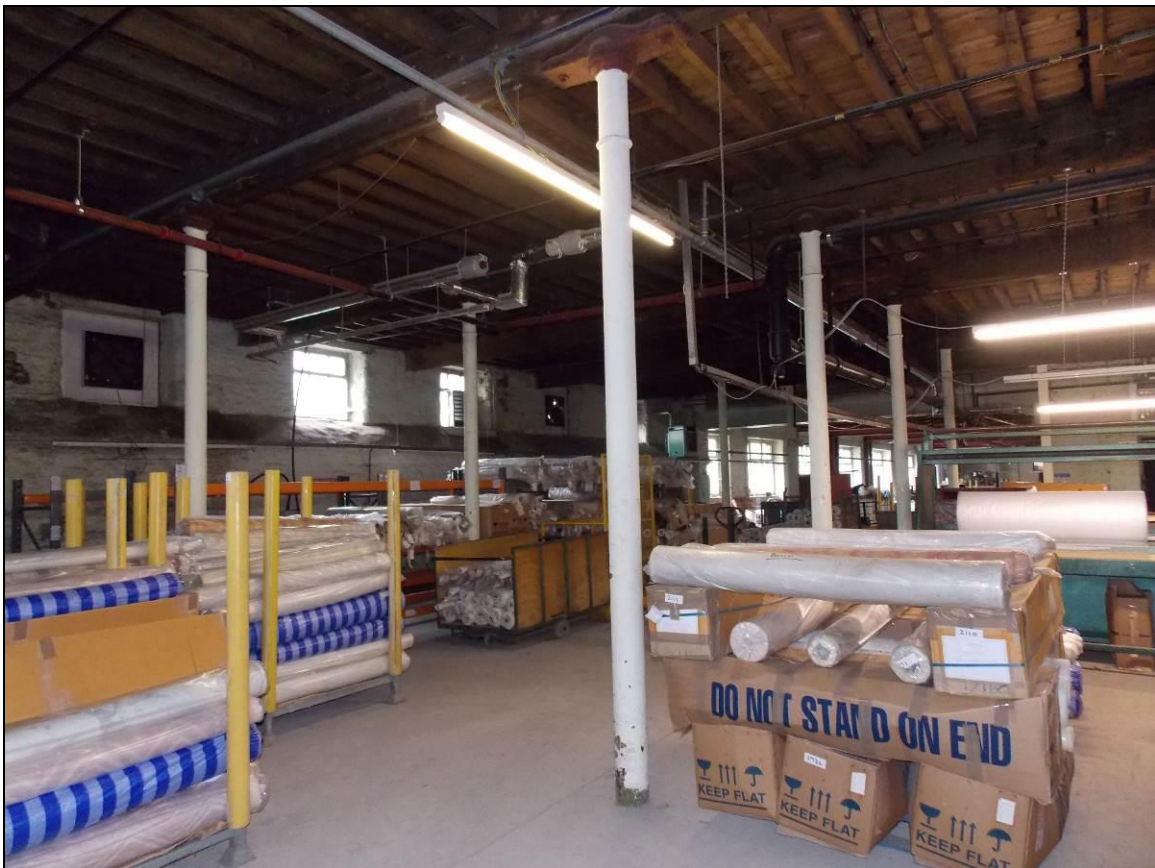
Plate 10: Internal view of the ground floor of Building 2, looking south-east.
