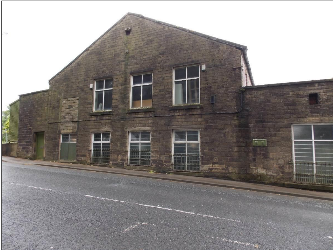
Plate 6: Gable front façade of Building 2 along Bolton Road North, looking south-west.
