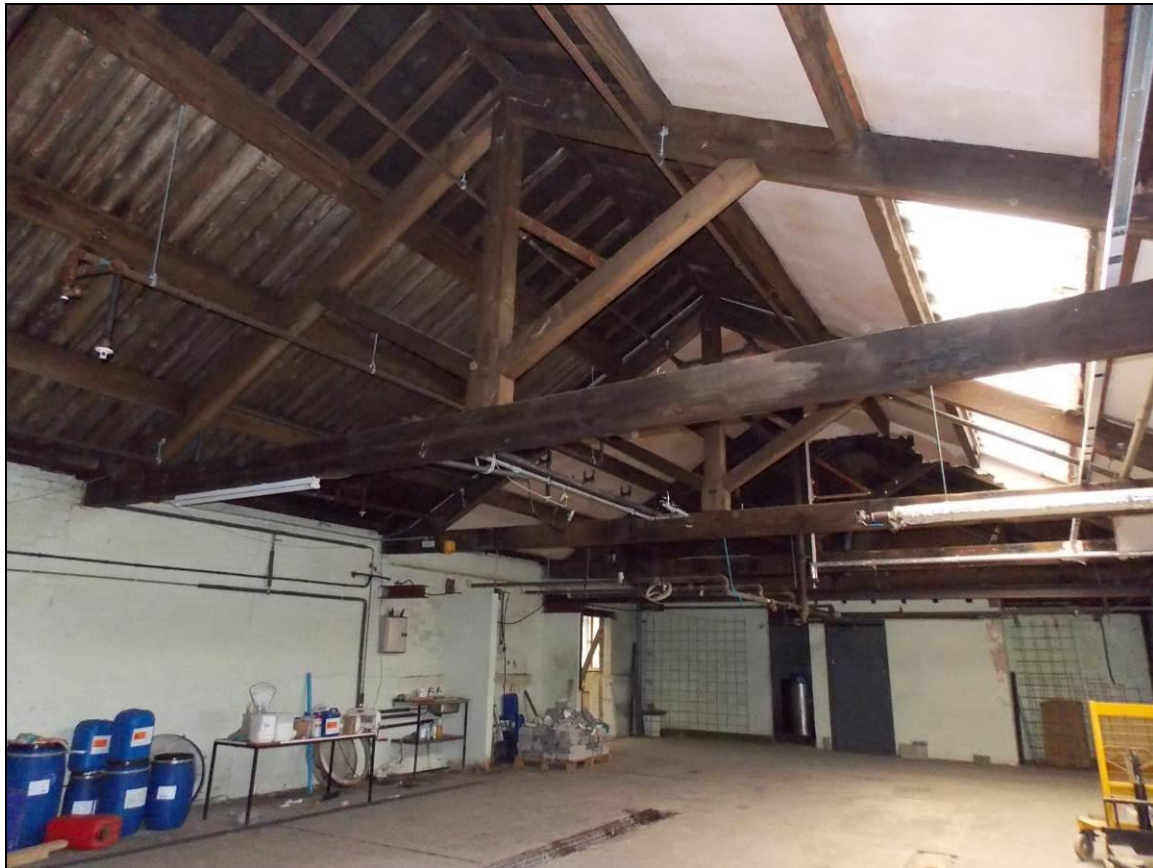
Plate 27: Roof structure of Building 4A, looking north-west.
