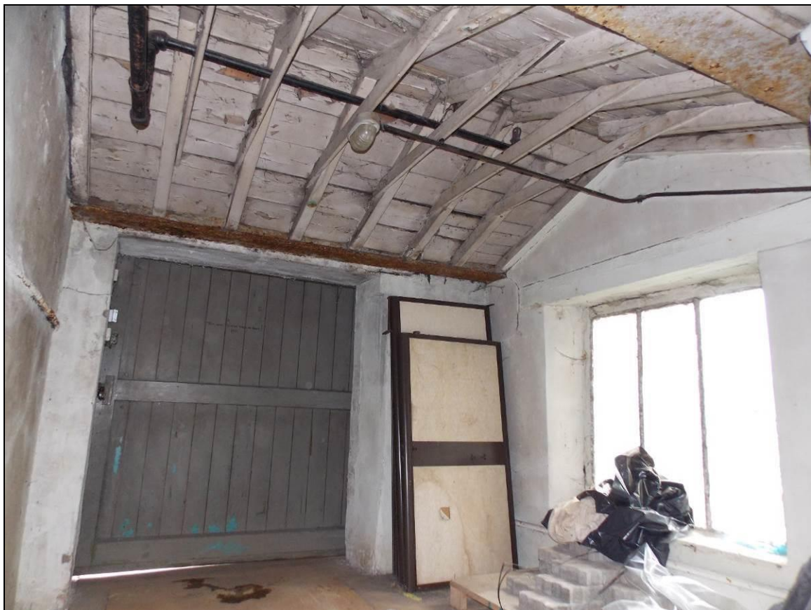
Plate 5: Internal view of Building 1, looking north-east.
