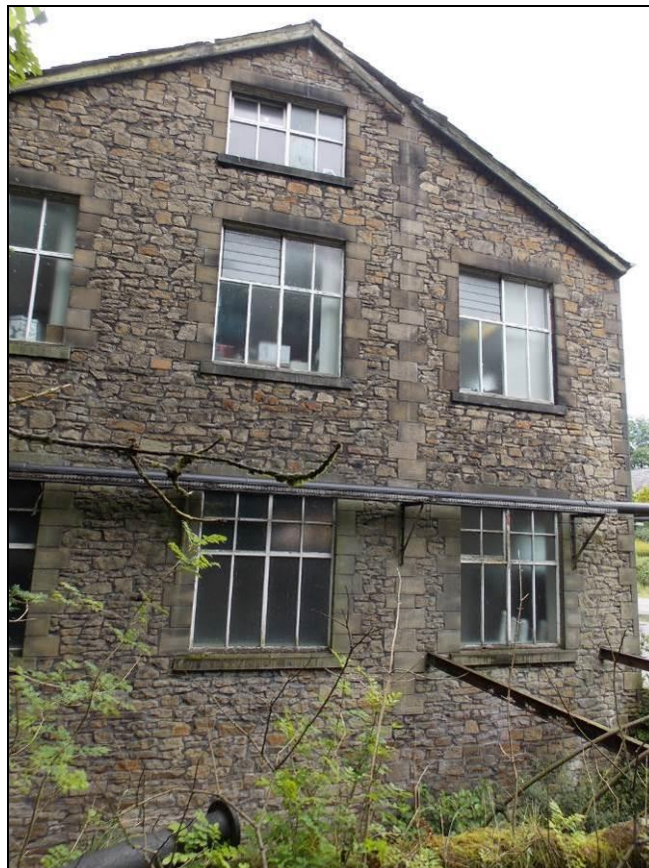
Plate 55: Gable elevation of Building 13 facing onto Dearden Brook, looking north-west.
