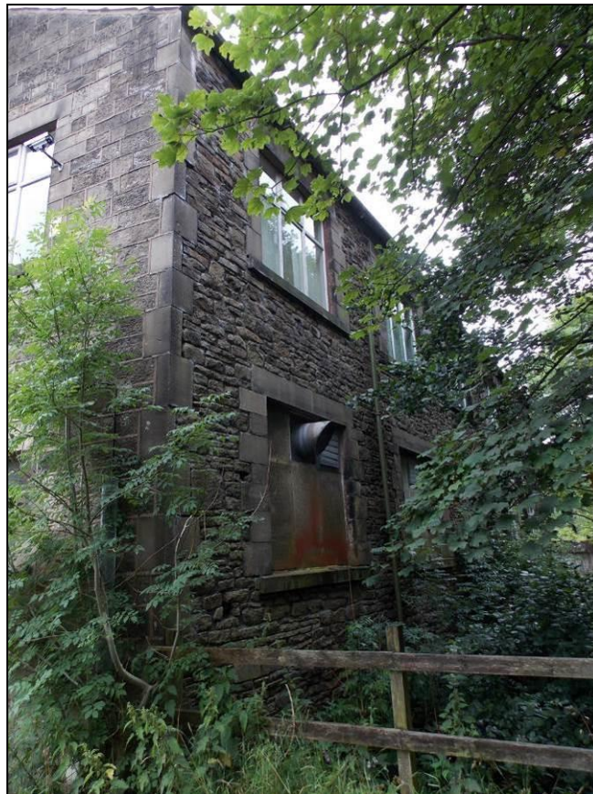
Plate 33: south-west corner of Building 7, looking north-east.
