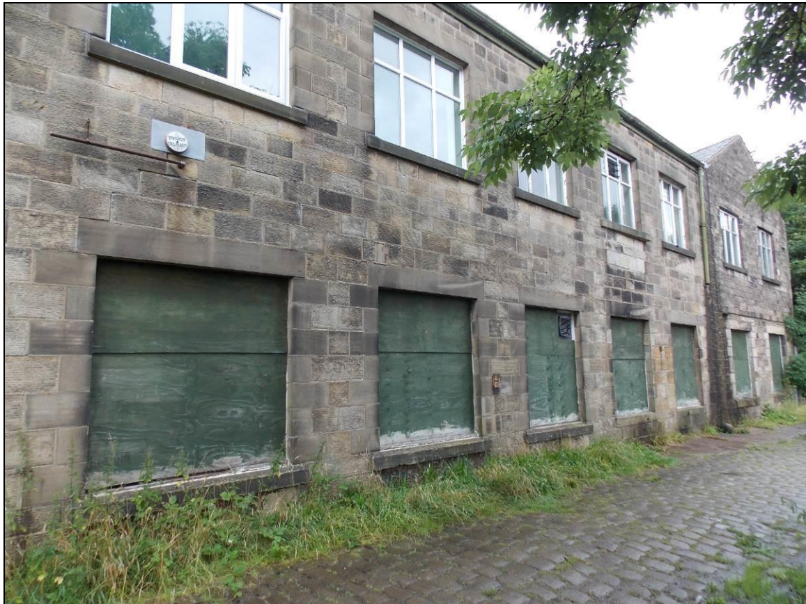
Plate 39: Detail of the front south-west elevation, looking north-east.
