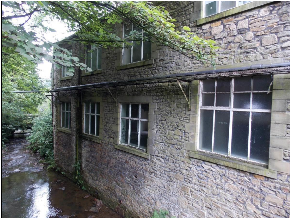
Plate 51: Building 12 facing onto Dearden Brook, looking south-west.
