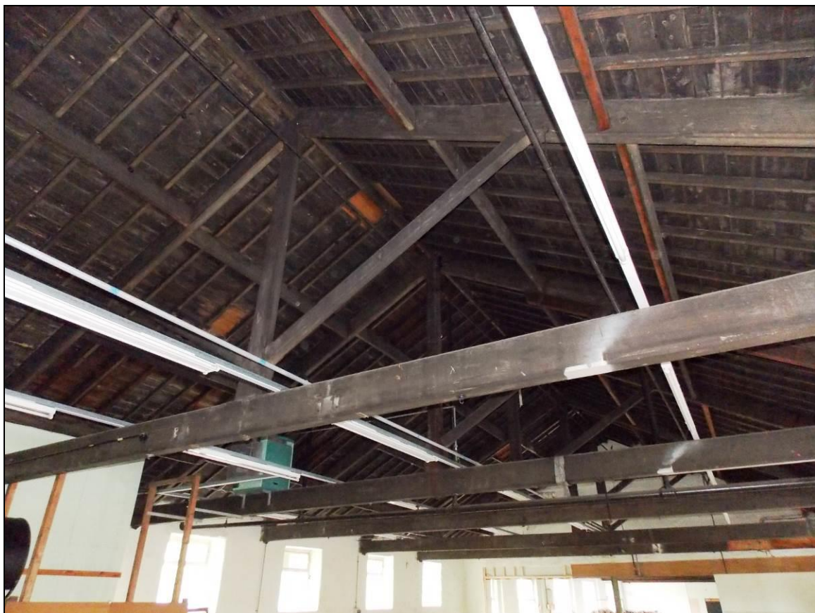
Plate 12: First floor of Building 2 with king-post trusses, looking north-west.
