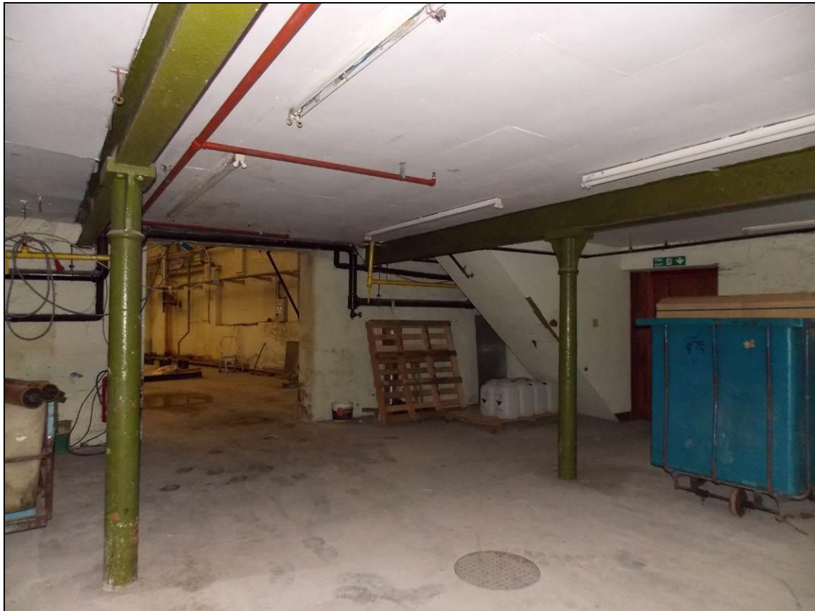
Plate 36: Cast-iron columns within the ground floor of Building 7, looking north-west.
