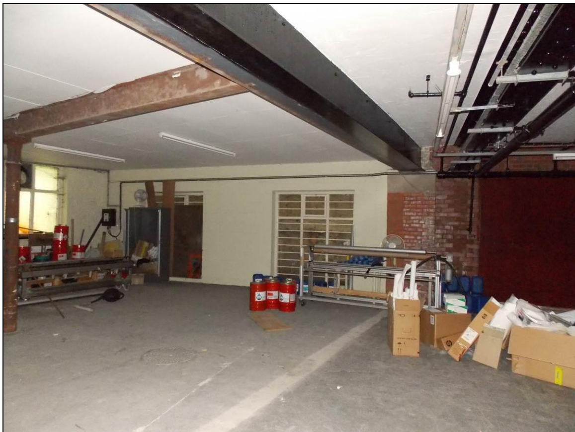
Plate 35: Ground floor of Building 7, looking south-west.
