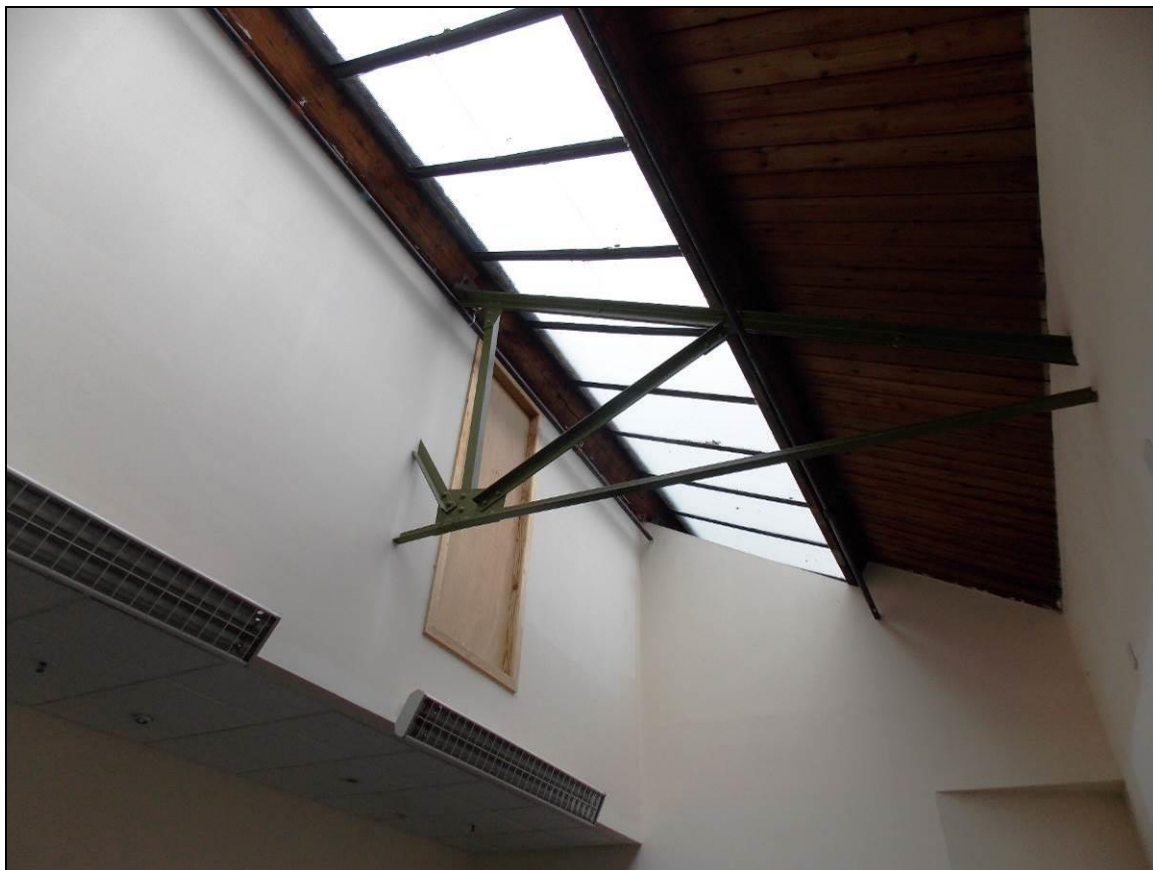
Plate 42: First floor of Building 8, looking south-east.
