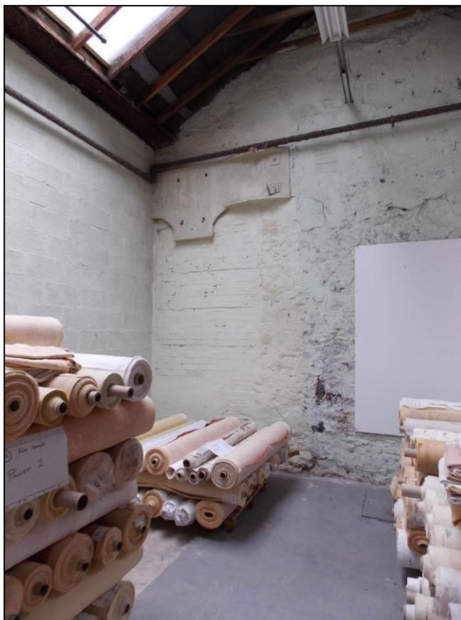
Plate 24: North-west wall with a bricked-up opening topped with a drive shaft plate, looking south-east.
