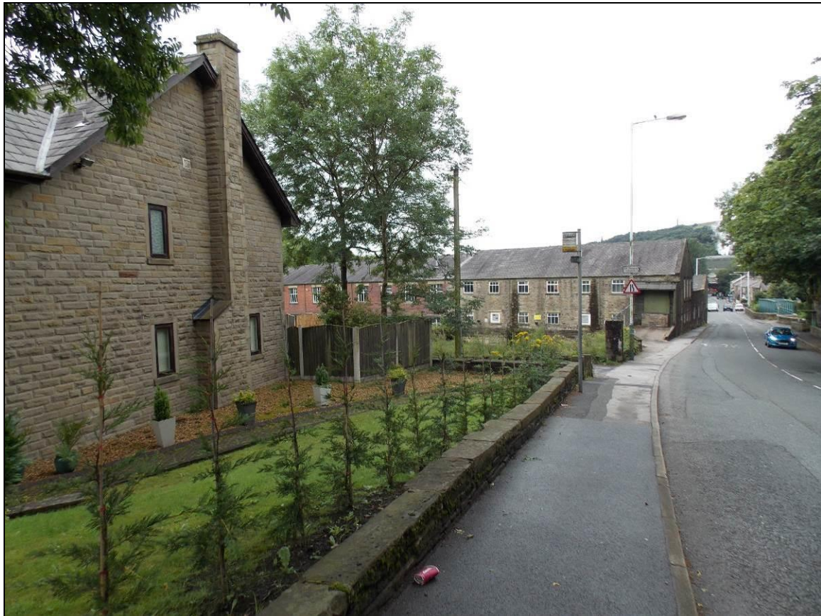
Plate 66: View of the site from the north-east along Bolton Road North.
