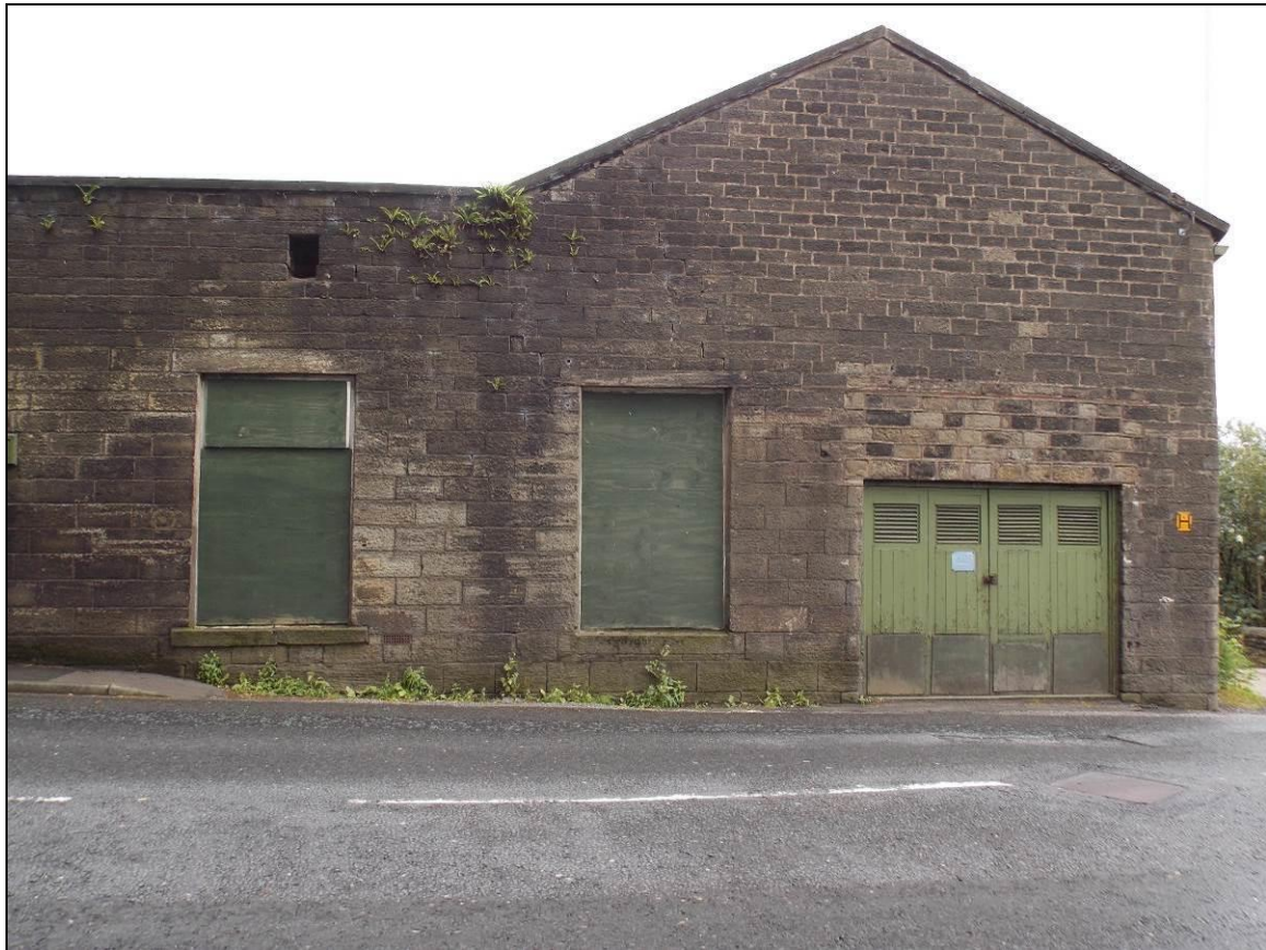
Plate 48: Front elevation of Building 11 facing onto Bolton Road North, looking south-east.
