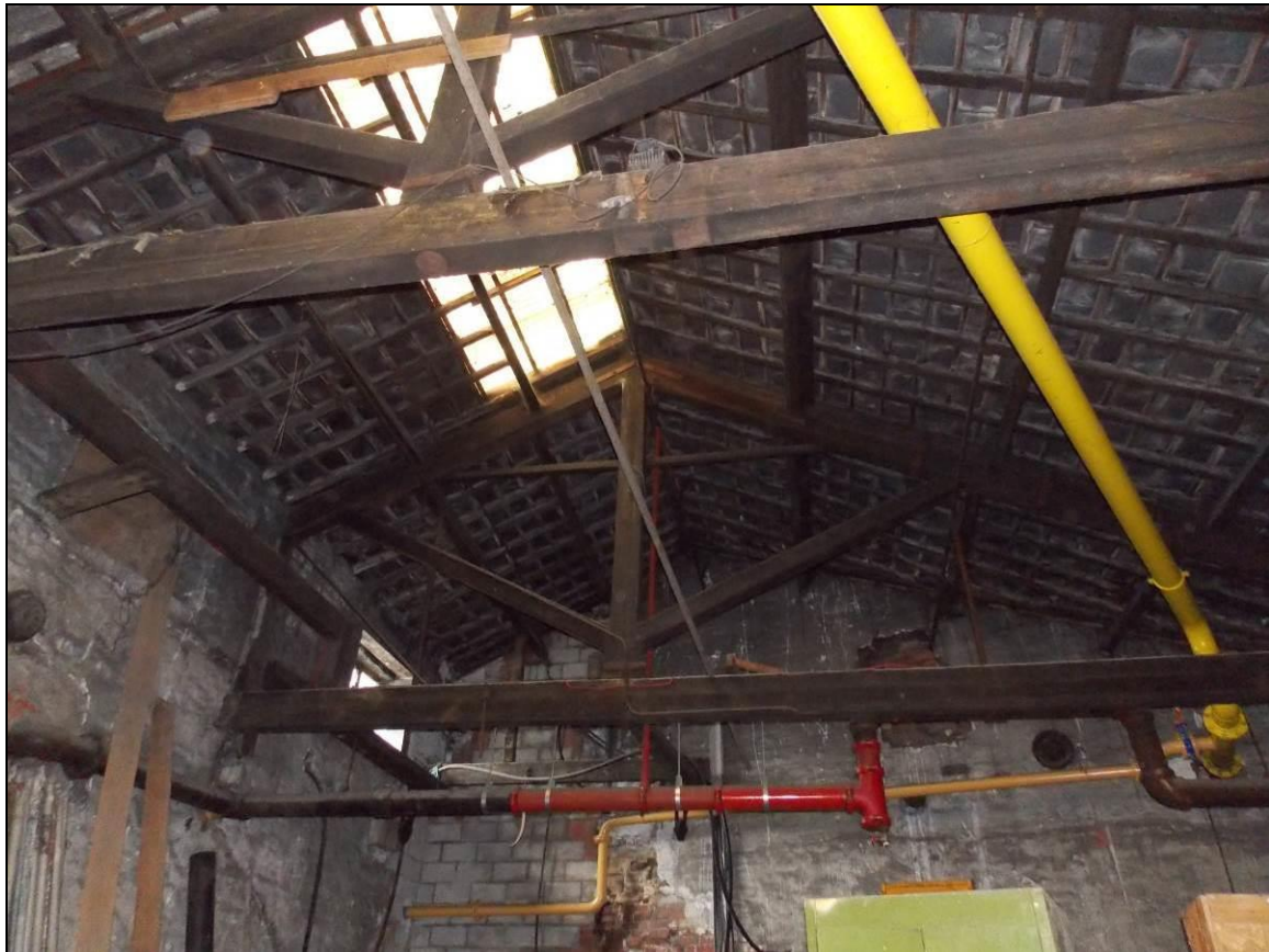
Plate 50: Internal view of Building 11, looking north-west.
