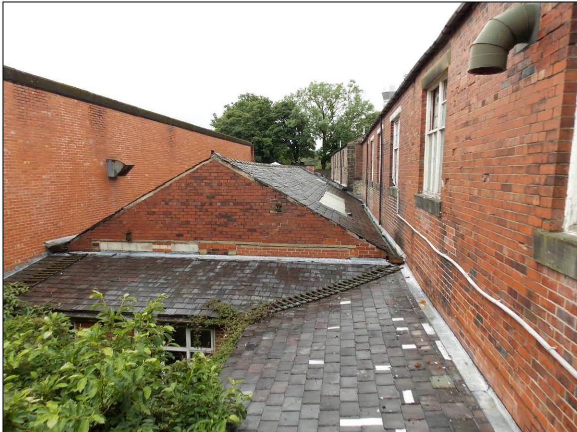
Plate 25: South-eastern gable wall of Building 4A, looking north-west.
