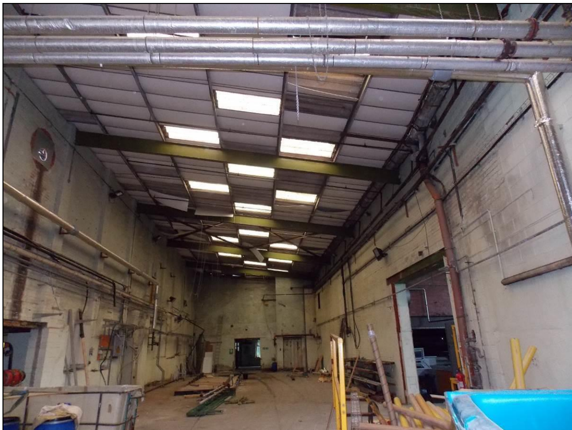
Plate 29: Internal view of Building 5, looking south-east.
