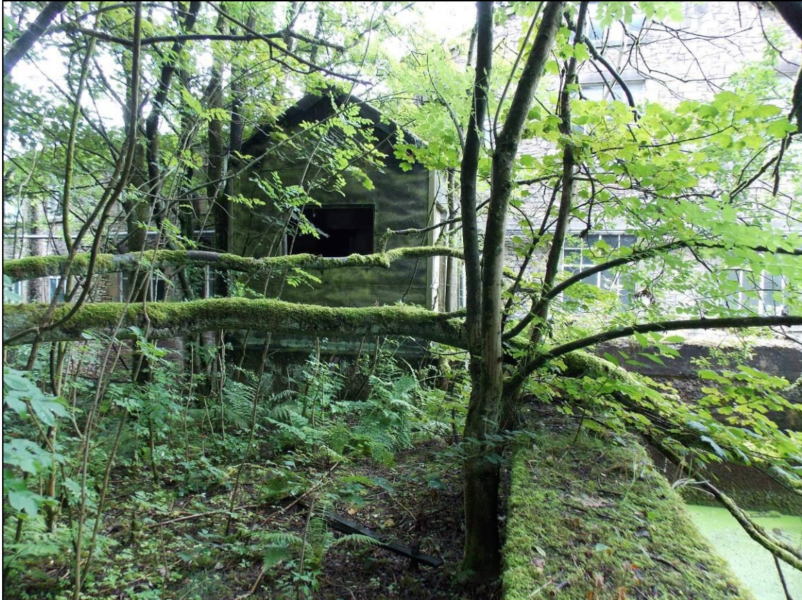
Plate 65: Detail of the shed, looking north-west.
