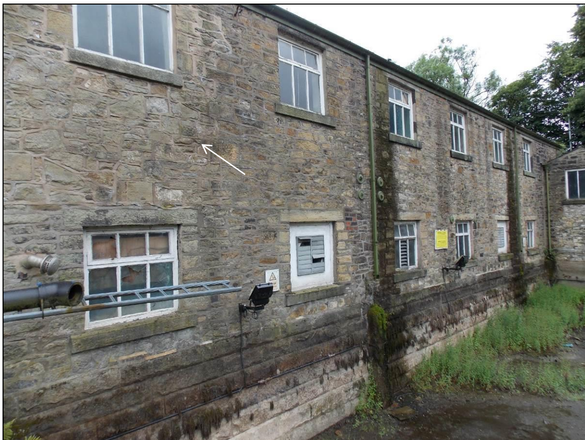
Plate 8: Repaired/rebuilt area (arrow) within the north-east elevation, looking north-east.
