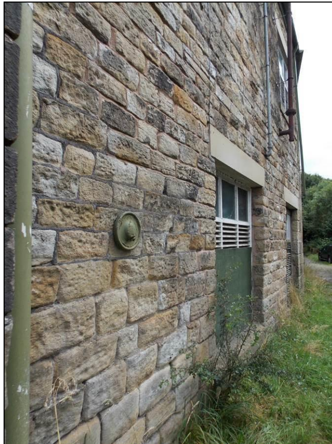
Plate 45: Detail of watershot stonework, looking south-east.
