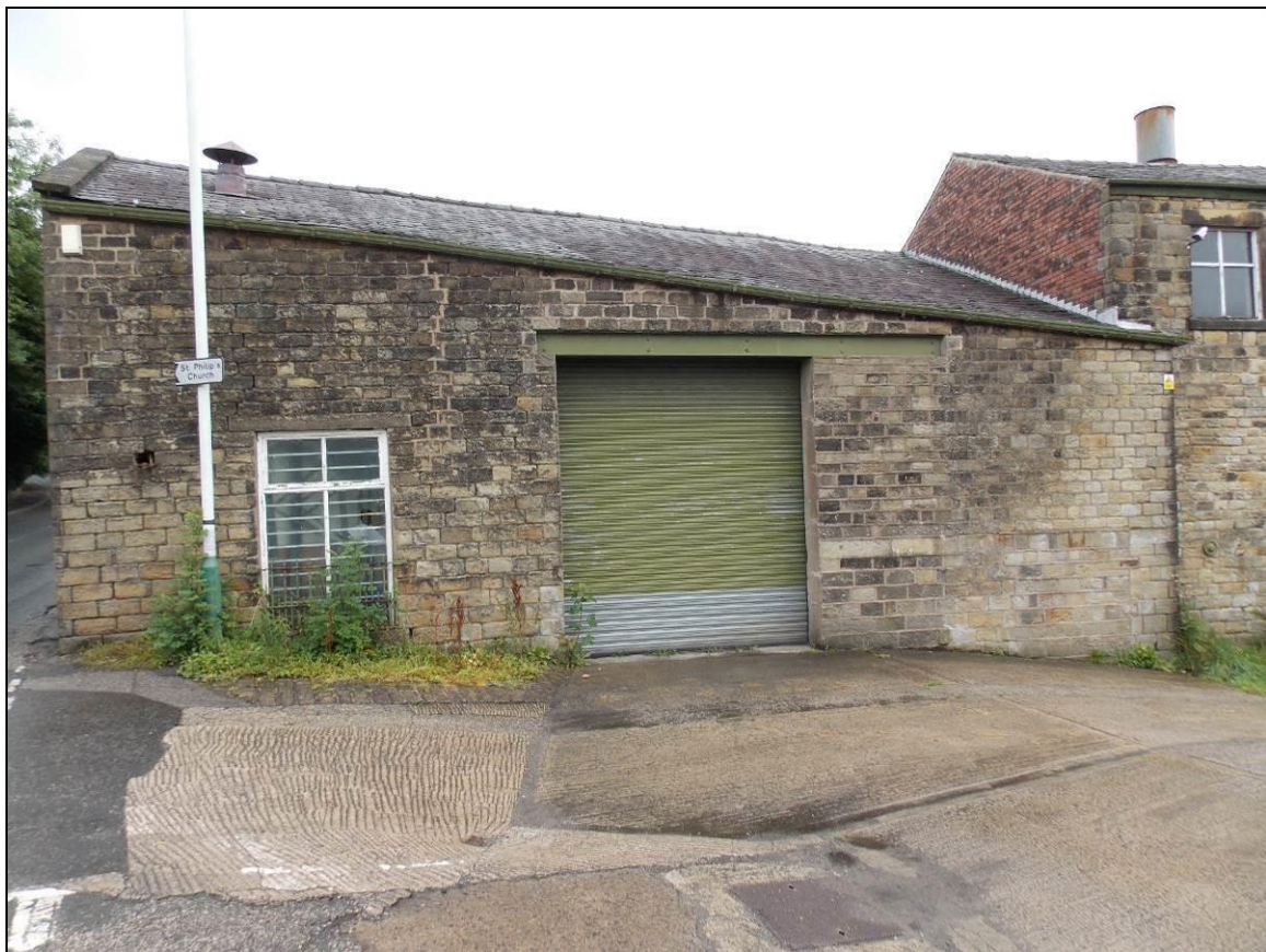
Plate 49: Side wall of Building 11 along the riverside trackway, looking north-east.
