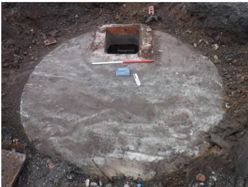
Figure 9. Modern soak away (006) (scale = 0.5m graduations).
