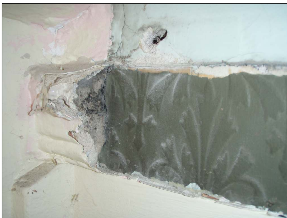
Fig. 36 Wallpaper underneath a later dado rail in Room Five
