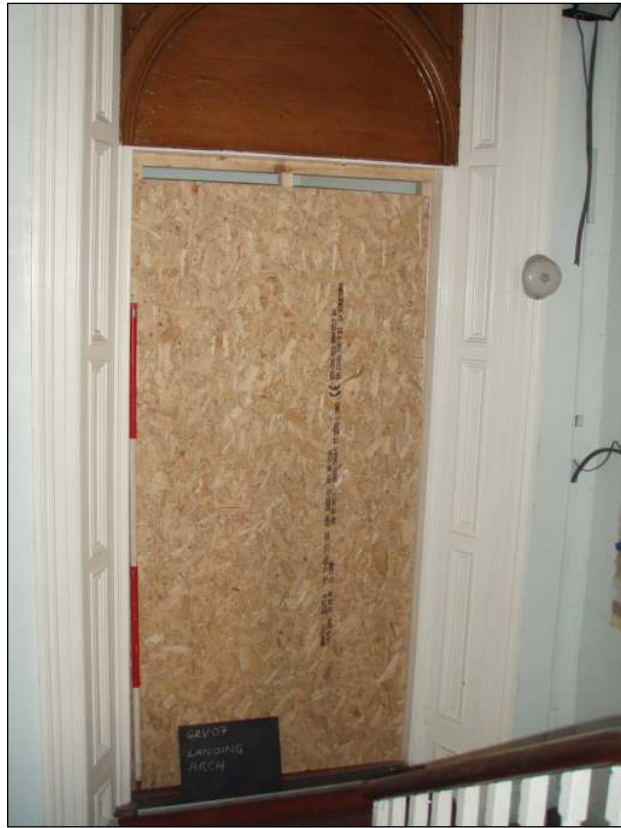
Fig. 41 Landing between Ground and First Floor, scale 2m
