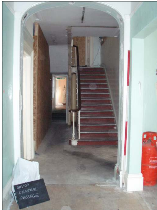
Fig. 20 Archway leading from front of passageway, scale 2m
