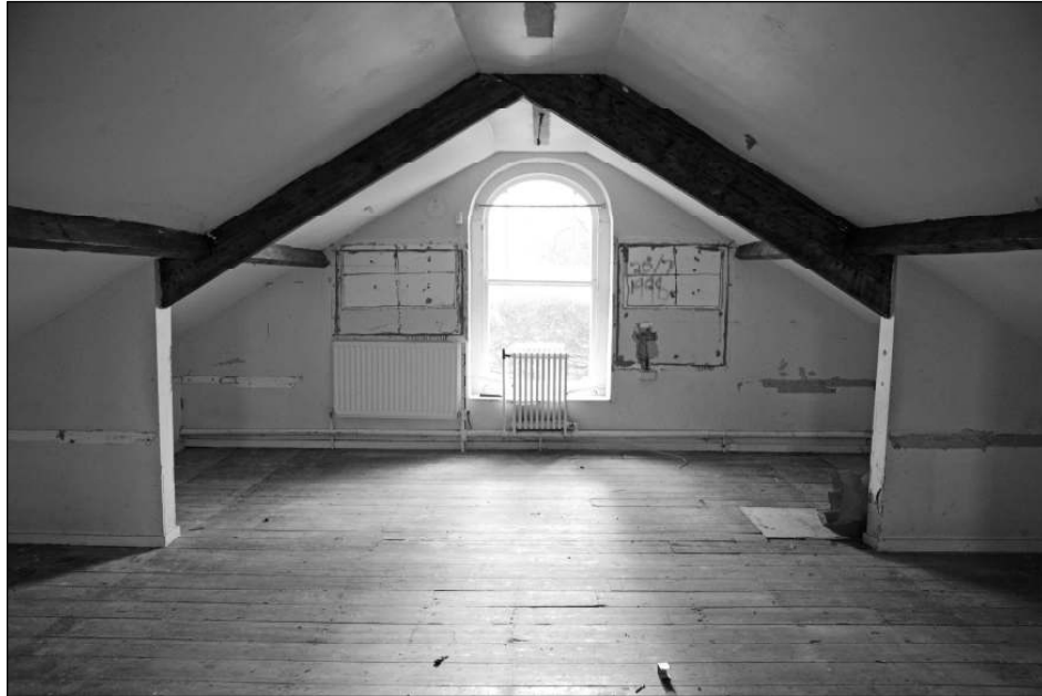
Fig. 50 Attic, south wall
