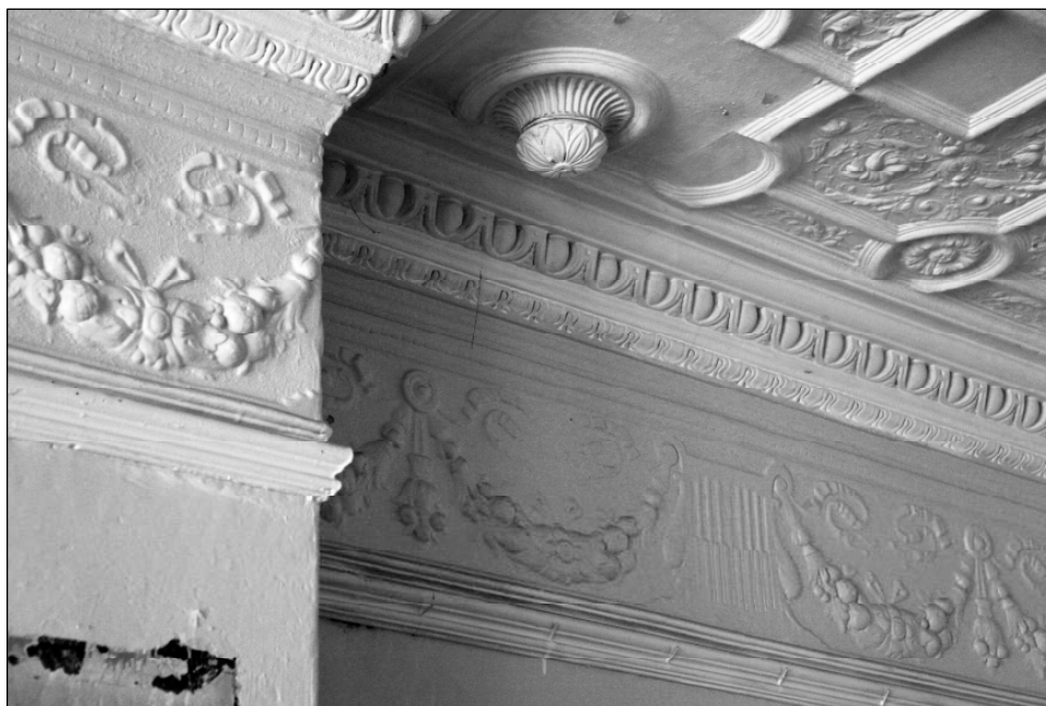
Fig. 35 Decorative cornice, border and picture rail in Room Five
