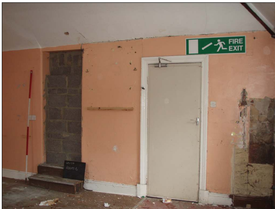
Fig. 40 Room Six, scale 2m
