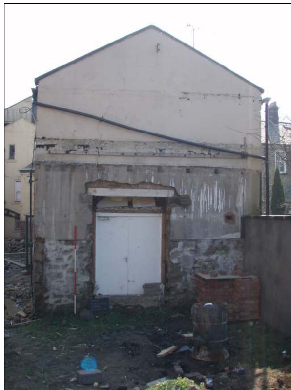
Fig. 62 The Coach House, north elevation
