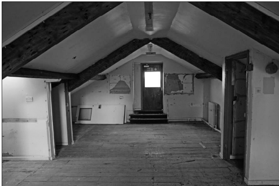
Fig. 51 Attic, north wall
