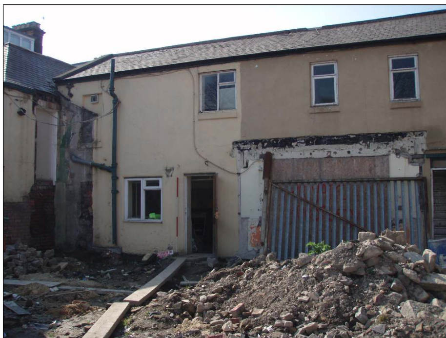
Fig. 60 The Coach House, east elevation, scale 2m
