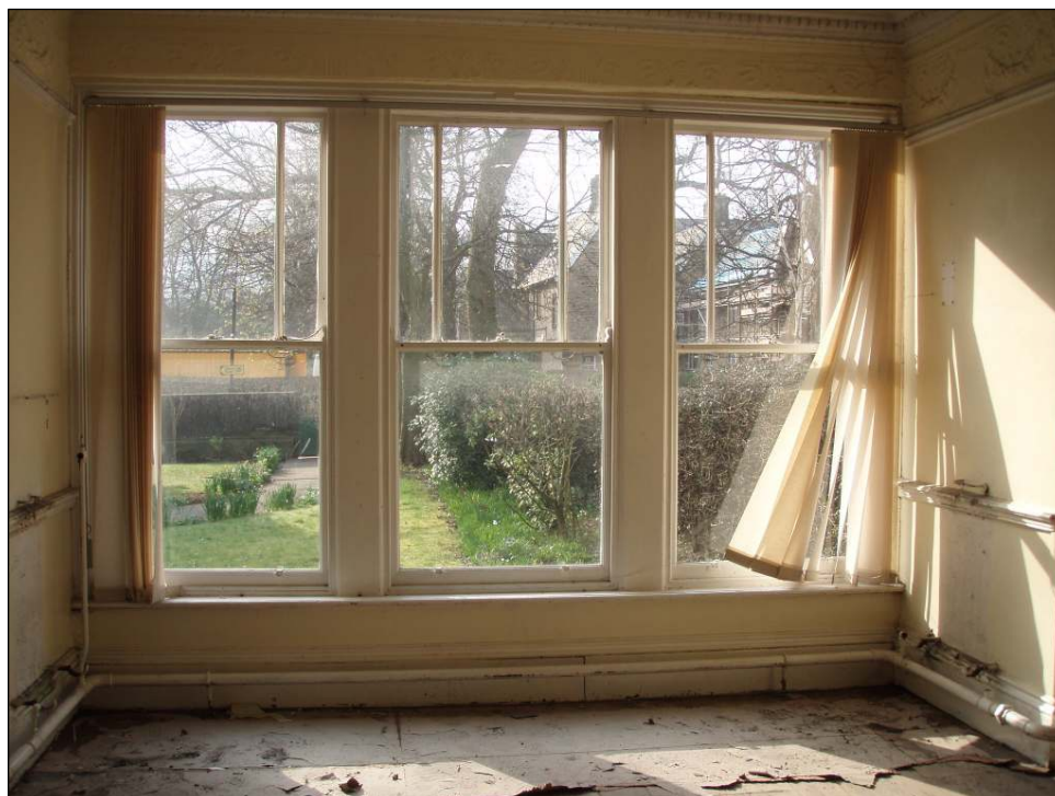
Fig. 38 Window in Room Five
