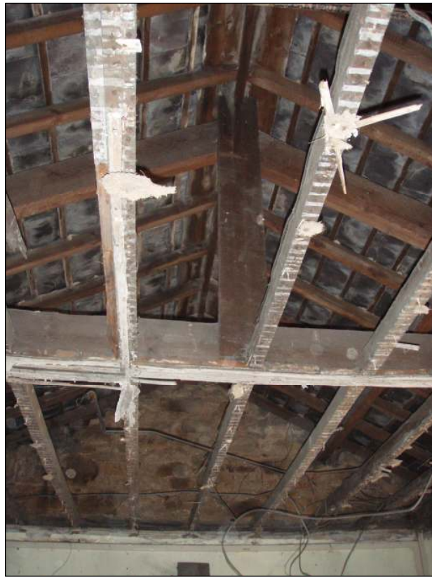
Fig. 66 Timber framed roof in Room Four of the Coach House
