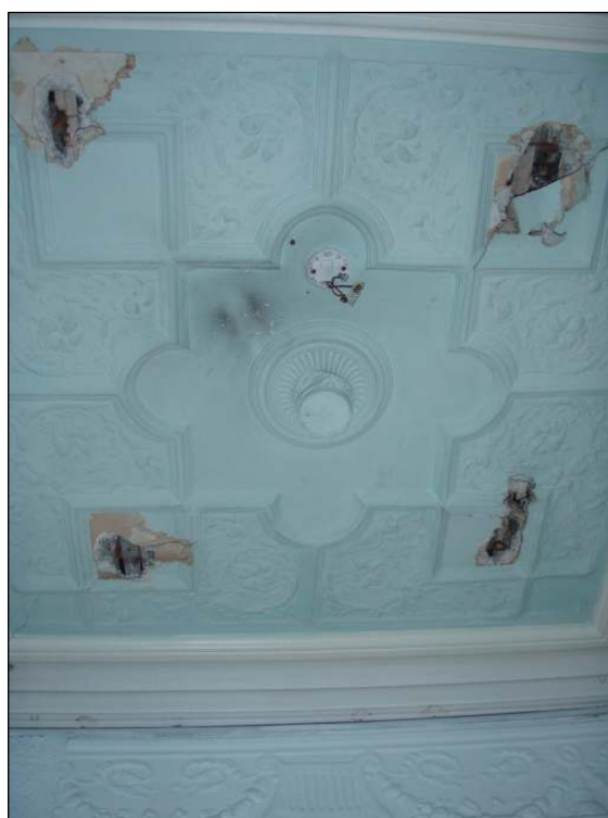
Fig. 19 Ceiling decoration in front passageway
