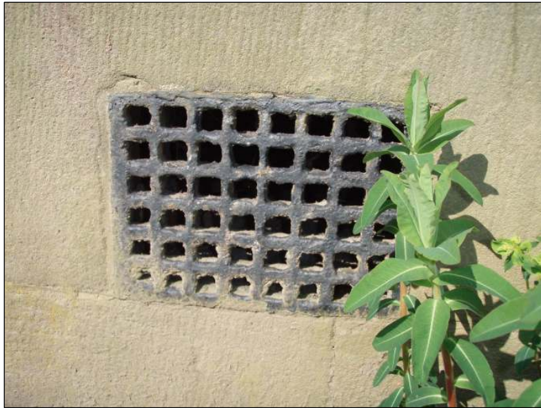
Fig. 9 Ventilation grate under west window, south elevation
