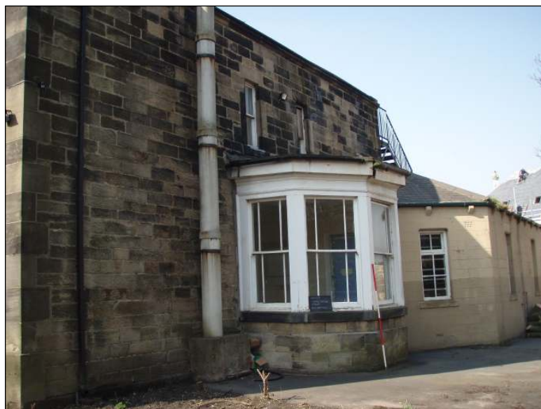
Fig. 10 East elevation, main building, scale 2m
