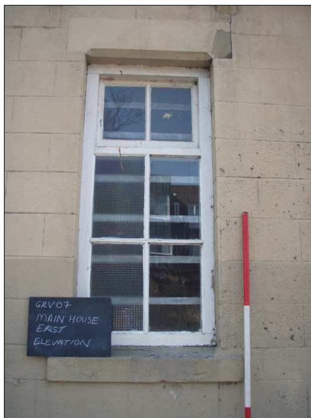
Fig. 13 East elevation, later extension window, scale 2m
