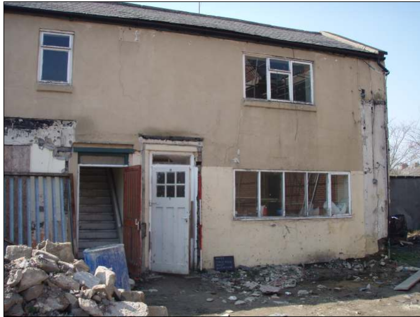
Fig. 61 The Coach House, east elevation, scale 2m
