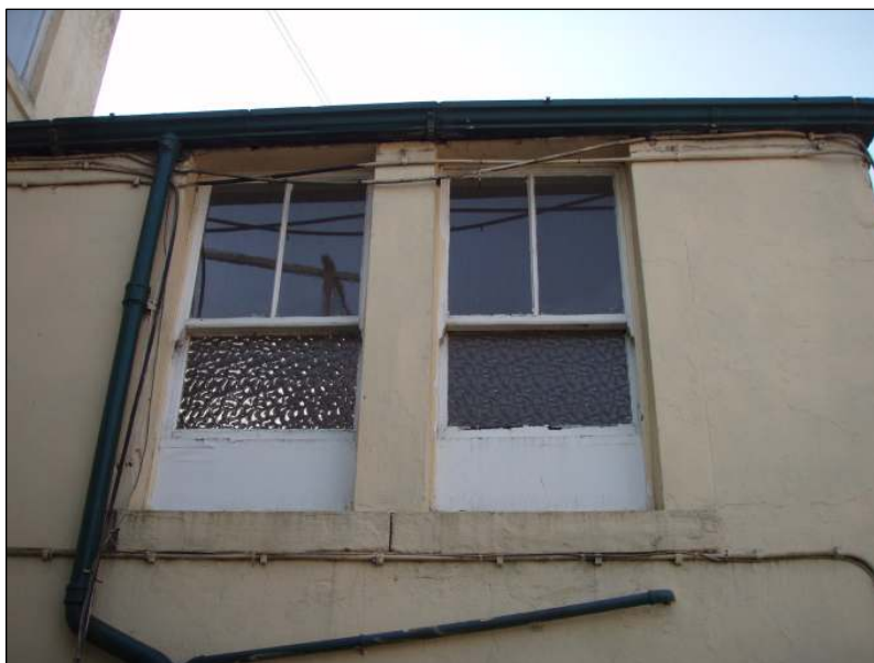
Fig. 17 Windows in east facing wall of extension in north elevation
