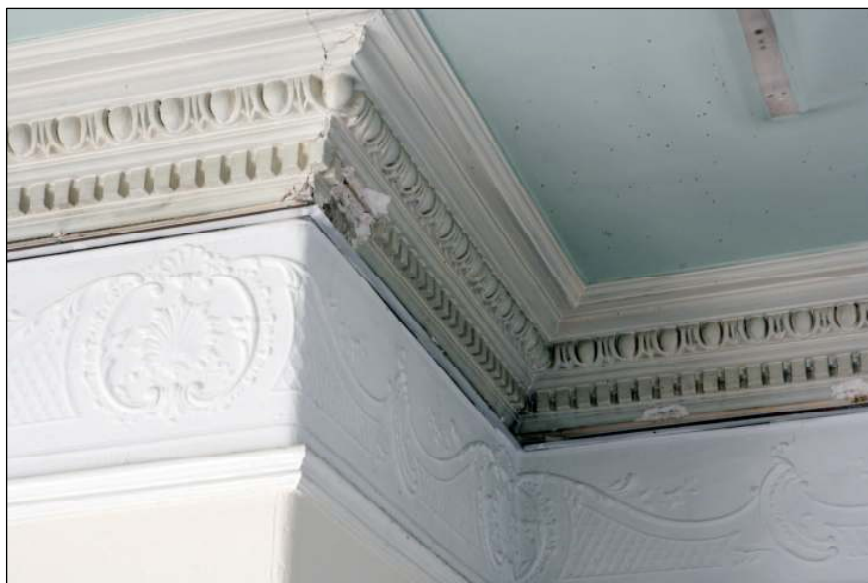
Fig. 27 Decorative cornice, patterned frieze and picture rail, Room One
