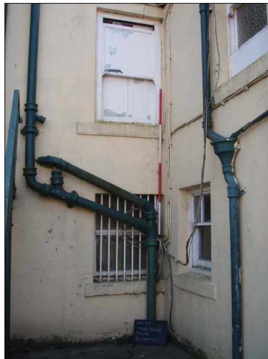
Fig. 16 North elevation, west corner, scale 2m
