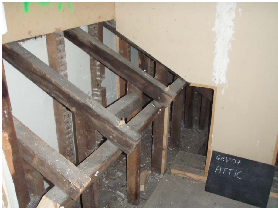
Fig. 53 Roof beams in the west side of attic
