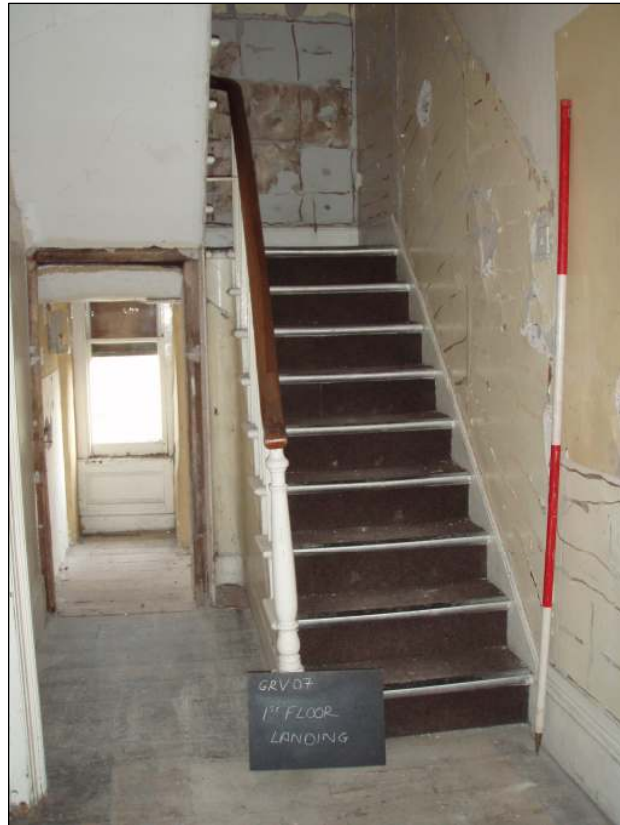
Fig. 43 First Floor landing
