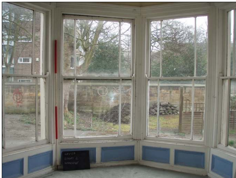
Fig. 30 Bay window in Room Two, scale 2m
