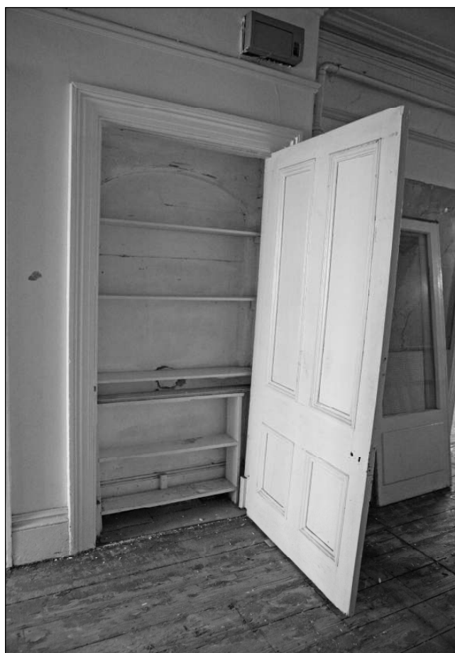
Fig. 49 Cupboard in Room Fourteen
