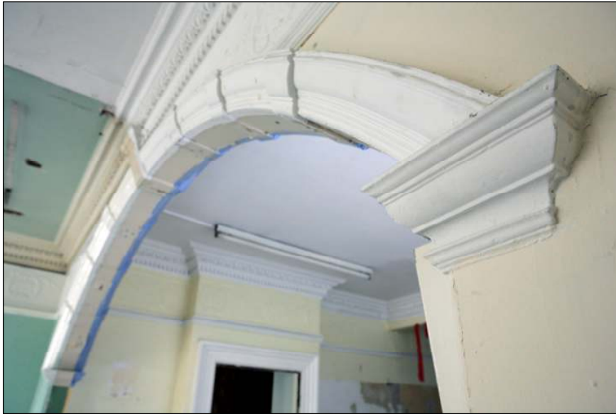
Fig. 29 Archway from Room One into Room Two
