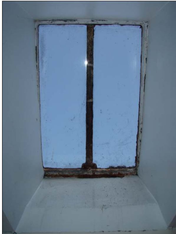
Fig. 52 Skylight in western niche of attic
