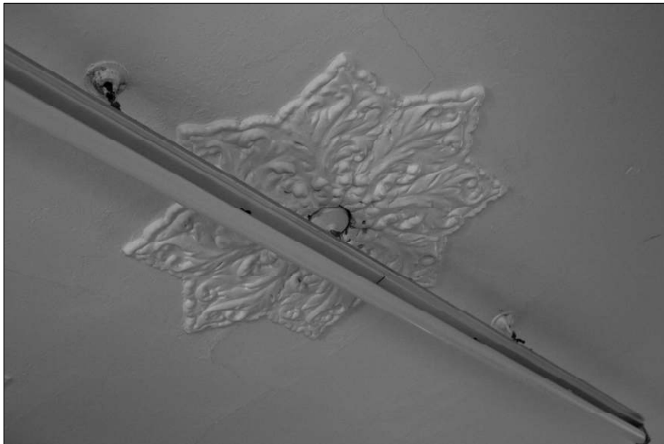
Fig. 42 Decorative ceiling rose on First Floor landing
