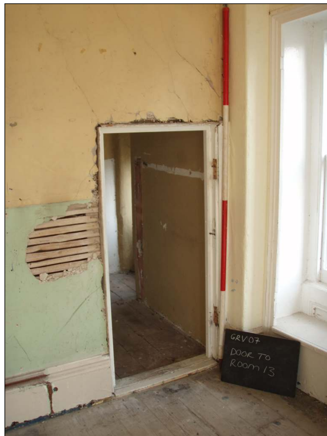
Fig. 48 Doorway leading to Room Thirteen, scale 2m
