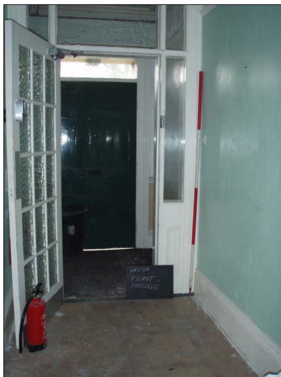
Fig. 18 Front passageway, scale 2m
