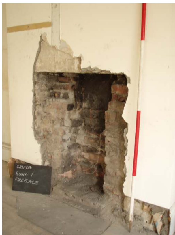
Fig. 28 Fireplace in Room One, scale 2m
