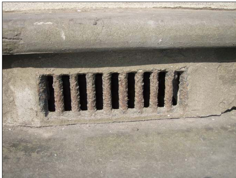
Fig. 8 Ventilation grate in doorway step, south elevation
