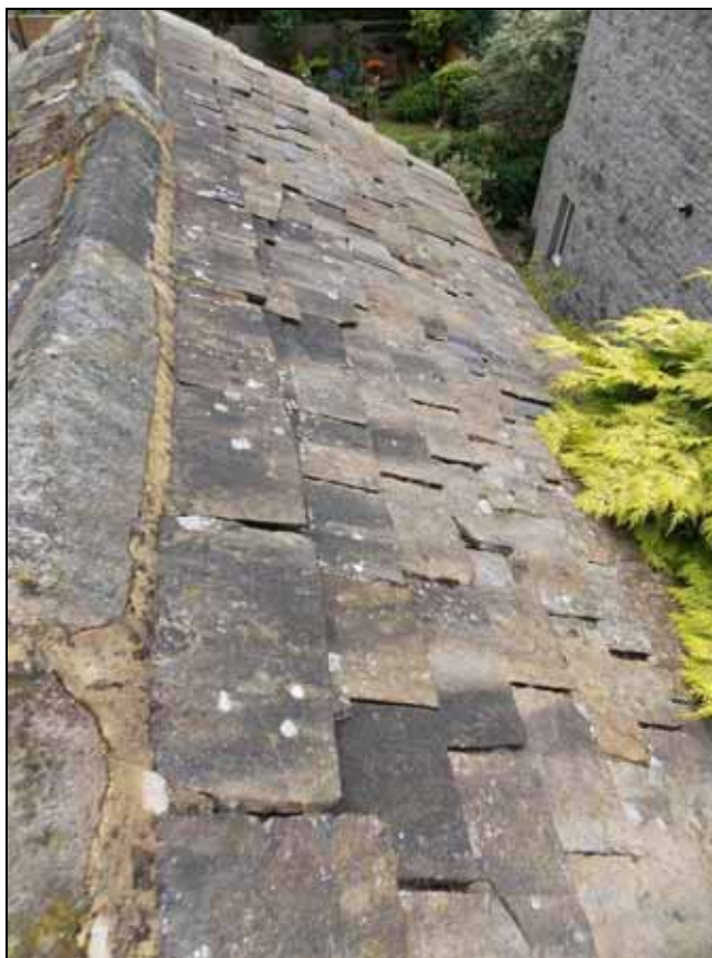
Plate 23: Southern slope of the stone roof, looking east.
