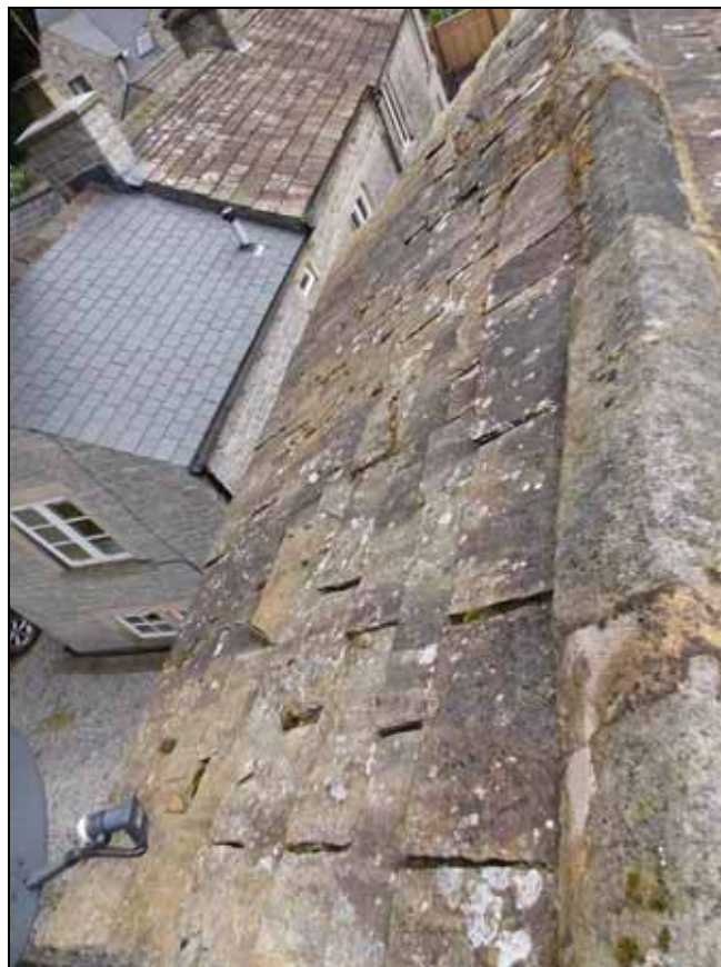
Plate 22: Northern slope of the stone roof, looking east.
