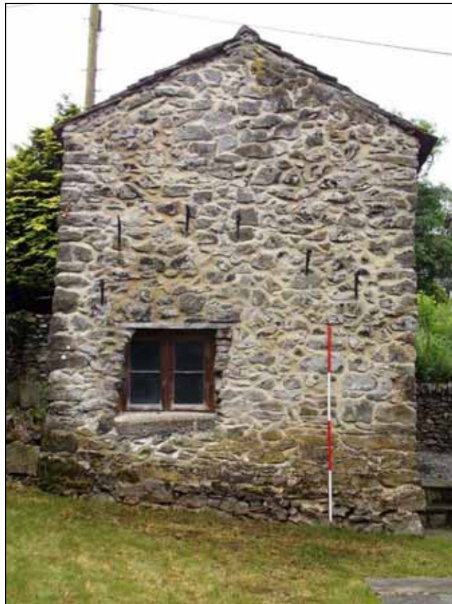
Plate 12: Detailed view of the east elevation (scale 2m).
