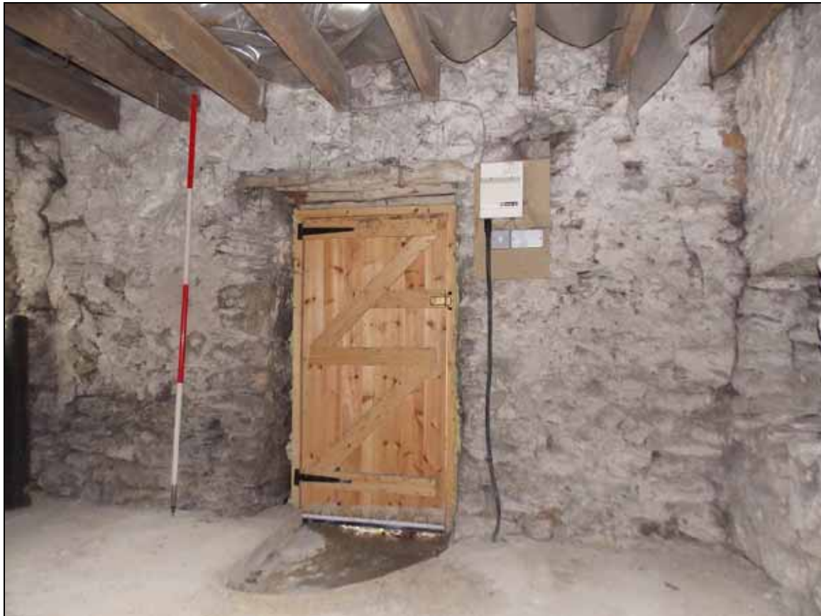
Plate 24: Doorway within the north wall (scale 2m).
