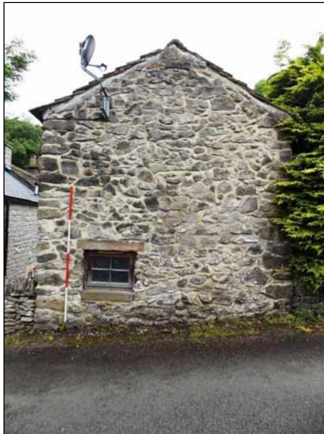
Plate 20: West elevation, looking east (scale 2m).
