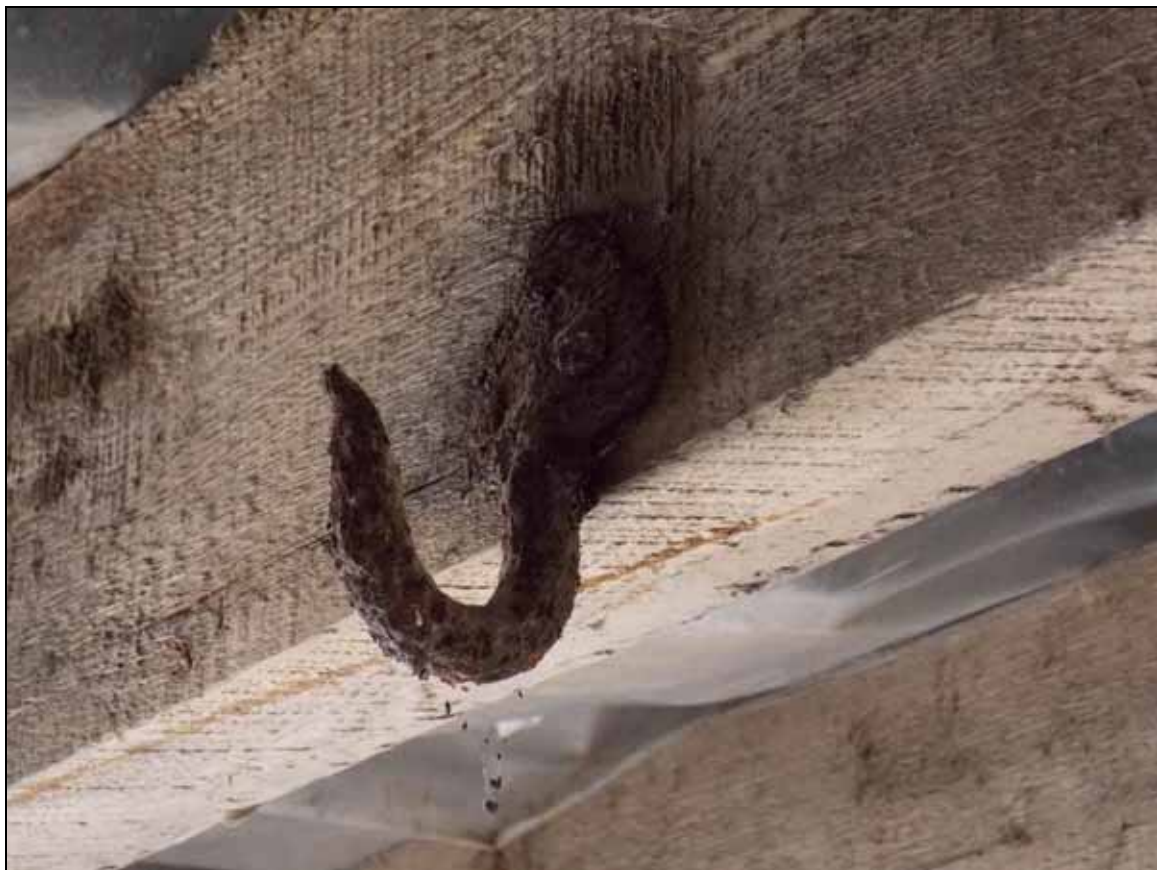
Plate 29: Detail of iron hook, looking north.
