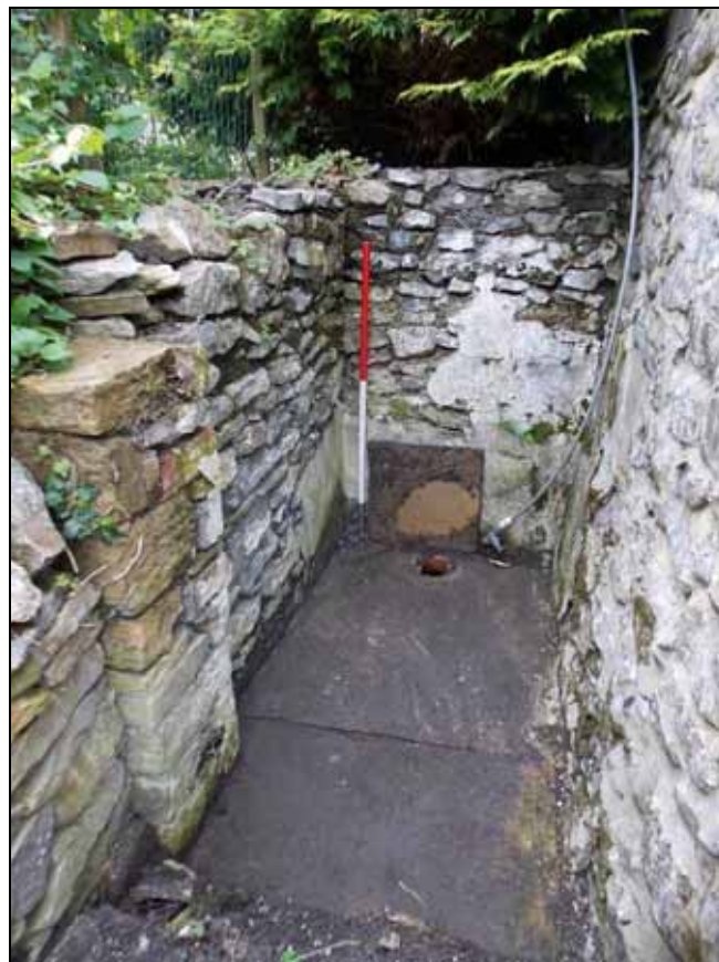
Plate 16: Flagstone floor with toilet drain following clearance (scale 1m).
