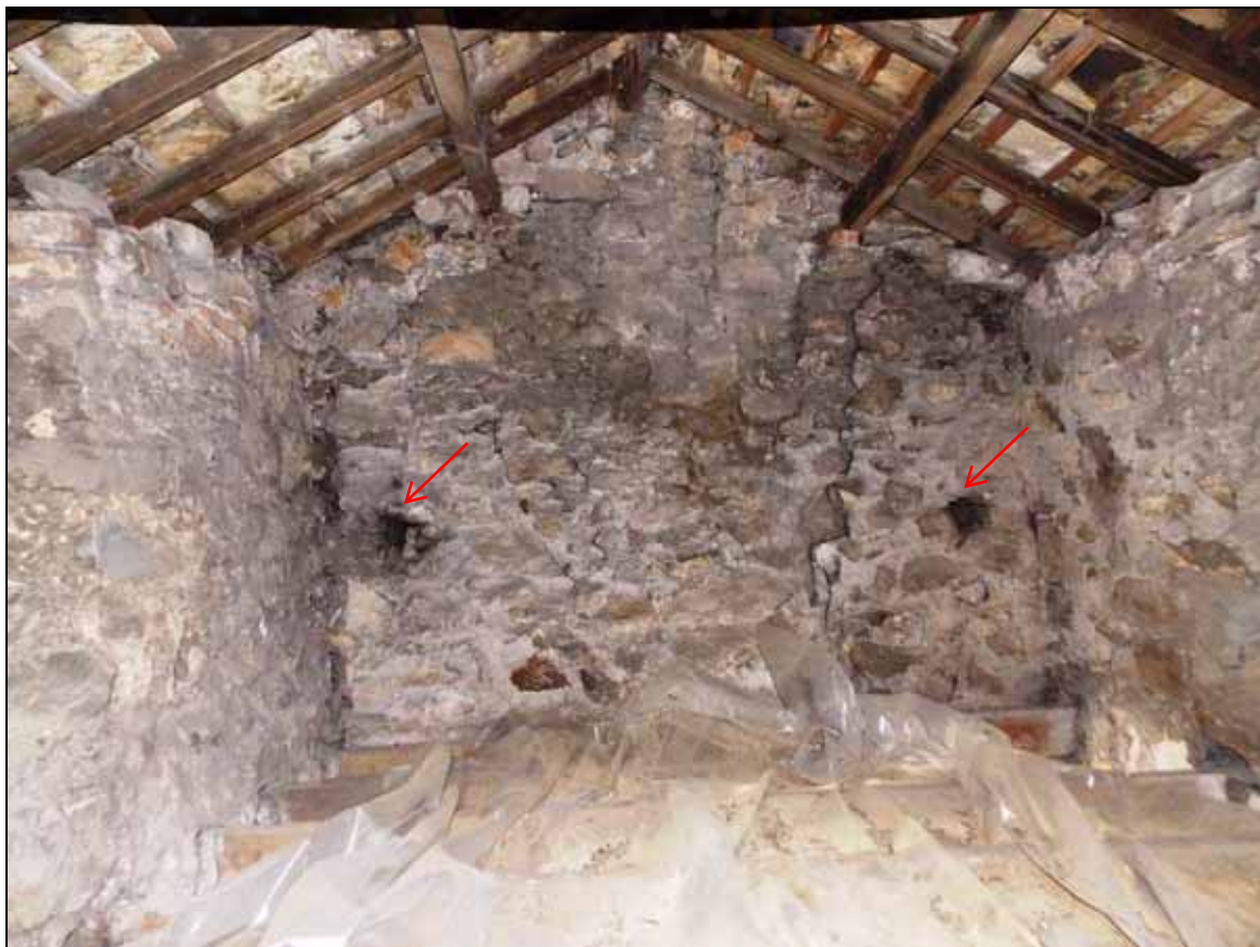
Plate 41: East wall of the loft with two deep slots (arrows).
