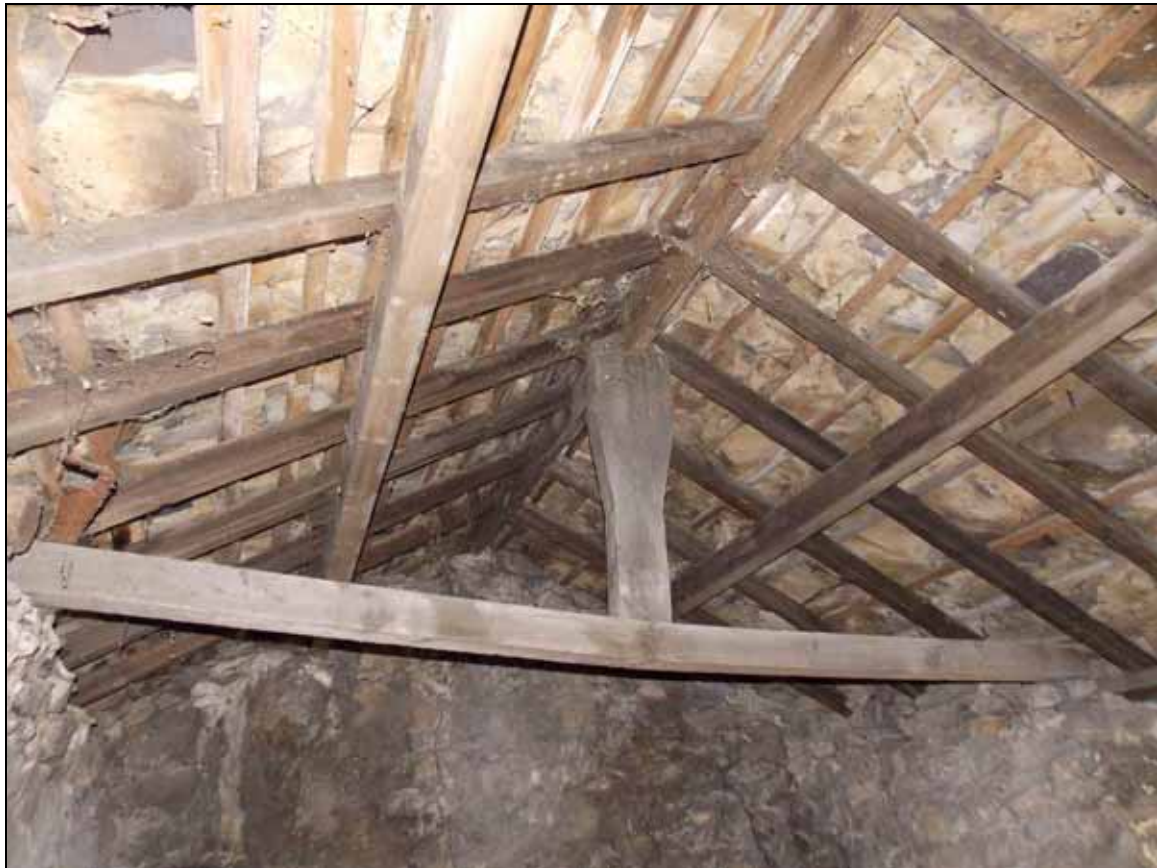
Plate 42: Roof structure, looking west.
