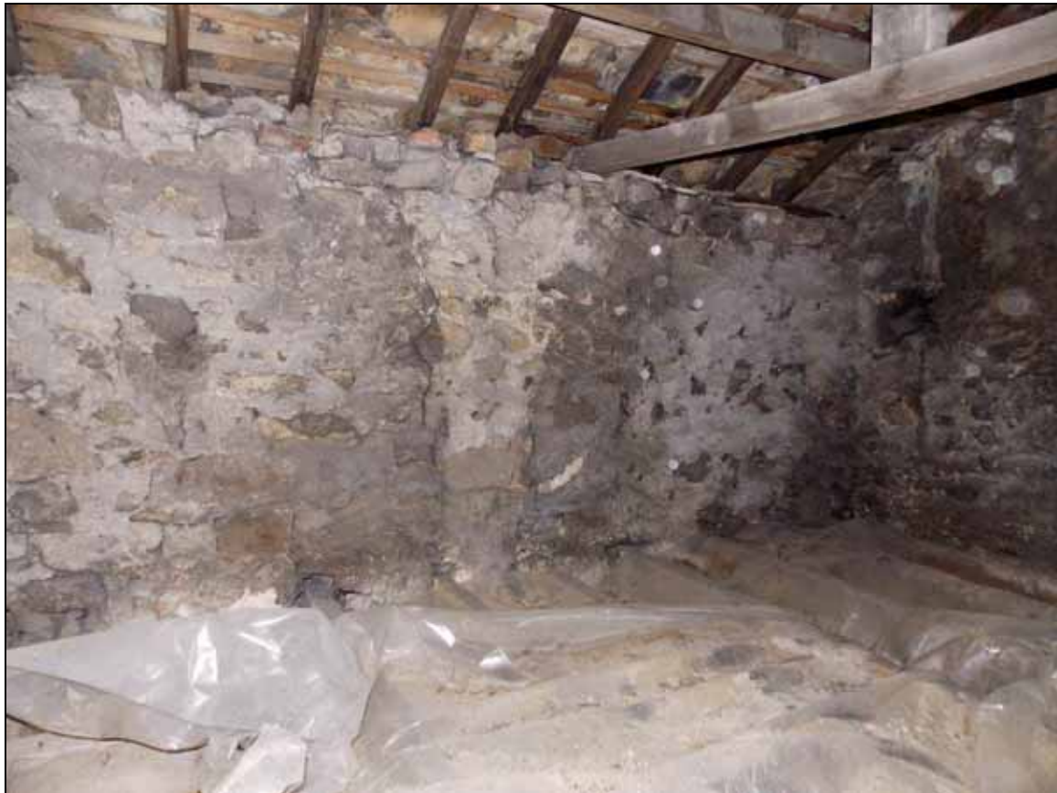
Plate 40: south wall of the loft, looking south-west.
