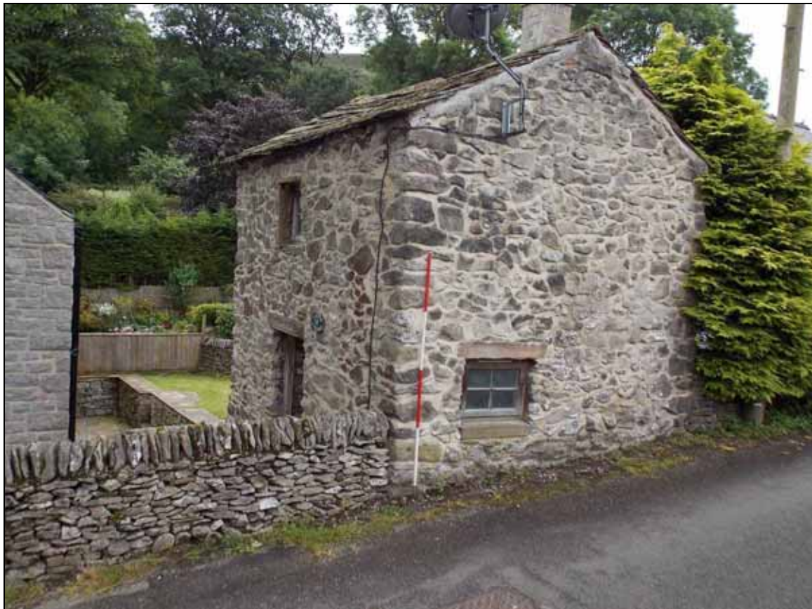
Plate 18: General view of the west elevation, looking south-east (scale 2m).
