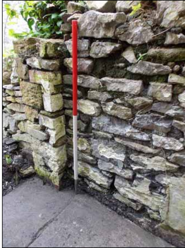
Plate 17: Rebate doorway jam of the toilet block, looking south-east (scale 1m).
