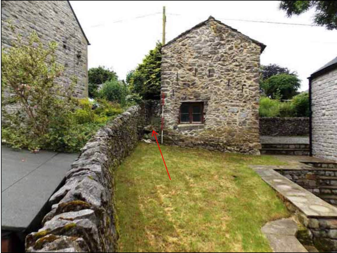
Plate 11: East elevation and remnants of toilet block (arrow) to the south (scale 2m).
