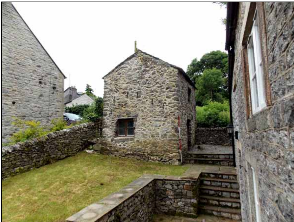
Plate 10: General view of the east elevation, looking south-west (scale 2m).
