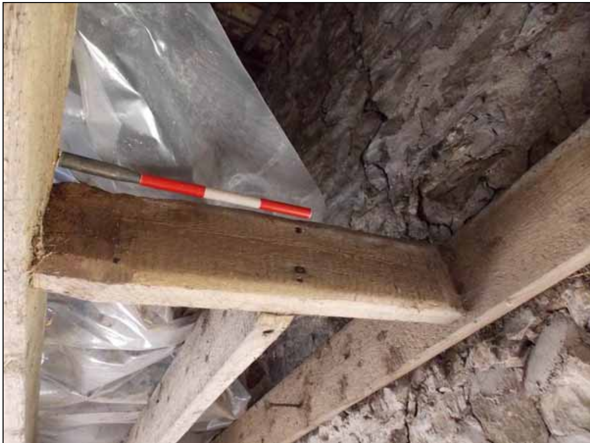
Plate 37: Detail of trimmer joist, looking north-east (scale 300mm).
