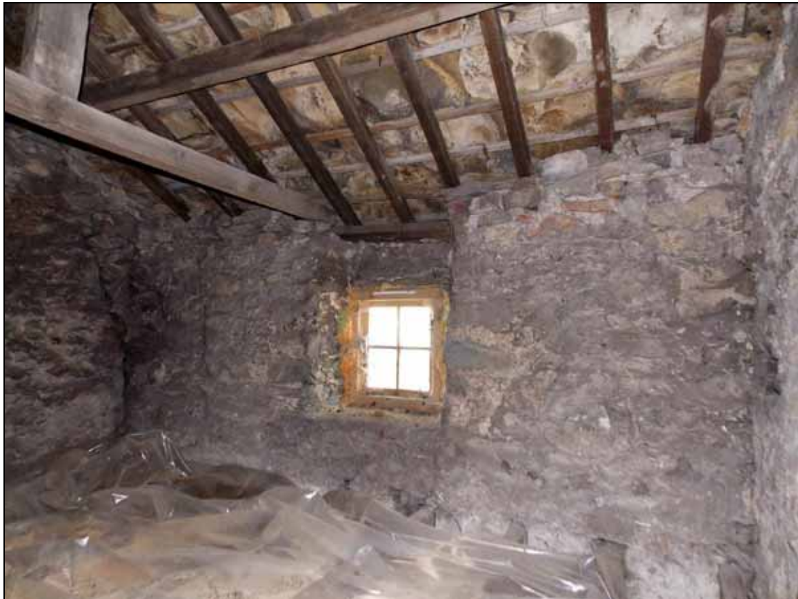
Plate 38: North wall of the loft storey with window opening, looking north-west.
