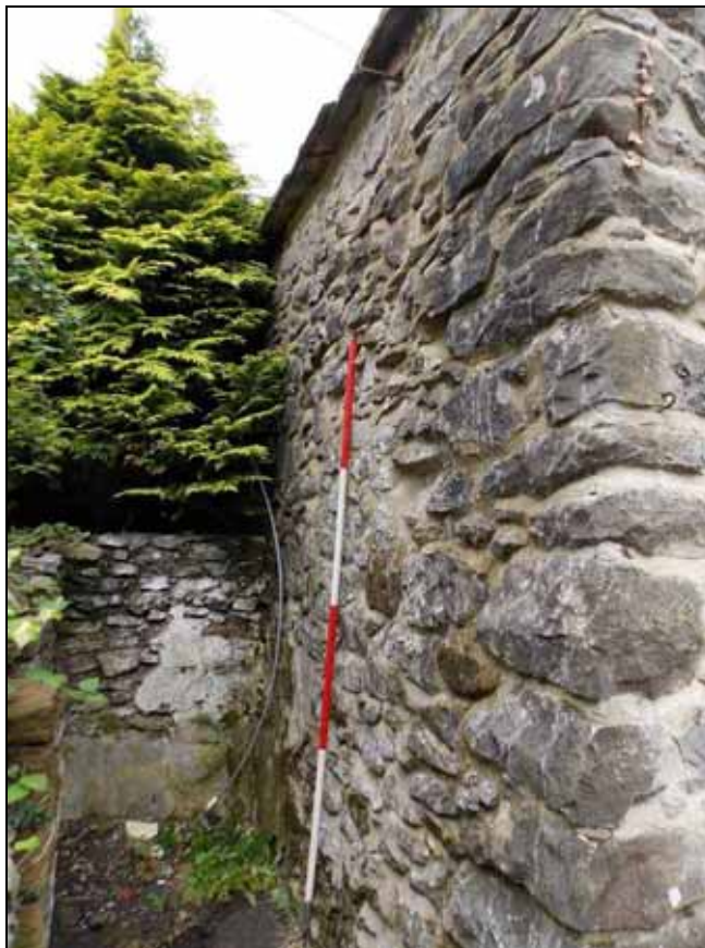
Plate 9: Short wall abutting the south elevation, looking west (scale 2m).
