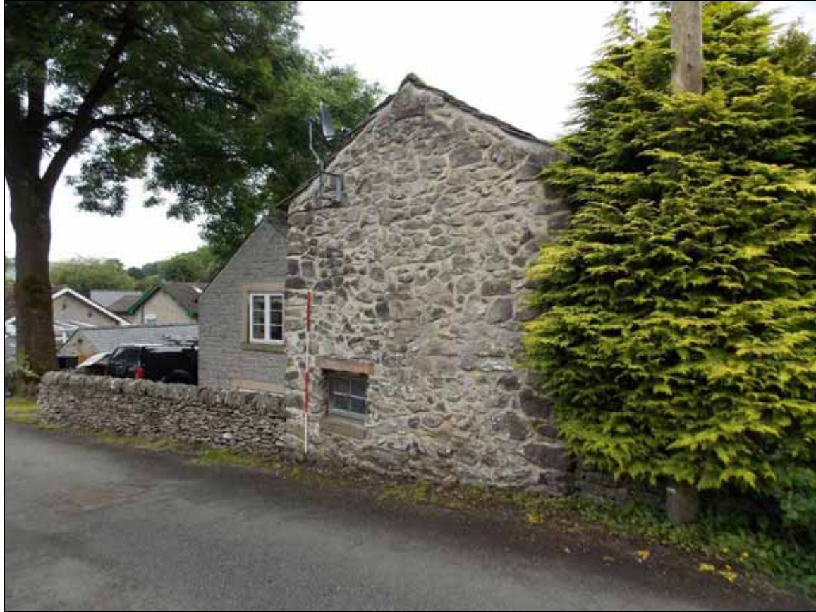
Plate 19: West elevation along Bessie Lane, looking north-east (scale 2m).
