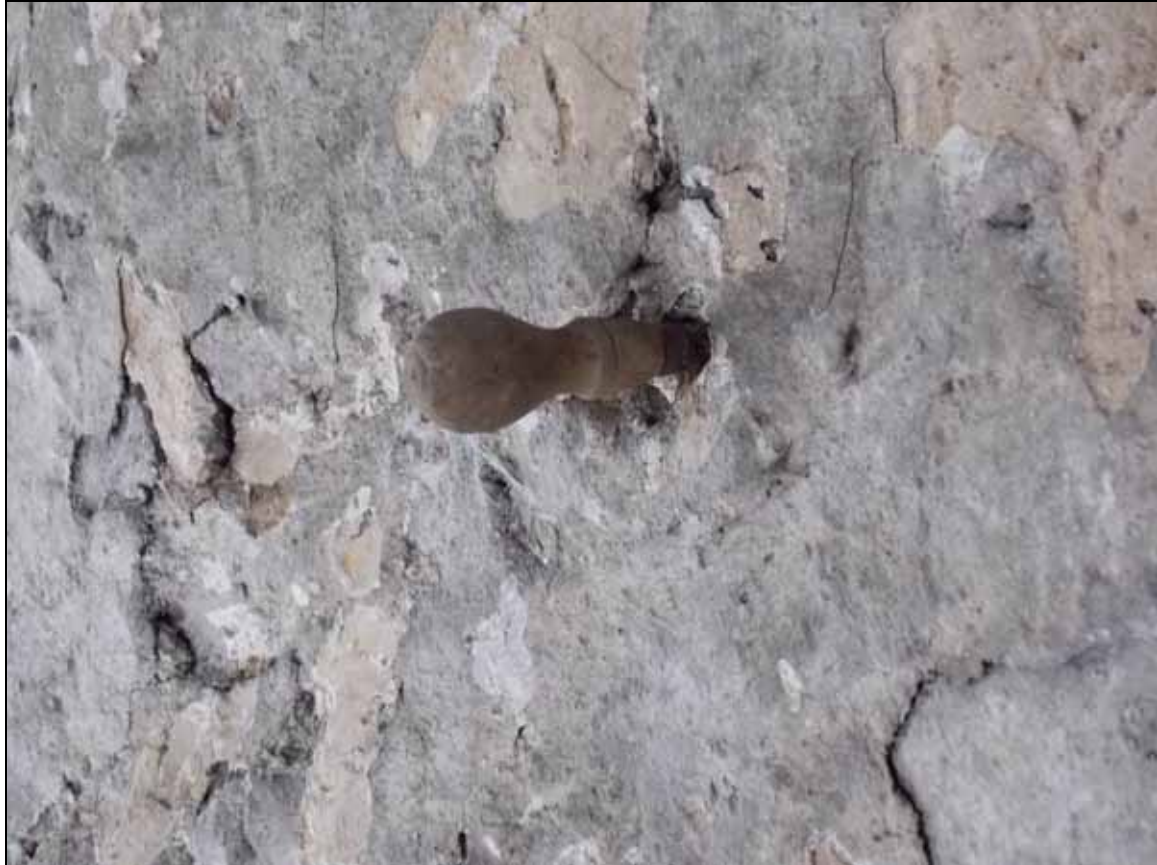
Plate 34: Detail of awl hole borer embedded in the south wall, looking south-east.
