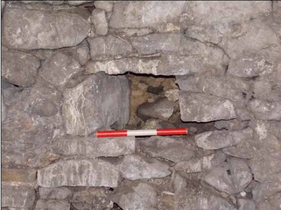
Plate 32: Detail of the lower niche within the south wall (scale 300mm).
