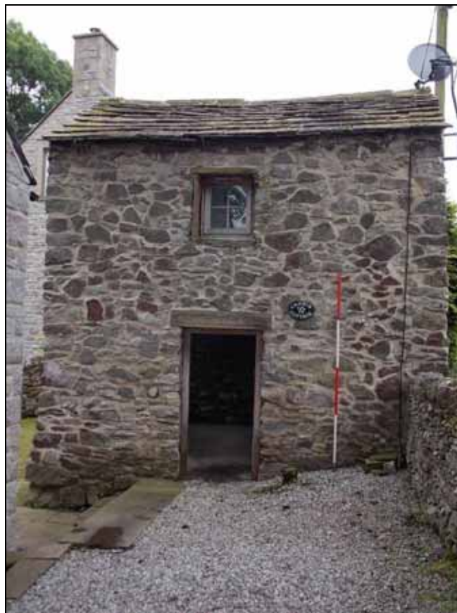
Plate 4: North elevation of Cannon Cottage (scale 2m).
