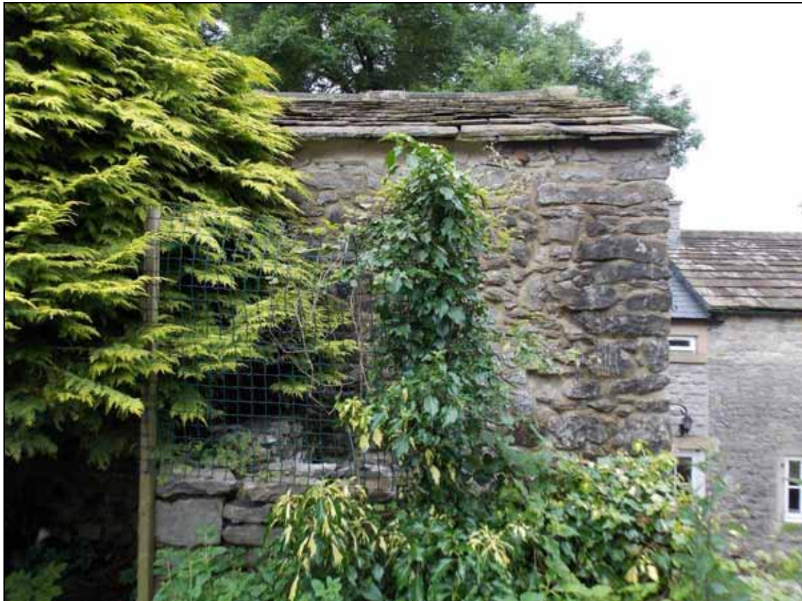
Plate 7: General view of the south elevation.
