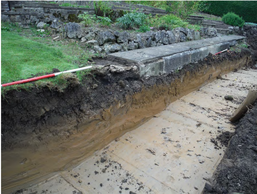
Figure 3. Excavated area with lawn and terraced garden in background.
