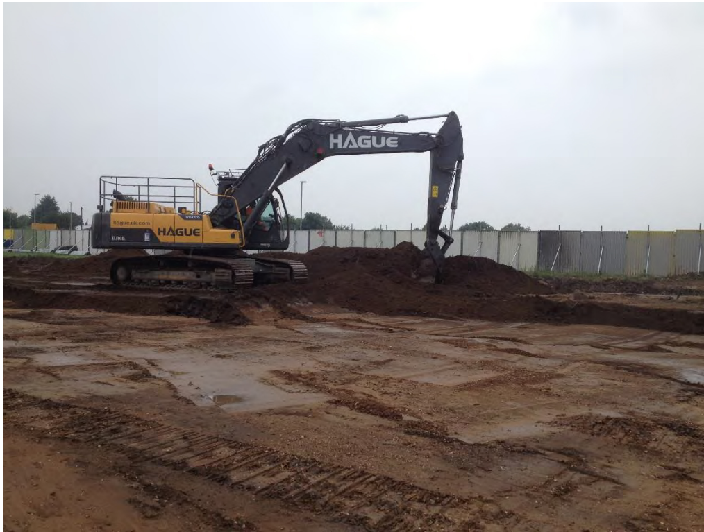
Figure 3. Working shot of topsoil stripping.
