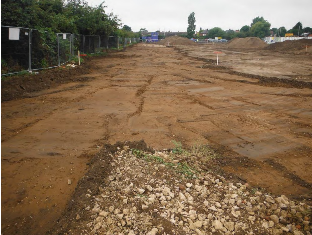
Figure 4. Stripped area along northern boundary of site.
