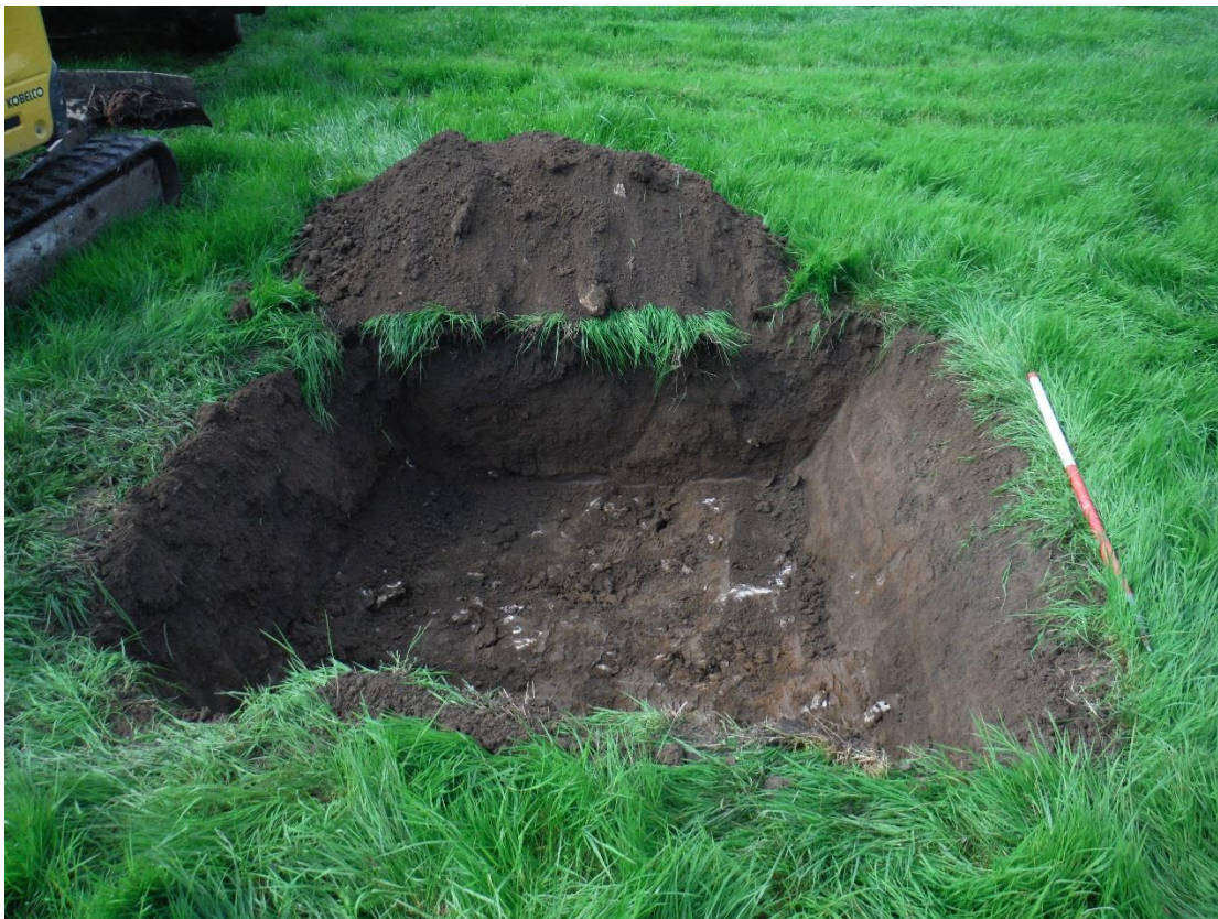
Figure 7. Small pit excavated for the installation of a septic tank.
