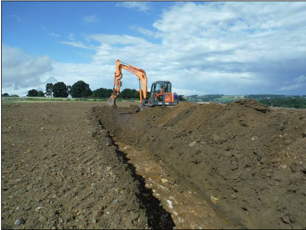
Figure 9. Excavation of the drainage trench.
